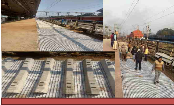
Lateral confinement of aggregates by PP Biaxial Geogrid for pavement and Track bed stabilization in Railway.
