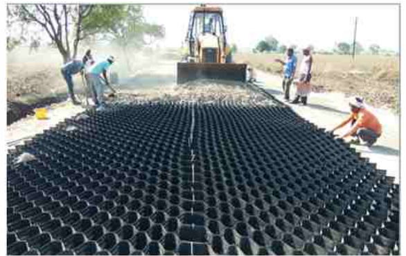
Consturction of Road with use of Geocell
