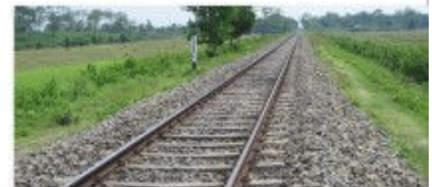
11 Condition of the track two years after rehabilitation (as on June 2008)
