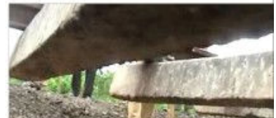
4 Removal of existing ballast from the trackbed
