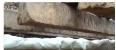
6 Laying of non-woven geotextile.
