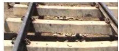
9 Placing ballast over the geogrid.
