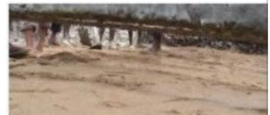
5 A thin layer compacted sand on the subgrade.
