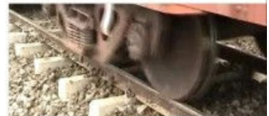
10 Train running over the rehabilitated track
