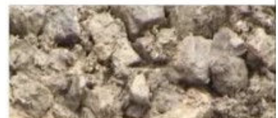
3 Ballast penetration into the subgrade
