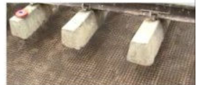
8 Laying TechGrid TGB-40 Knitted Polyester Biaxial Geogrid
