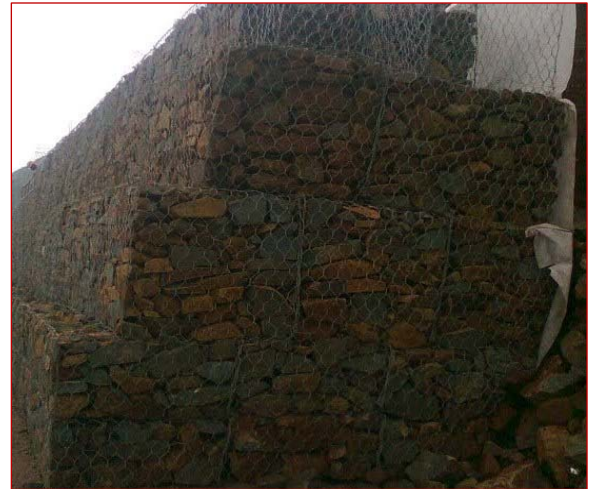
TechFab Metal Gabion Wall -Side View
