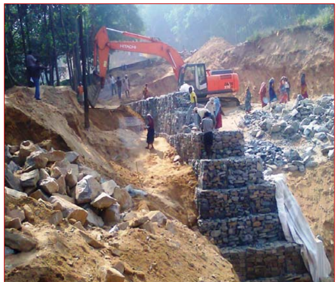
TechFab Metal Gabion Installation
