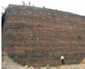
Fig.2: Geogrid RSW with Block
