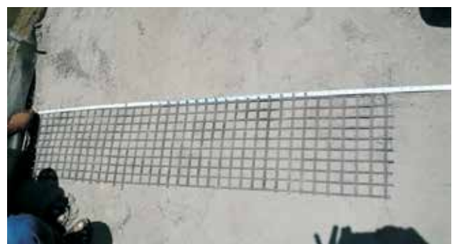
Fig.8: Details for field pullout test for RSW
