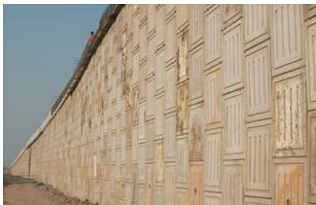
Fig.8: RSW for Nagpur Bypass with Fly ash
