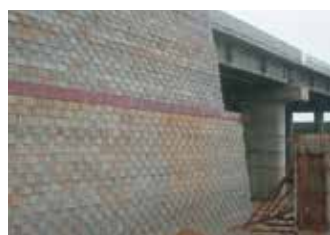
Fig.3: Geogrid RSW with welded wire mesh
