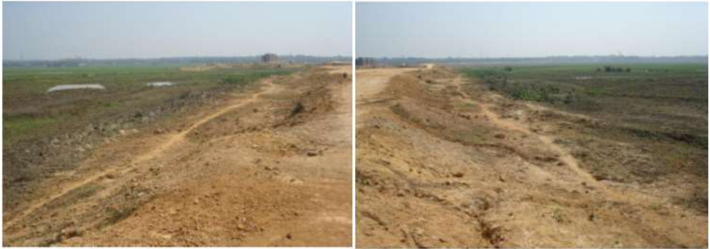
Figure 1. Left and Right side of the Embankment
