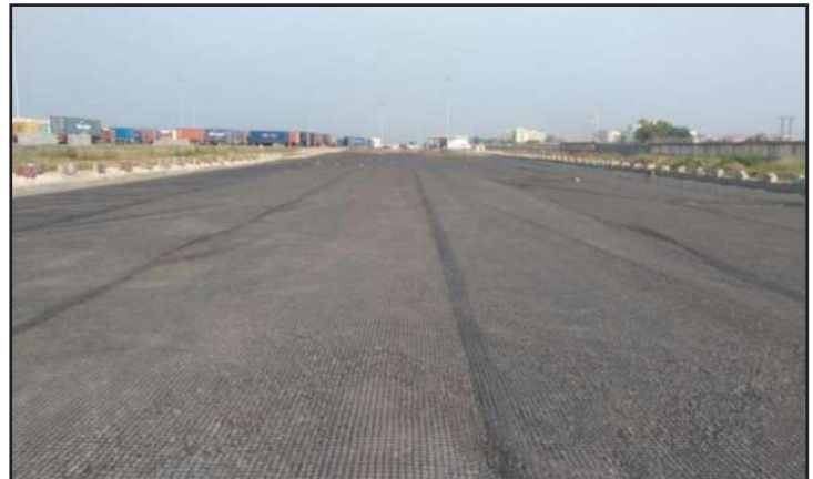
A layer of Techgrid PP Biaxial Geogrid was laid in JNPT, Navi Mumbai
