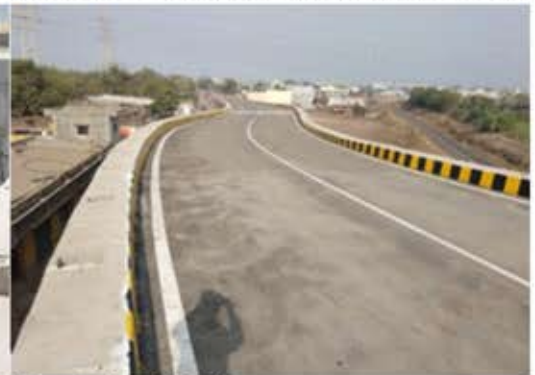
Completed RSW with TechStrap Polymeric Strip
