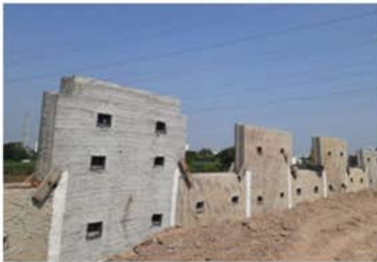
Erection of RCC Panel in progress
