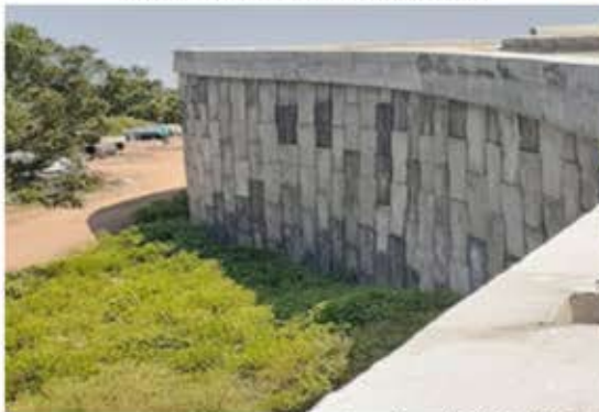
Completed RSW with TechStrap Polymeric Strip
