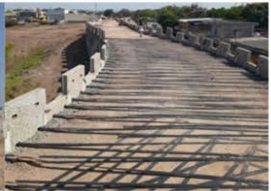
Installation of Techstrap polymeric strip in progress
