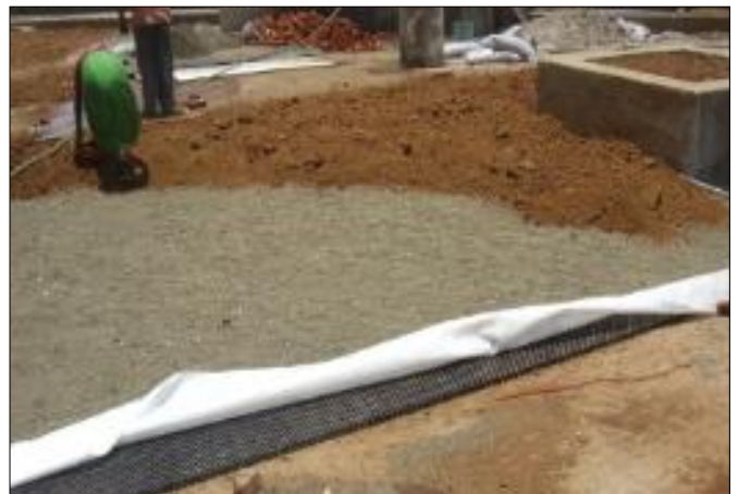
Fig 5 & 6 : Laying of Coarse Sweet Sand
