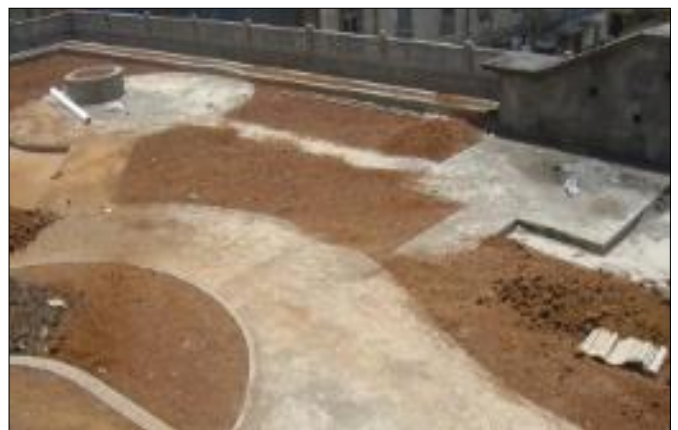
Fig 7 & 8 : Laying of Soil Planting Mixture
