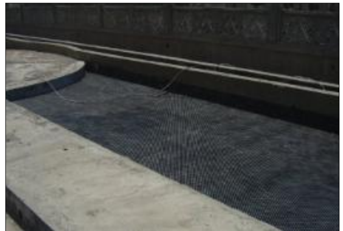
Fig 1 & 2 : Laying of Drain Board
