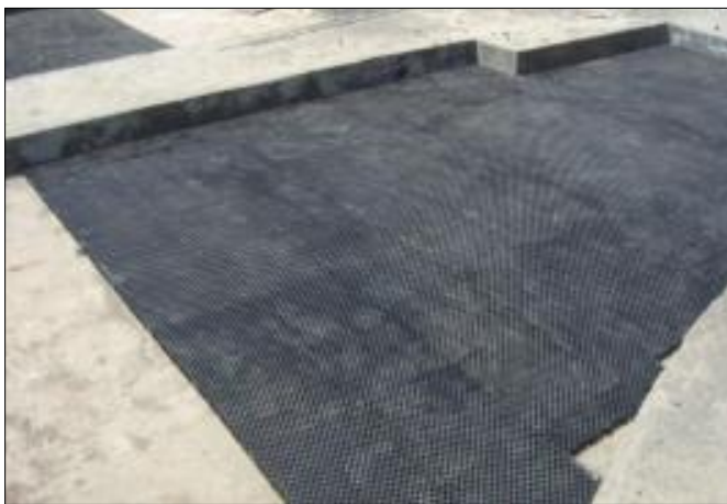
Fig 1 & 2 : Laying of Drain Board
