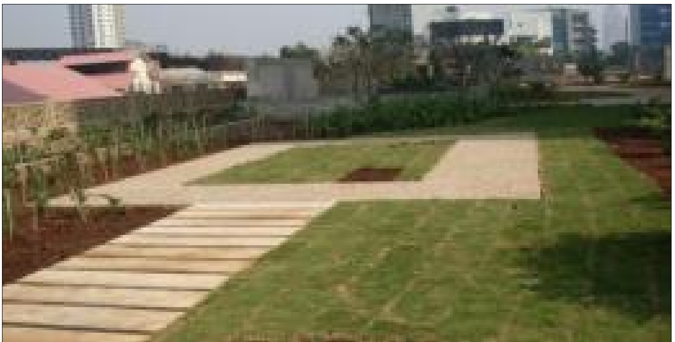
Fig 9 & 10 : completed Podium Garden / Landscape
