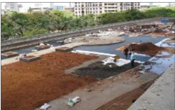
Fig 7 & 8 : Laying of Soil Planting Mixture
