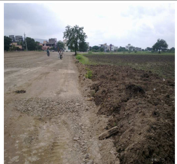
Subgrade Preparation (Stage-II)
