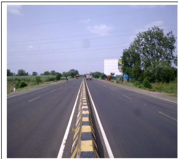
After Completion of Project
