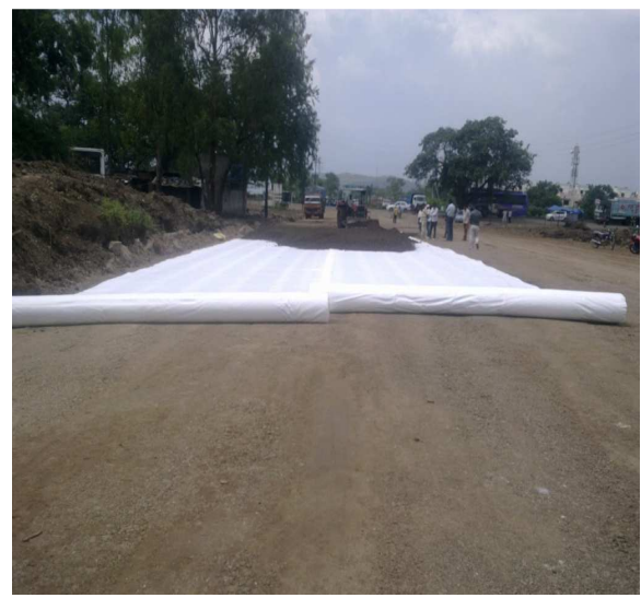
Placing of WMM Layer over PR-25
