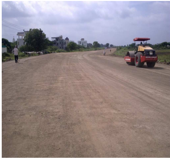
Subgrade Stabilization
