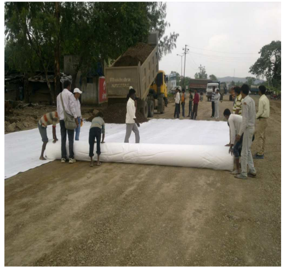
Laying of TFI PR-25
