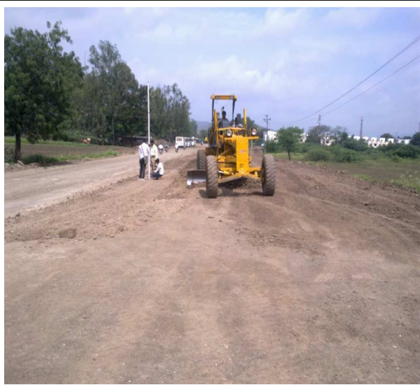
Subgrade Preparation (Stage-I)
