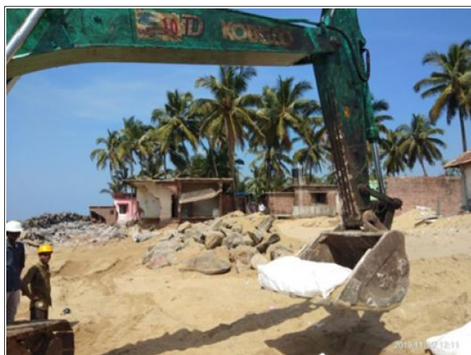
Dumping of Geotextile bags in progress
