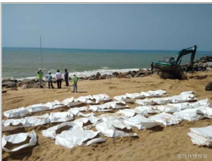
Filled Geotextile bags
