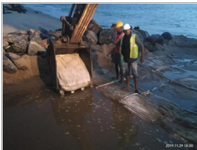
Laying of Geotextile bags in progress
