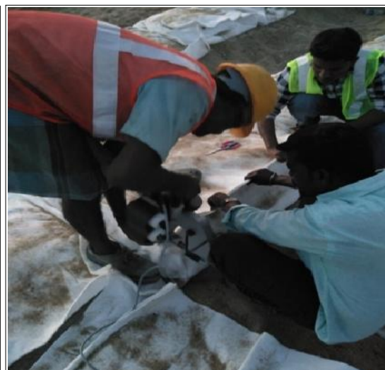
Stitching of geotextile bags by machine
