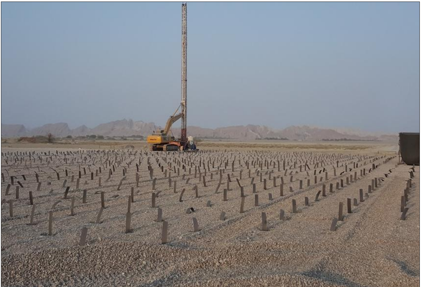
Photo 4 - TechDrain PVD installation is in progress
