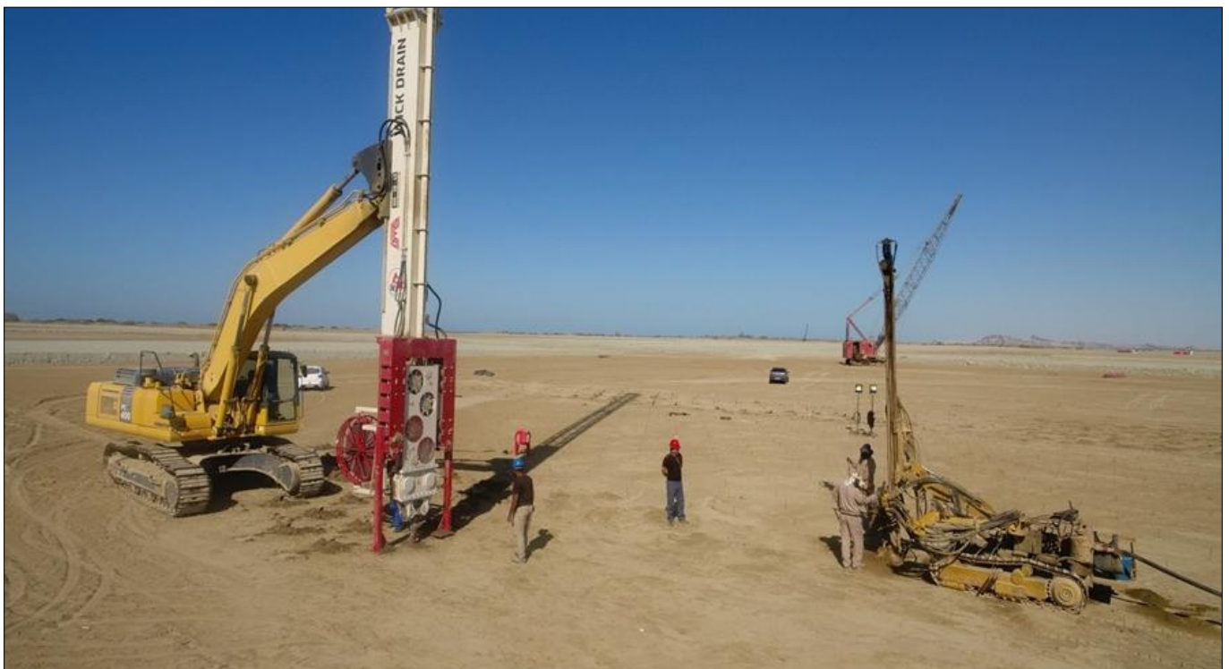
Photo 1 : TechDrain PVD installation starting at site
