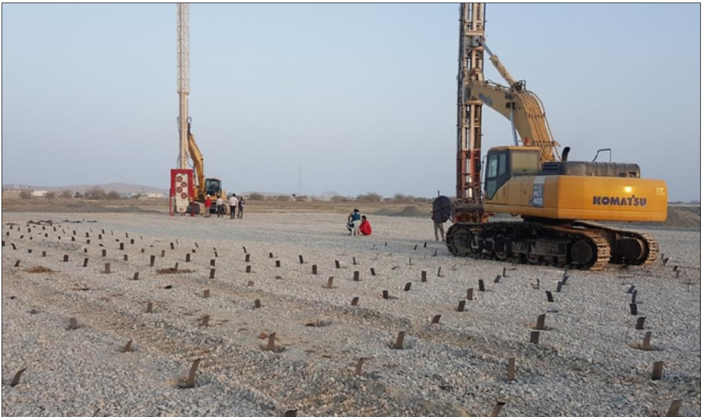
Photo 2&3 - TechDrain PVD installation is in progress
