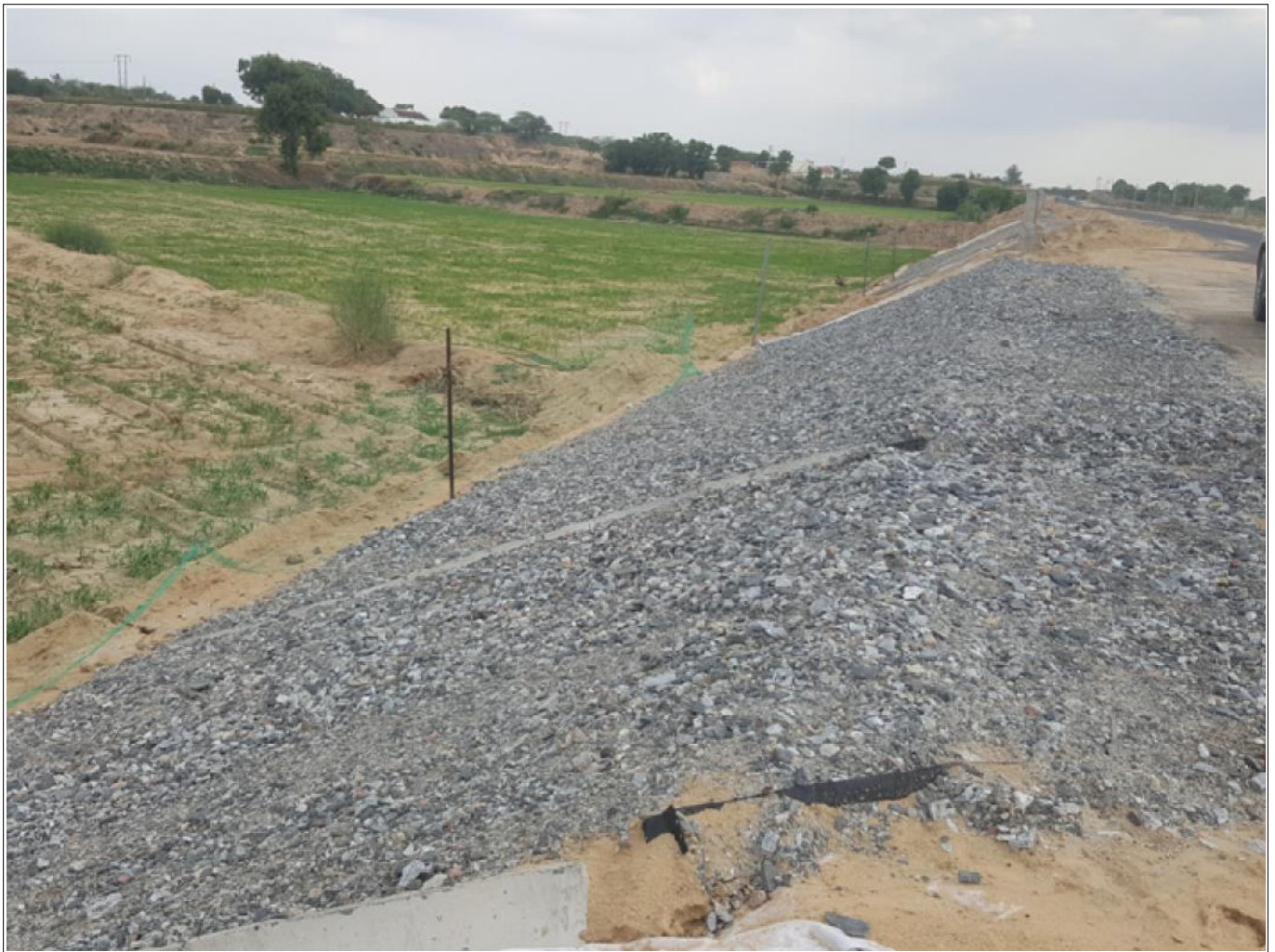
Slope is ready and filled with GSB
