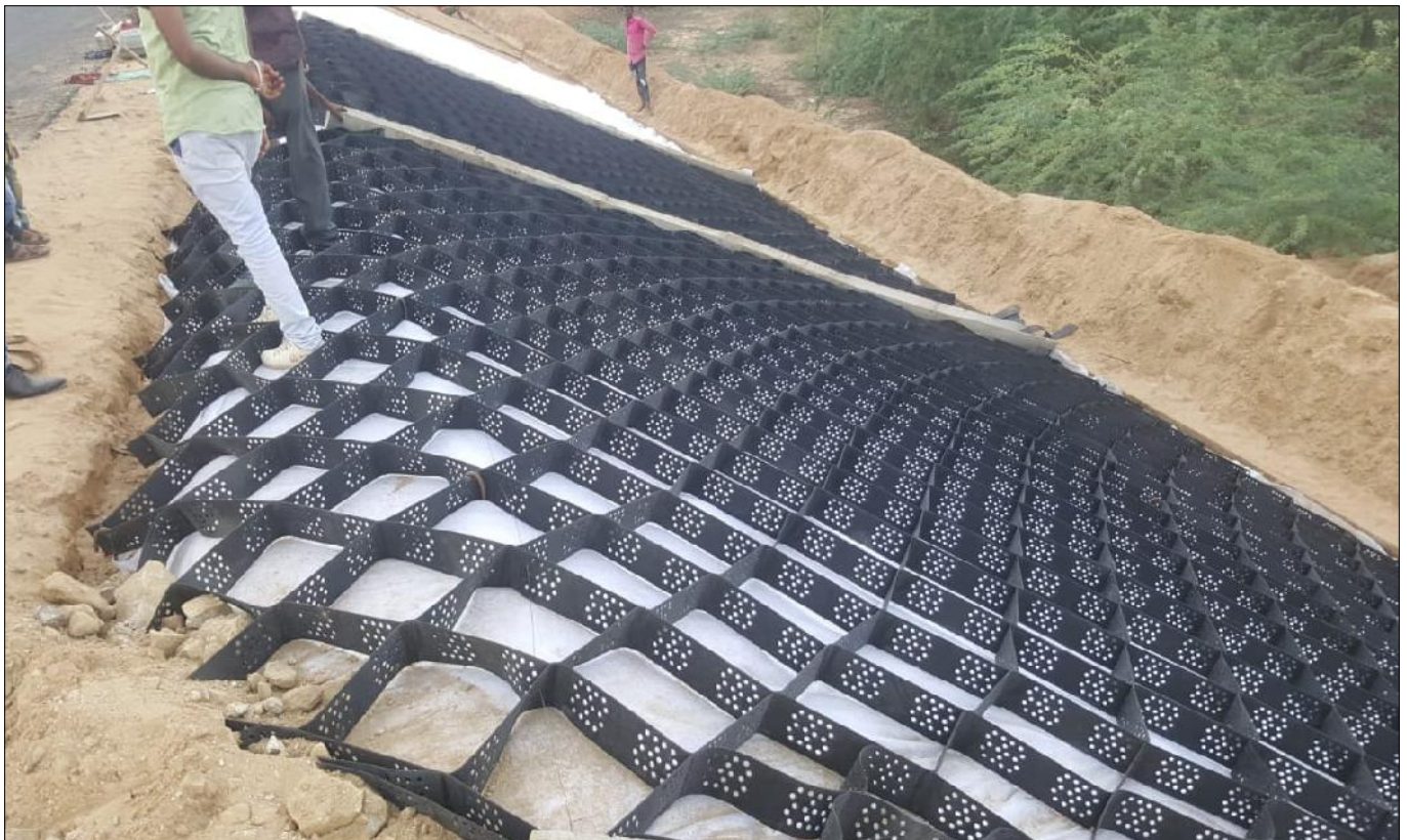
Installation of Geocell
