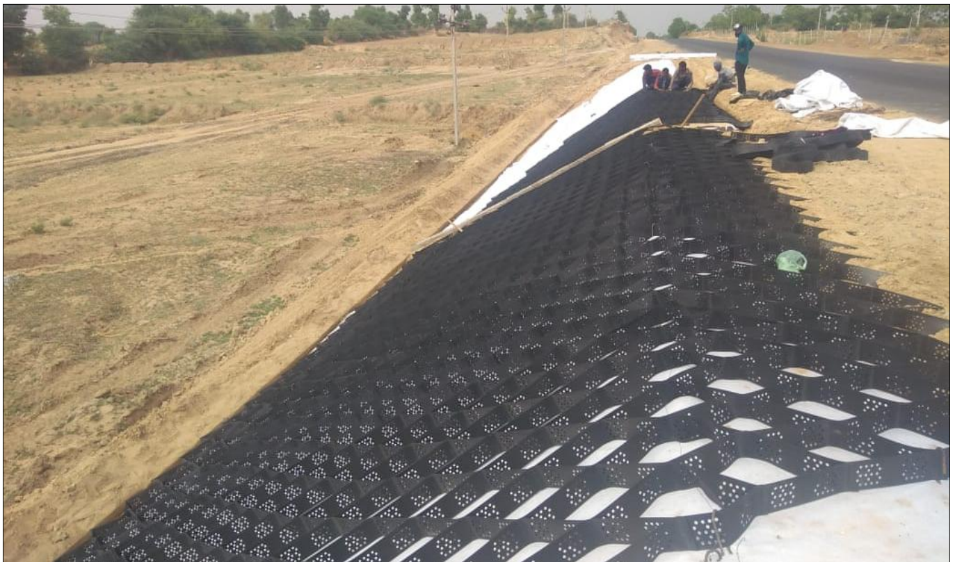
Installation of Geocell
