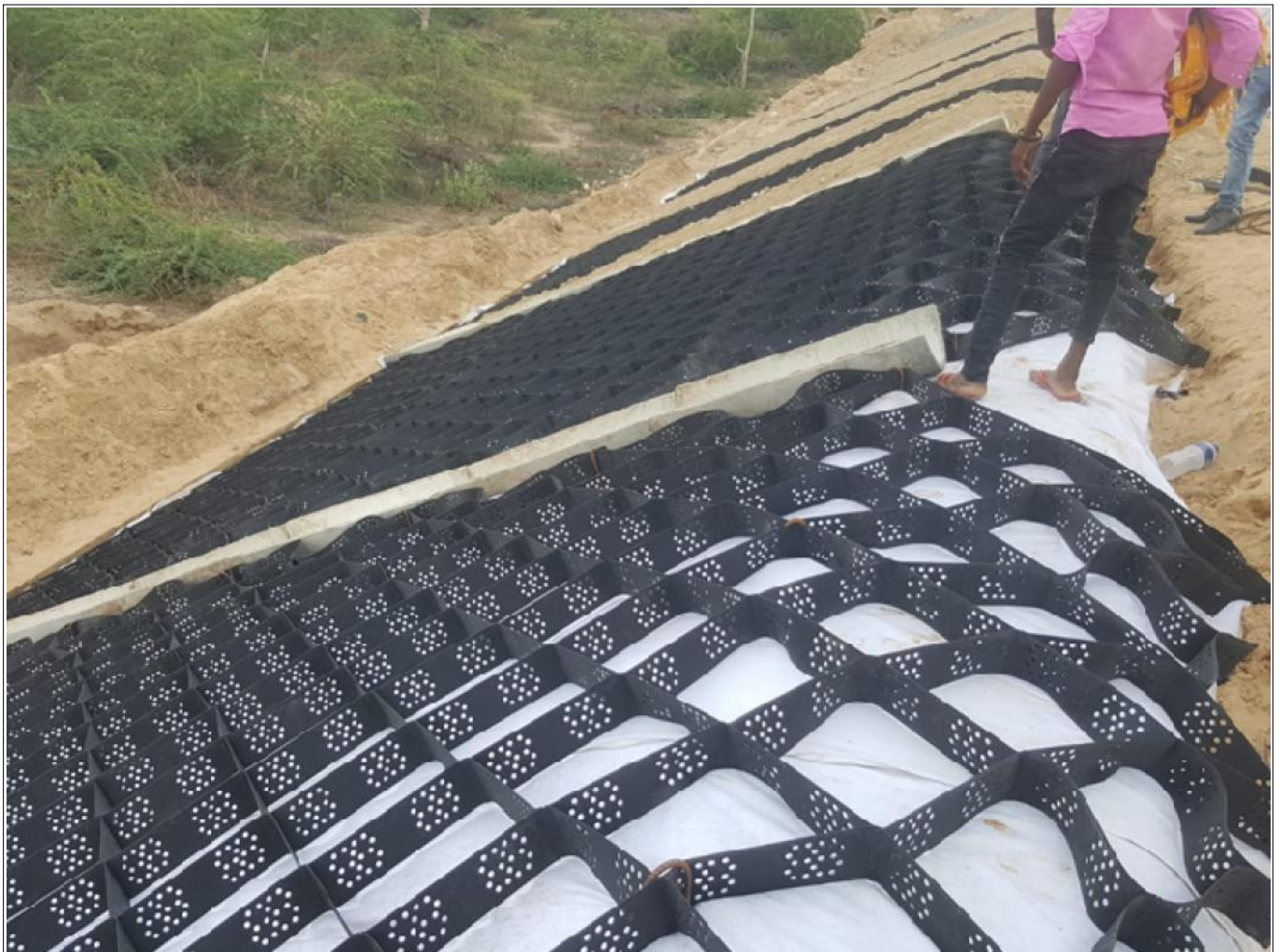
Installation of Nonwoven Geotextile & Geocell completed
