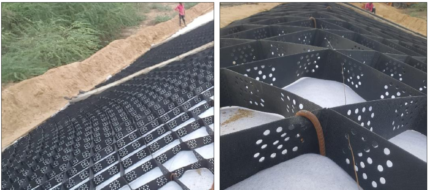
During Construction Photographs
