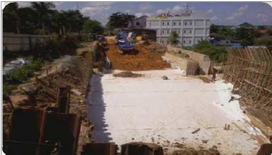
Installation of TGC Geotextile
