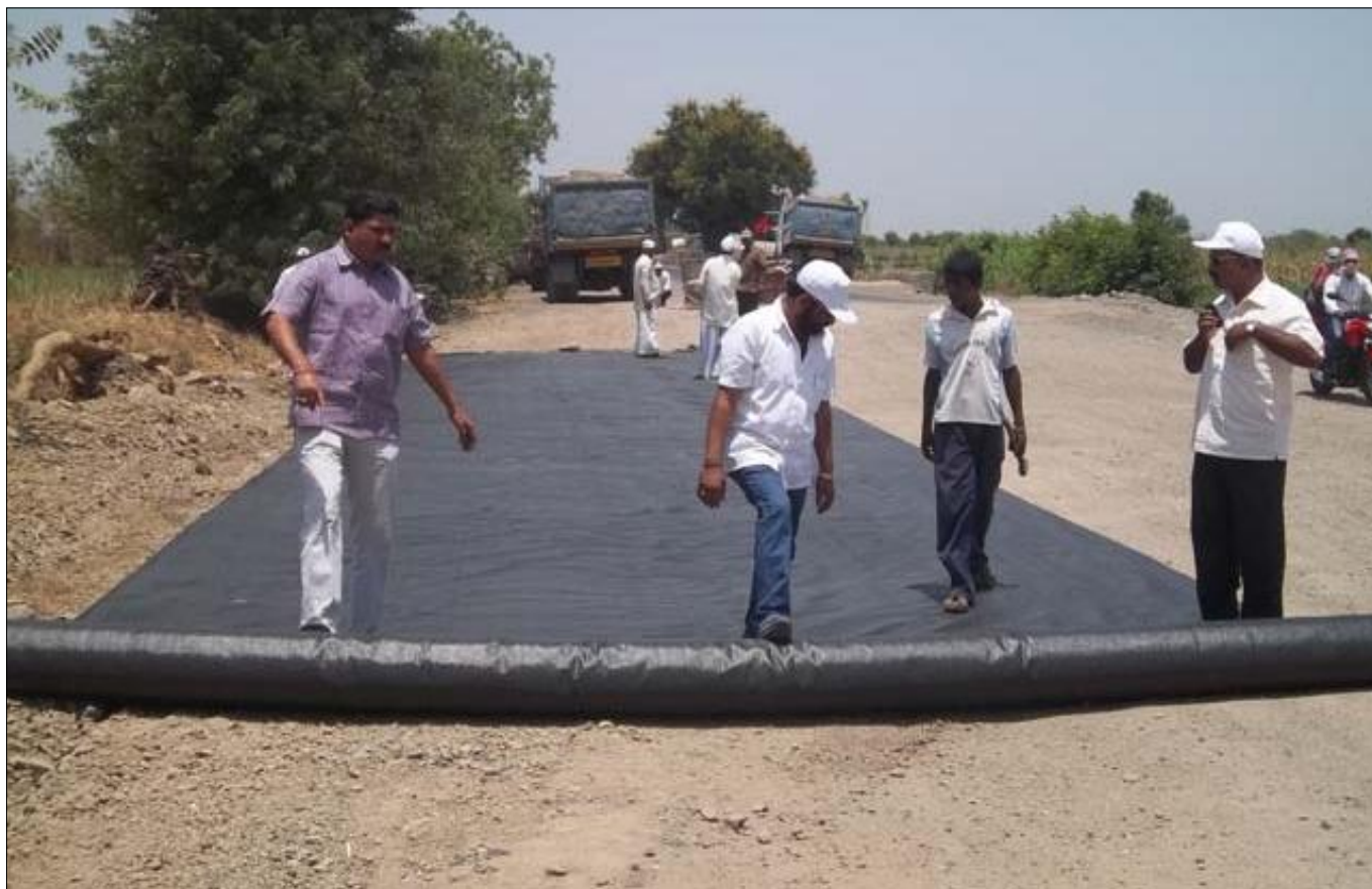
Laying of TFI-5300 at Subgrade
