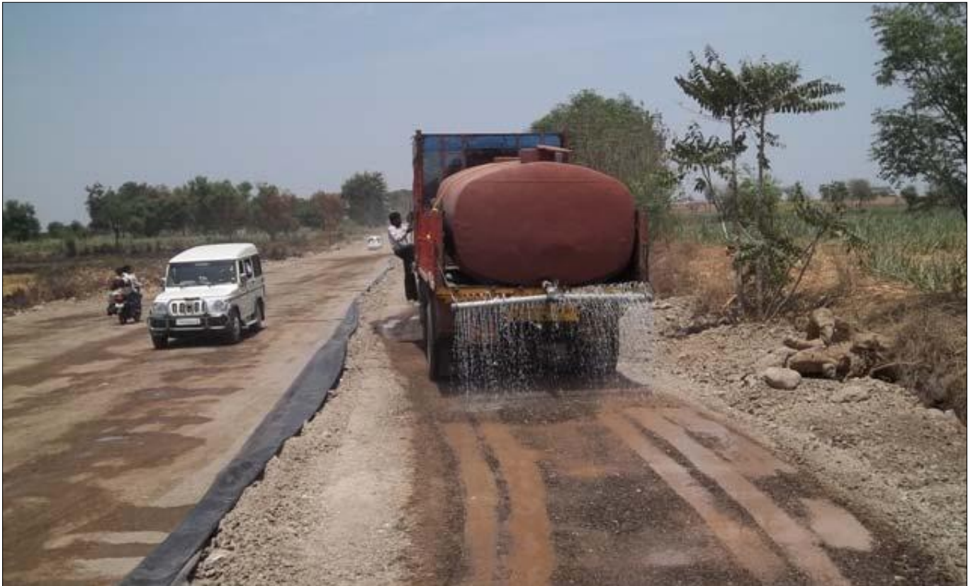
Sprinkling of Water & Compaction of Pavement
