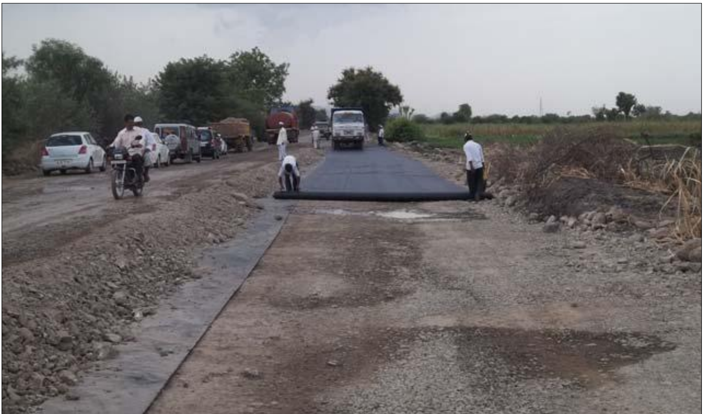
Unrolling TFI-5300 in 5m Widths
