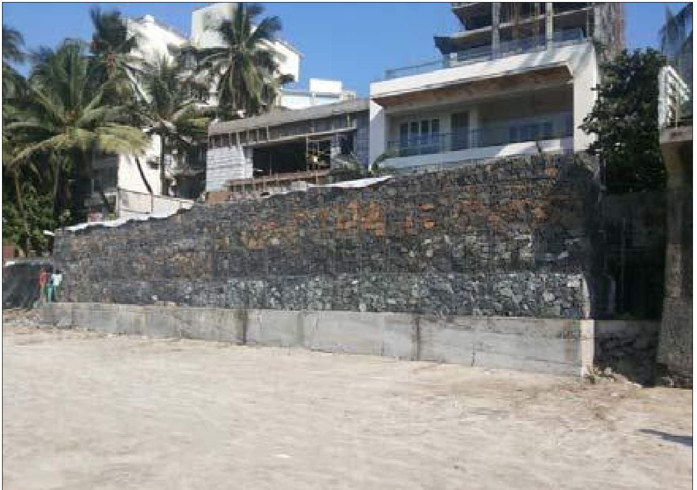
Photo 1 : TechFab Metal Gabion - Longitudinal view
