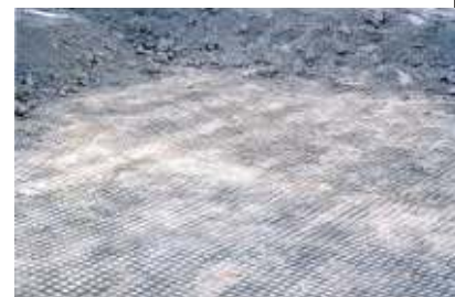
Laying down fill over Techgrid U-40 for Embankment
