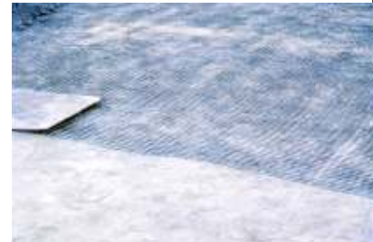
Laying of Techgrid U-40 as a basal reinforcement
