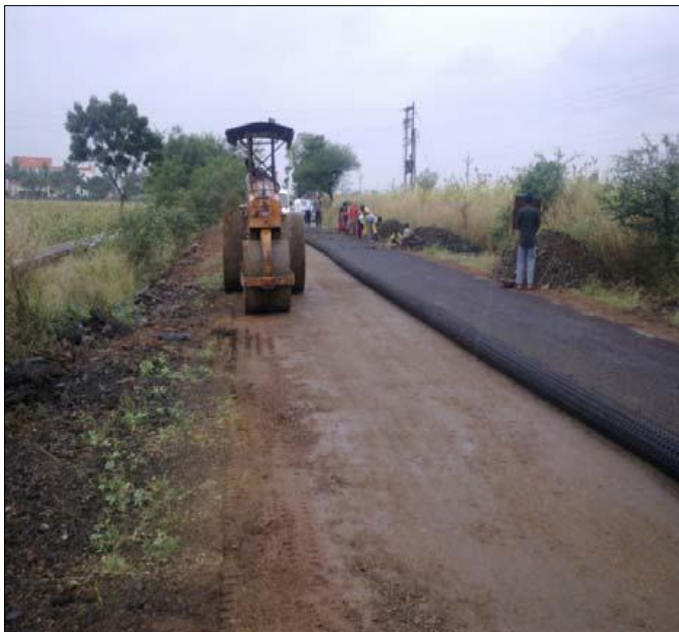
Compaction of Subgrade
