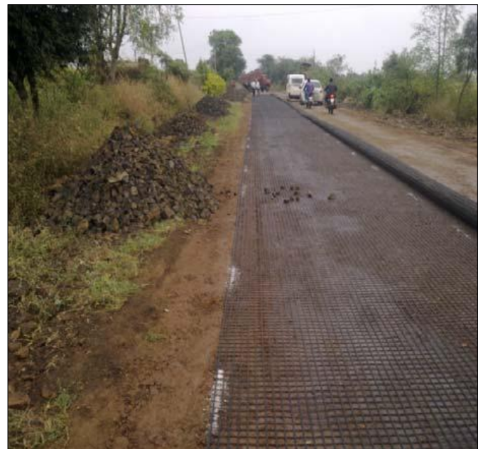
Laying of TGB-40
