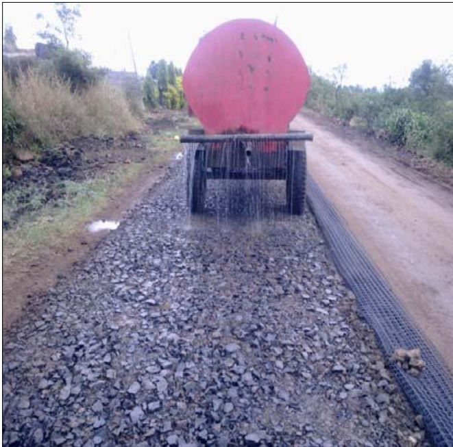
Watering on Compacted layer
