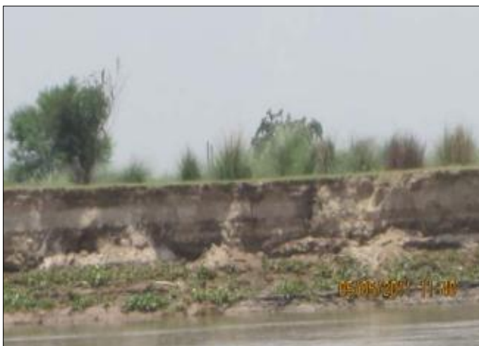
Before Rehabilitation – Churni River Bank
