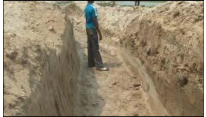
Excavation of Trench at the End
