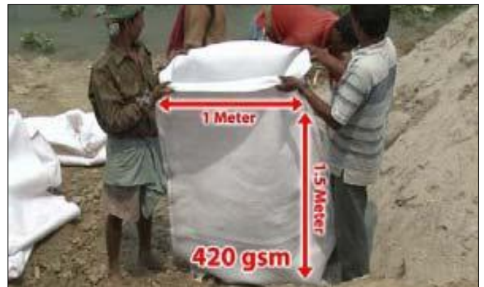
TechGeo Nonwoven Geotextile Bag Being Filled with Local
