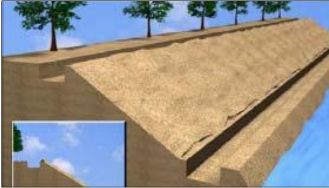
Dressing of the Embankment Slope
