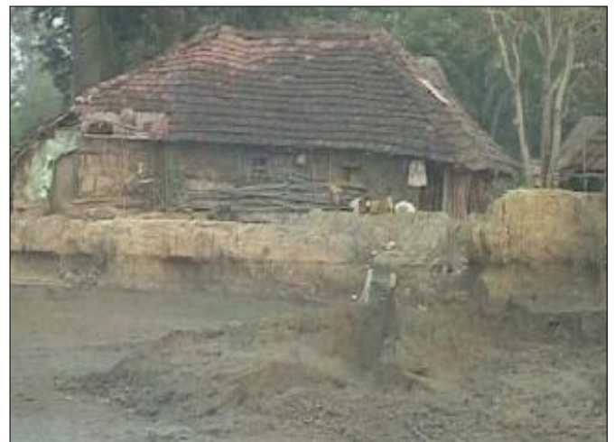
Before Rehabilitation – Churni River Bank
