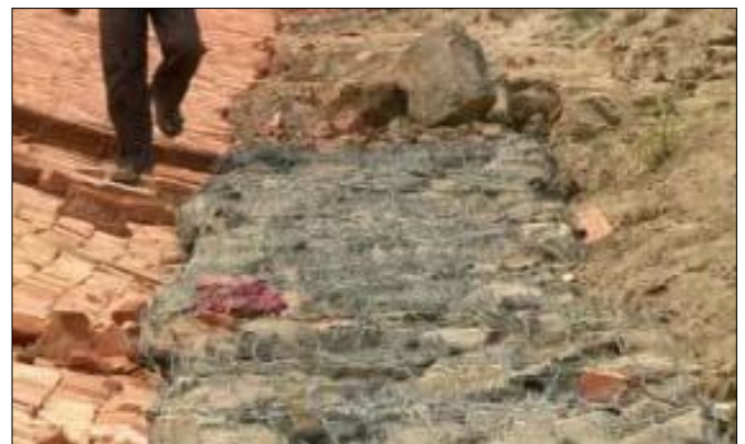
Metal Gabion Placed at Bottom Trench
