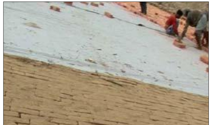
Unrolling of TechGeo Nonwoven Geotextile
