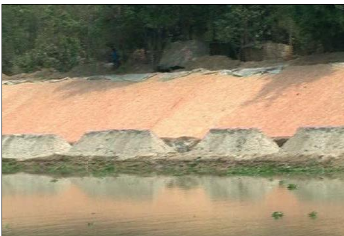
After Rehabilitation – Churni River Bank
