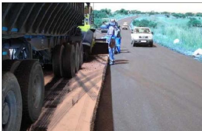
Asphalt Overlay over TechGlass AIC 50
