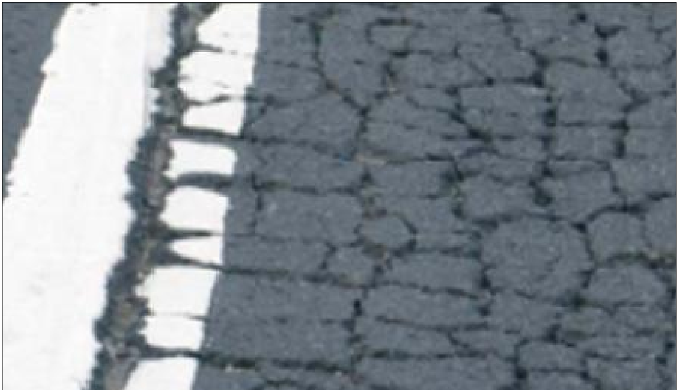
Initial Condition of Road
