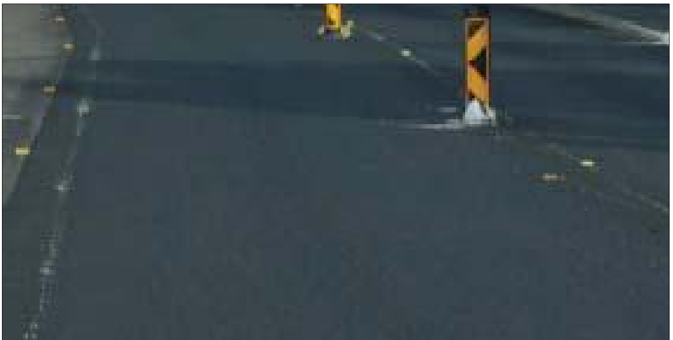
Road Condition – After 4 Months
