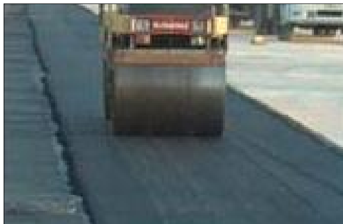
Asphalt Compaction with Roller
