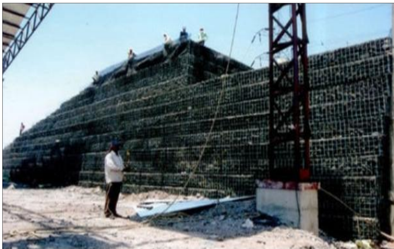
During construction photograph
