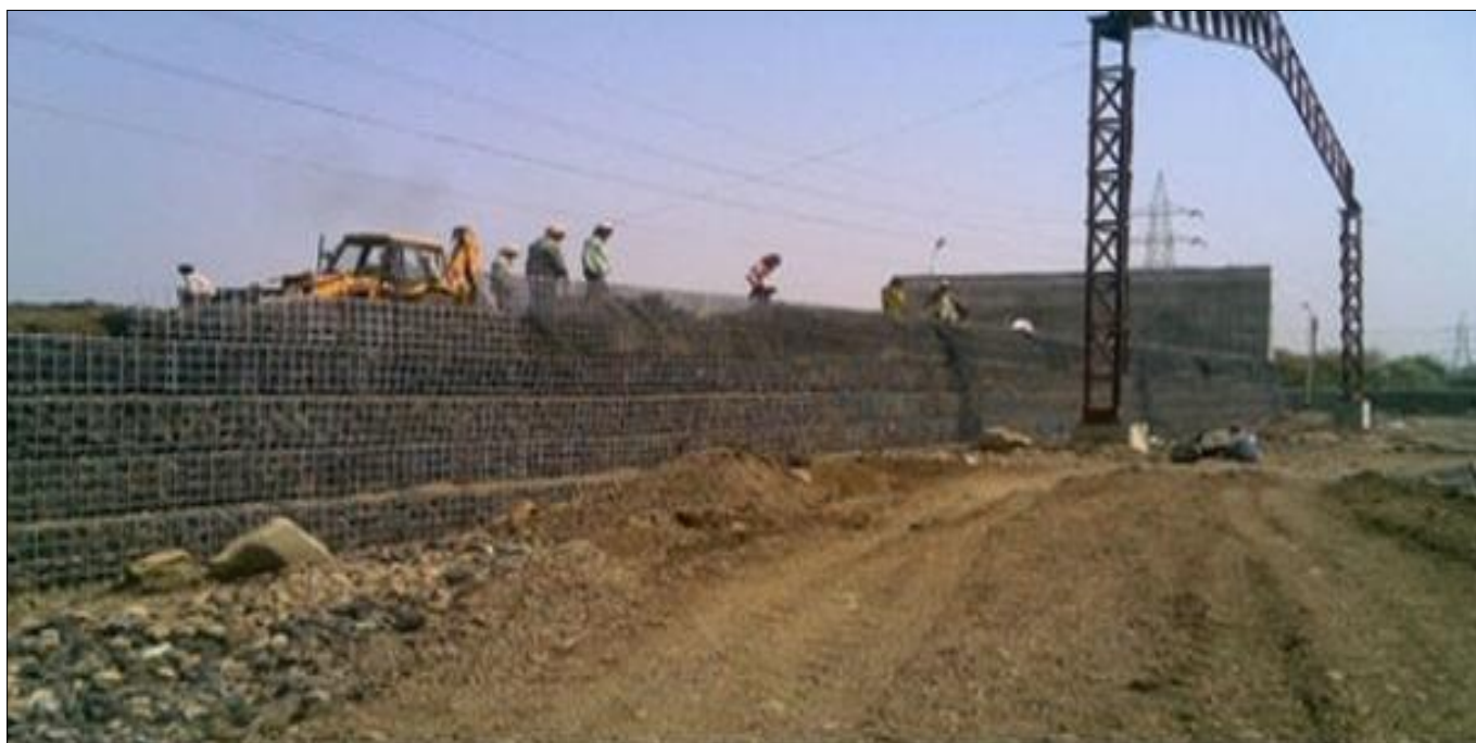
During Construction Photograph
