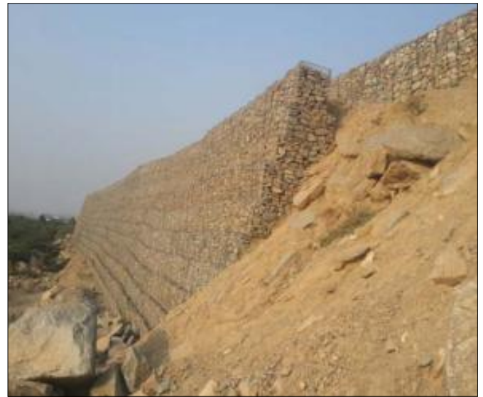
Construction Stage - II
