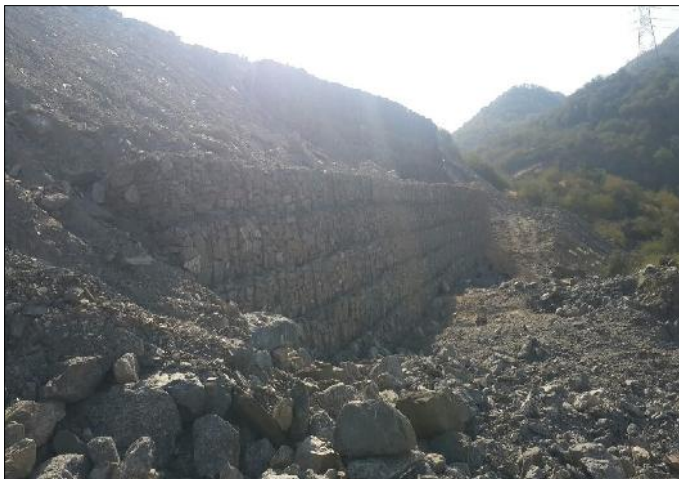
TechFab Metal Gabion - Initial Stage
