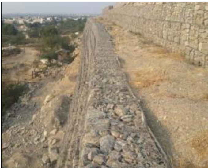
Two Tier Wall – Longitudinal View
