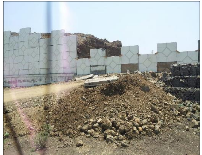
TechFab Reinforced soil wall - Installation
