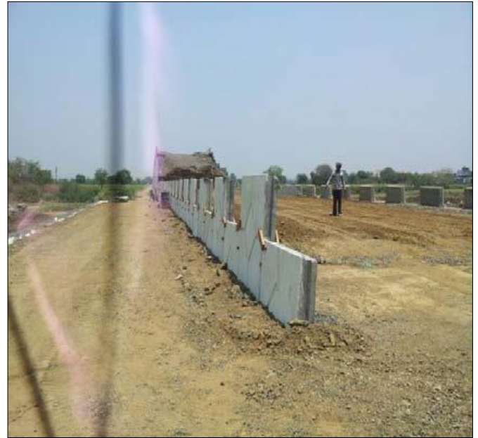
TechFab Reinforced soil wall
