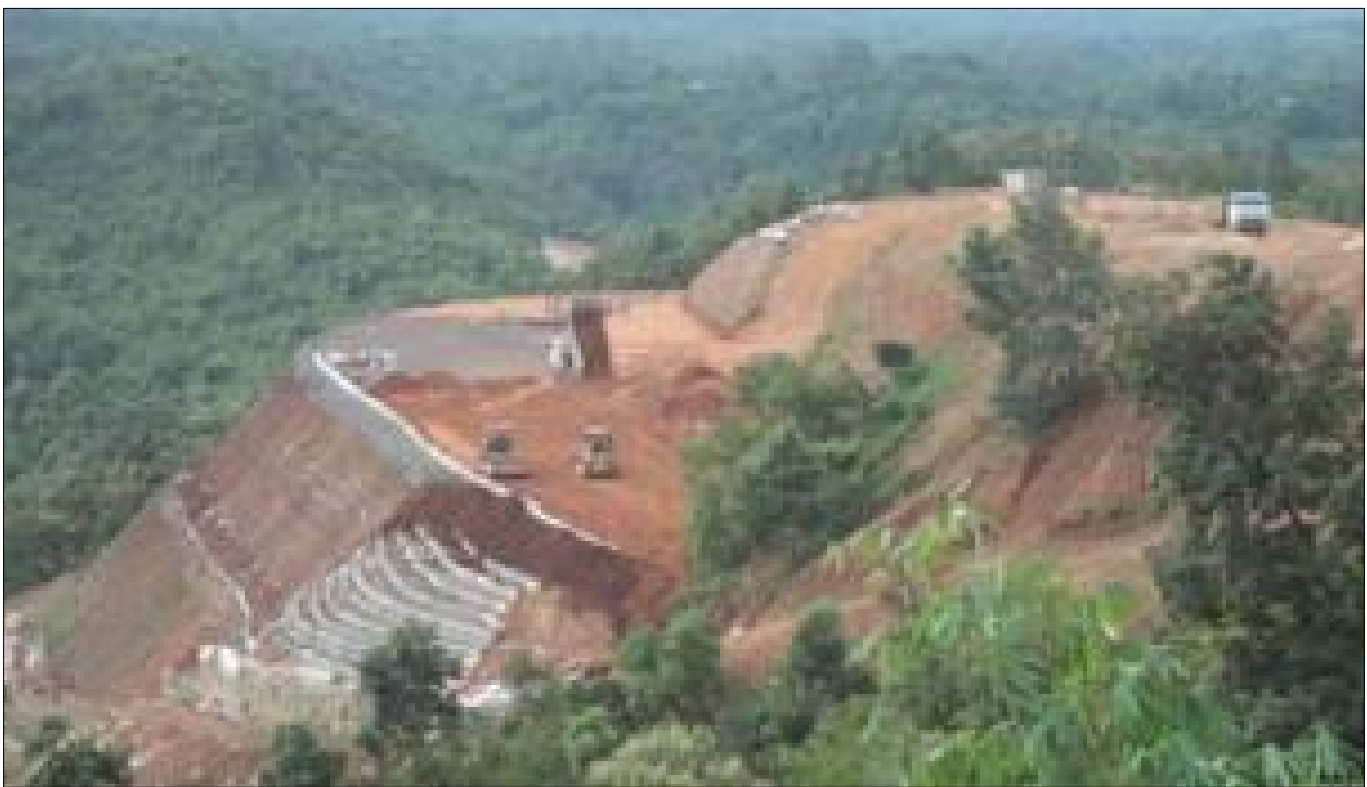
RSS with TechGrid GeoGrid – Under Construction
