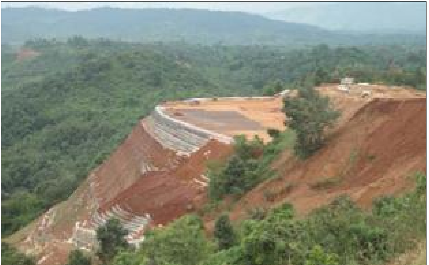
Pre Final Stage of Construction
