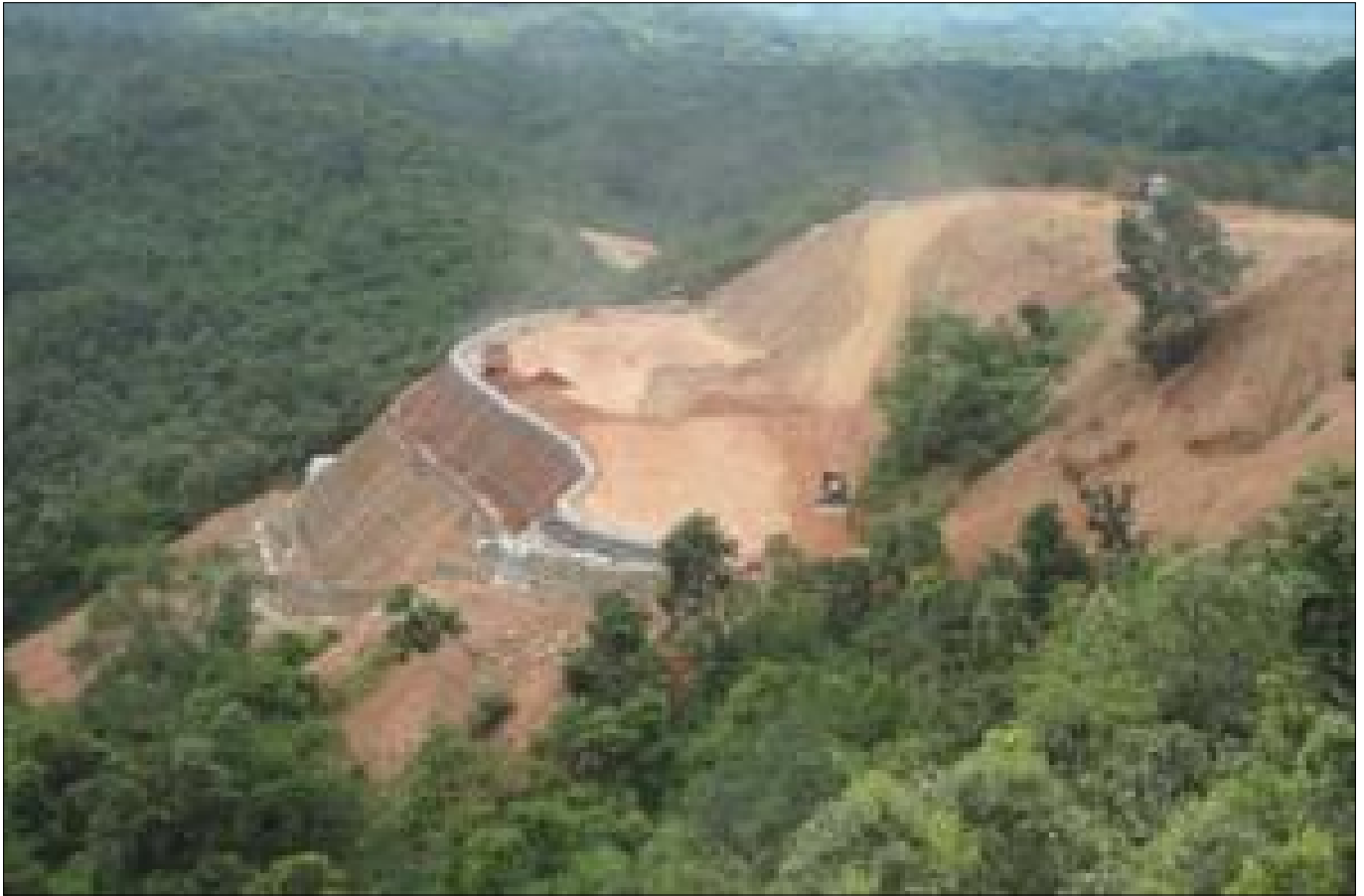
RSS with TechGrid GeoGrid – Under Construction
