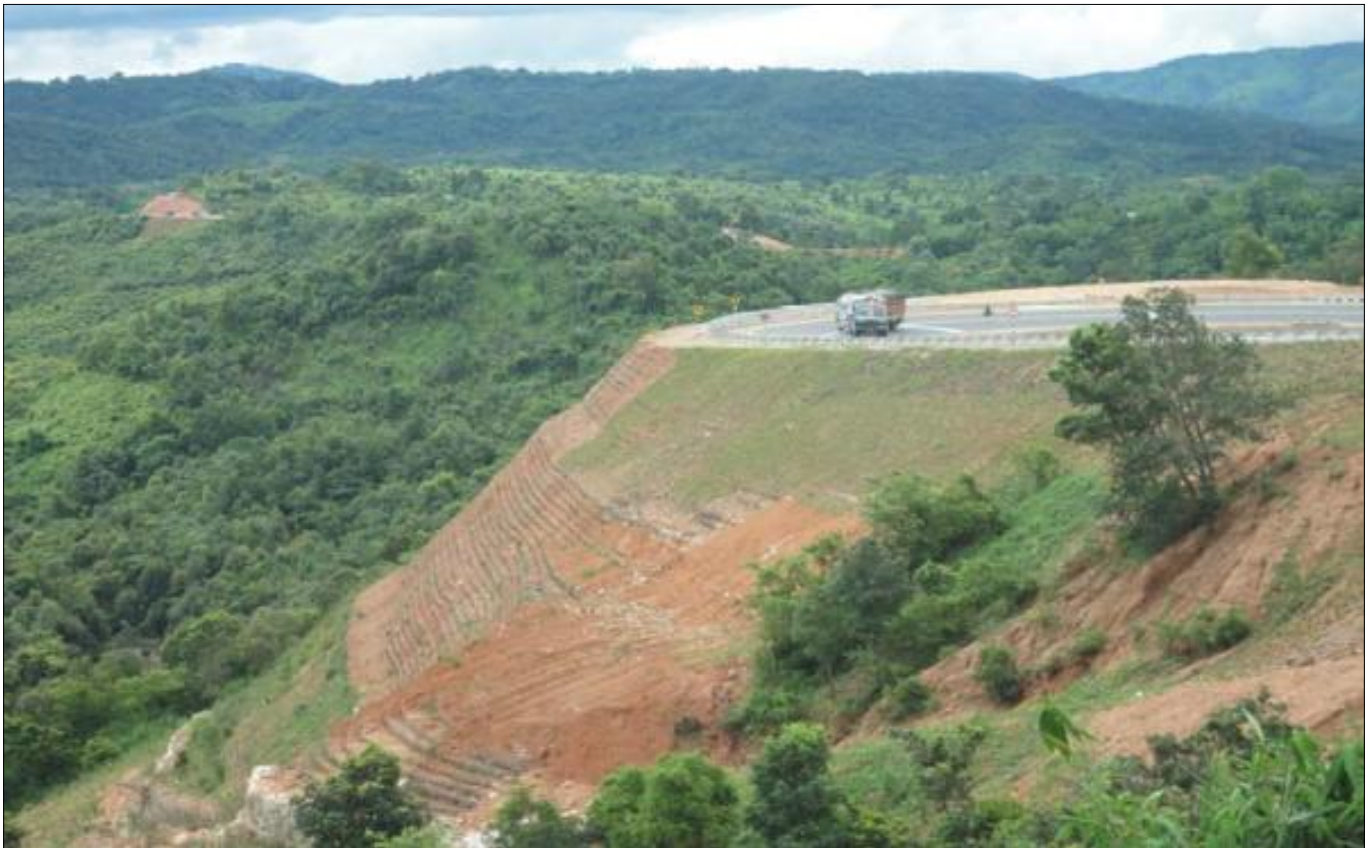
After Completion of Project with vegetation
