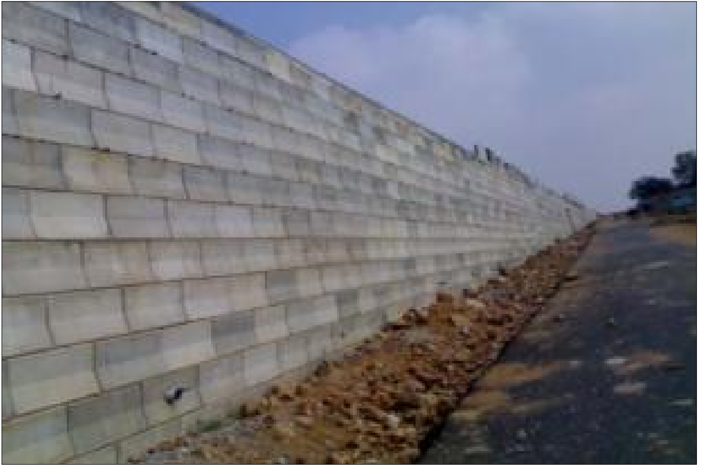
Elevation view of RS Wall
