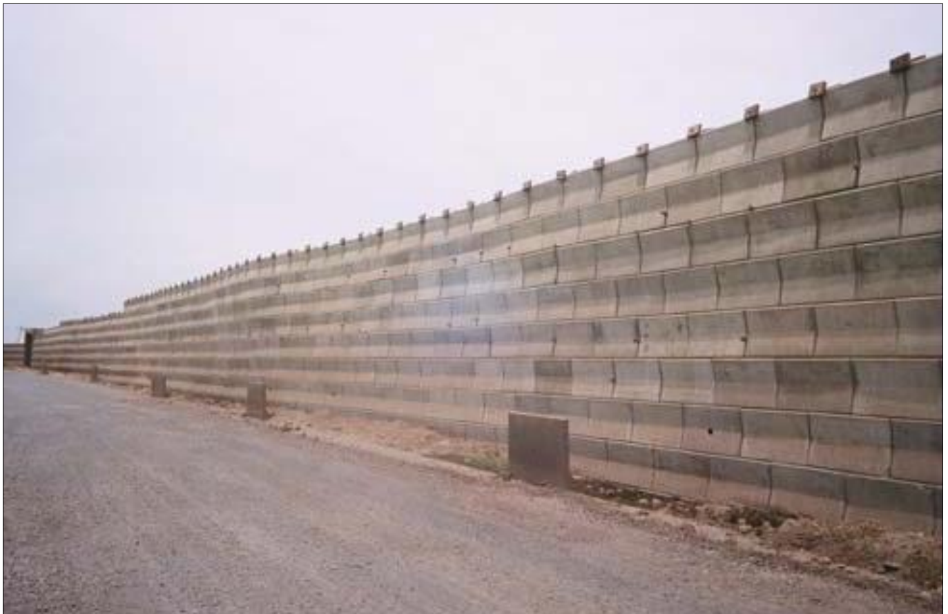
Elevation view of RS Wall
