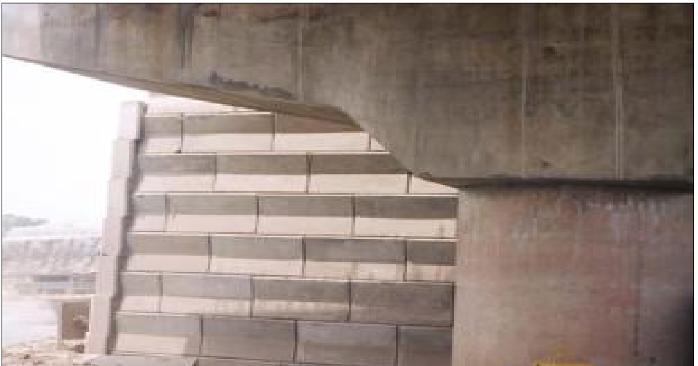
Abutment of RS Wall
