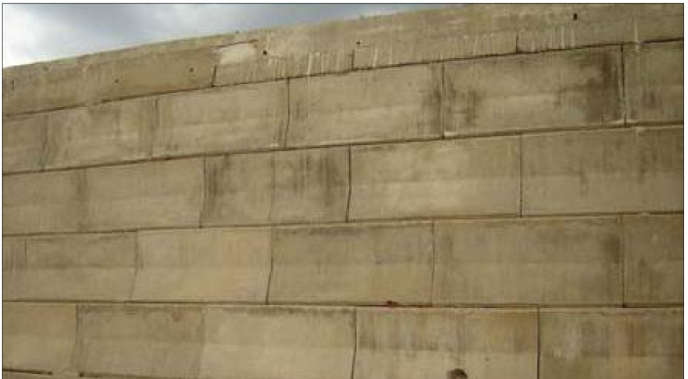
Photo 1 : Elevation view of RS wall
