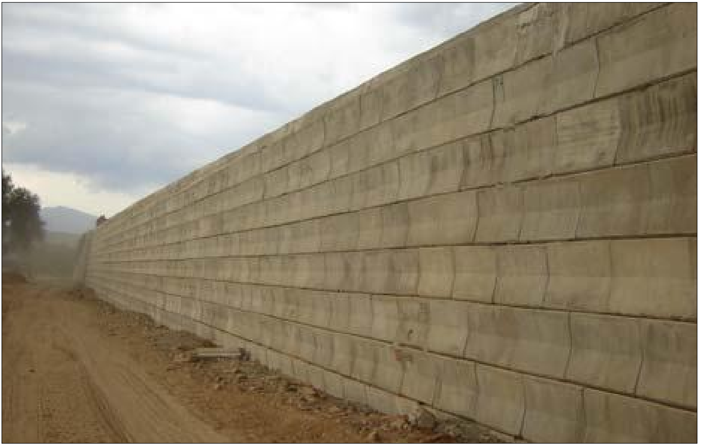
Photo 3 : Elevation view of RS wall
