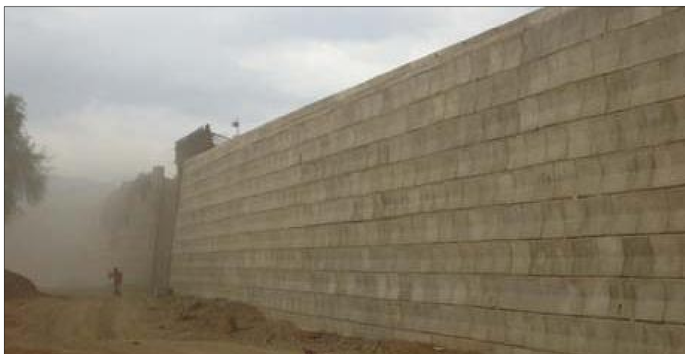
Photo 2 : Elevation view of RS wall
