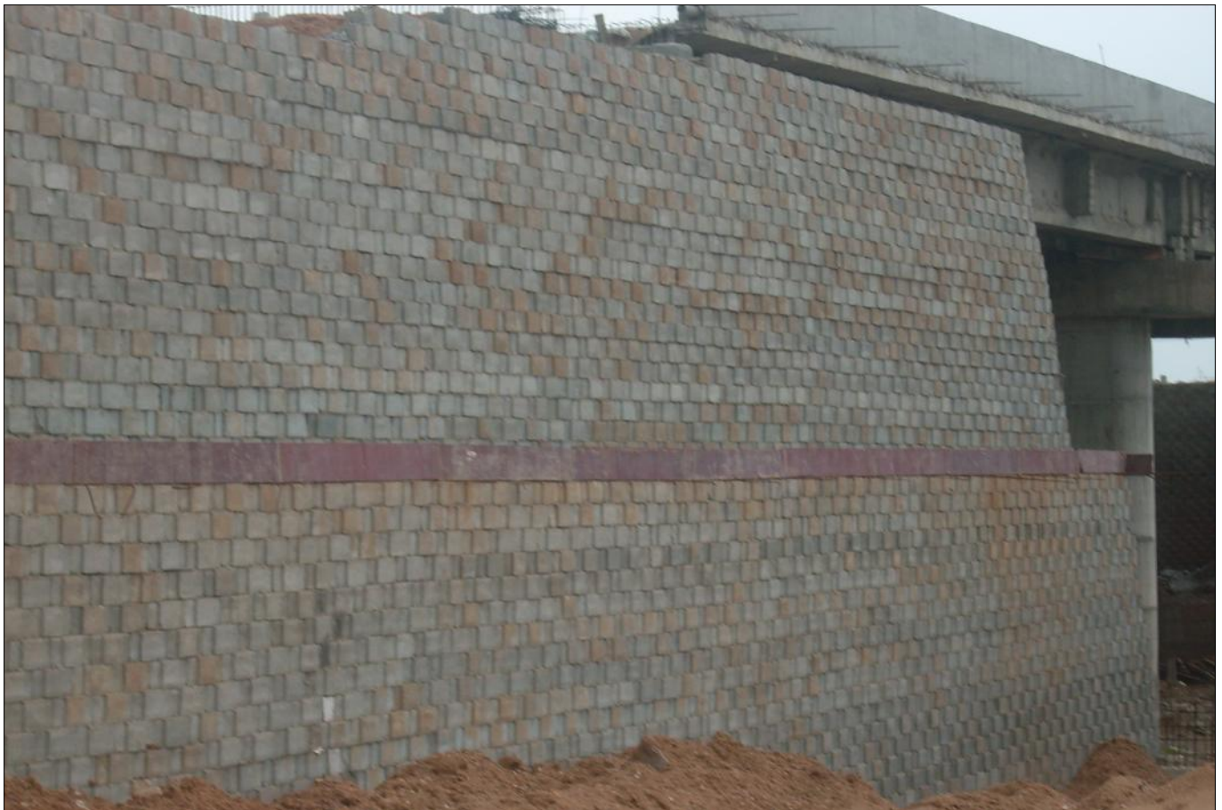
Photo 1 : Elevation view of Two Tier RS wall
