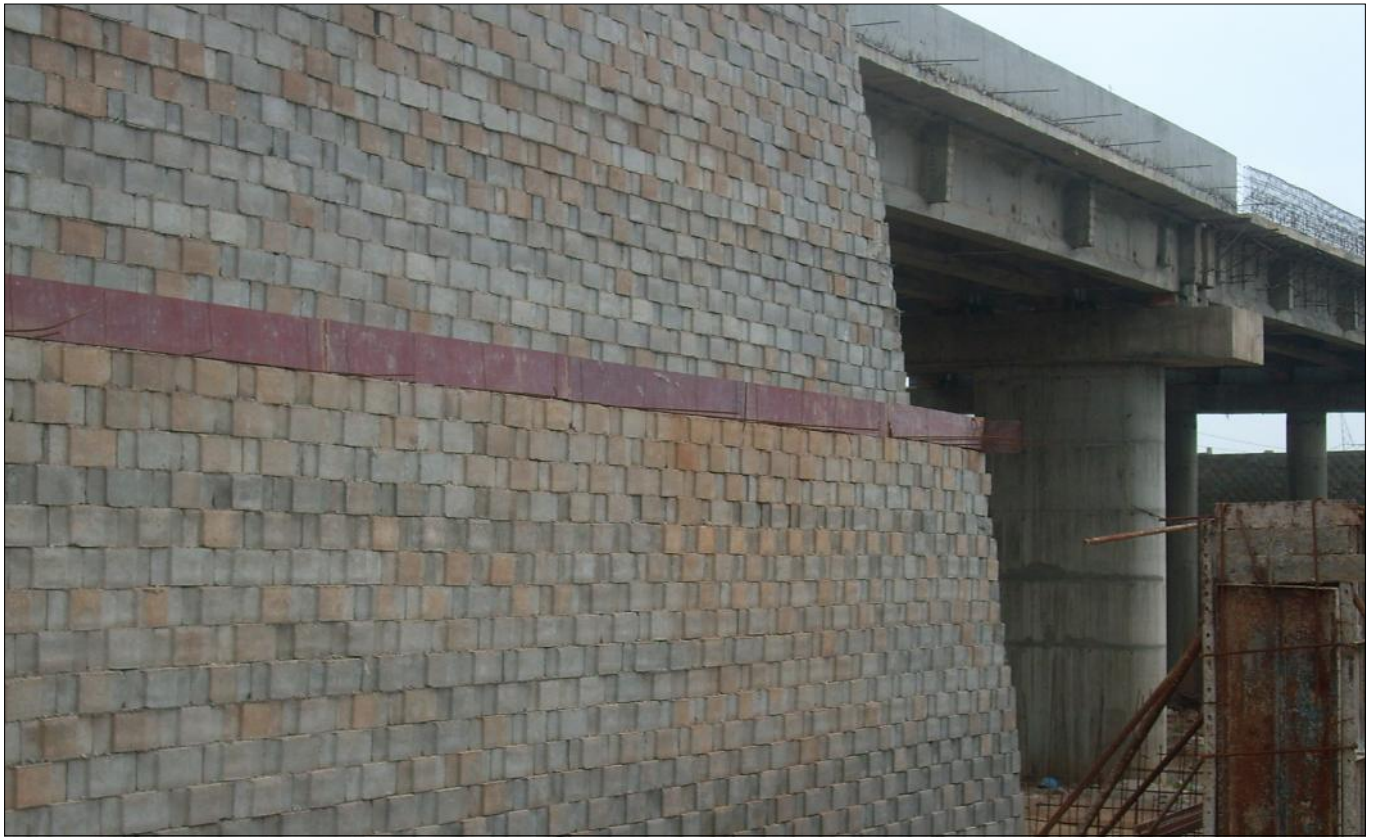
Photo 3 : Elevation view of Two Tier RS wall
