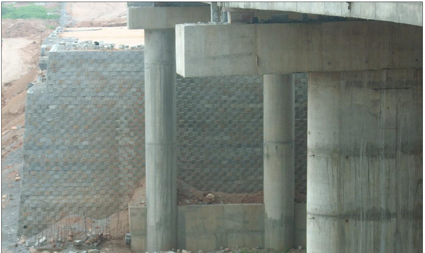
Photo 2 : Abutment RS wall
