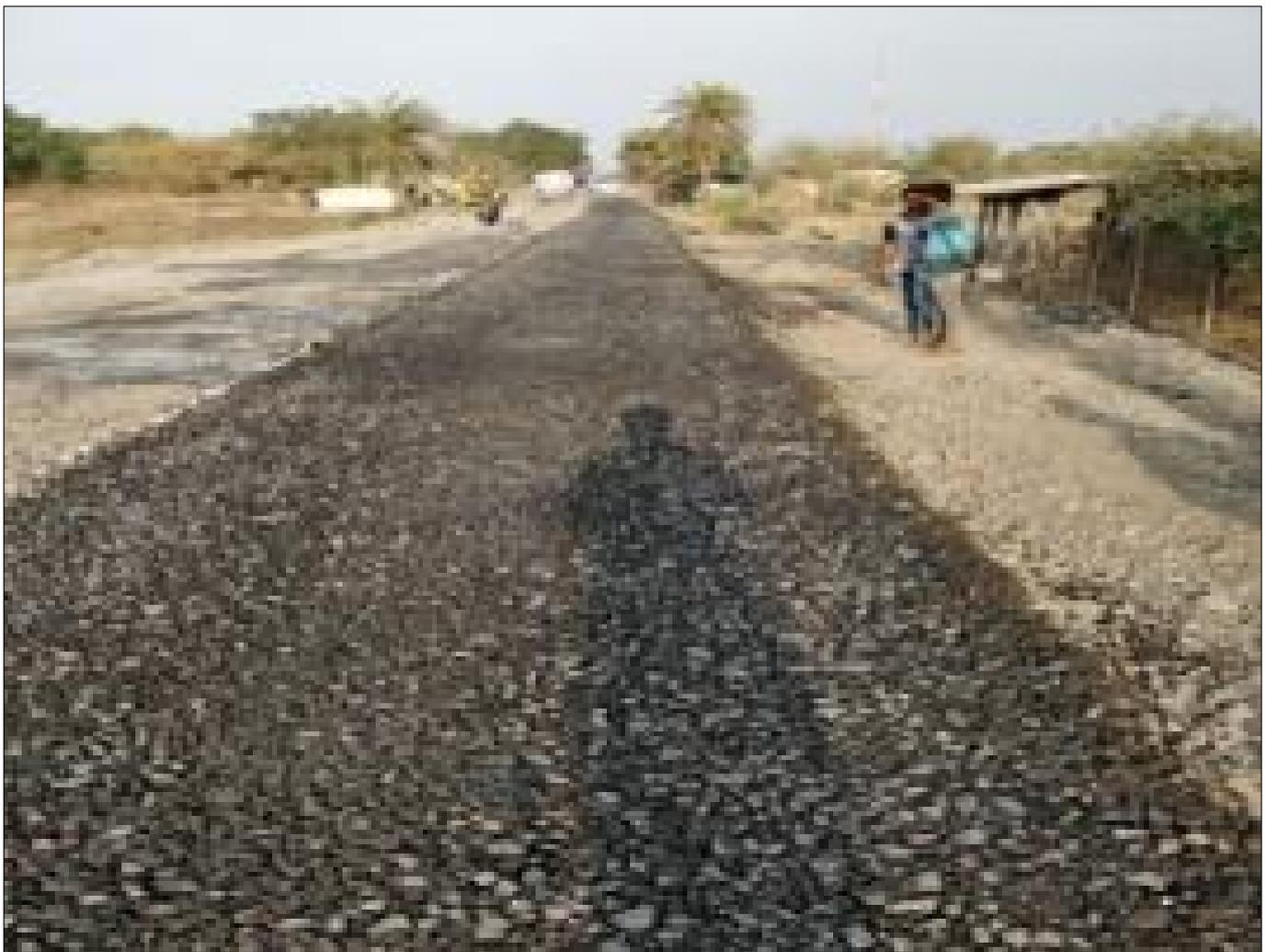
WMM compaction in progress
