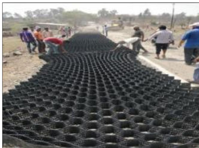
Laying of Techcell Geocell in Progress
