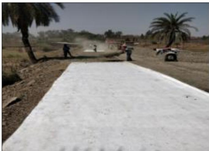
After laying geotextile, laying of 25mm bottom cushion of WMM
