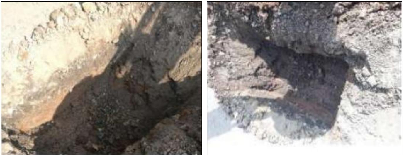
After site visit and detailed observation it is concluded that the softening of sub base layer can be the main reason of failure under heavy axle loading which was not anticipated. Conventional methods of pavement/soil improvement were already tried and which proved ineffective, so it is very important to offer solution considering the life of pavement; anticipated growth in traffic and cost.
