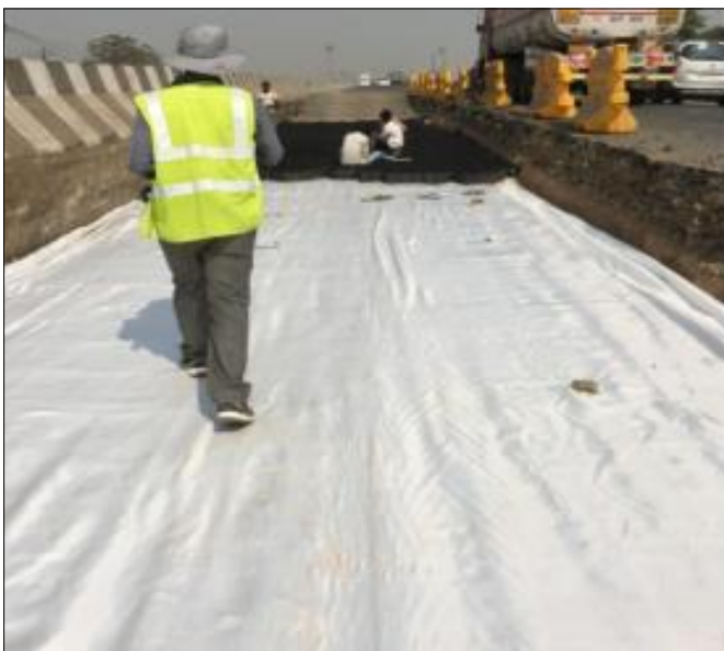
High Strength Woven PET Geotextile laid
