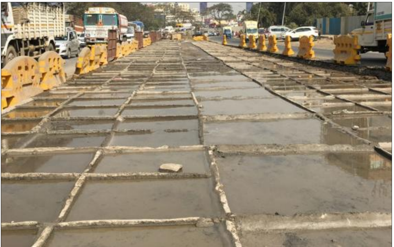
Curing of PQC layer by water ponding method
