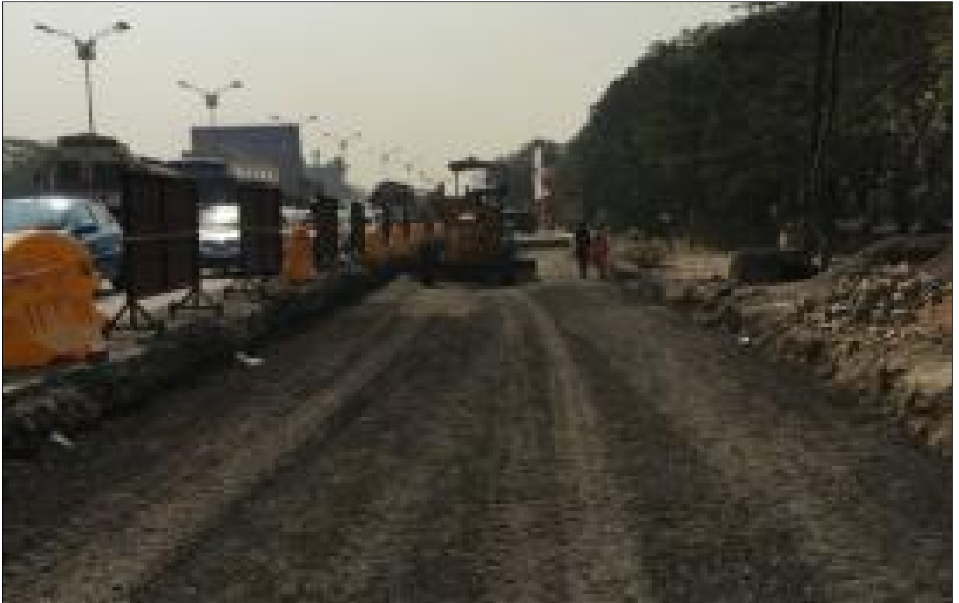
Compaction of Infill material in progress
