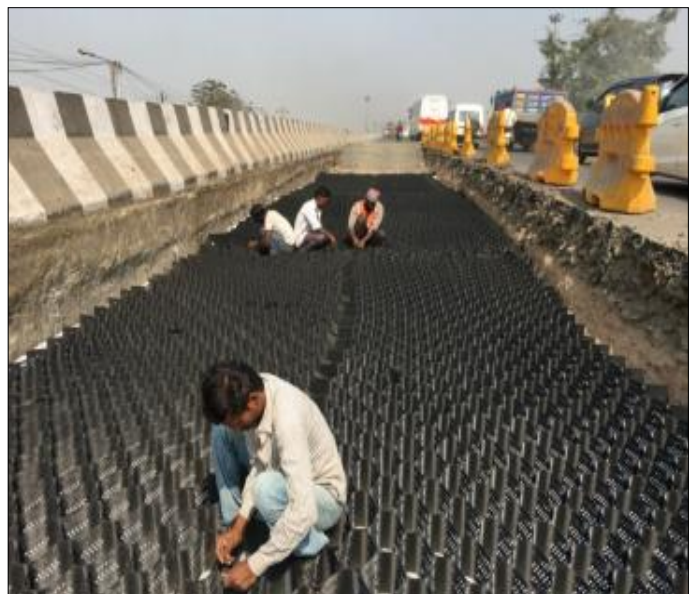
Techcell geocell tying in progress
