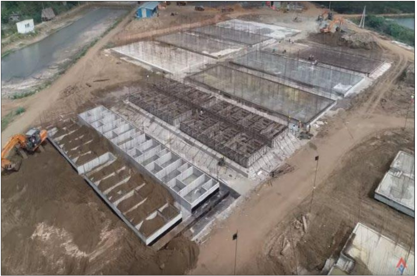
Aerial View: Raft Foundation completed
