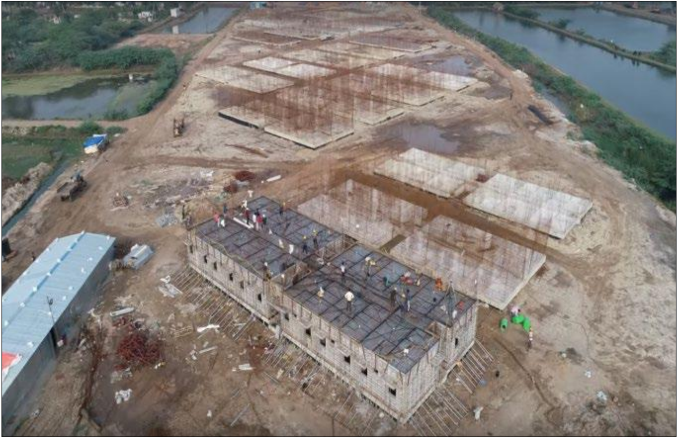
Aerial View: Construction of house over foundation is in progress
