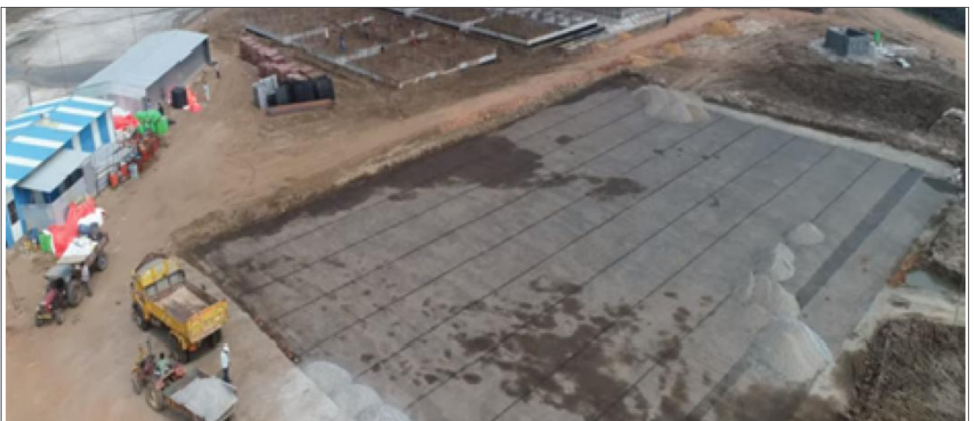
Aerial View: Compaction of infill and PET Geogrid on top
