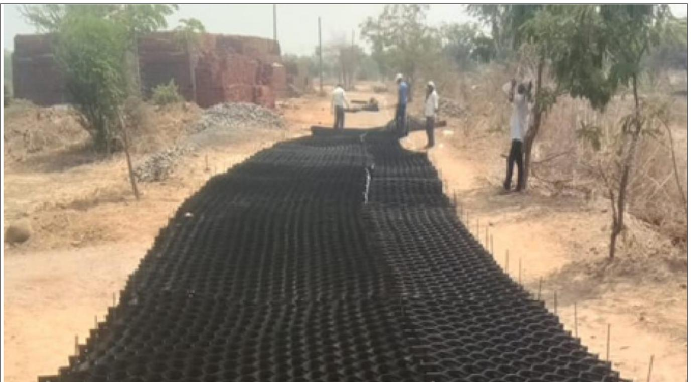
**Spreading of TechCell Geocell above the subgrade**
