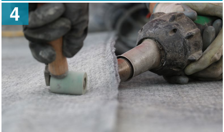
Thermally bonding overlapping layers of CCX™
