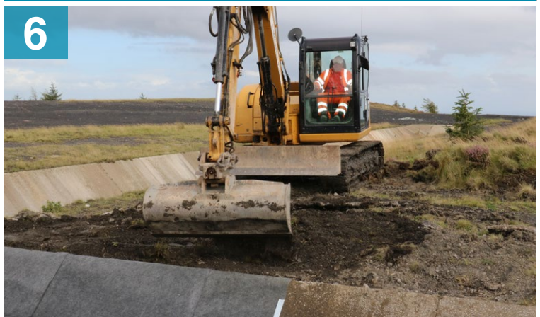
Backfilling anchor trenches to prevent ingress
