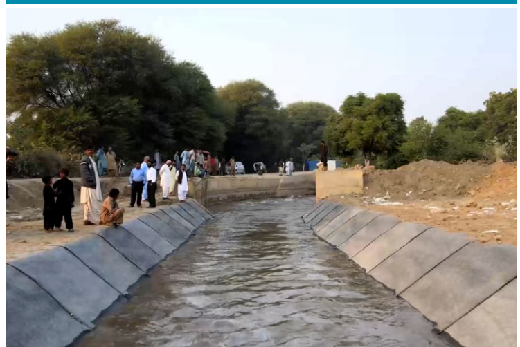
A CCX™ Bulk Water Infrastructure Remediation Installation
