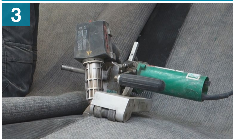
Thermal welding of CCX-B™ LLDPE backing
