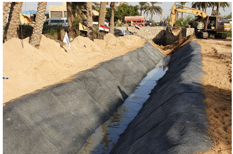
A CCX™ Irrigation Canal Installation
