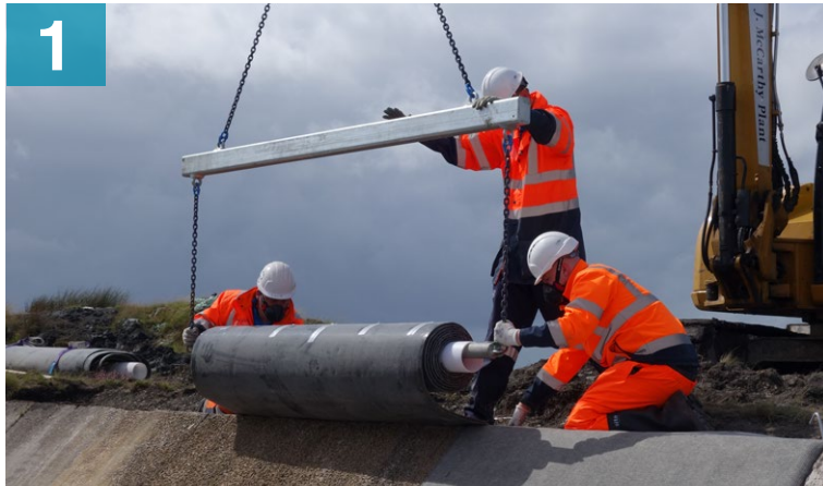
Deploying Bulk Roll of CCX™
