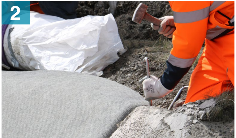
Pegging CCX™ within anchor trenches
