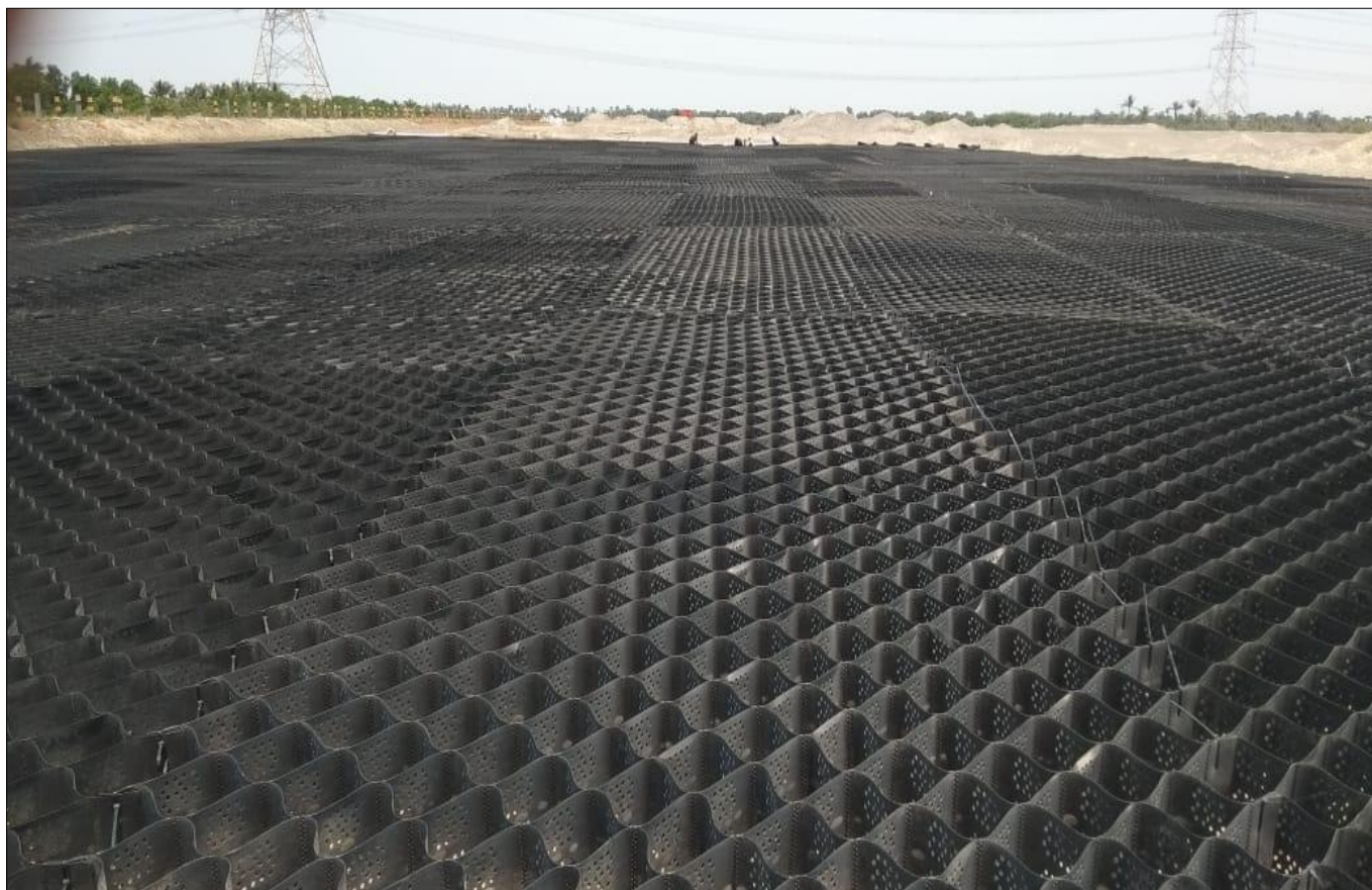
Photo 7 - Spreading of Techcell Geocell is in progress
