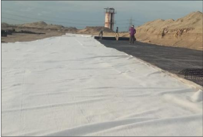
Photo 2 & 3 - Laying of Geotextile is in progress
