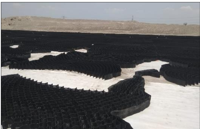
Photo 5 - Laying of Techcell Geocell
