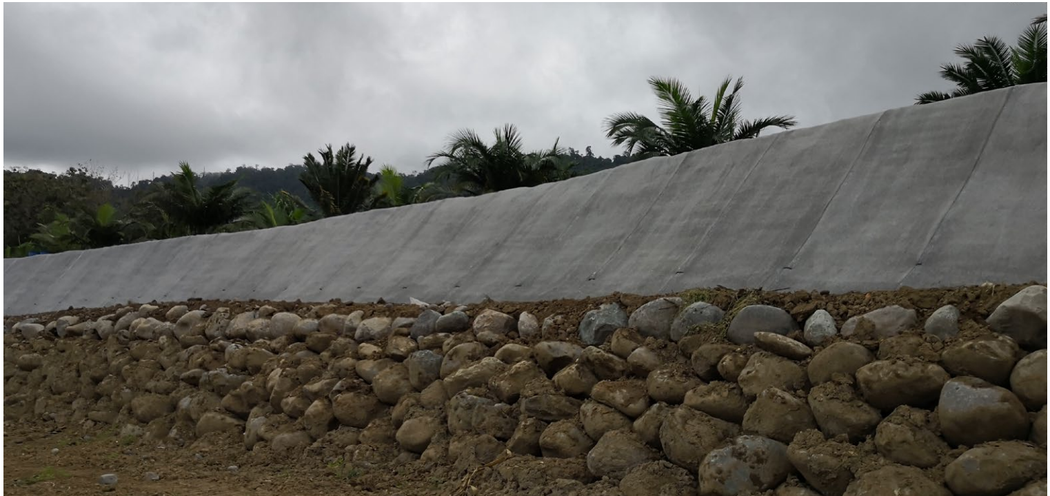
Completed erosion protection works
