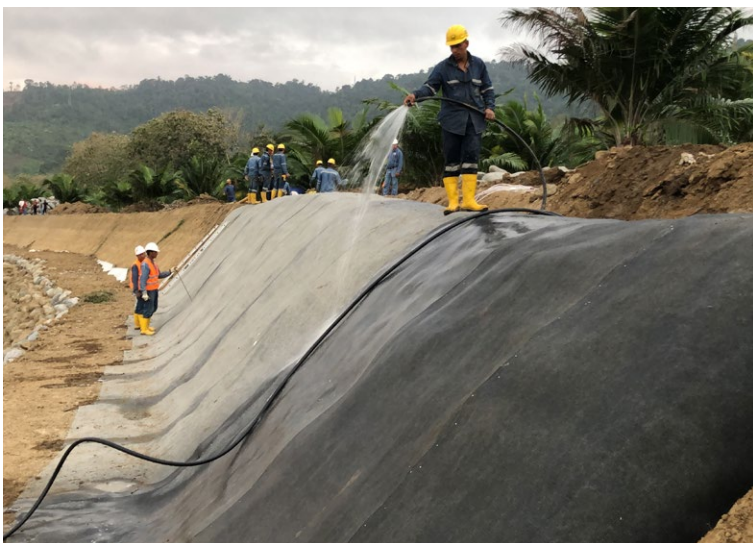
Once installation was complete, the CCX-M™ was hydrated
