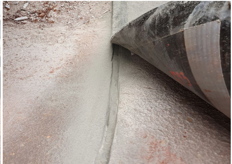
Termination slot created to secure CCX-M™ edge
