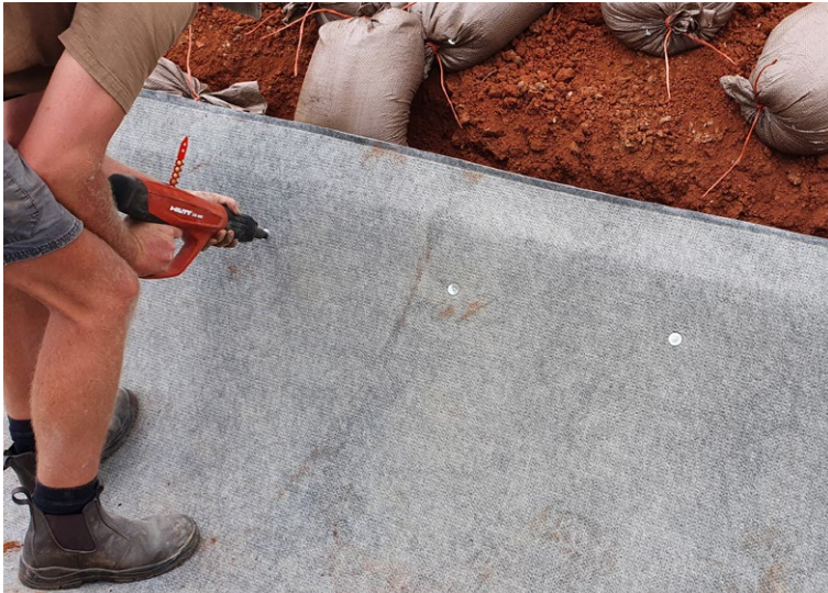
Installation of shot-fired nails
