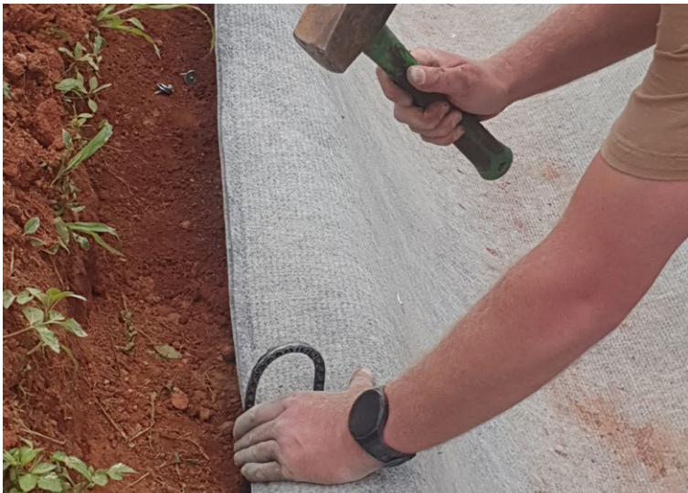
CCX-M™ secured within shallow anchor trenches using custom pegs
