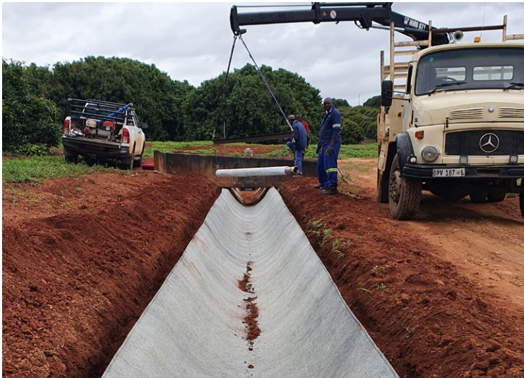
CCX-M™ rolls deployed from Hiab and spreader beam
