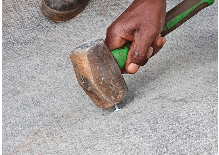
Fixing CCX-M™ to channel invert with nails and washers
