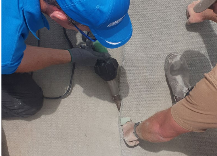
Thermal welding of CCX-M™ joint
