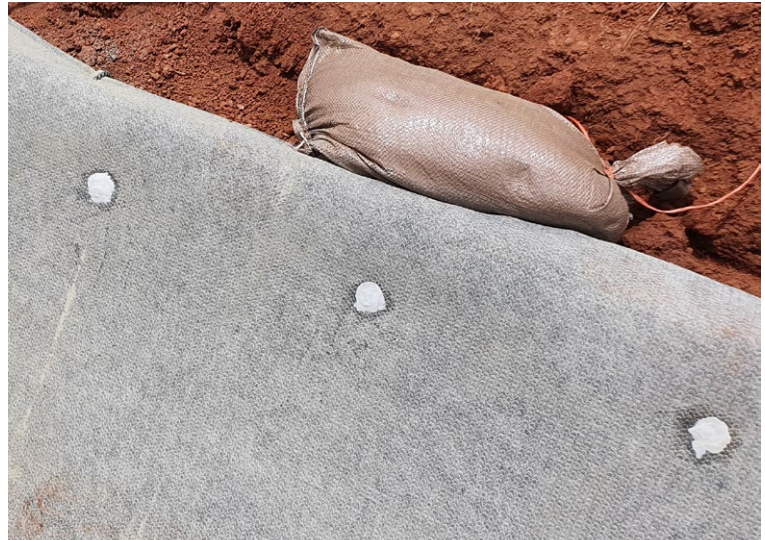
All nails were covered with epoxy
