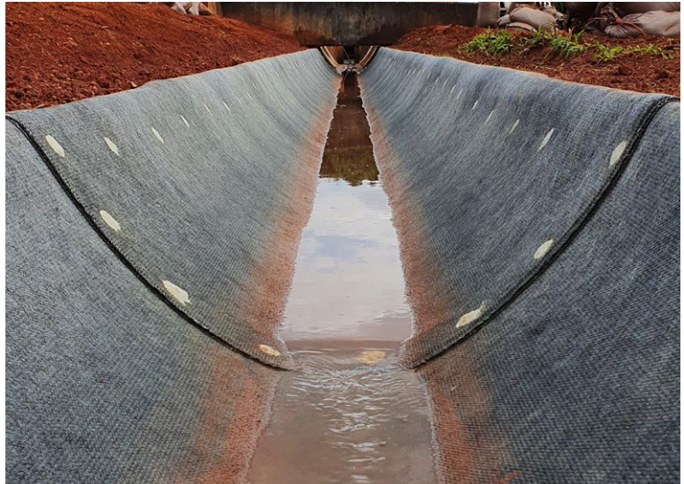
Shot-fired nails were also inserted in overlap joint and sealed with epoxy
