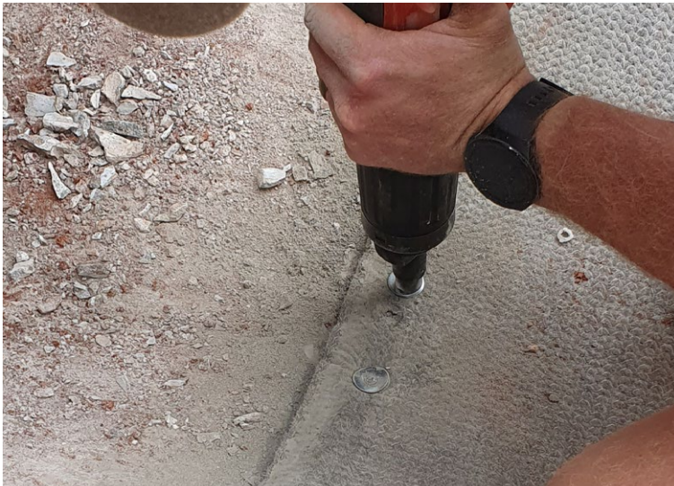
Shot-fired nails used to secure CCX-M™ edge within termination slot
