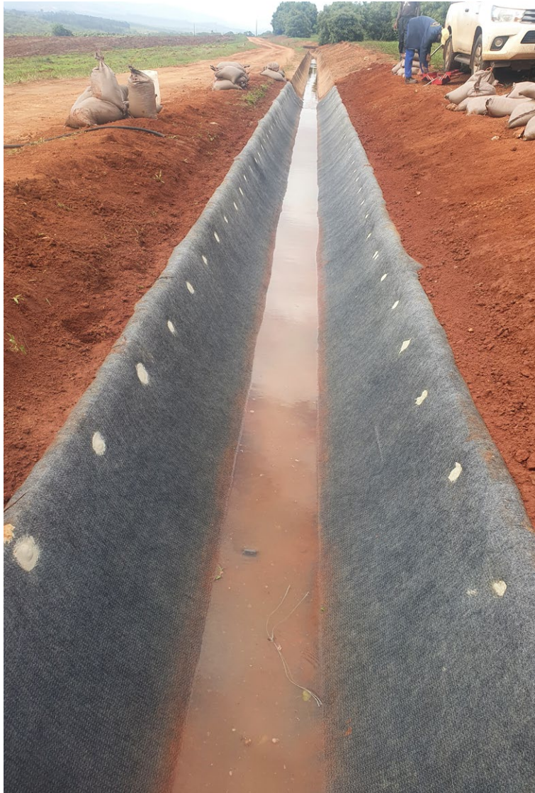
Completed installation following hydration
