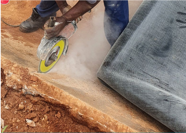
Creation of downstream termination slot in existing concrete
