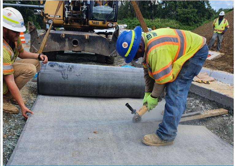
CCX-M™ cut to desired length with hand tools
