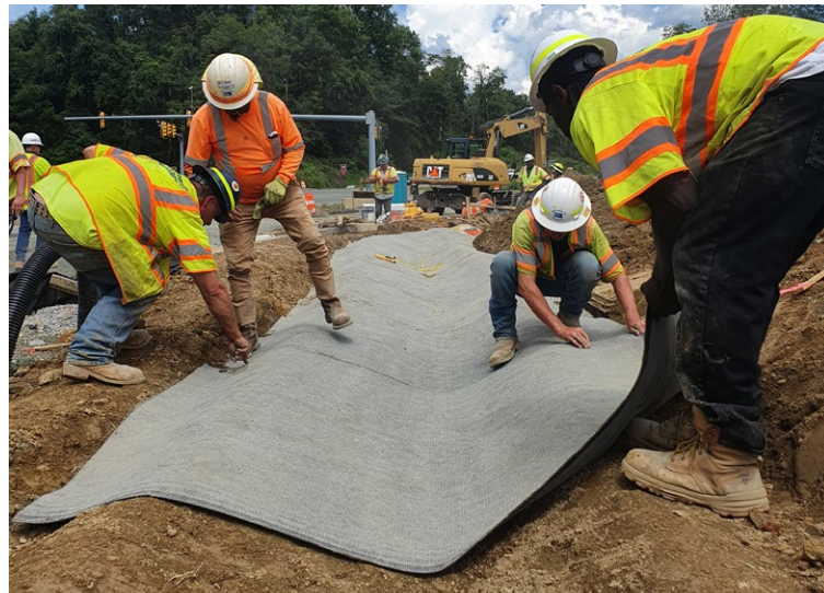
CCX-M™ laid transversely
