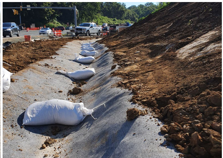
Temporary ballasting sandbags
