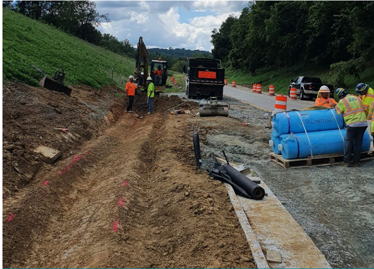
V-ditch dug with excavator
