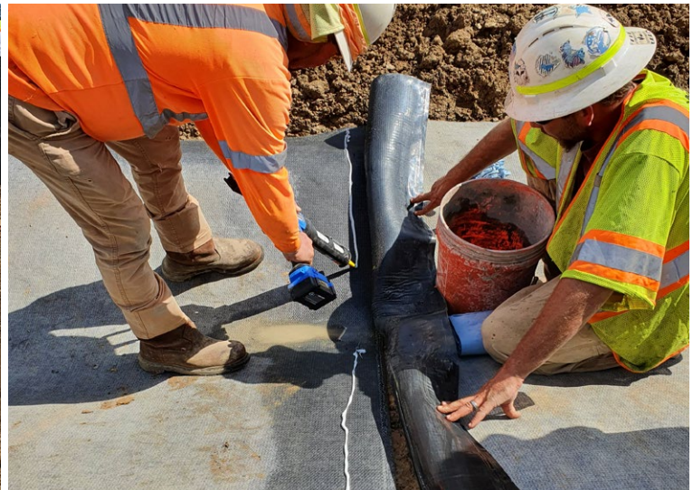
Overlapping layers sealed and screwed
