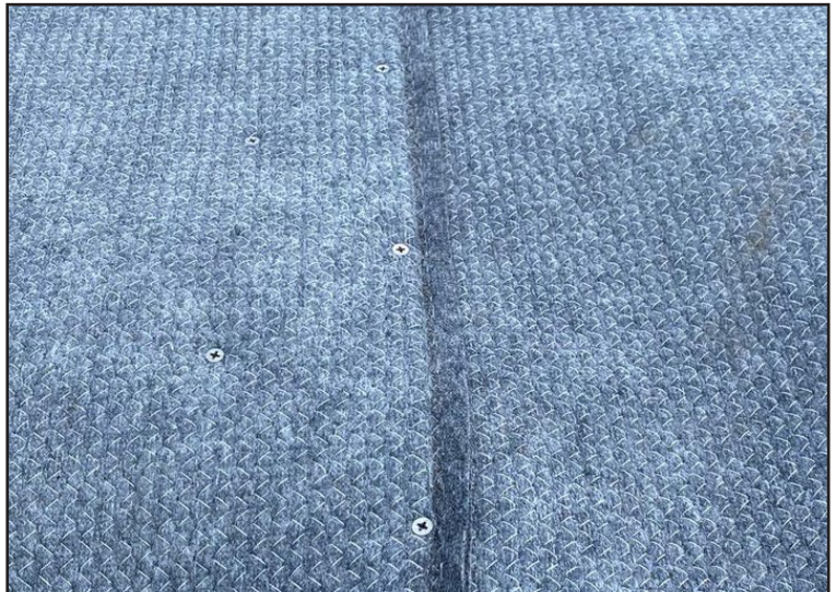
Overlapping layers secured with 100mm screws in zigzag pattern
