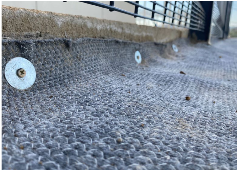
CCX-U™ fixed with 6x50mm masonry anchors
