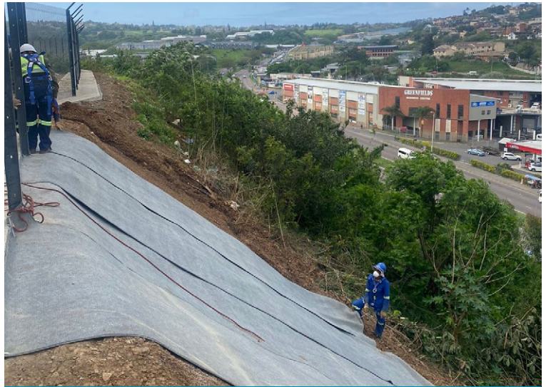
CCX-U™ Installed transversely down the slope
