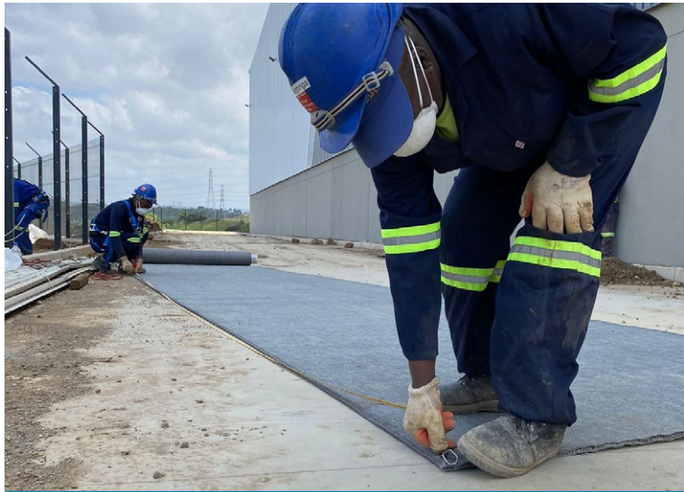
CCX-U™ measured before cutting and installing
