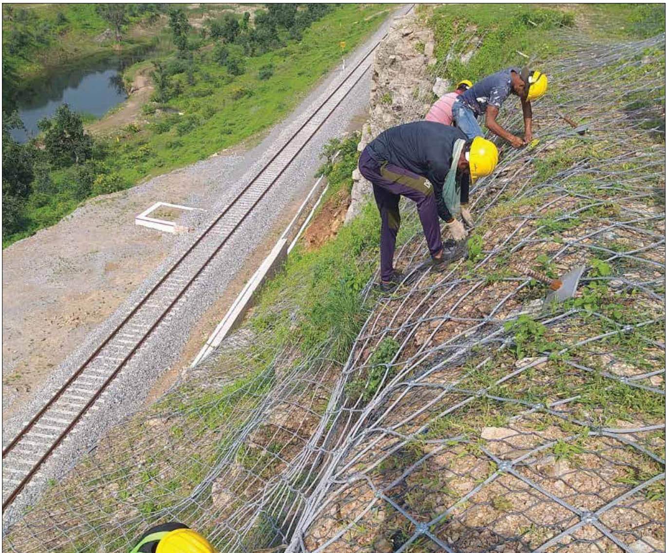
Photo 3 : Ensuring Safety: Installation of Rockfall Protection Systems
