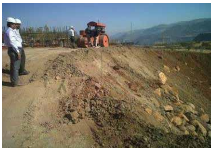
RSW with Weld Mesh - Under Construction
