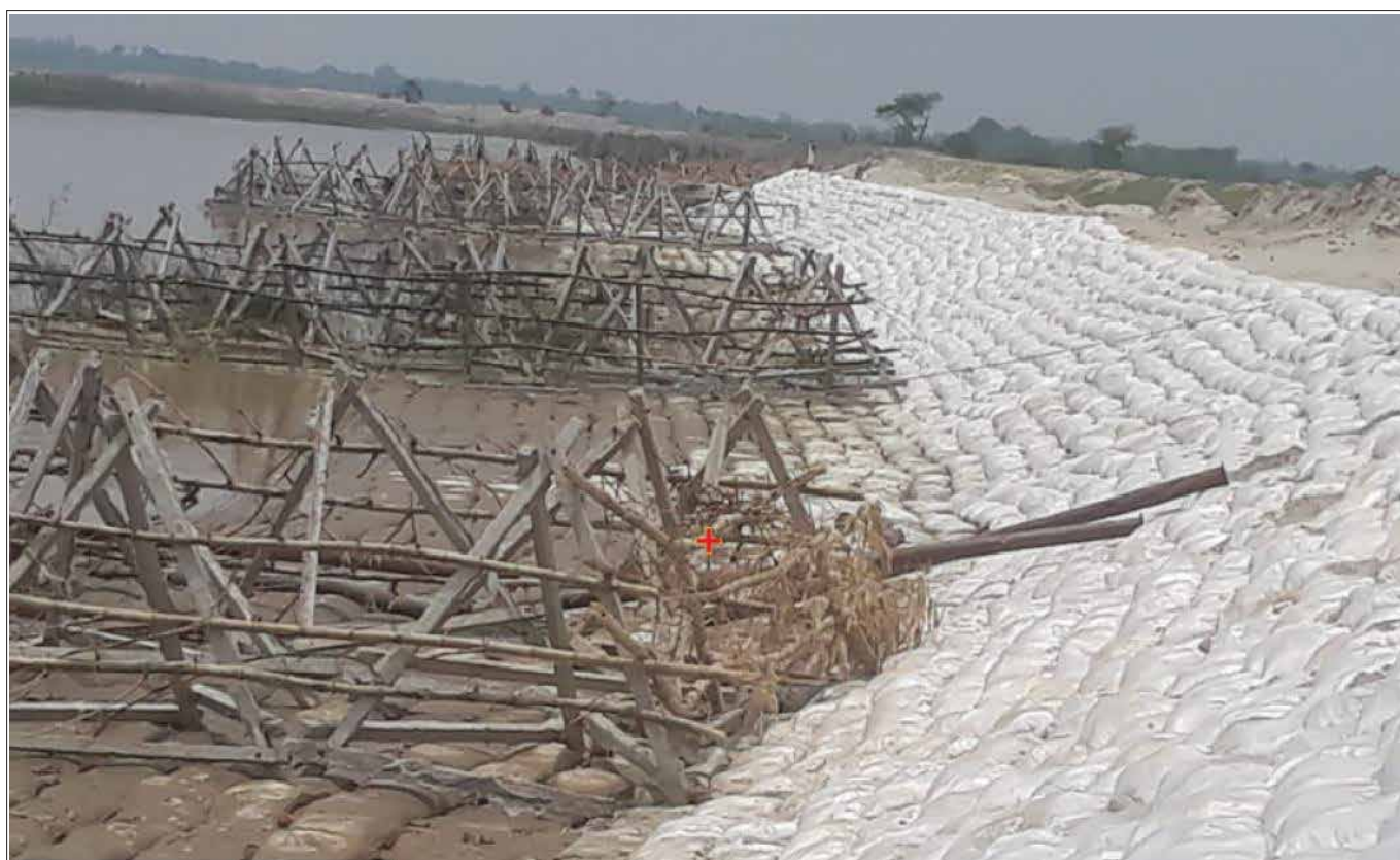
Photo 3: Porcupine concrete spurs
