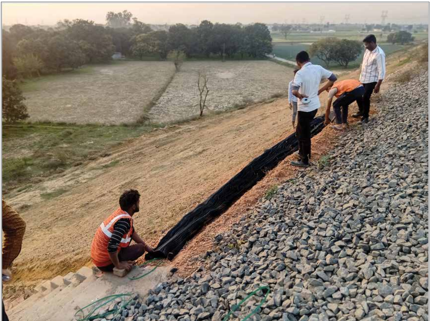
Photo 2 : Spreading of Geocell on Slope Surface
