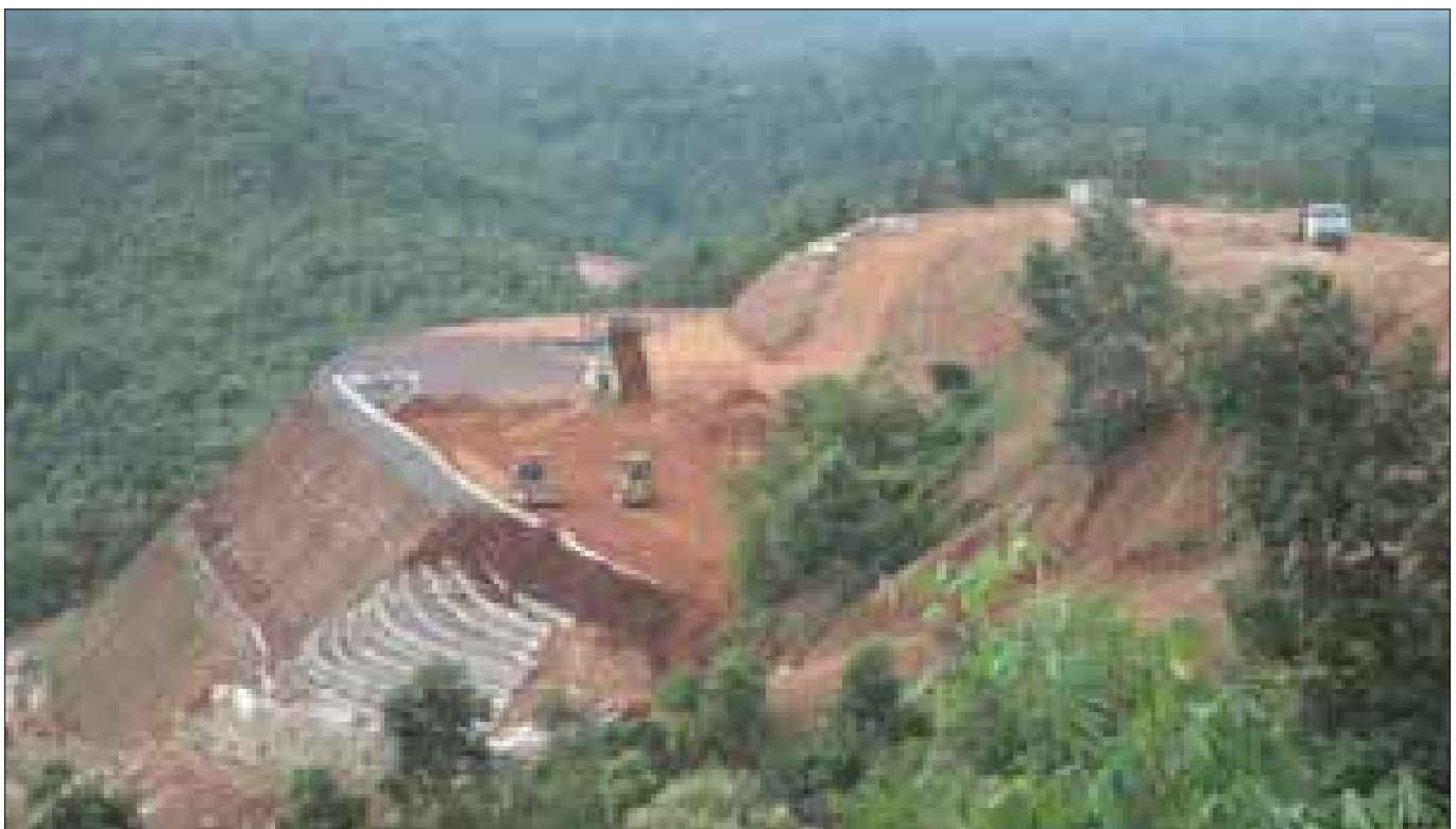
RSS with TechGrid GeoGrid – Under Construction
