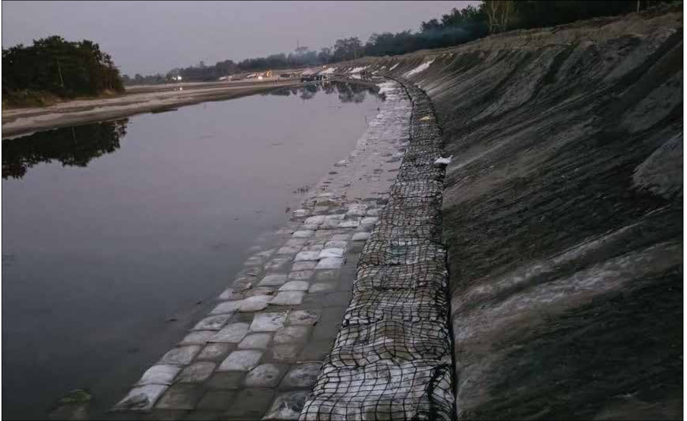
Photo 3 : Installation of Geotextile Bags on River bed (For Launching Apron)
