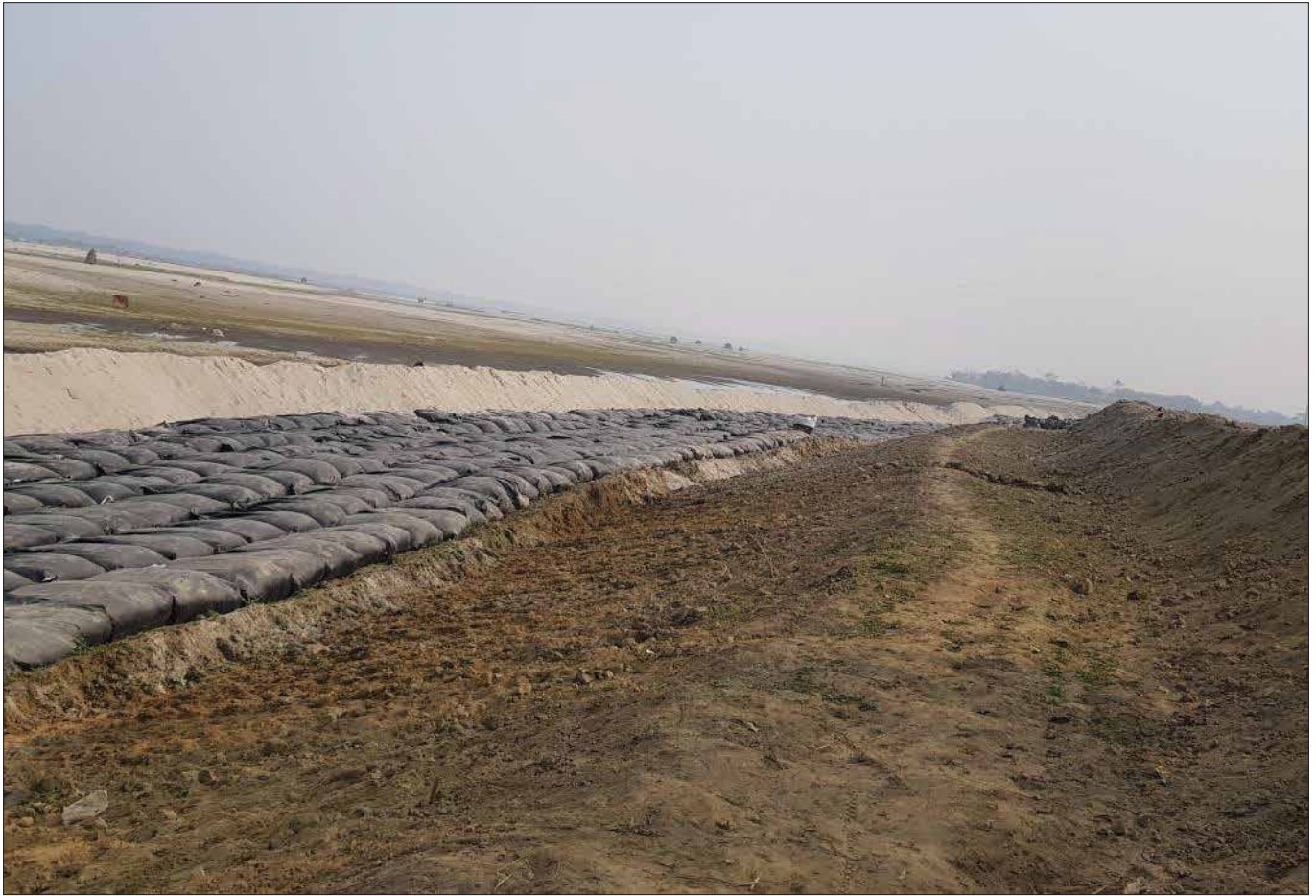
Photo 4 - Placement of Techfab Geotextile bags
