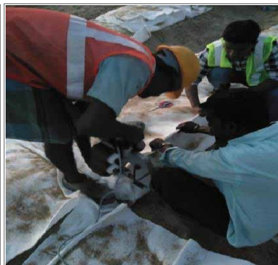
Stitching of geotextile bags by machine
