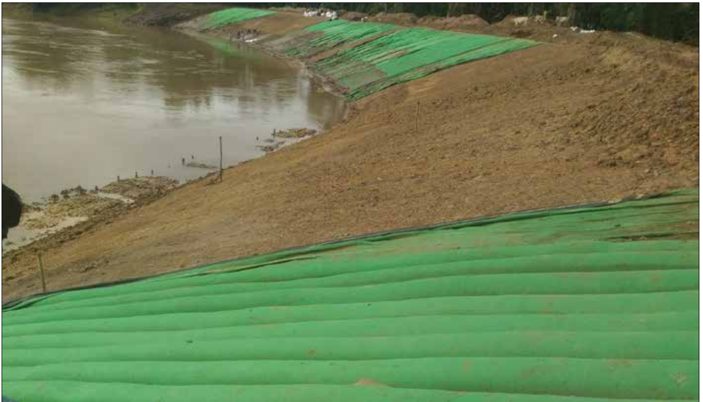
Photo 2 : Laying of Tech GeoMattress on Dressed Slope
