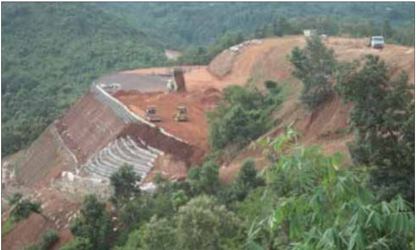
Reinforced Soil Slope – Top View
