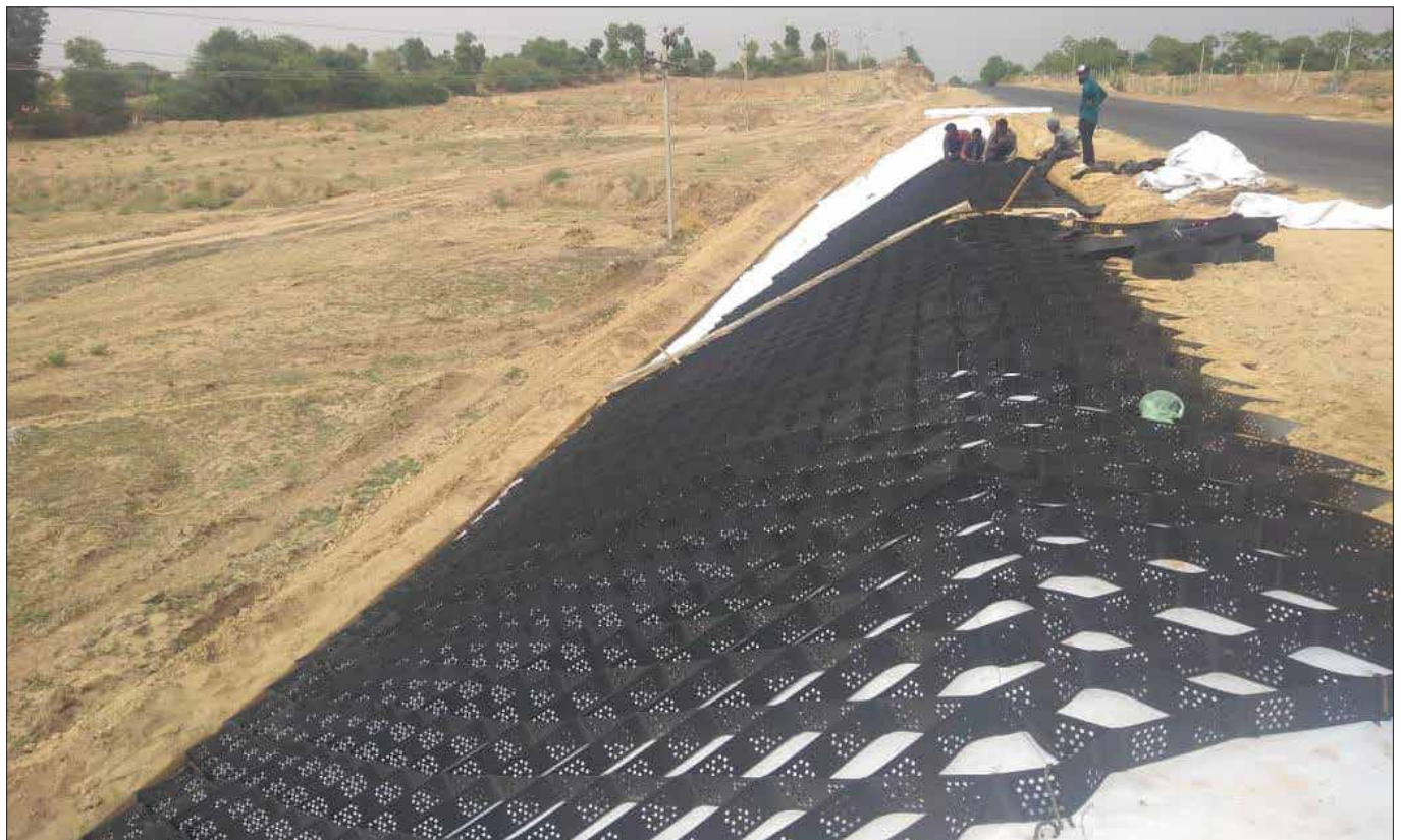
Installation of Geocell
