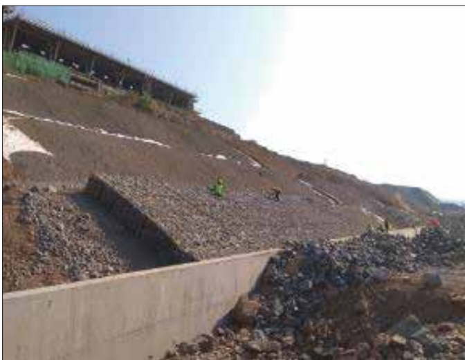
TechFab Metal Gabion Mattress laying in progress
