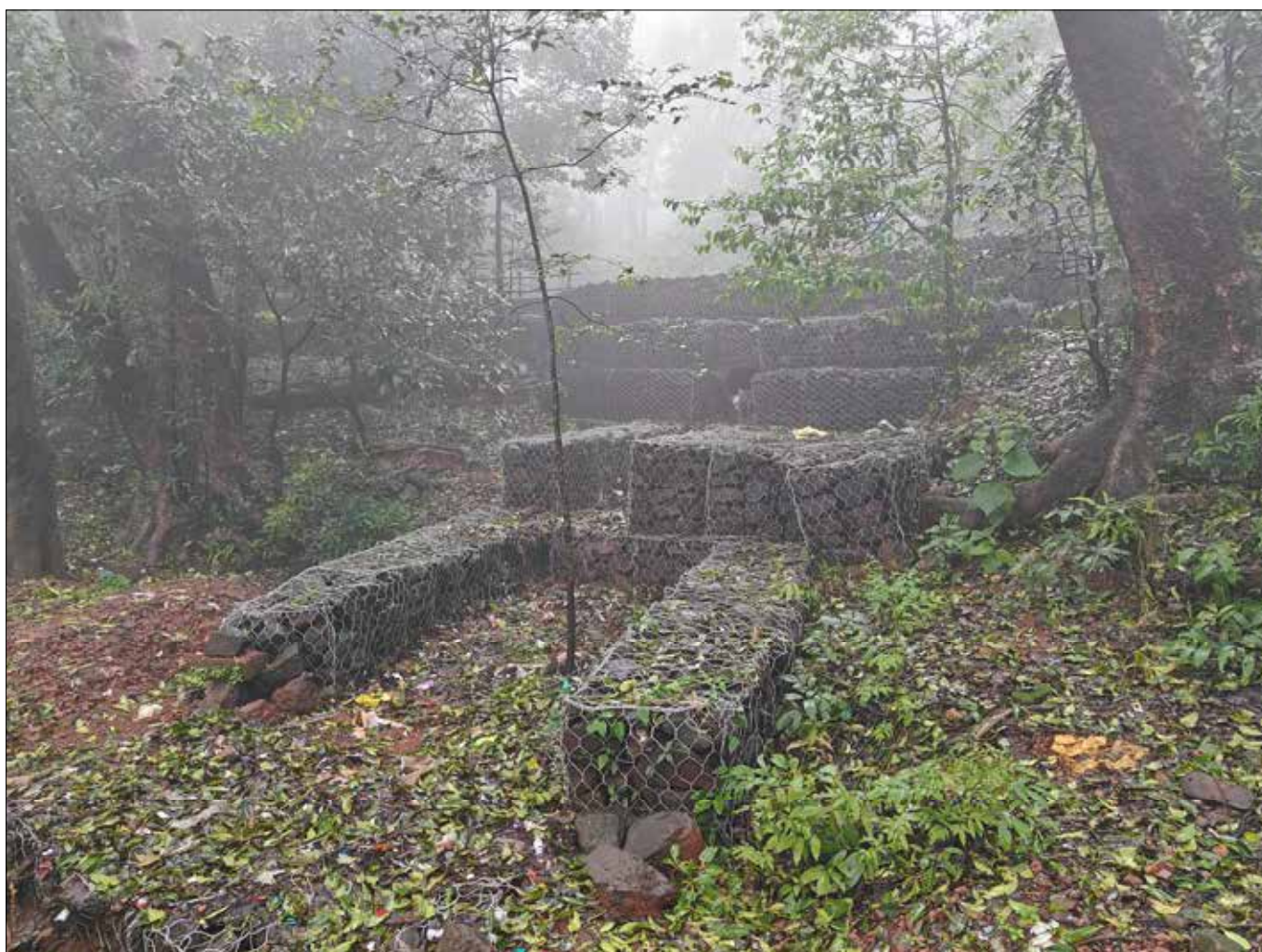
Photo 5 : Enhancing Drainage with Gabion Culvert Solution
