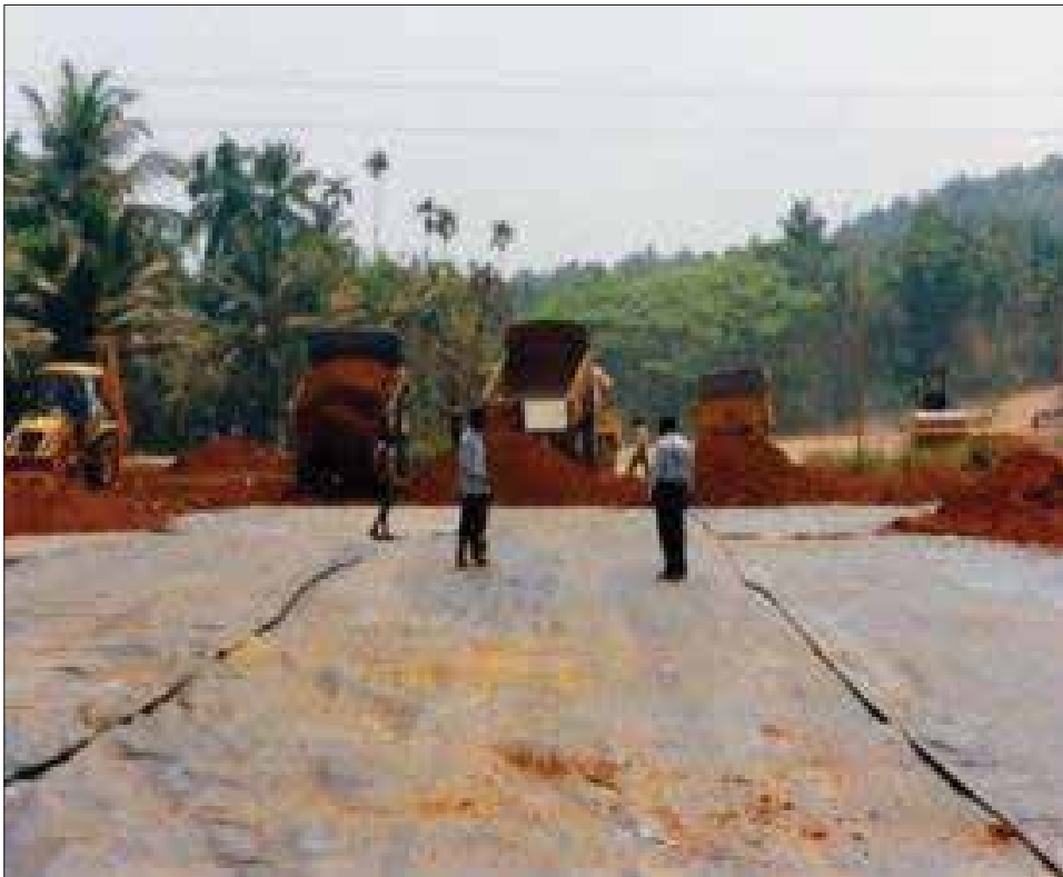
Installation of Techfab TPP 250 Woven Geotextile
