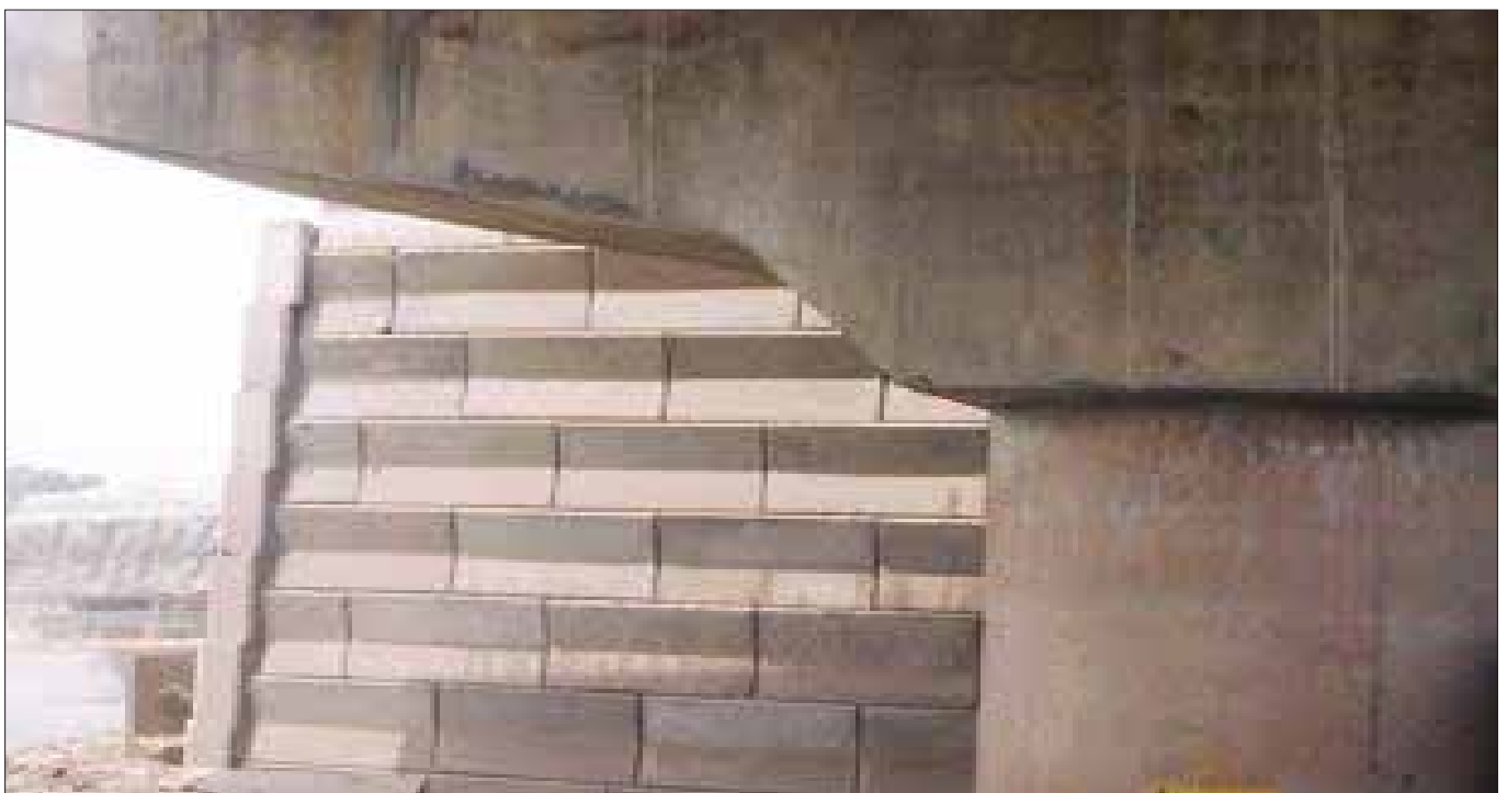
Abutment of RS Wall
