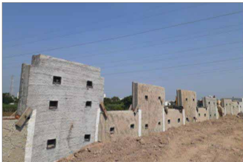
Erection of RCC Facia Panel in Progress
