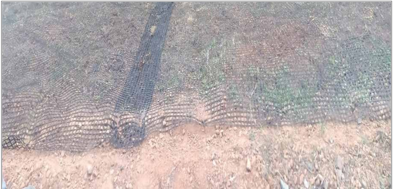
Photo 3 : Over lapping of Geogrid
