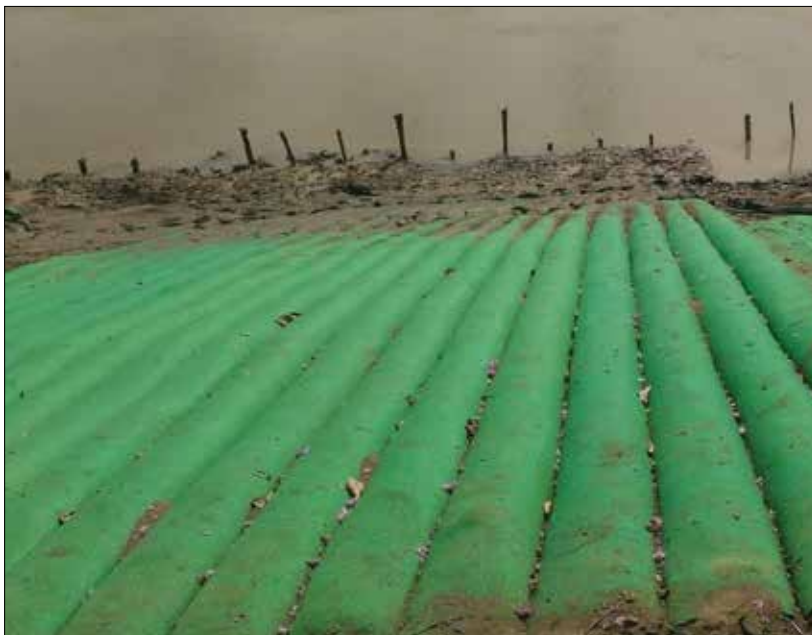
Photo 1 : Installation of Tech GeoMattress
