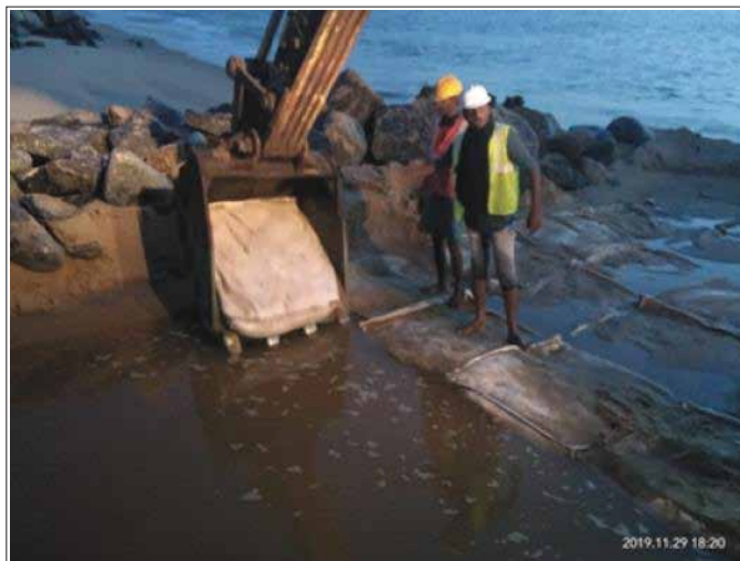
Laying of Geotextile bags in progress
