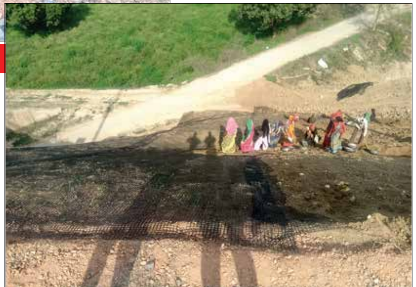
Photo 5 : Spreading the Vegetative Soil evenly over Geogrid
