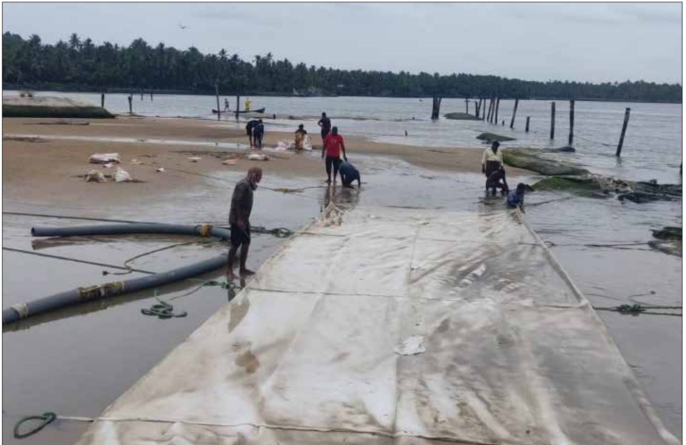
Laying of TechTube Geotextile Tubes in progress
