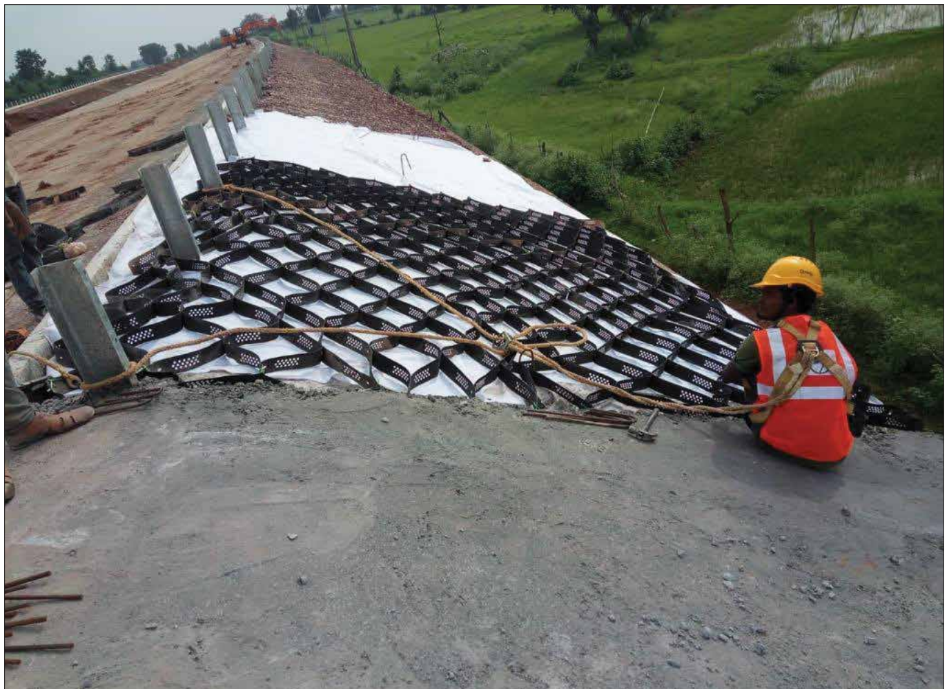
Progress of Concrete filling in Geocell
