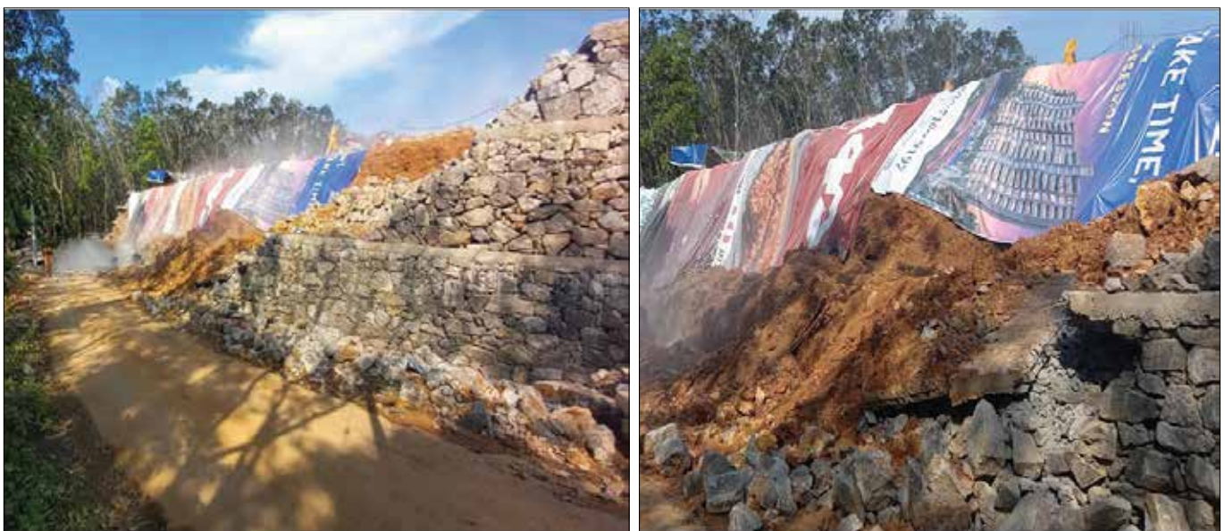
Photo 1 & 2 : View of the Collapsed Existing Stone Masonry Retaining Wall
