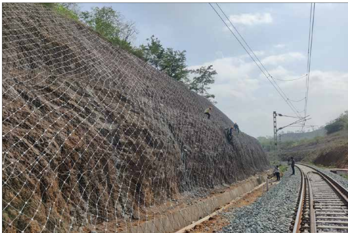
Photo 8 : Secured Slope : Post-Installation of Rockfall Protection Measures
