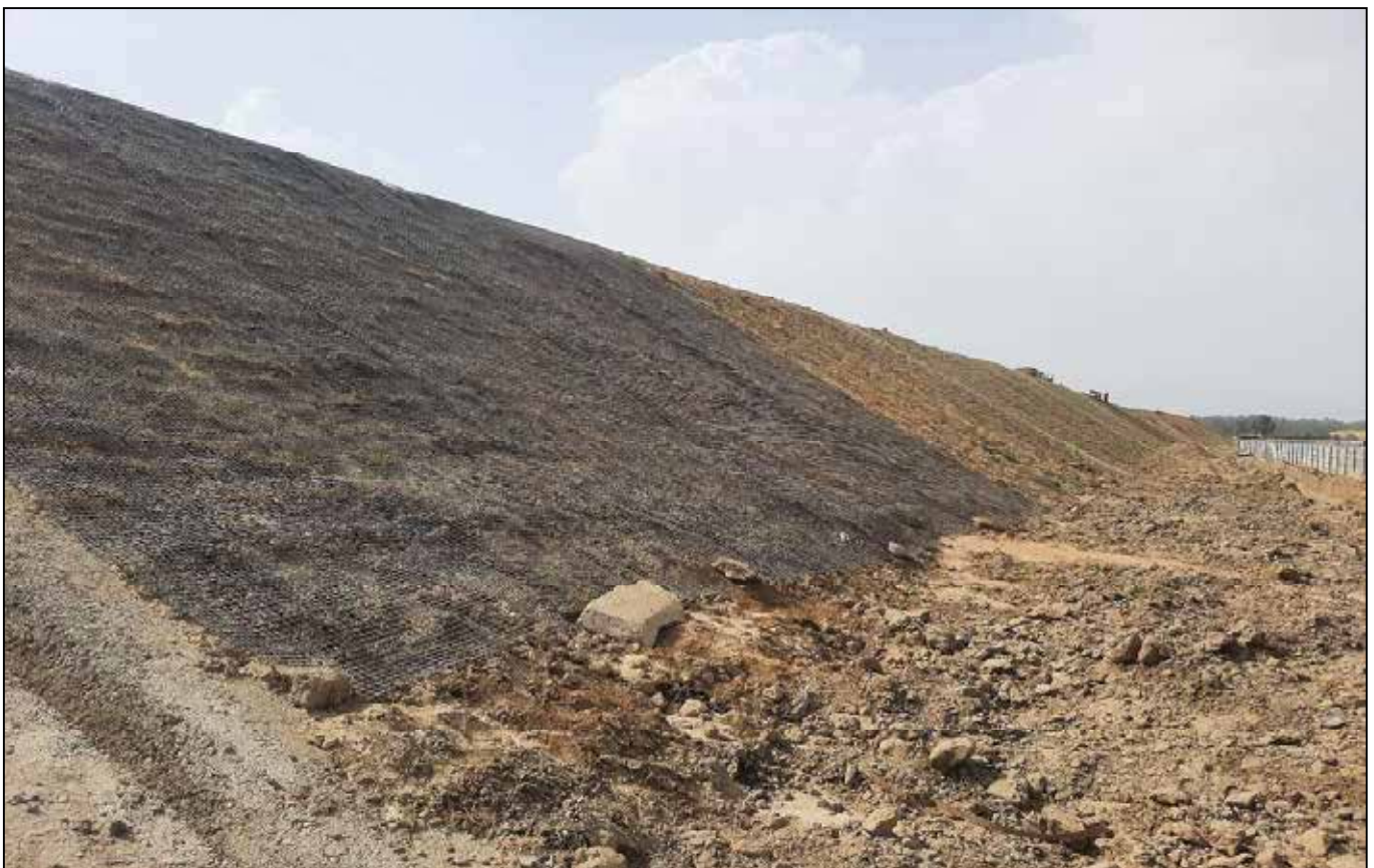
LAYING OF TECHGRID OVER THE SLOPE
