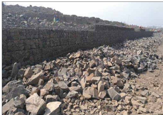
Figure 5 & 6 : Installation, Filling of Gabion mesh with stone in progress
