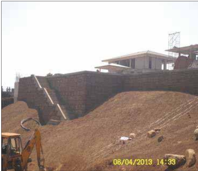
RSW with Weld Mesh - Entrance
