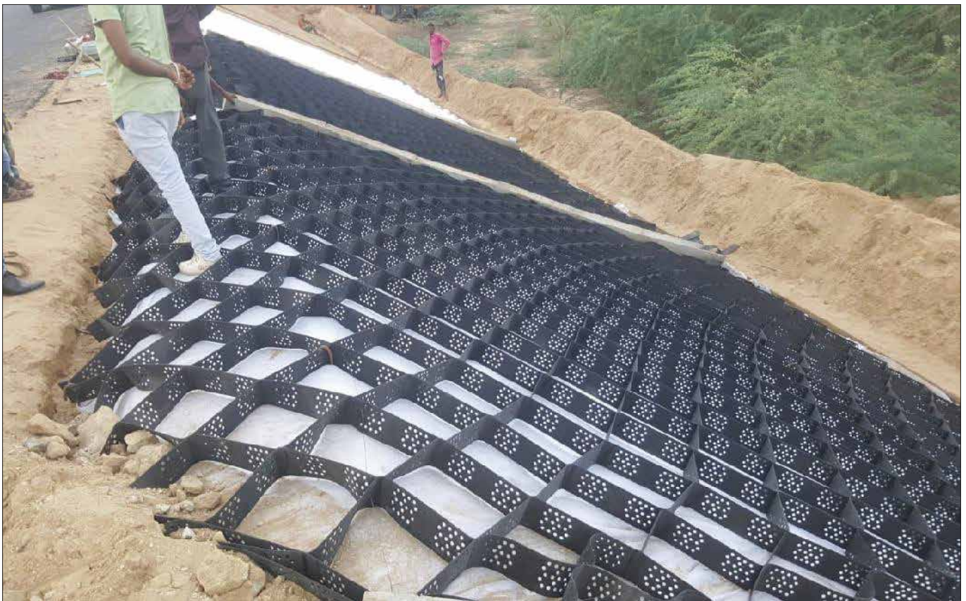
Installation of Geocell
