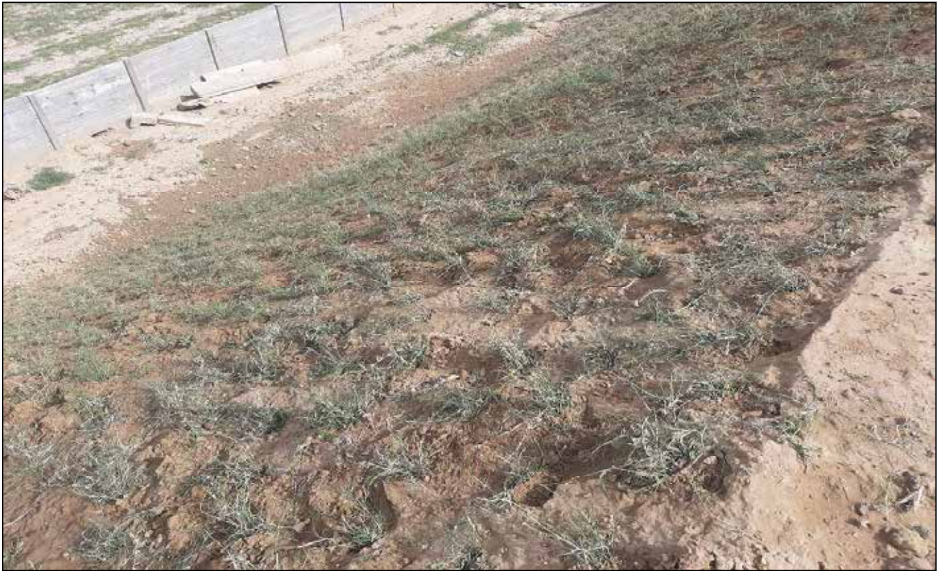
PLACEMENT OF GRASS OVER THE SLOPE
