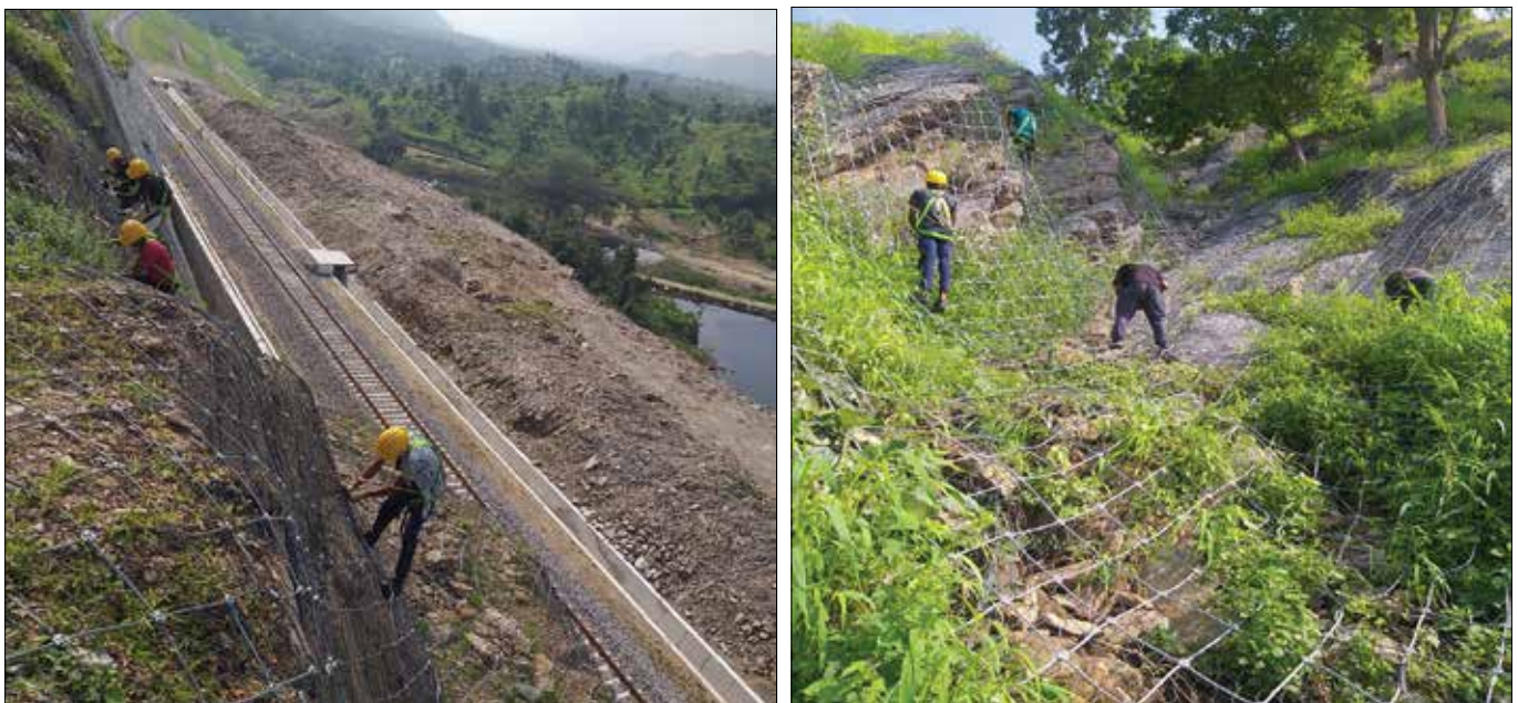
Photo 1 & 2 : Construction Progress: Primary and Secondary Mesh Integration
