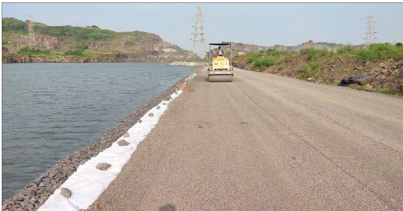
Figure 7 : Compaction behind the wall in progress
