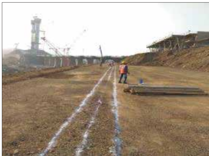
Marking in progress for RS Walls
