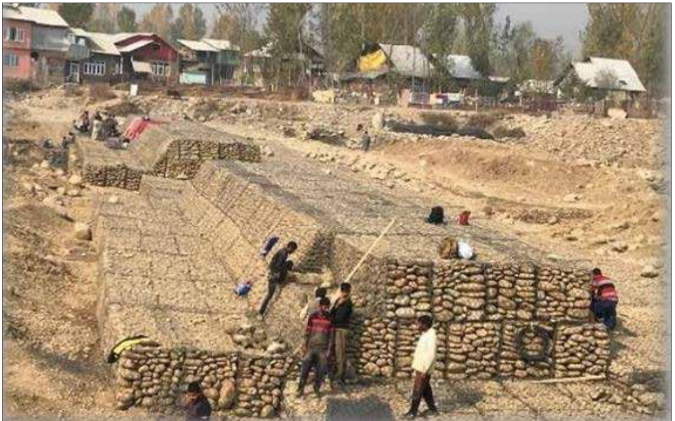
Photo 1: Gabion Installation in progress
