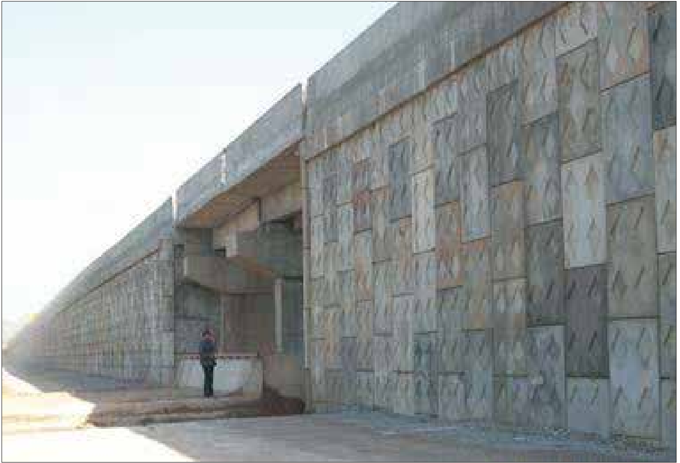
Elevation view of RS wall
