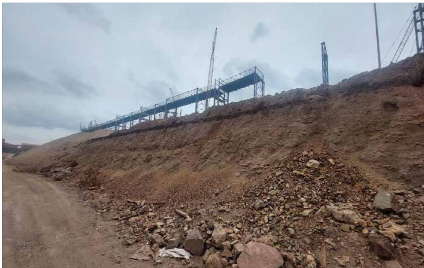
Photo 1 : Pre-Construction Site Condition : Unstable Slope
