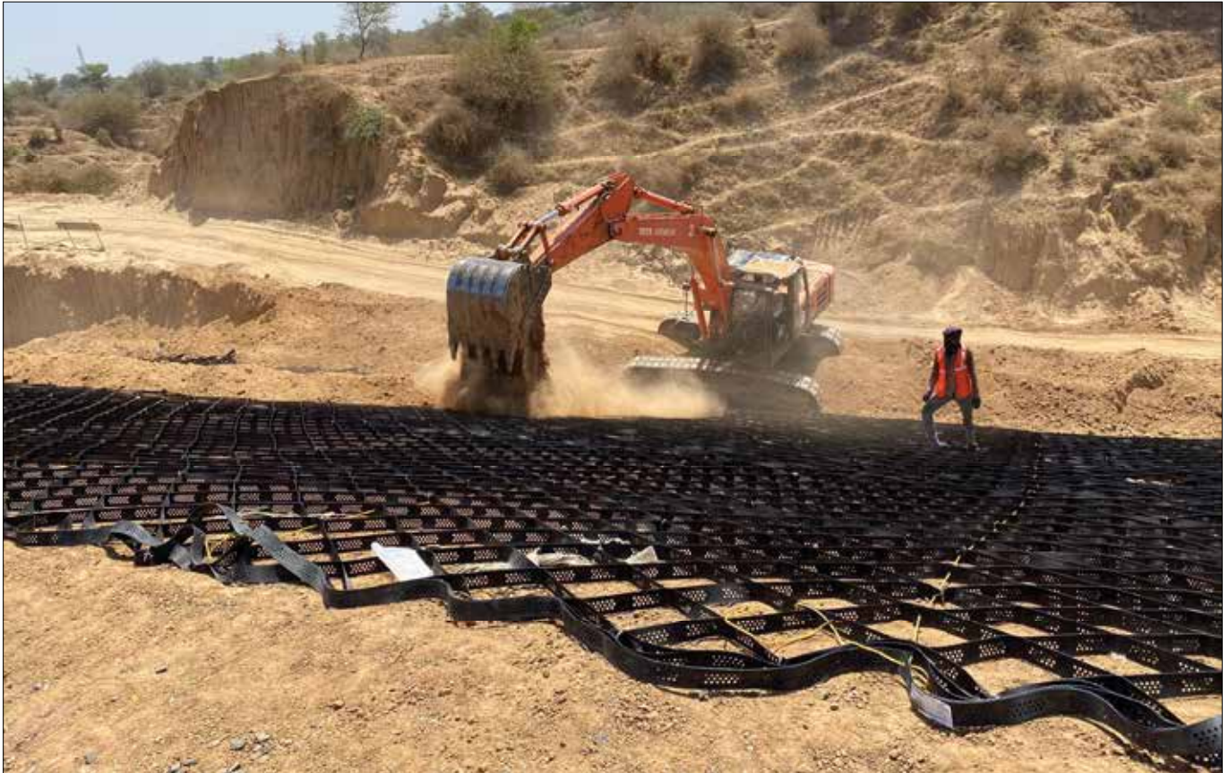
Photo 2 : Filling of vegetative soil in Techcell Geocell
