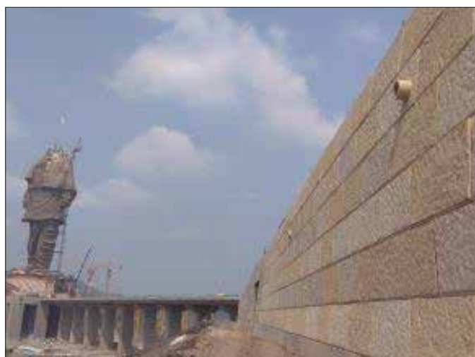
Finished view of RS Wall Panels
