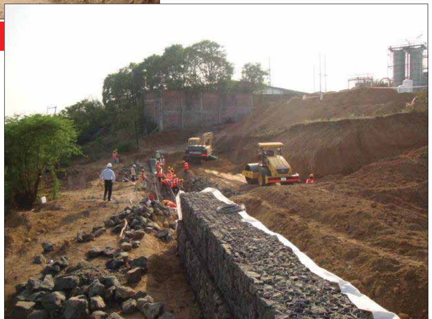
Installation of Gabion fascia units
