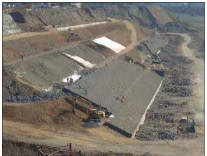
TechFab Metal Gabion Mattress laying in progress
