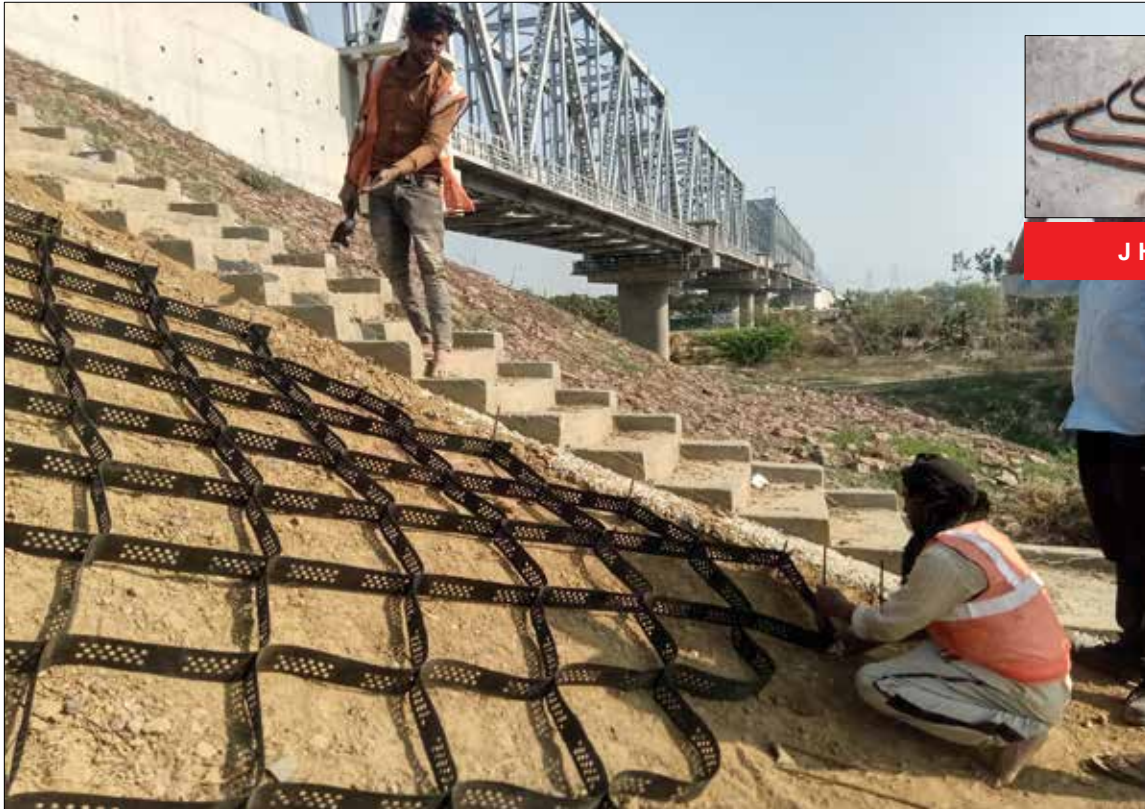
Photo 3 : Anchoring of J Hooks
