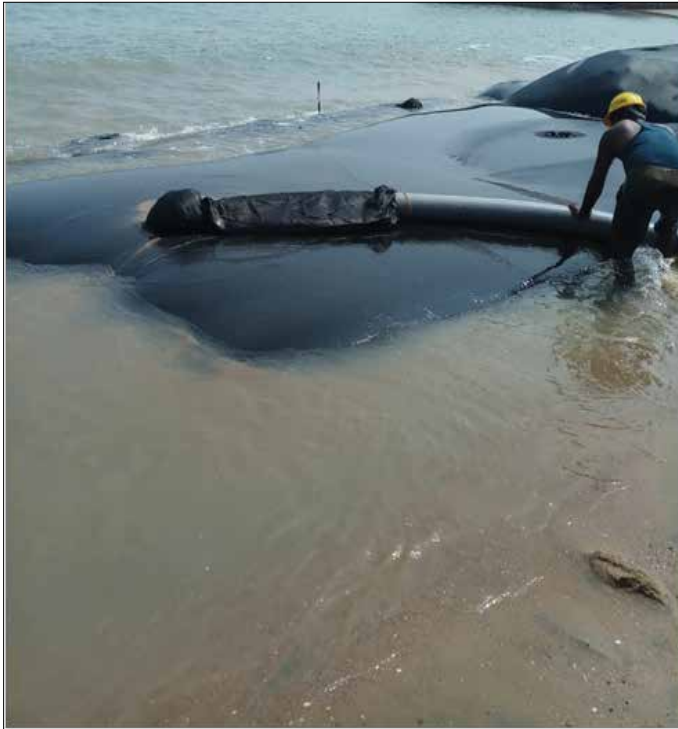
Geotextile Tube filling is in progress
