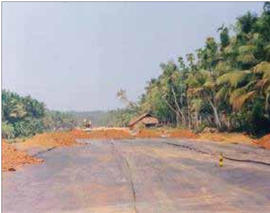
Installation of Techfab TPP 250 Woven Geotextile
