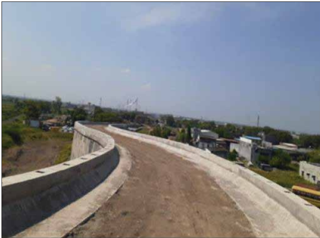
Coping beam installation completed
