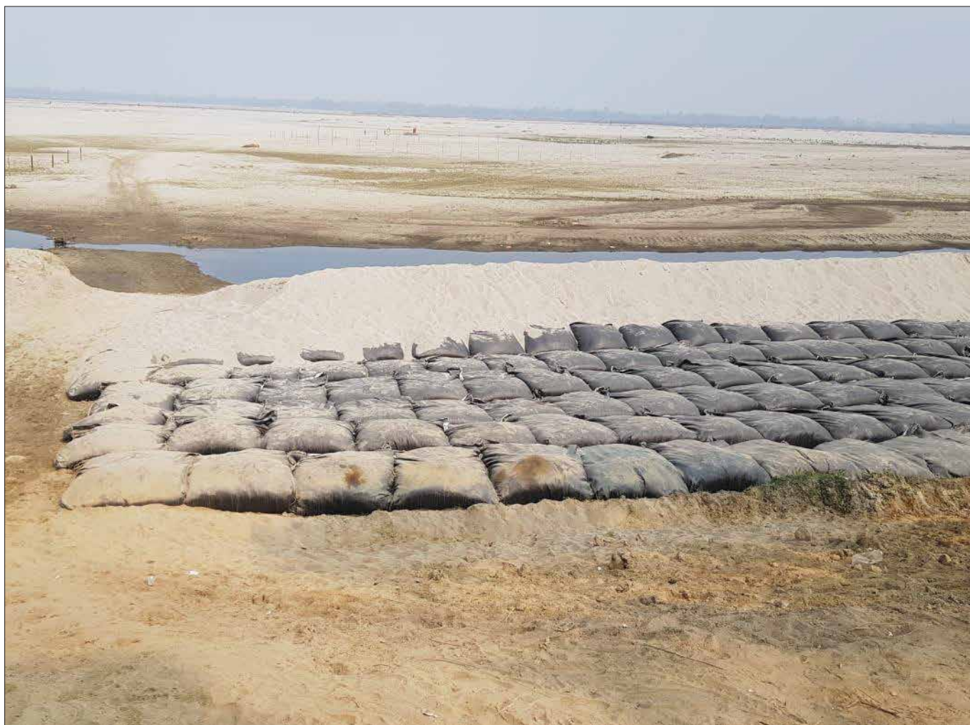
Photo 3 - Placement of Techfab Geotextile bags
