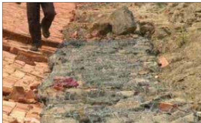
Metal Gabion Placed at Bottom Trench
