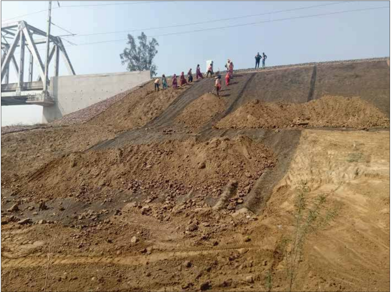
Photo 6 : Spreading the Vegetative Soil evenly over Geogrid
