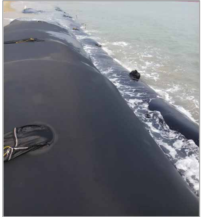
Filled first layer of Geotextile Tube
