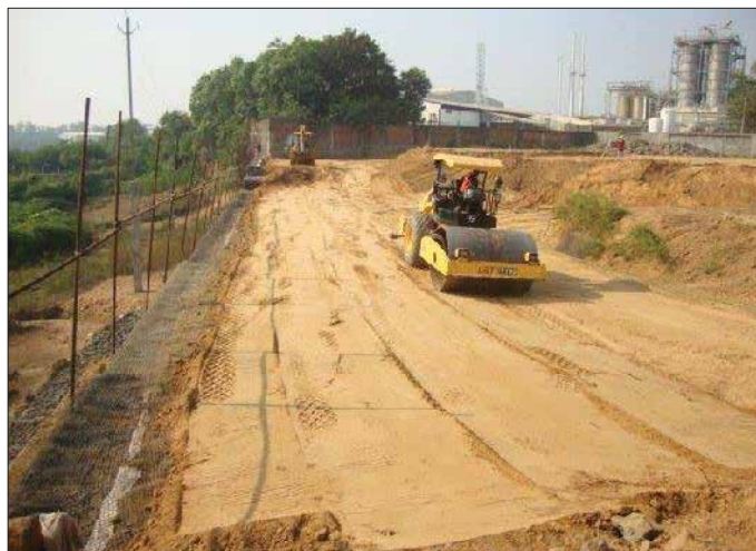
Compaction behind the wall
