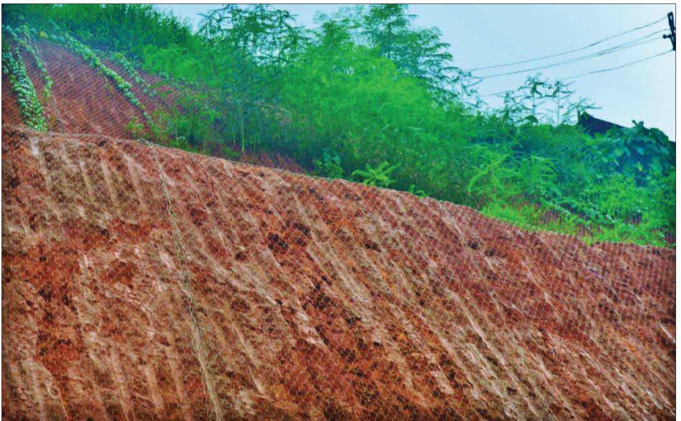
Slope after installation of Rockfall Netting
