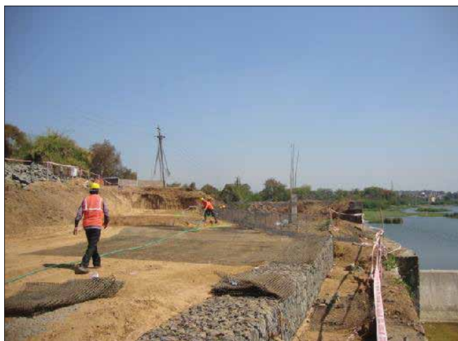
Installation of TechGrid Geogrid
