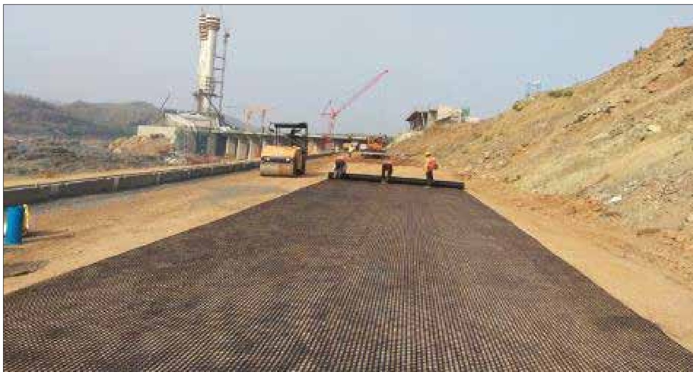
Laying of TechGrid Geogrid in Progress
