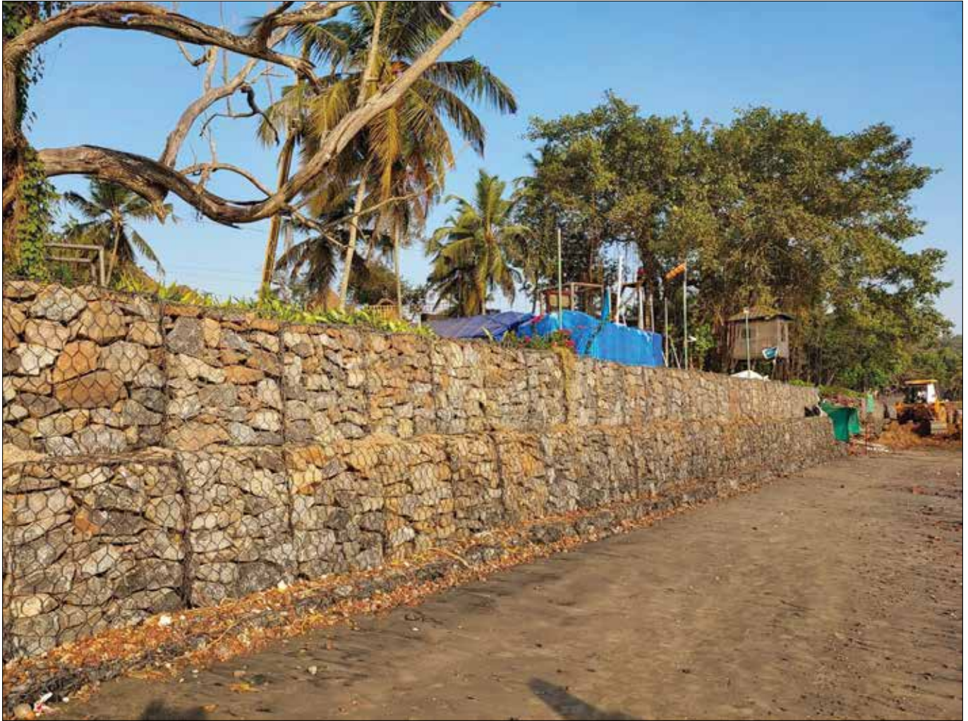
Completed Structure of Gabion Wall
