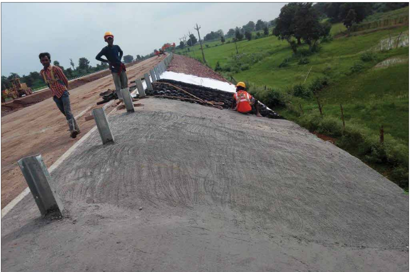
Progress of Concrete filling in Geocell
