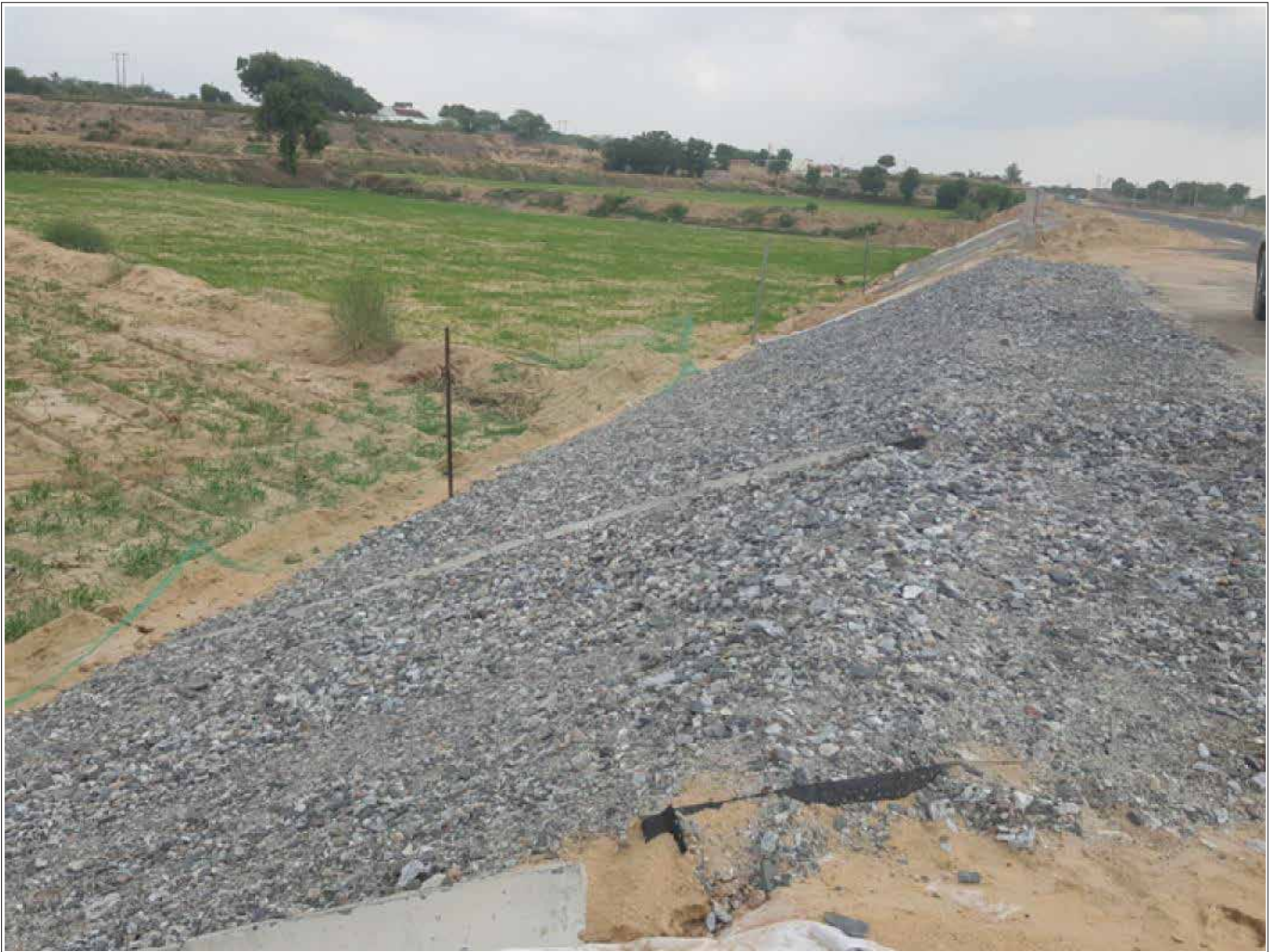
Slope is ready and filled with GSB
