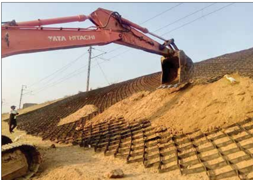
Photo 4 : Placing Vegetative Soil onto the Geocell
