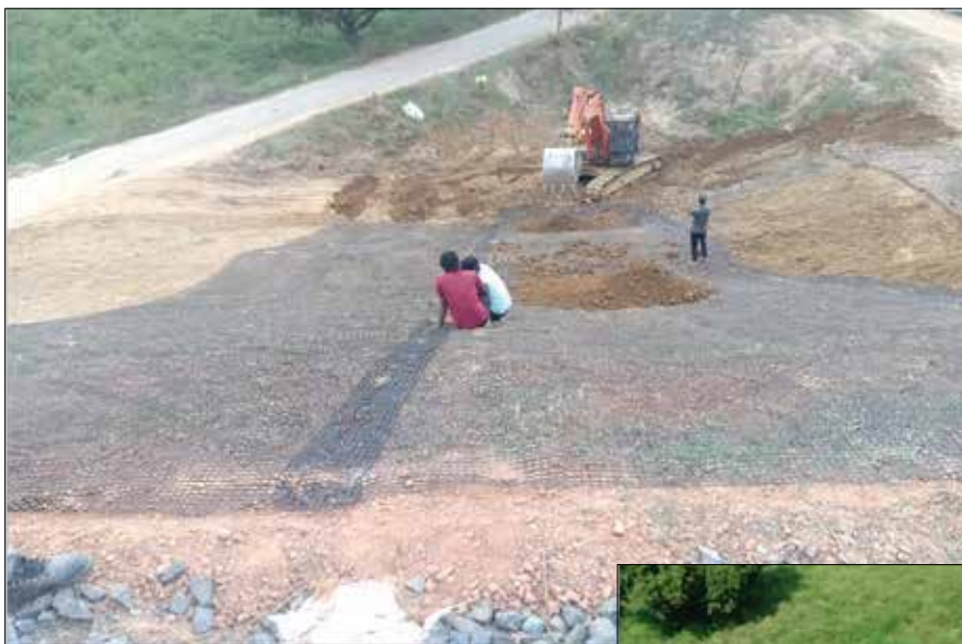
Photo 4 : Placing Vegetative Soil over Geogrid
