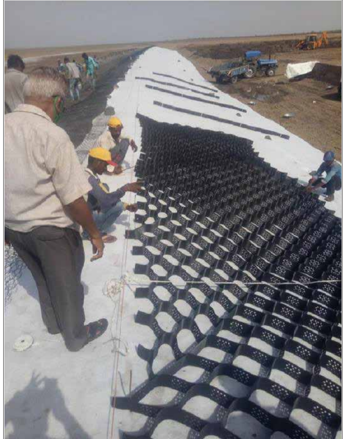
Techcell Geocell installation in progress
