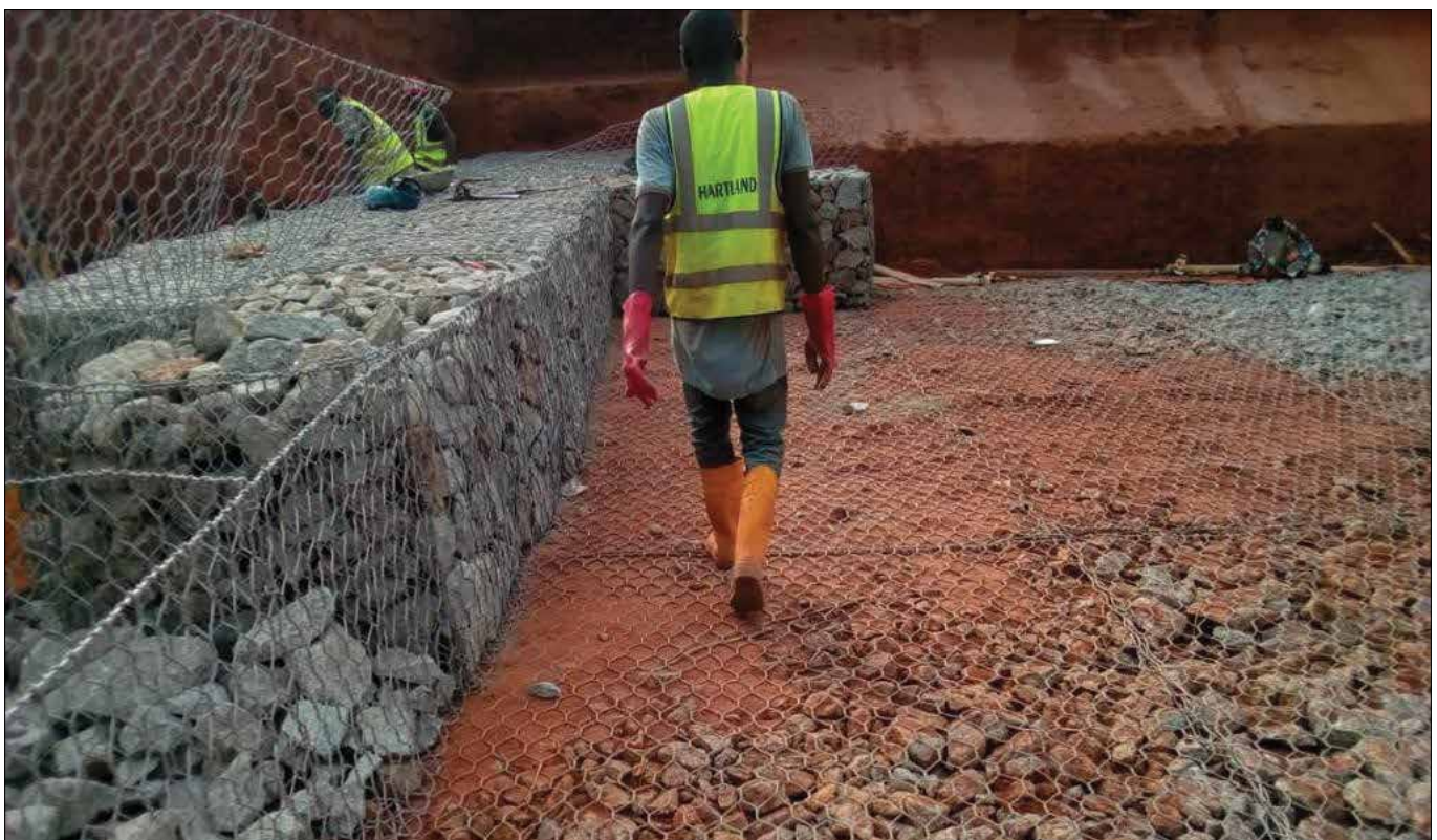
During Construction Photographs - Gabion filling with boulders
