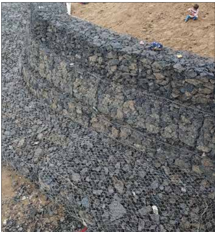
Photo 3 & 4 : Completed Structure - TechFab Metal Gabion & Mattress
