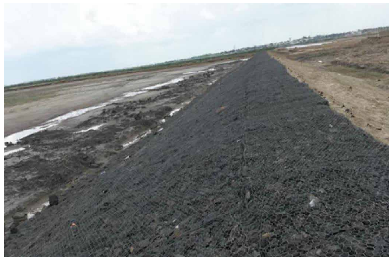
Sea side slope with Metal Gabion Mattress
