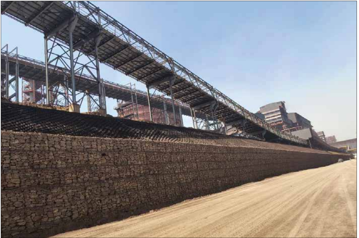
Photo 5 : Installation of Geocell above Gabion Wall
