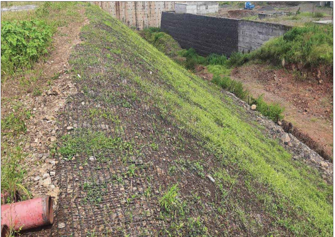
Slope after installation of Geogrid
