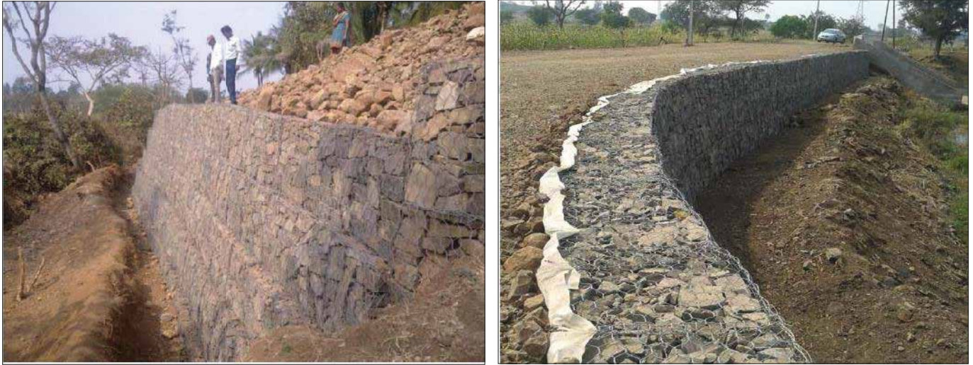
TechFab Metal Gabion Installation Photographs
