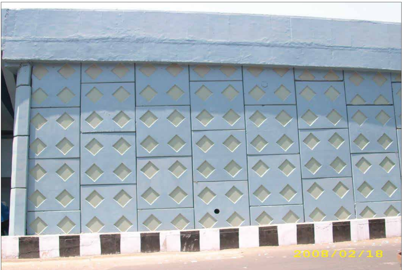
Elevation view of RS wall
