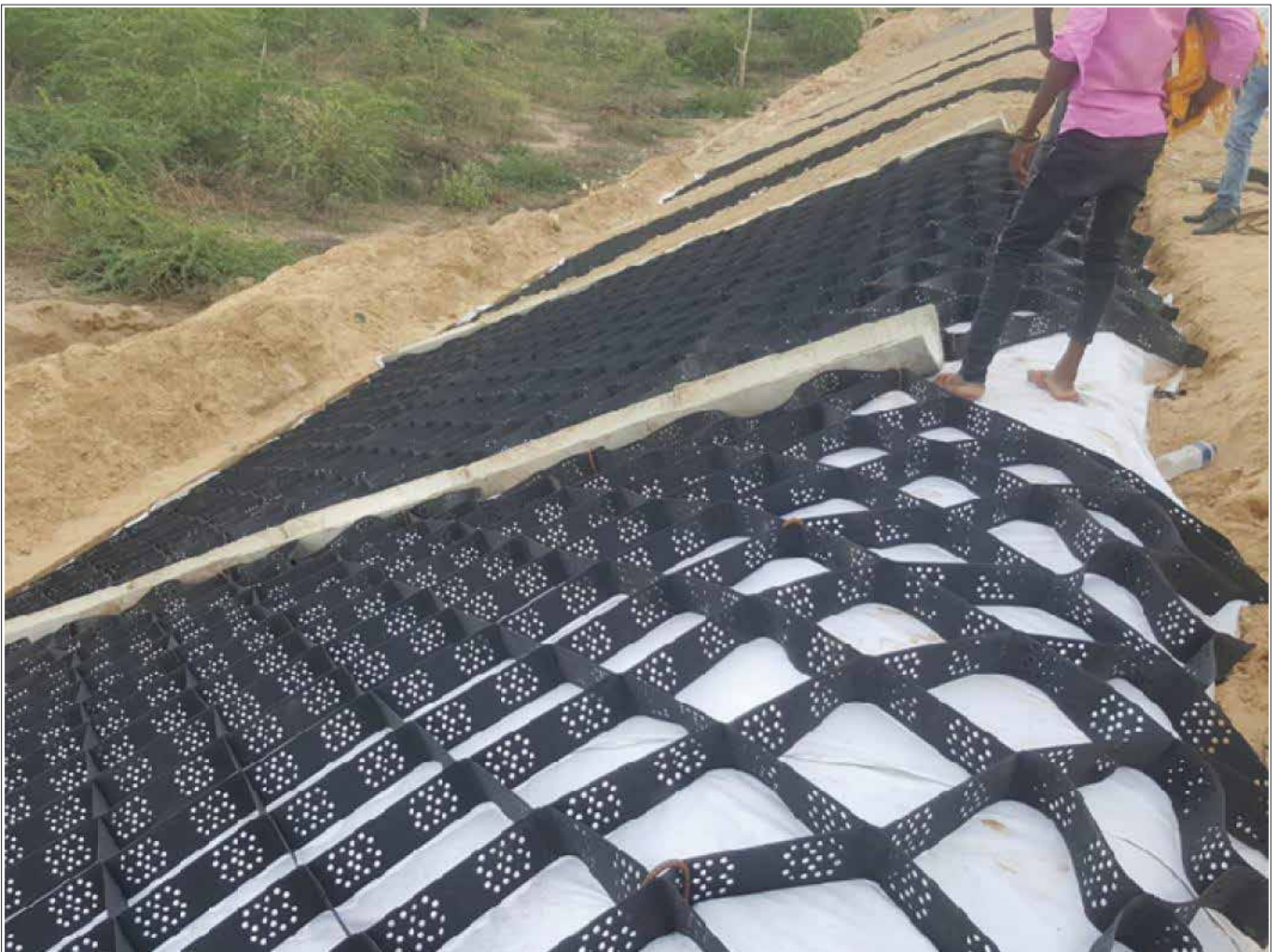
Installation of Nonwoven Geotextile & Geocell completed
