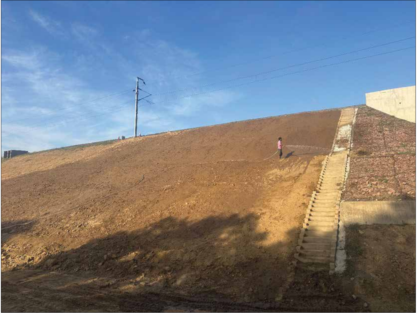
Photo 6 : Slope After Application of Vegetative Soil
