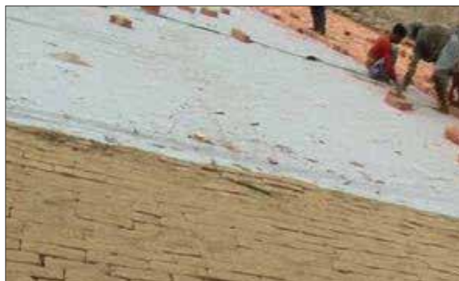
Unrolling of TechGeo Nonwoven Geotextile
