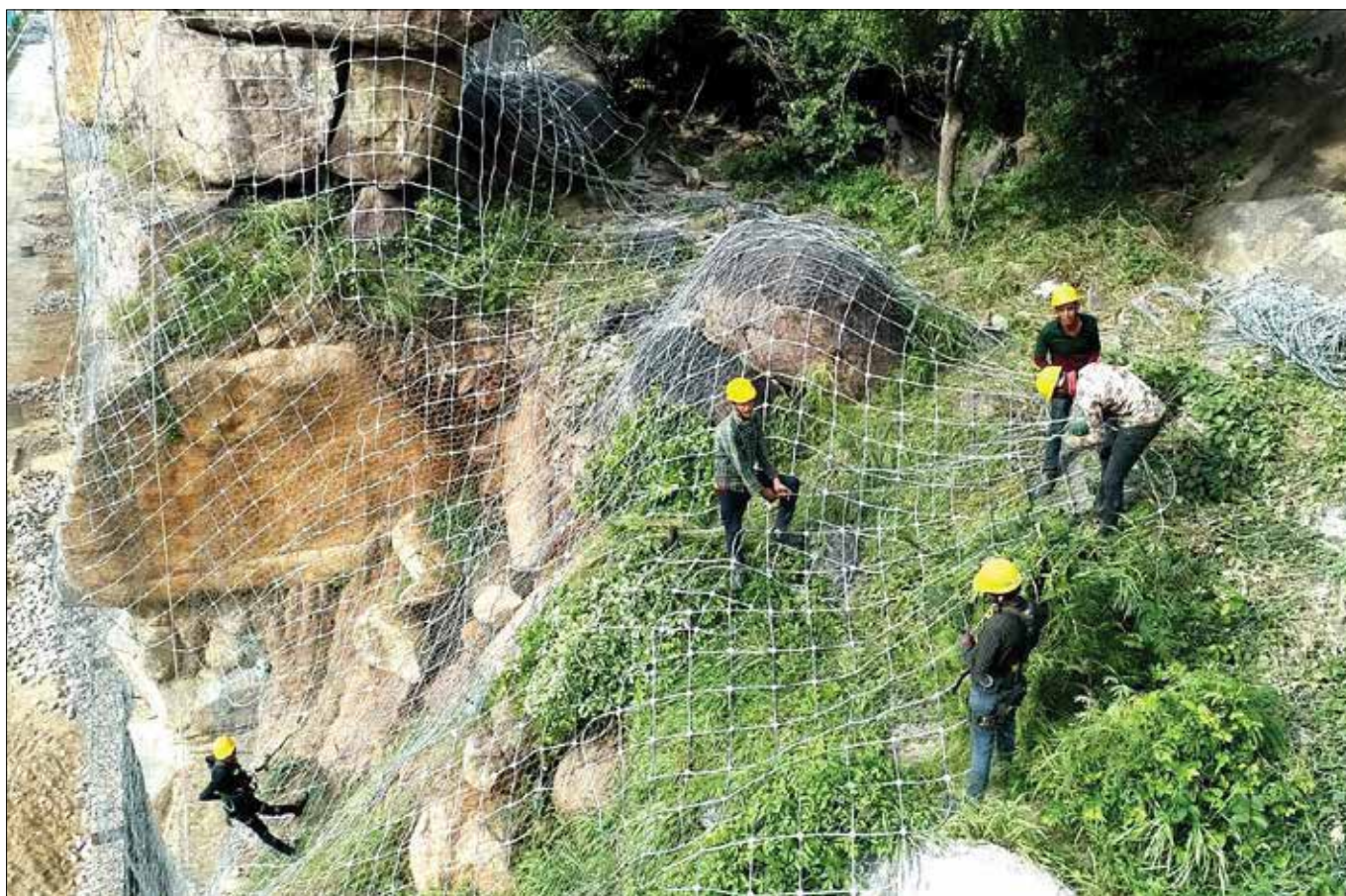
During Construction Photographs (Installation of TechRhombus)
