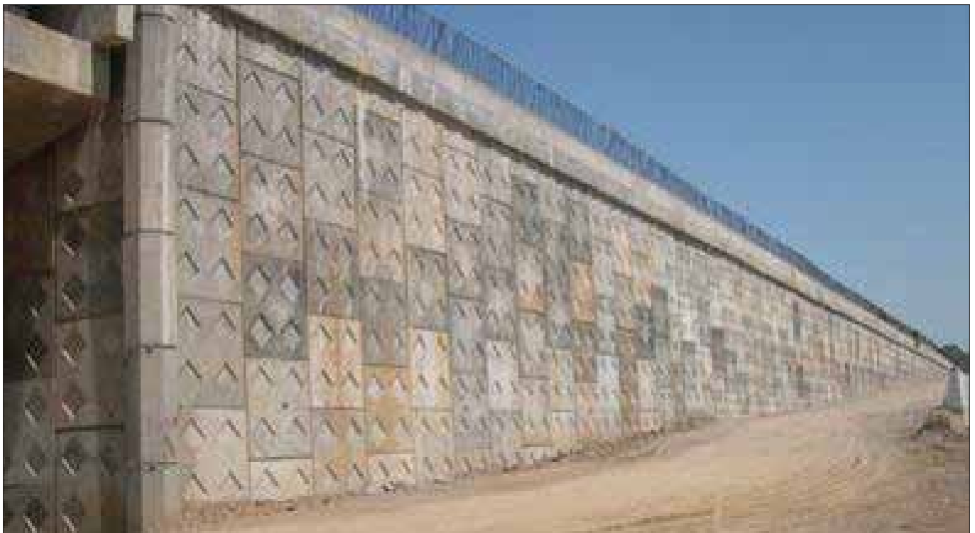
Photo 1 : Elevation view of RS Wall
