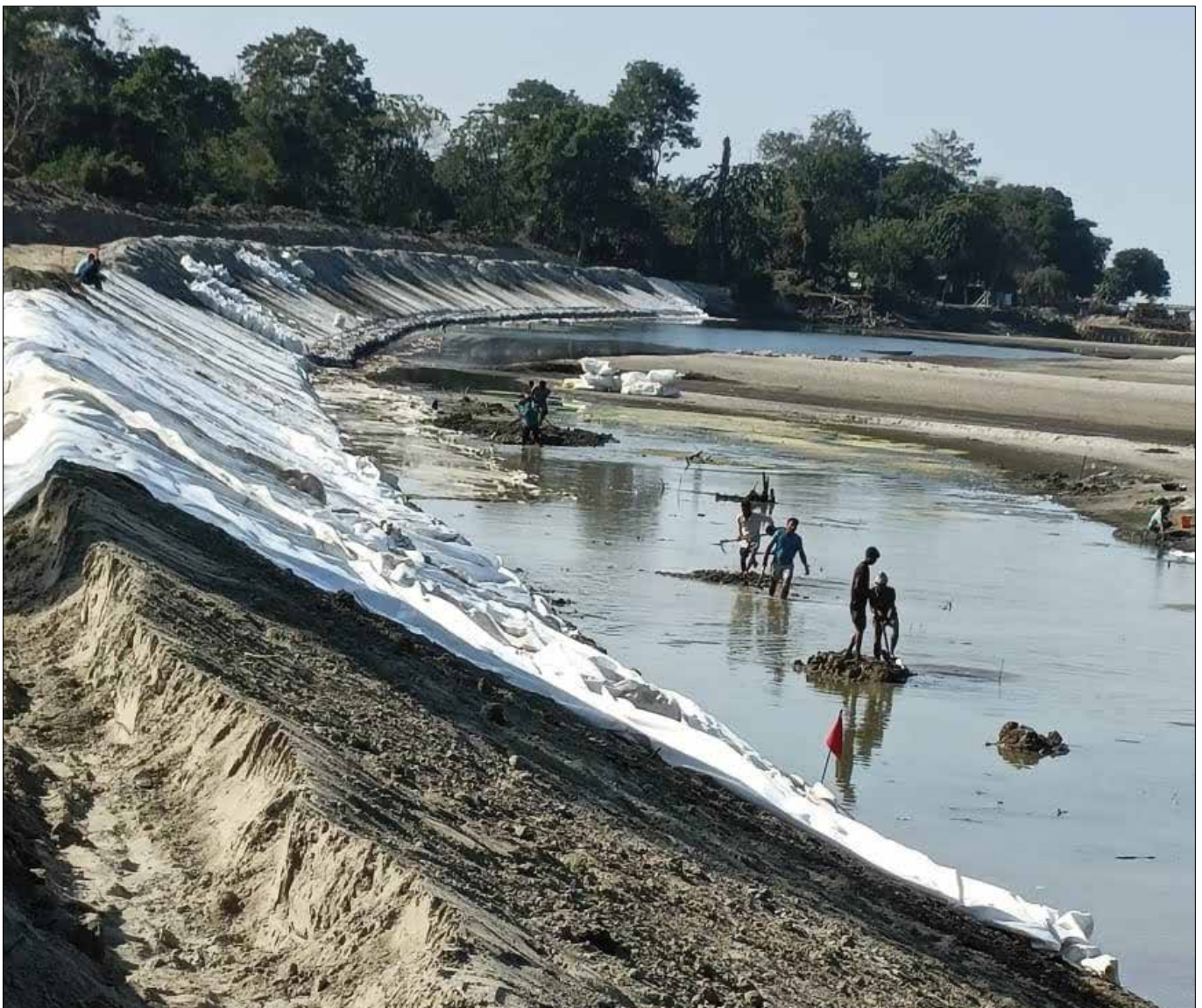
Photo 2 : Laying of TechGeo Nonwoven Geotextile on Dressed Slope
