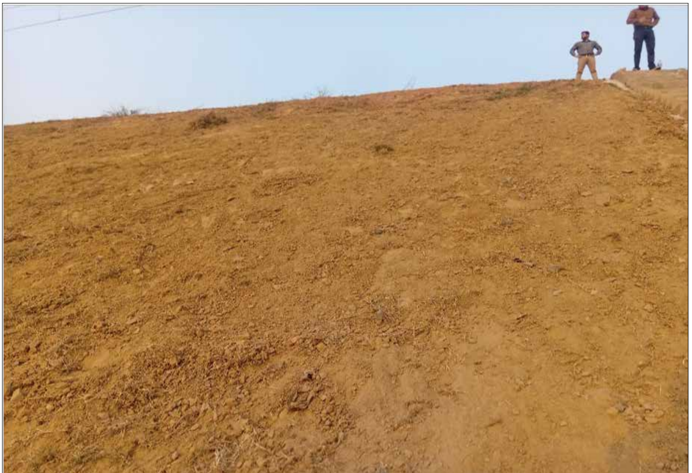
Photo 1 : Preparation of Slope (1V : 2 H)
