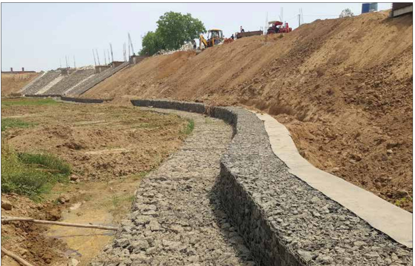
Photo 2 : Installation of Gabion Toe Wall
