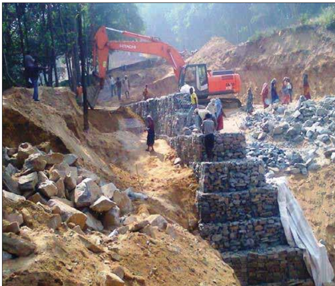
Photo 1 & 2 : TechFab Metal Gabion Installation in progress
