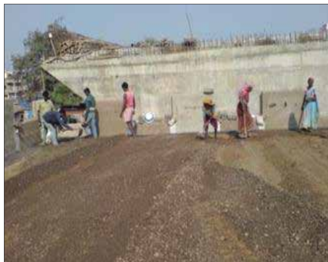
Erection of RS Wall
