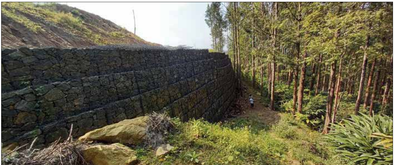
Photo 1 : View of TechFab Metal Gabion Retaining Wall
