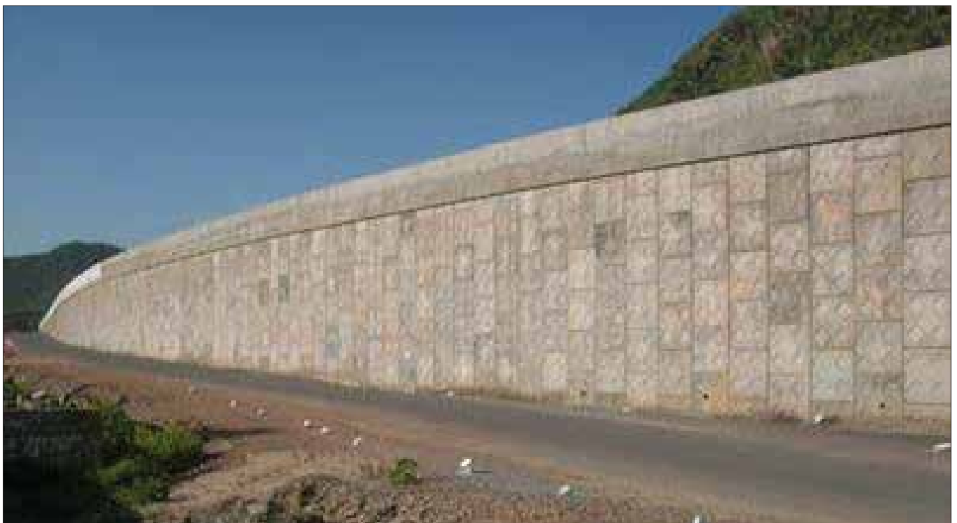
Photo 1 : Elevation view of RS Wall
