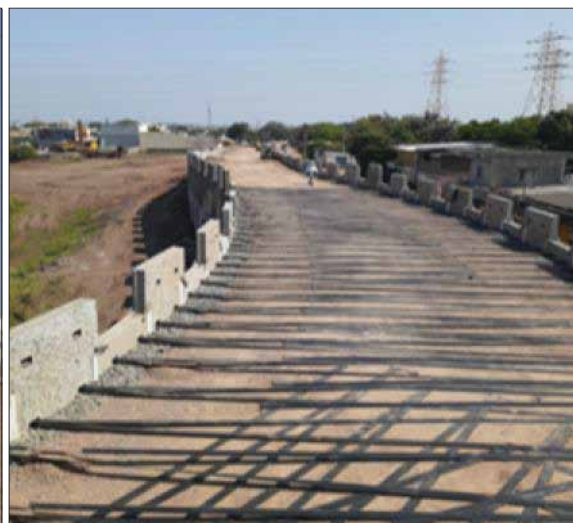
Installation of top layer TechStrap Polymeric Strip
