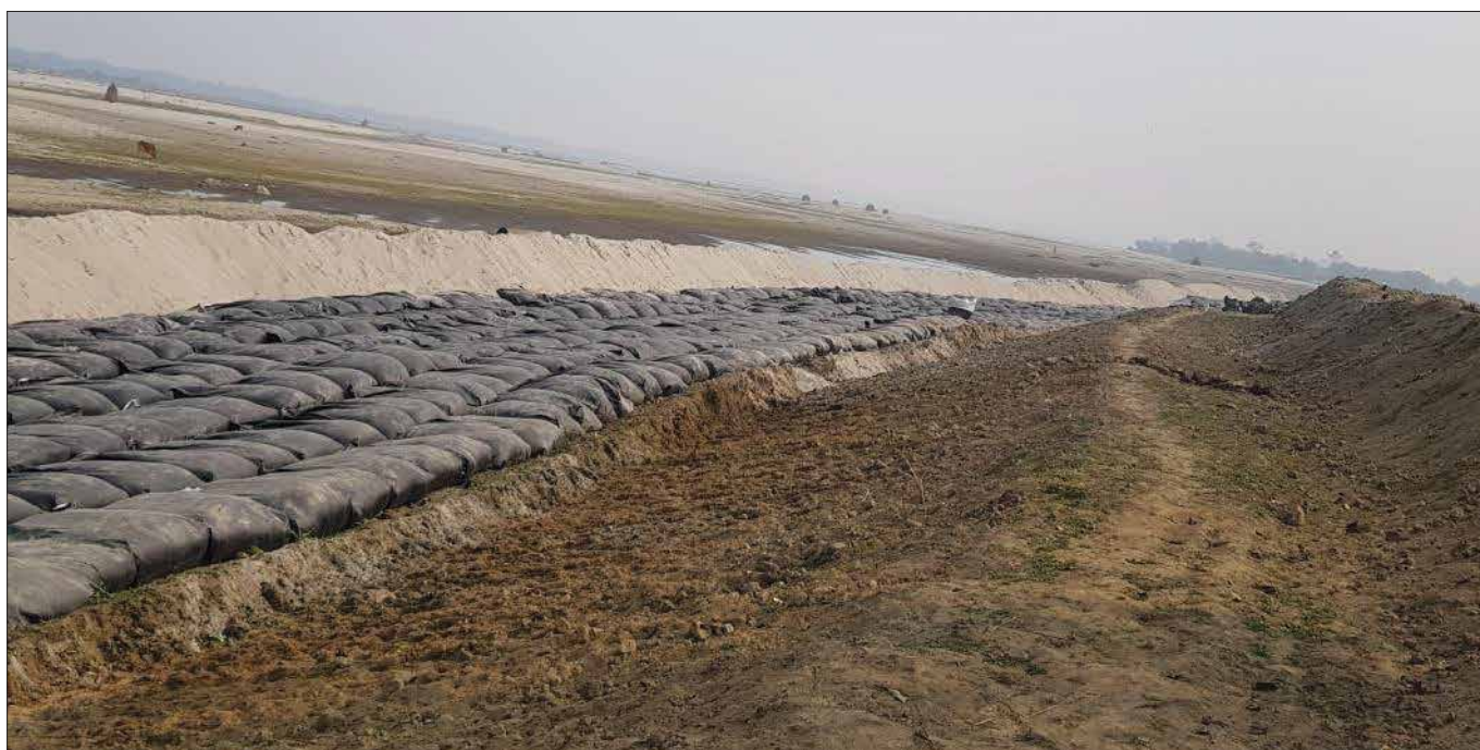
Photo 1 & 2 - Filling & Placement of TechFab Geotextile bags
