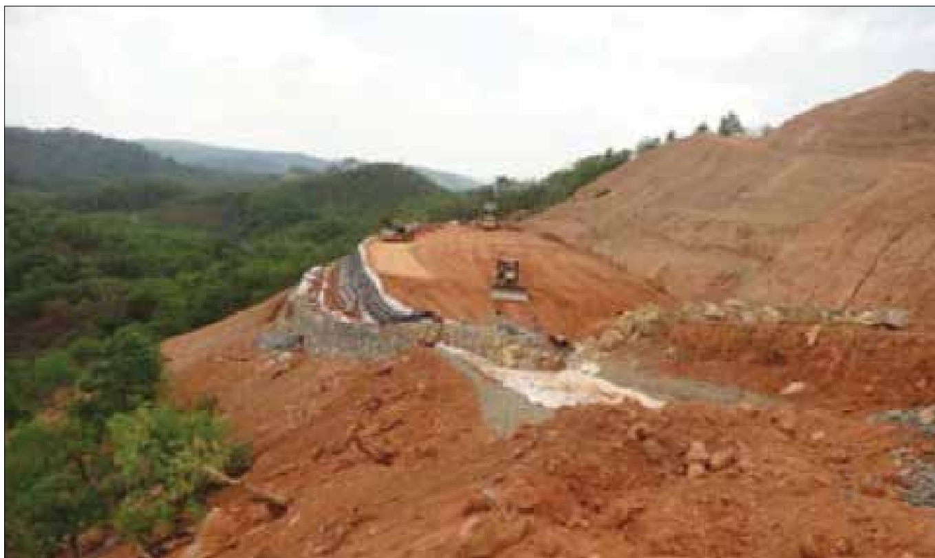
TechFab Metal Gabion Wall Layout – Initial Stage
