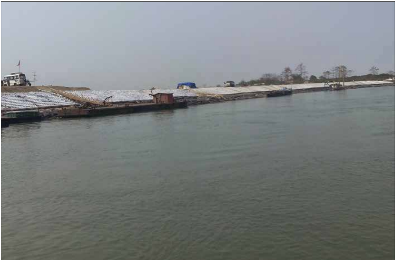
Photo 4 & 5 : Laying of Geotextile Bags on Slope
