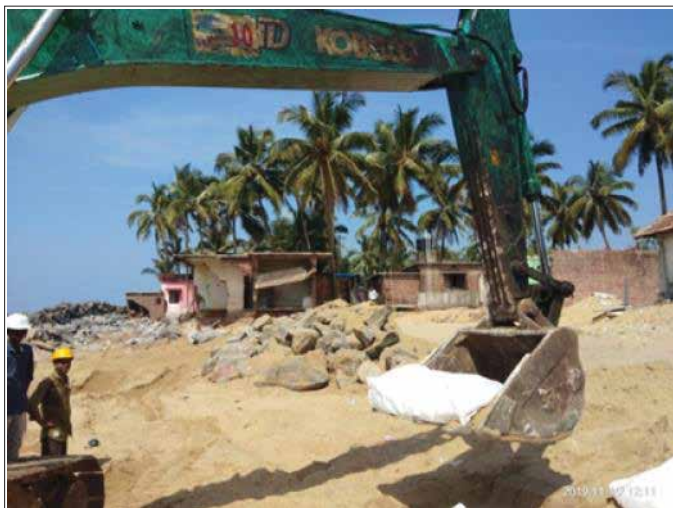
Dumping of Geotextile bags in progress
