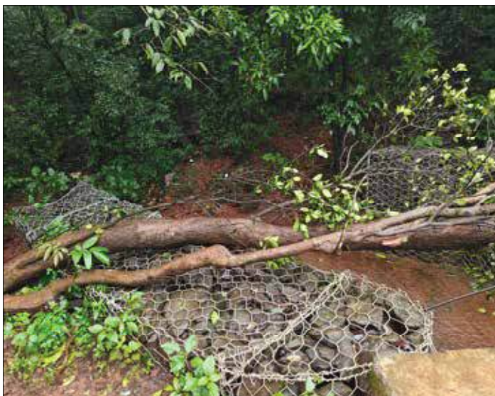
Photo 1 & 2 : View of TechFab Metal Gabion Retaining Wall
