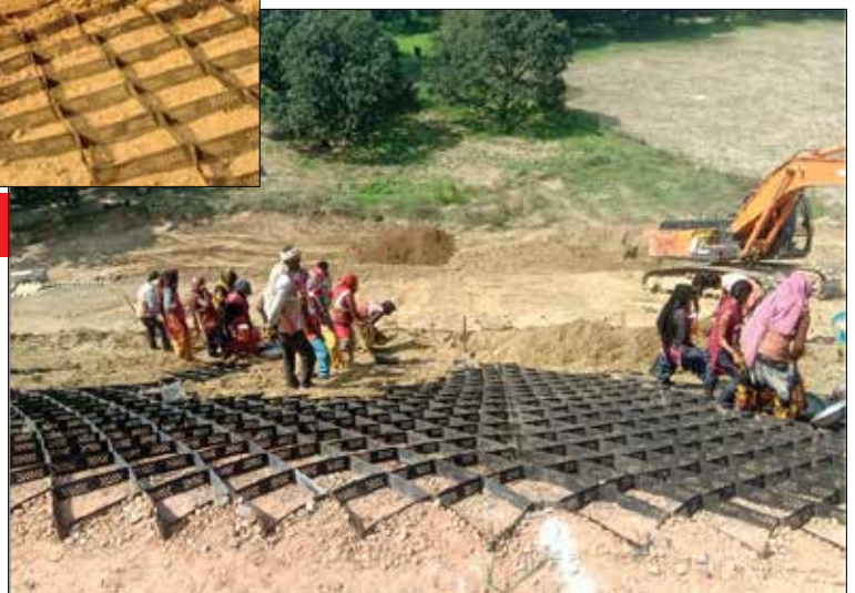
Photo 5 : Spreading the Vegetative Soil evenly over the Geocell
