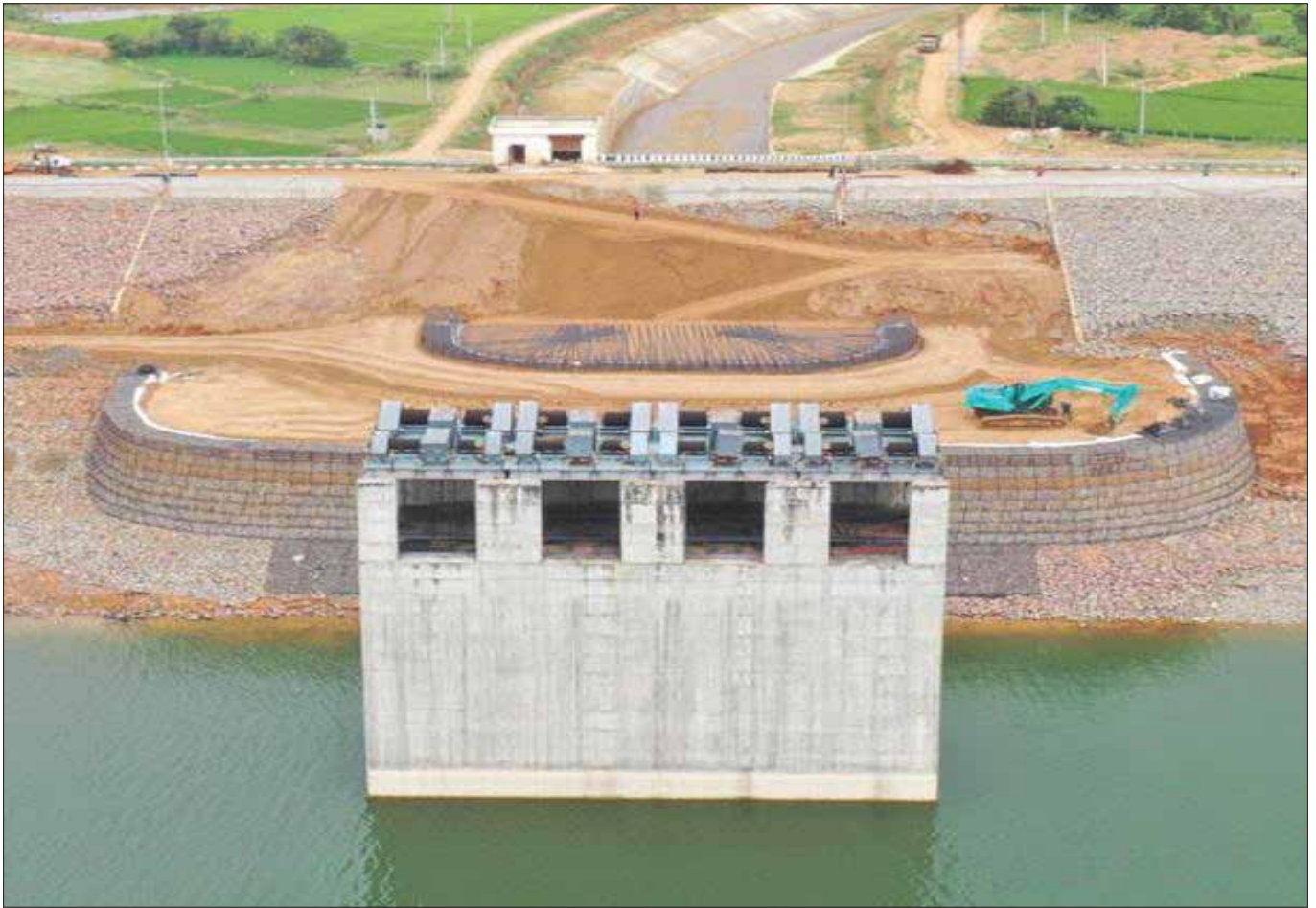
Photo 2 : During Construction - TechStrap Geostrips installation
