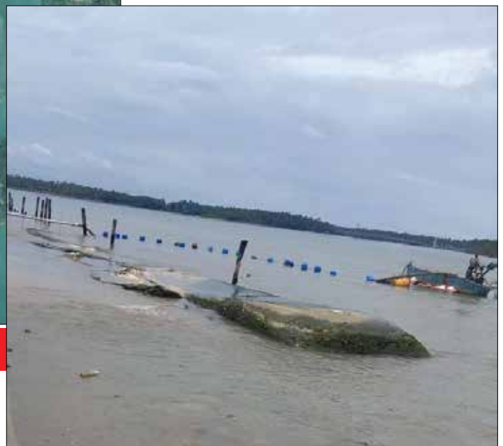
Damaged existing Geotextile Tubes
