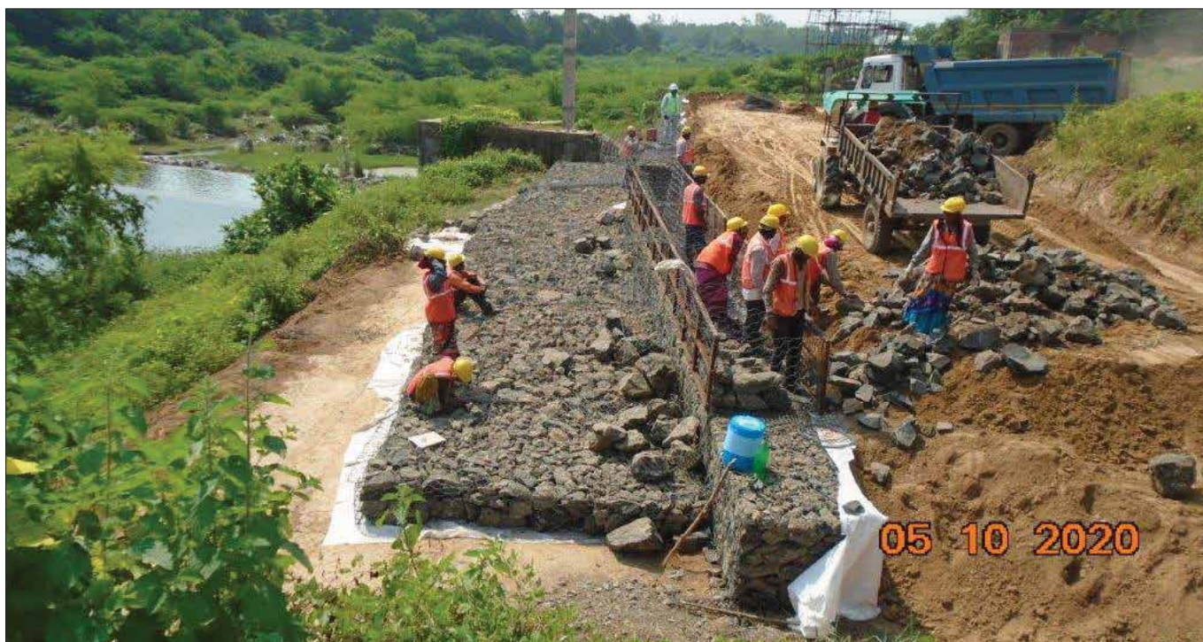
Work under Construction - Gabion Facia & Mattress Installation
