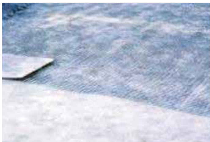
Laying of TechGrid TGU-40 as Basal Reinforcement
