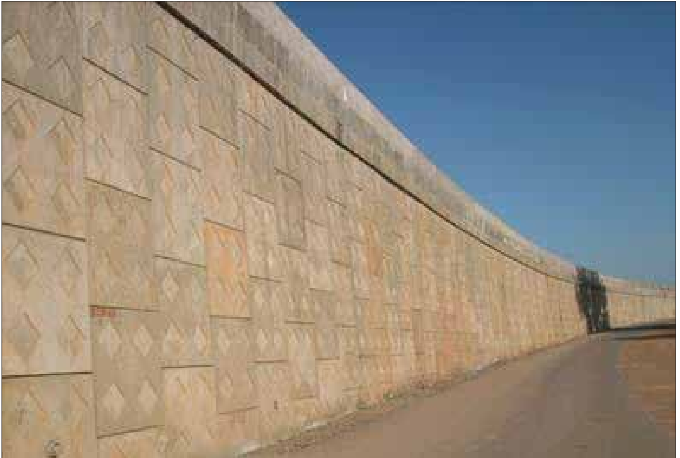
Elevation view of RS wall
