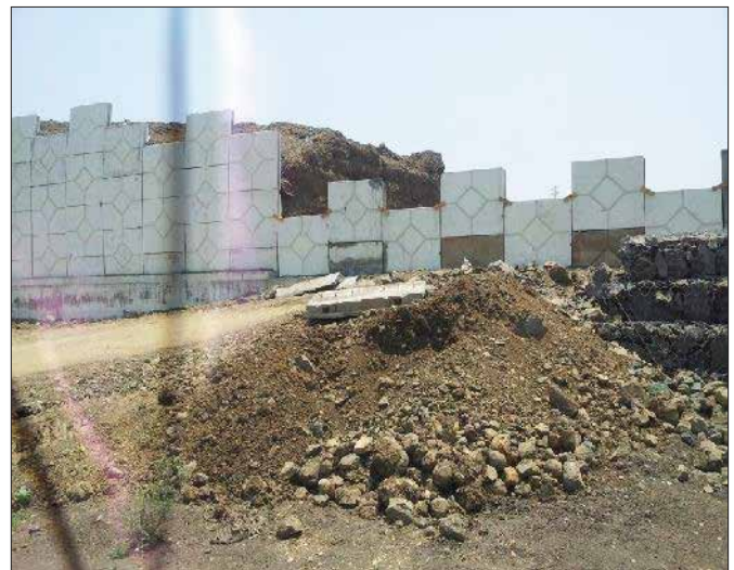
TechFab Reinforced soil wall - Installation
