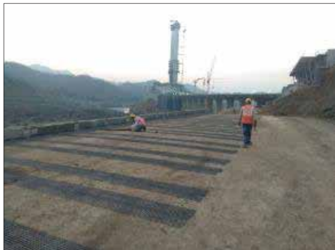
Geogrid Laying for RS Walls
