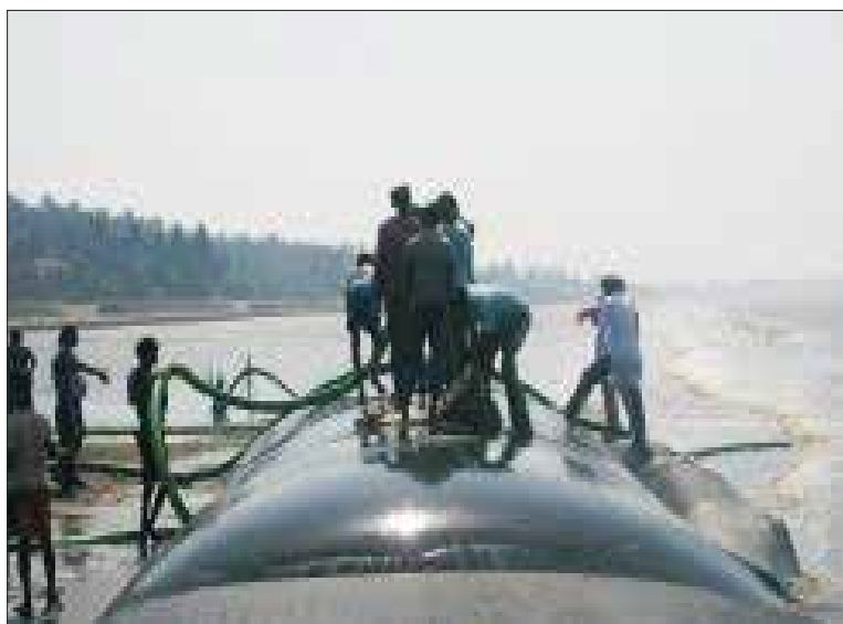
Installation of TechTube
