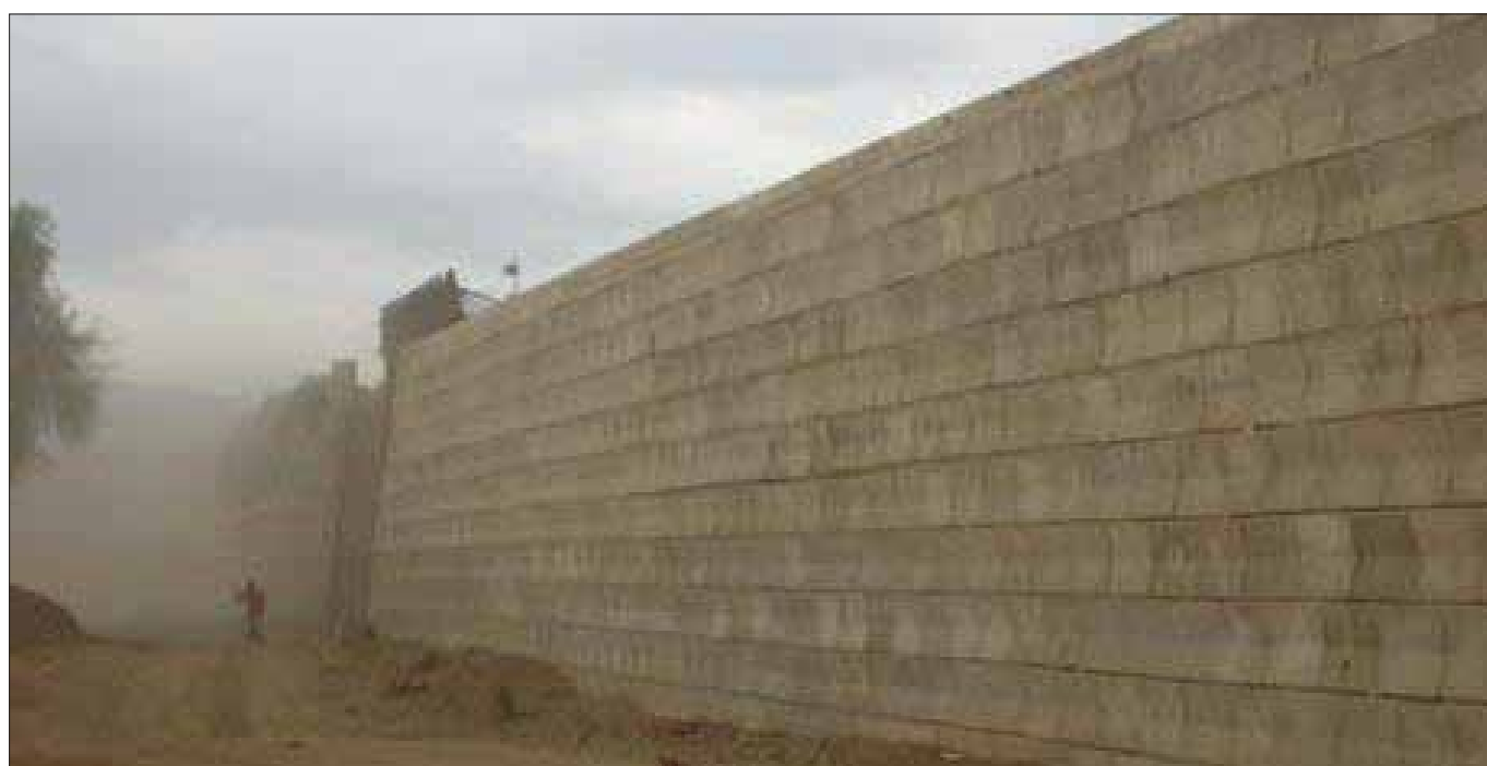
Photo 2 : Elevation view of RS wall
