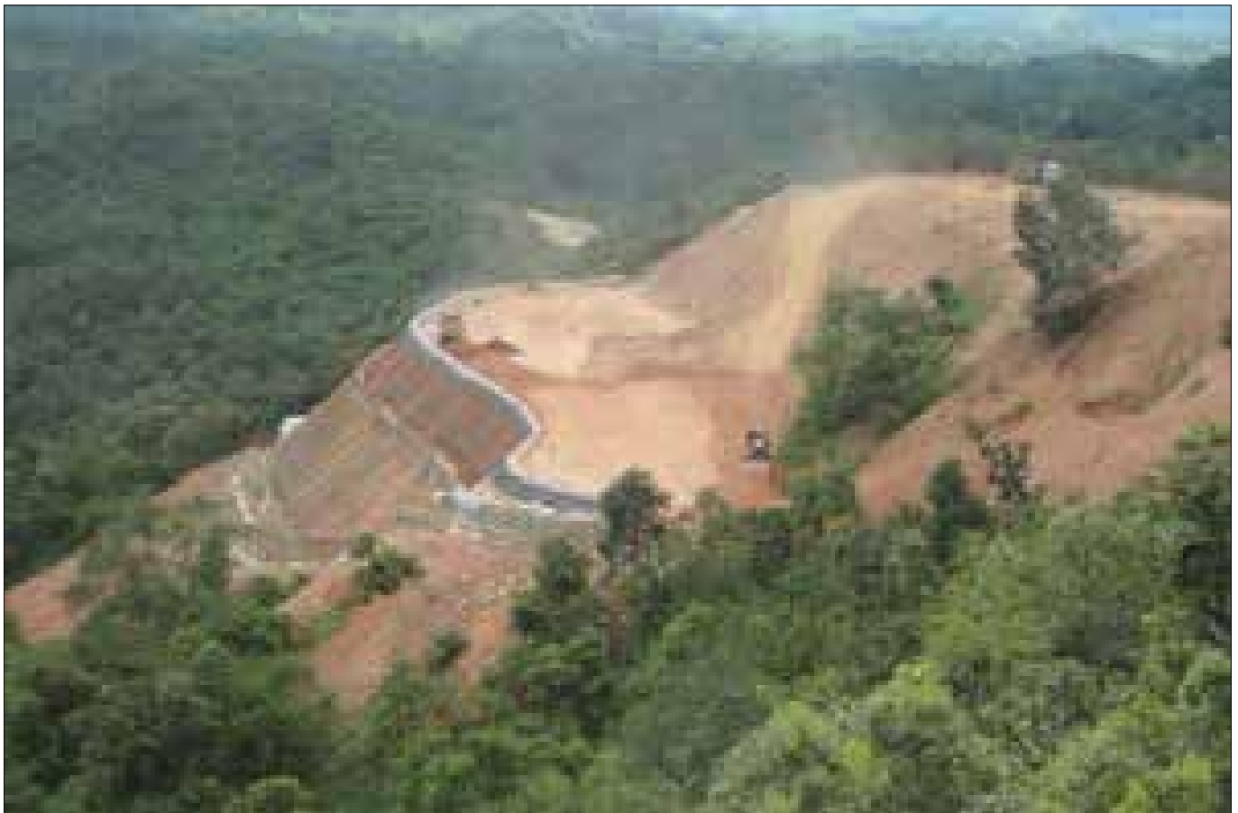
RSS with TechGrid GeoGrid – Under Construction
