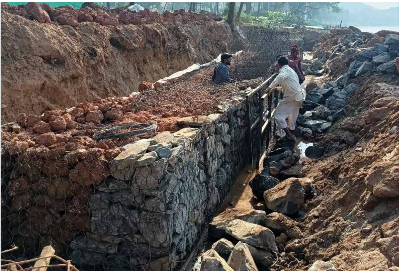
During Construction Photographs. Back side filling of units done with locally available lateritic boulders
