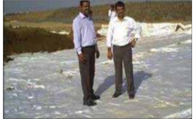
Laying of High Strength Geotextile TFI 3200
