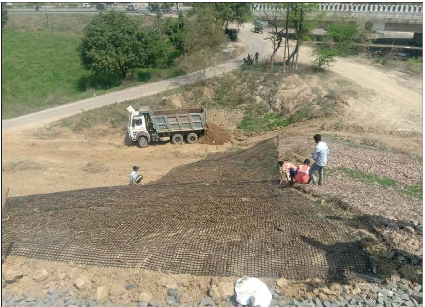
Photo 2 : Spreading of Geogrid on Slope Surface
