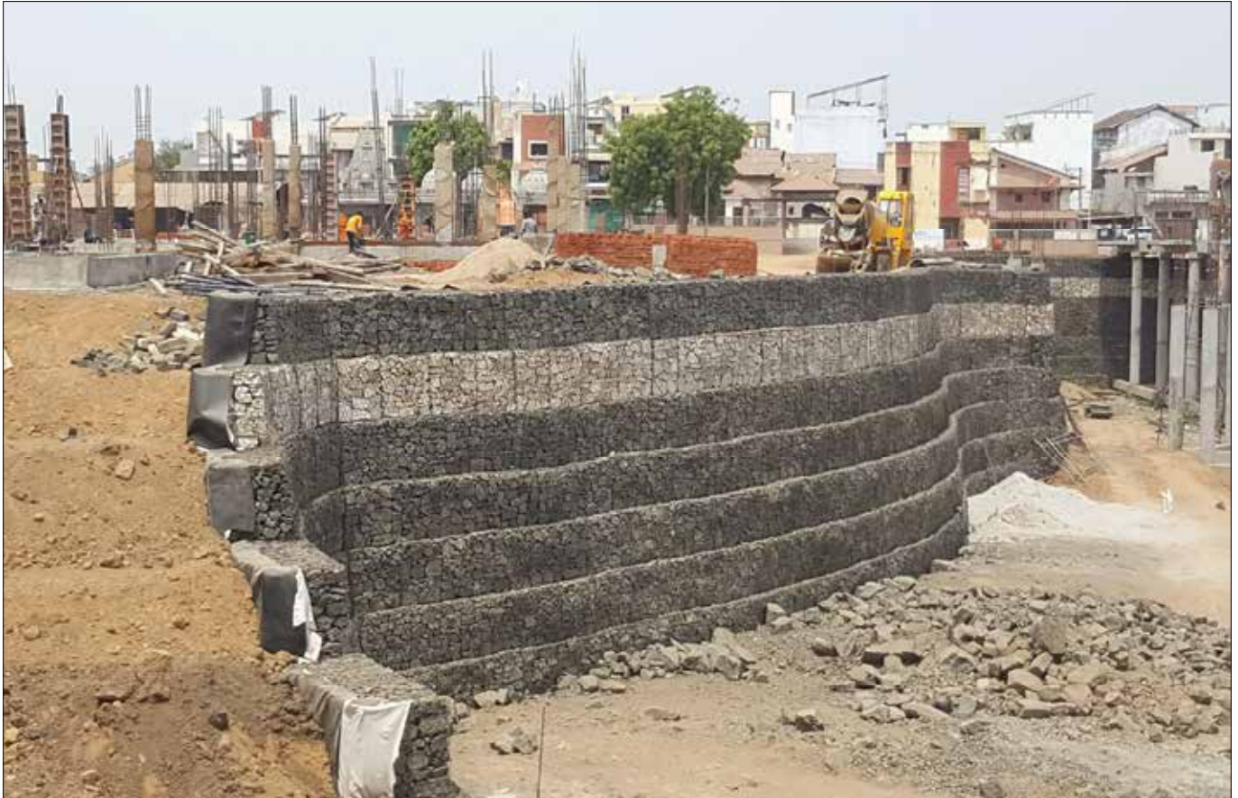
Photo 1 : Installation of Gabion Retaining Wall
