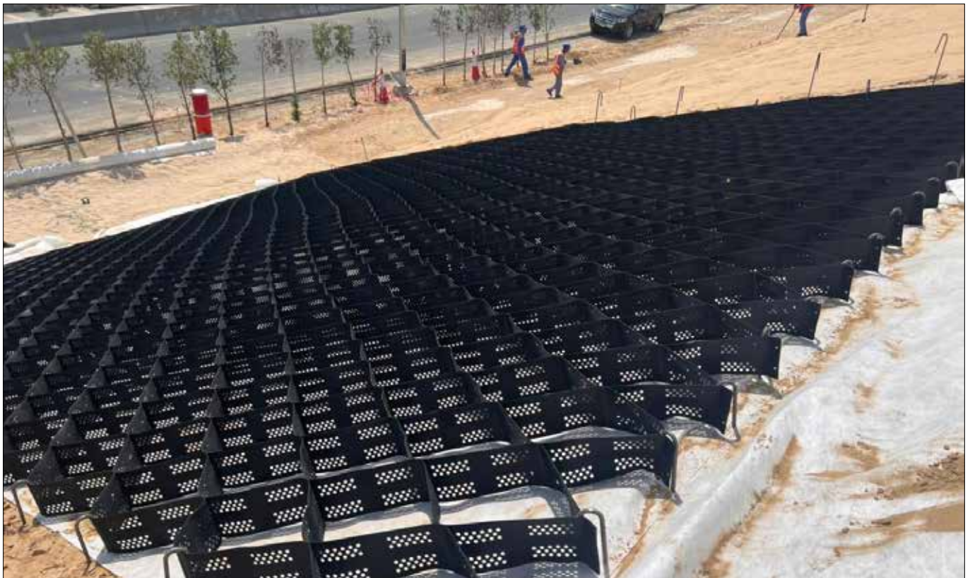
Photo 1 : Installation of Techcell Geocell over the slope
