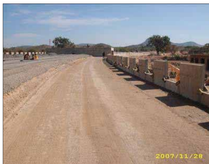
Photo 2 & 3: Erection of RS wall
