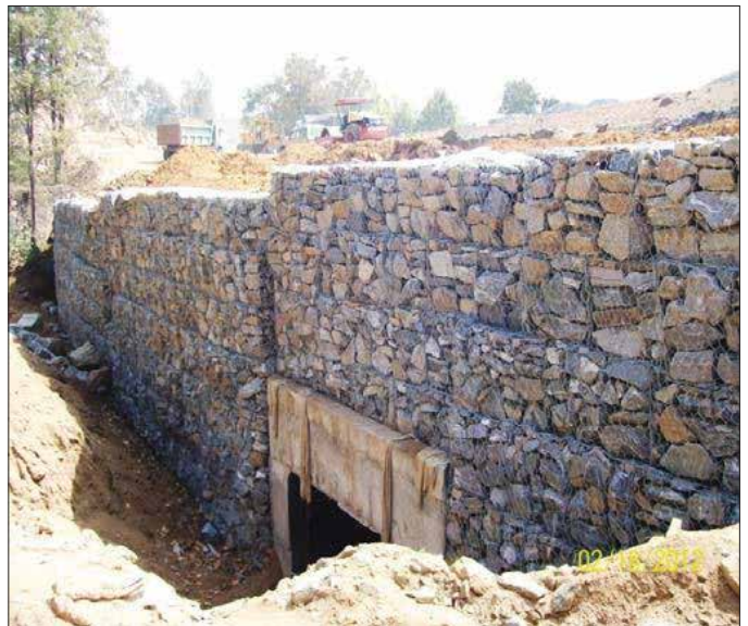
Photo 1 & 2 : TechFab Metal Gabion Installation in progress
