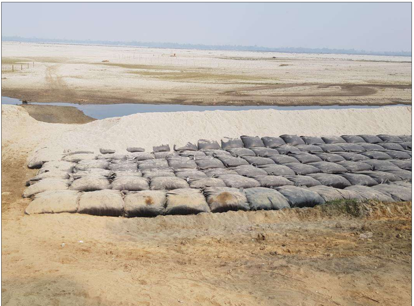
Photo 3 - Placement of Techfab Geotextile bags
