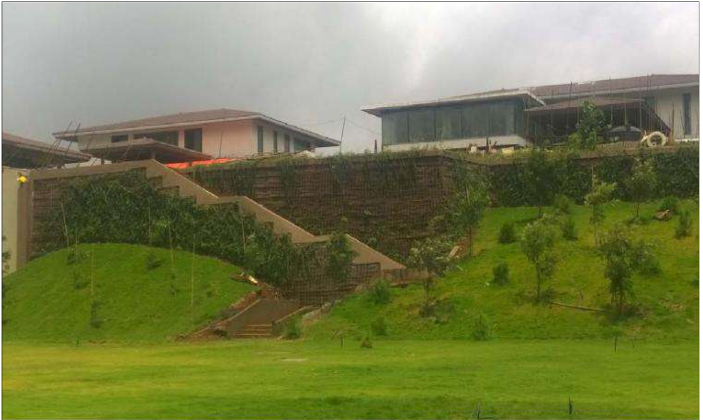
After Completion of Project with full vegetation
