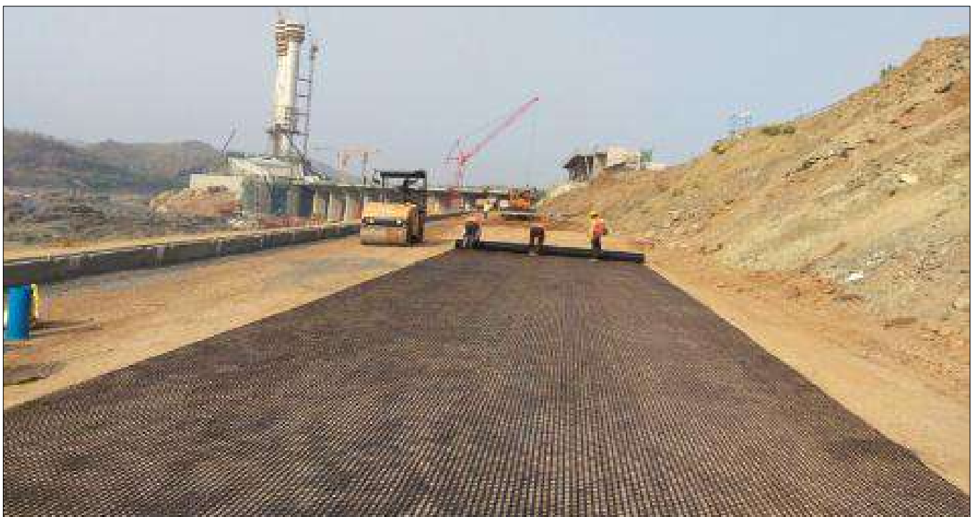
Laying of TechGrid Geogrid in Progress
