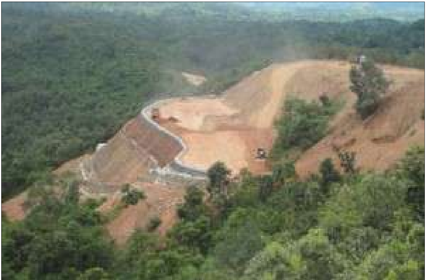
RSS with TechGrid GeoGrid – Under Construction
