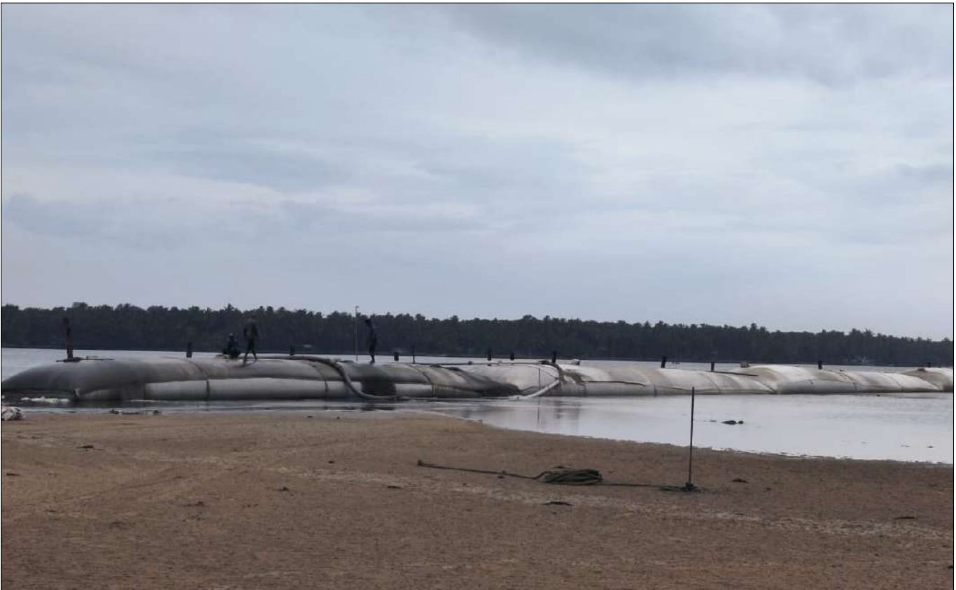
During Construction Photographs
