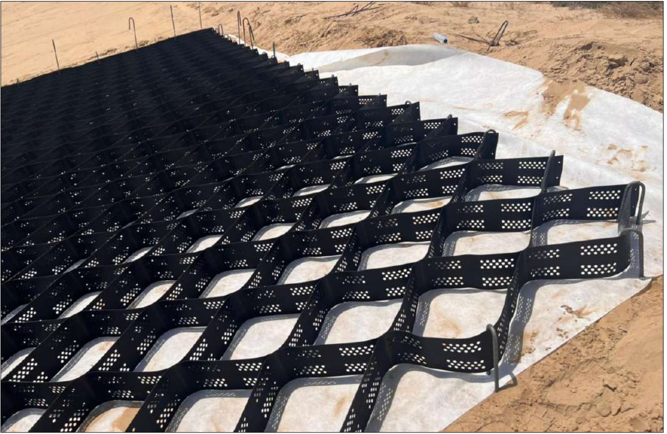
Photo 2 : During Construction Photograph
