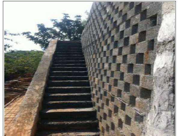
Fig 2 : Stairs over reinforcement
