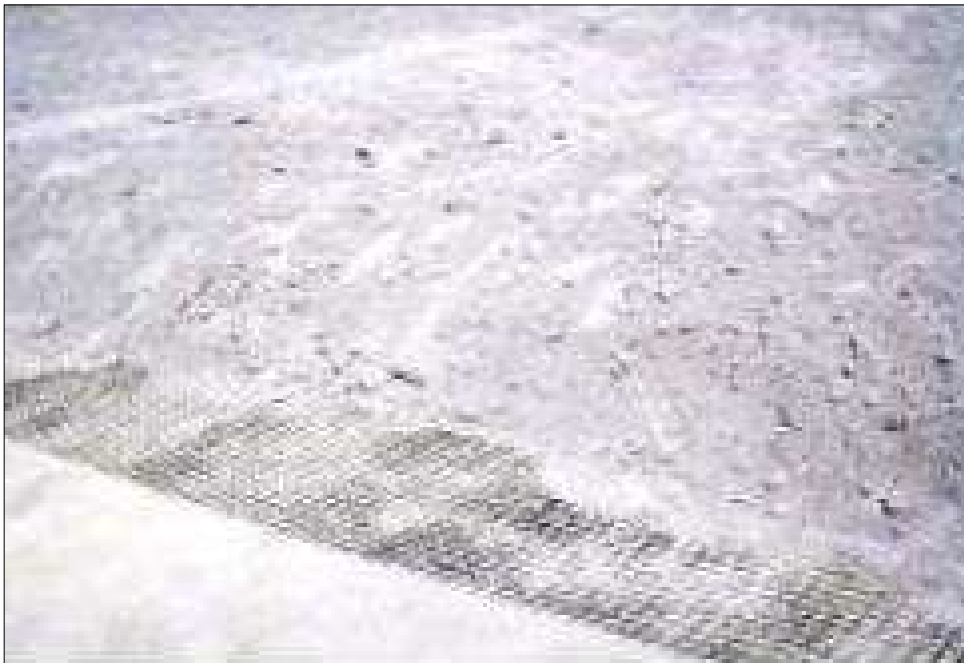
Laying down fill over TechGrid TGU-40 for Embankment
