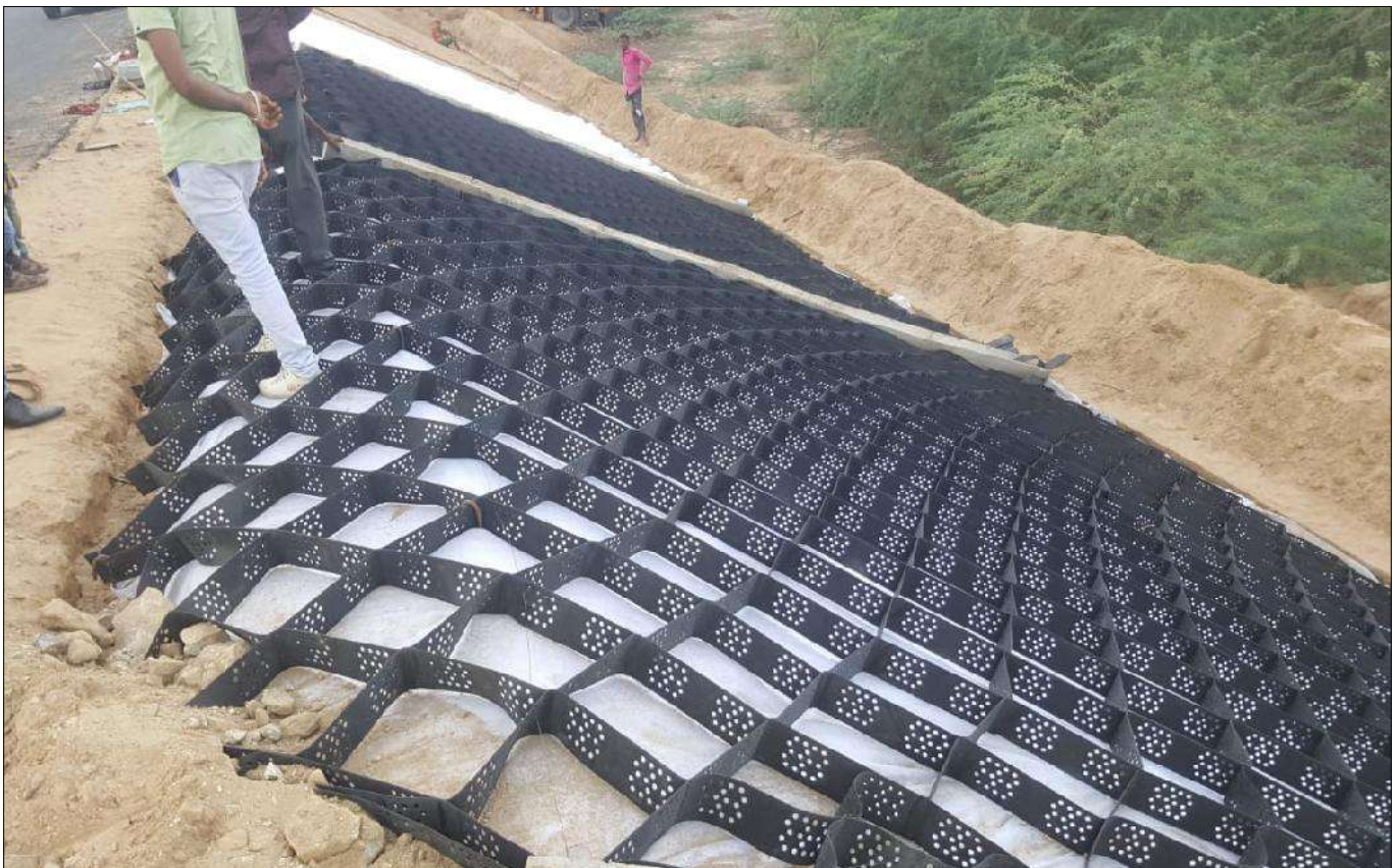
Installation of Geocell
