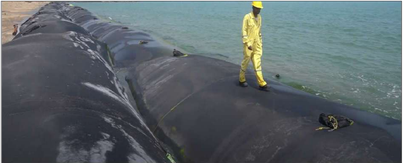
After complete laying Geotextile Tube in base layer and in middle layer (3+2 )
