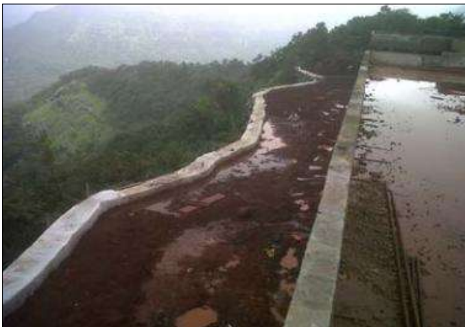
Techfab Metal Gabion Wall – Top View
