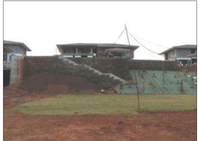
RSW with Weld Mesh - Staircase Completed
