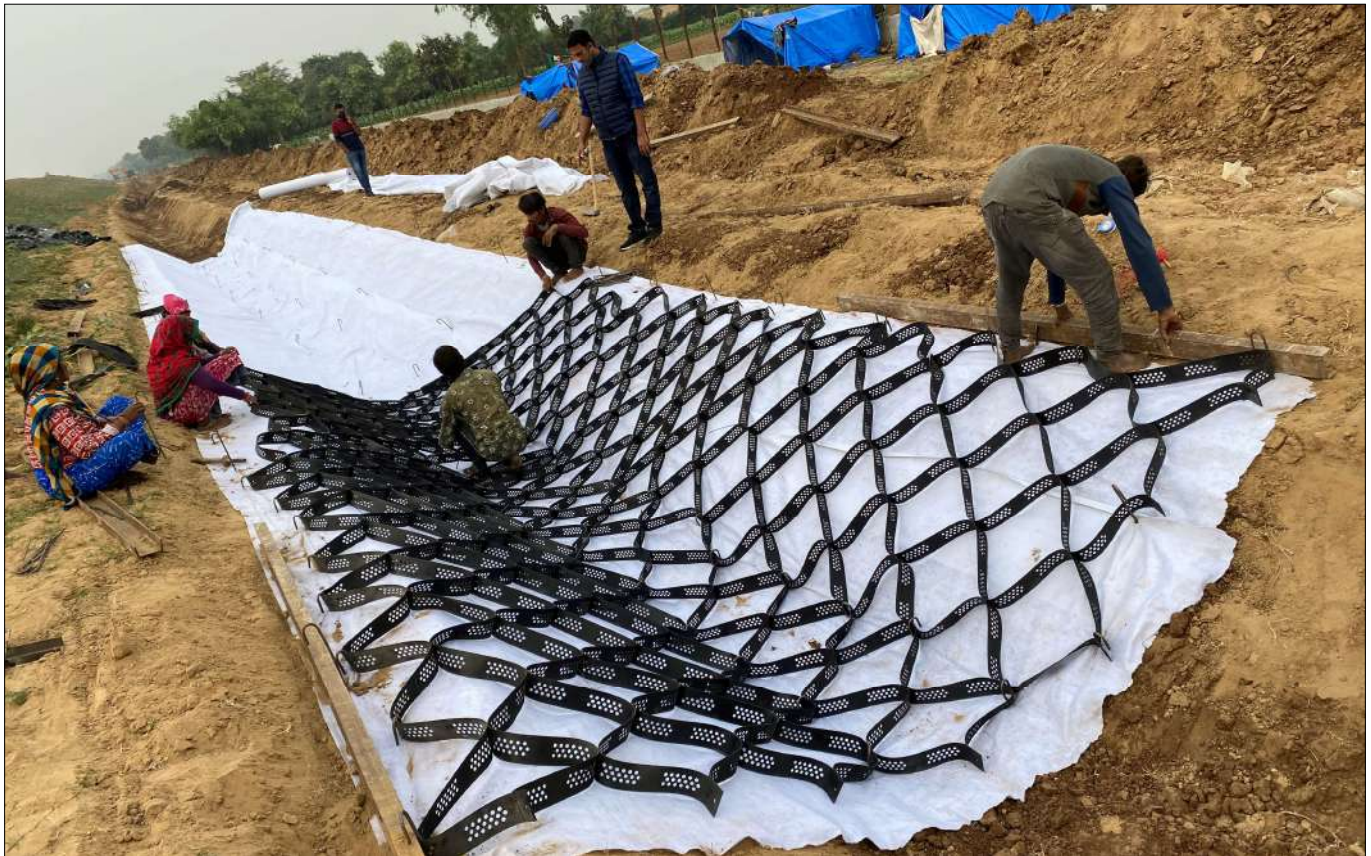
Photo 4 : Construction of Drains lined with concrete filled Geocells
