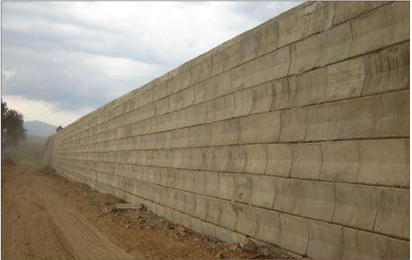
Photo 3 : Elevation view of RS wall
