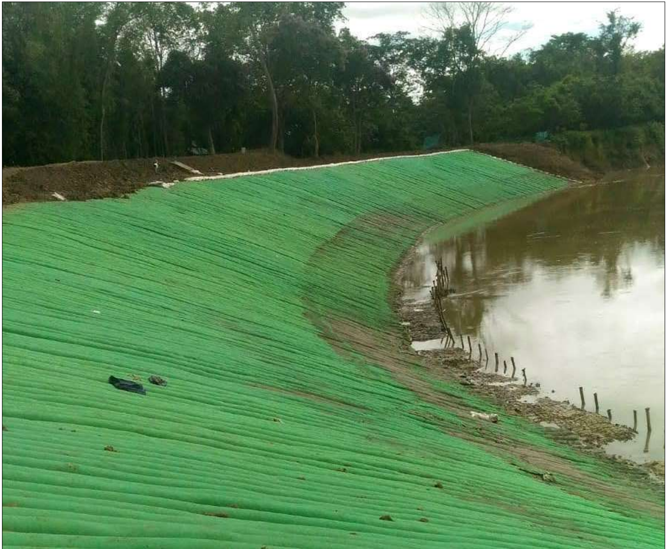
Photo 3 : After Completion Photograph
