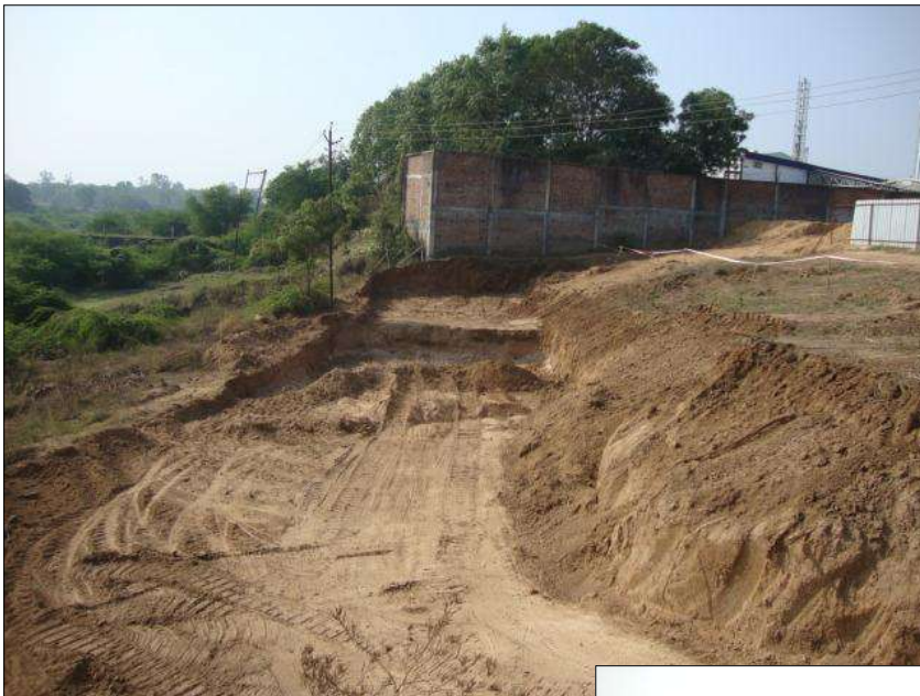
Preparing site with proper surface
