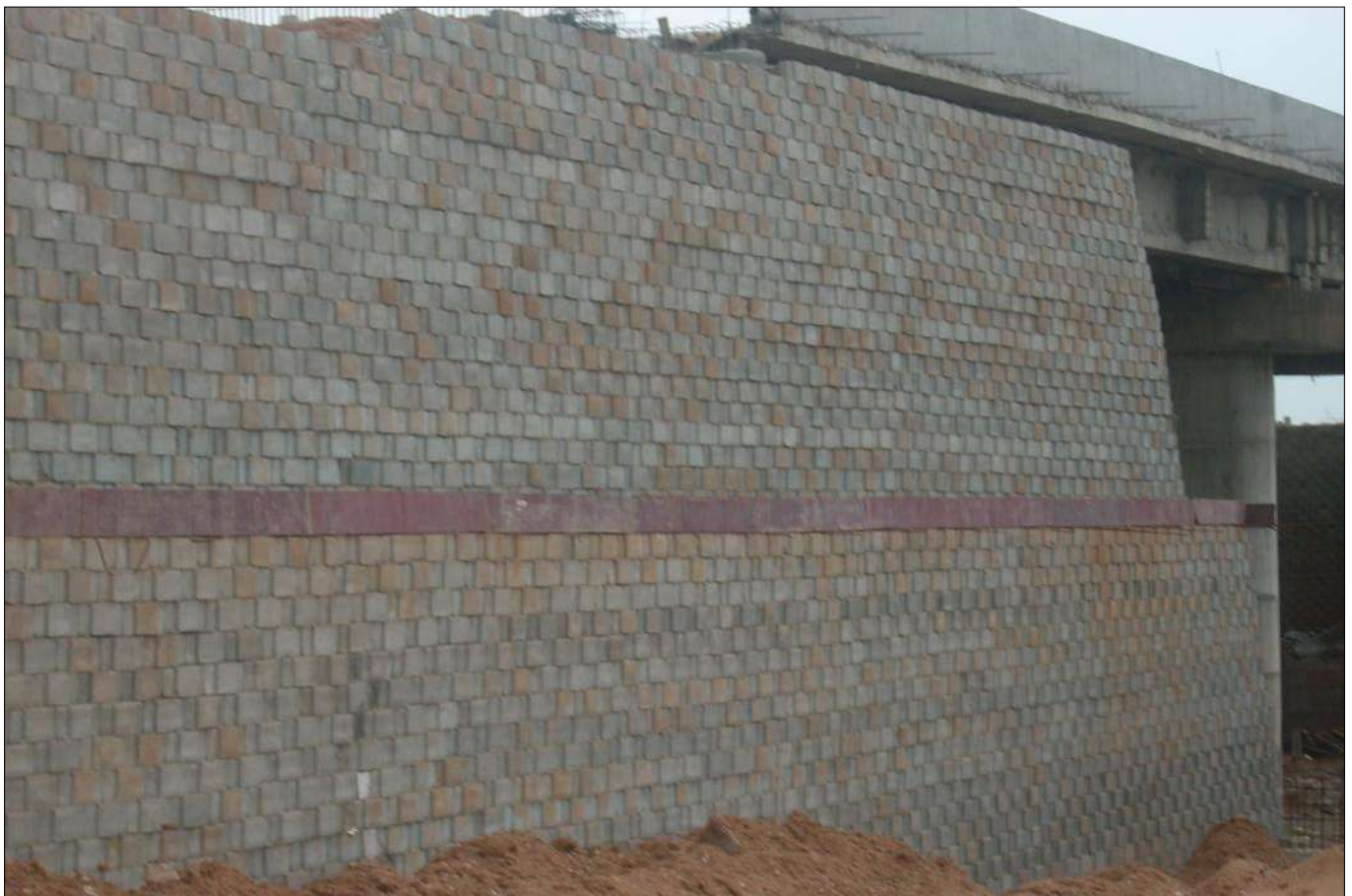
Photo 1 : Elevation view of Two Tier RS wall
