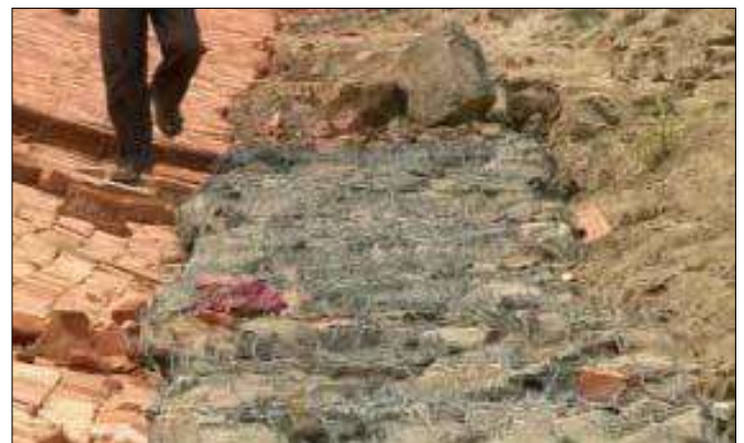
Metal Gabion Placed at Bottom Trench
