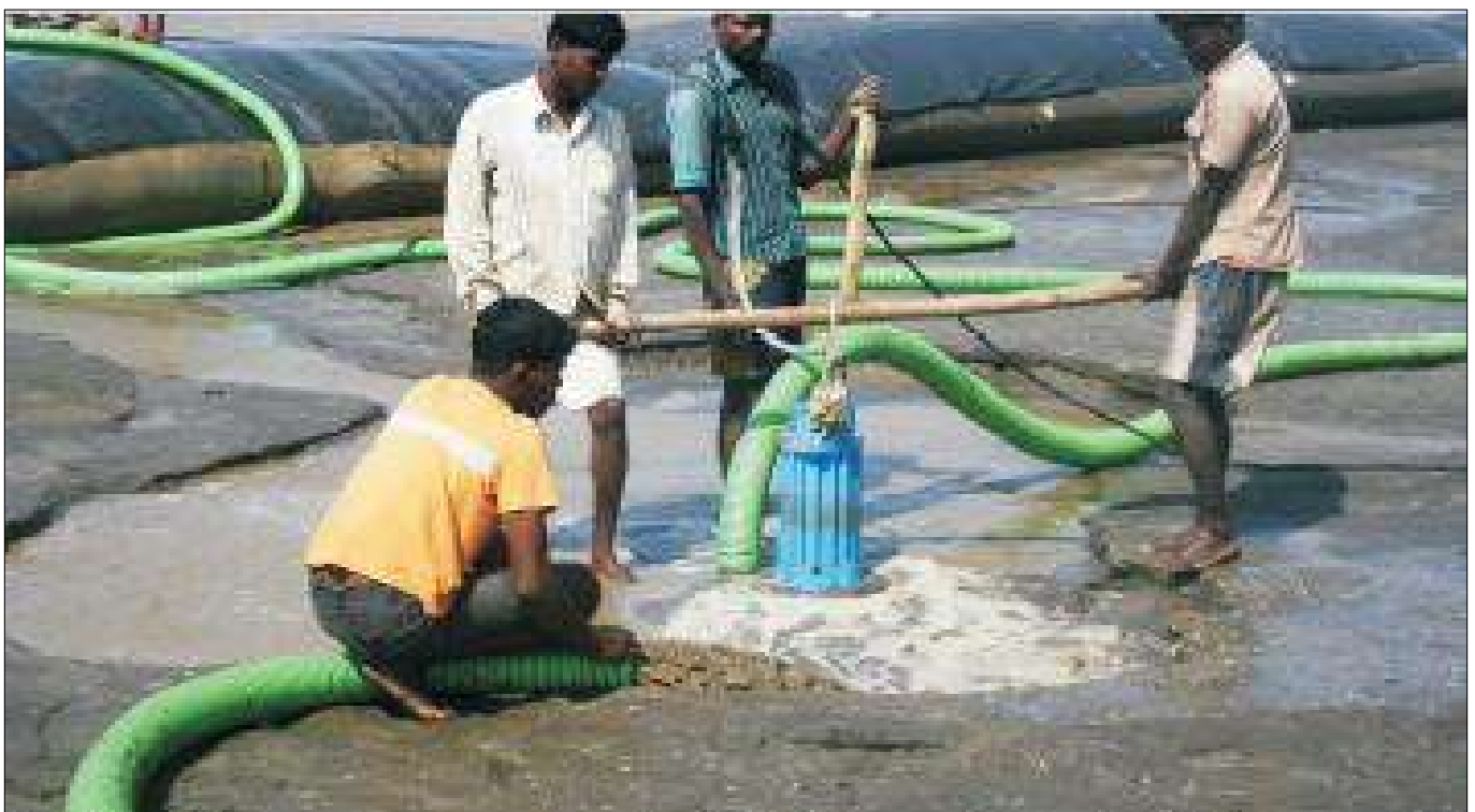
During Installation of TechTube
