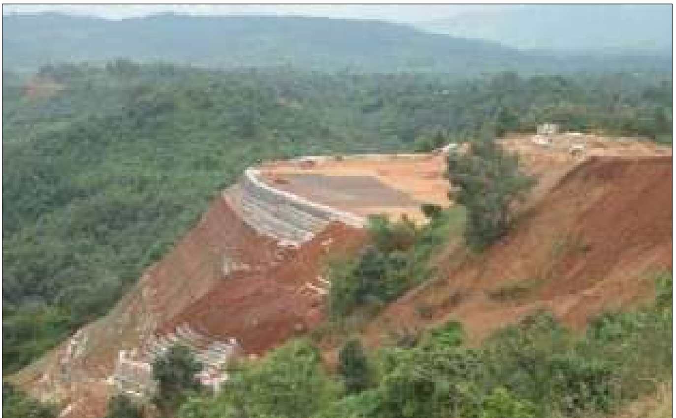
Pre Final Stage of Construction
