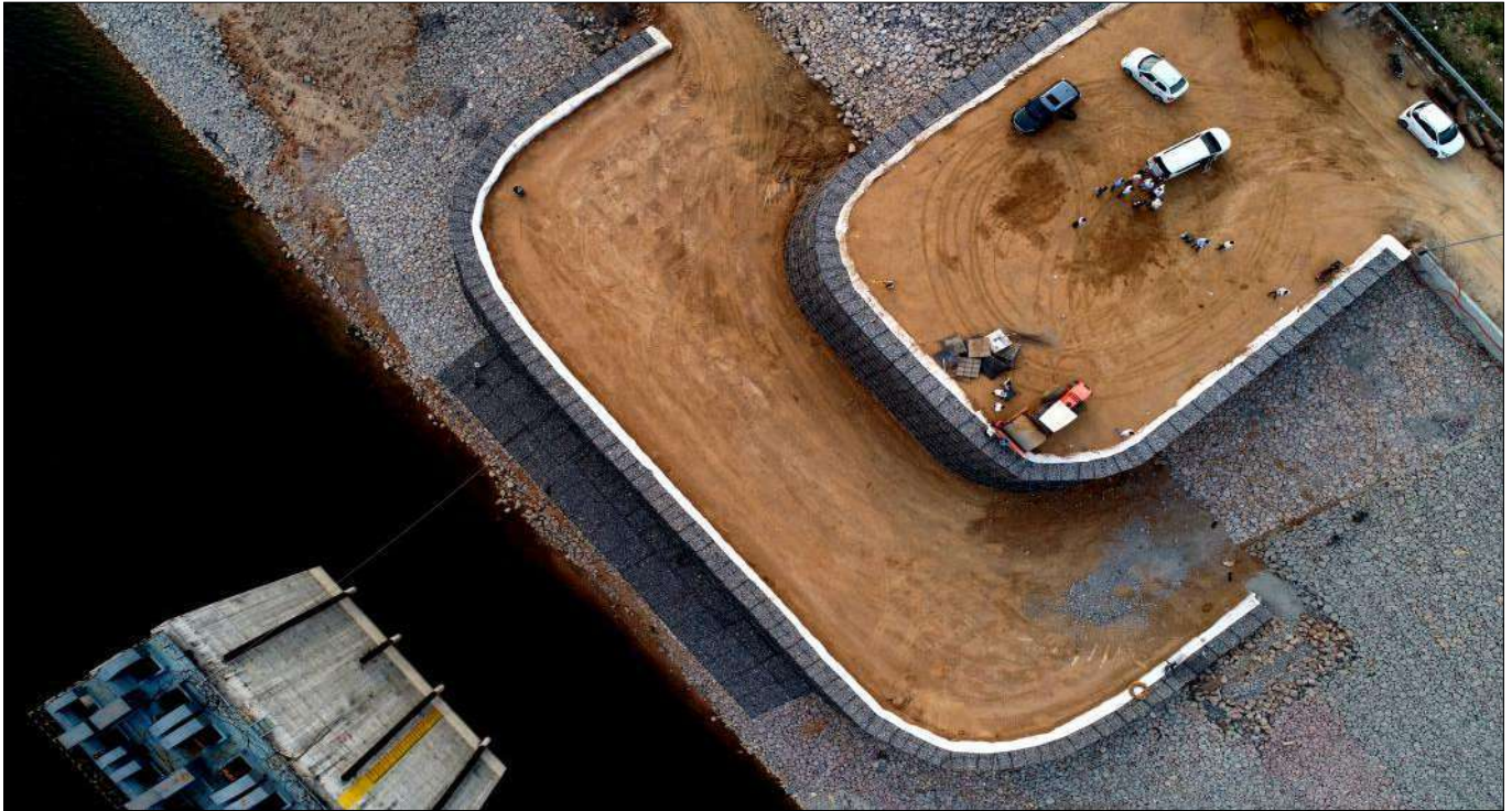
Photo 6 : Top view of the Structure
