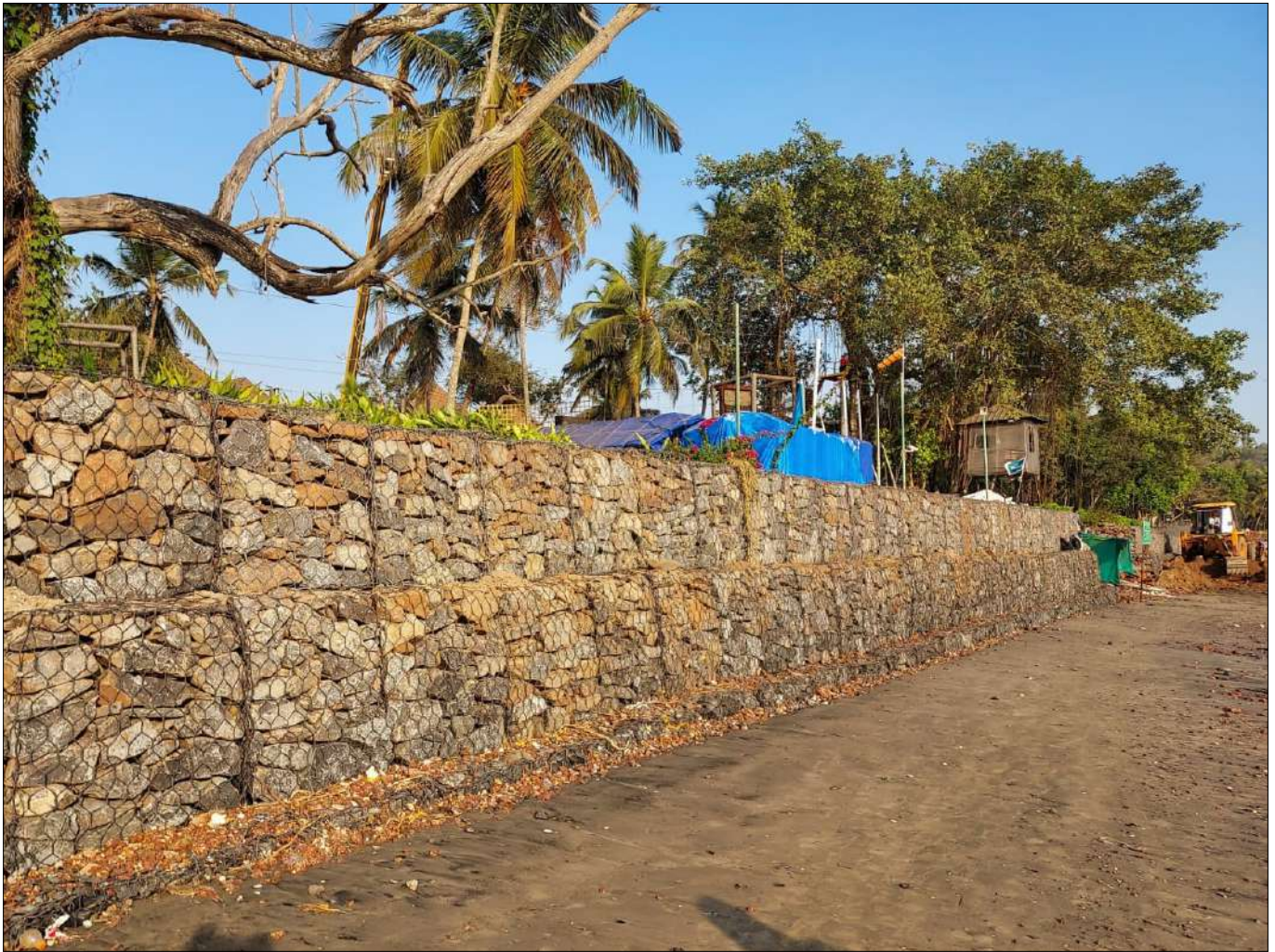
Completed Structure of Gabion Wall
