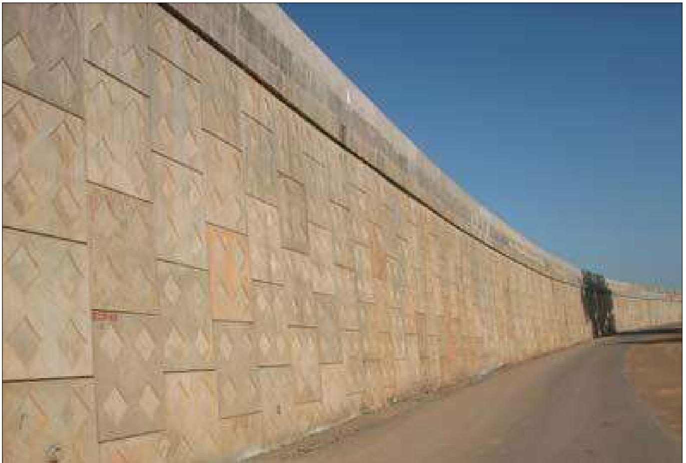
Elevation view of RS wall
