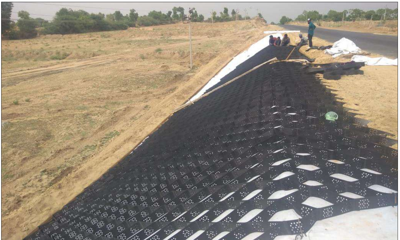
Installation of Geocell
