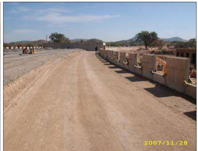
Photo 2 & 3: Erection of RS wall
