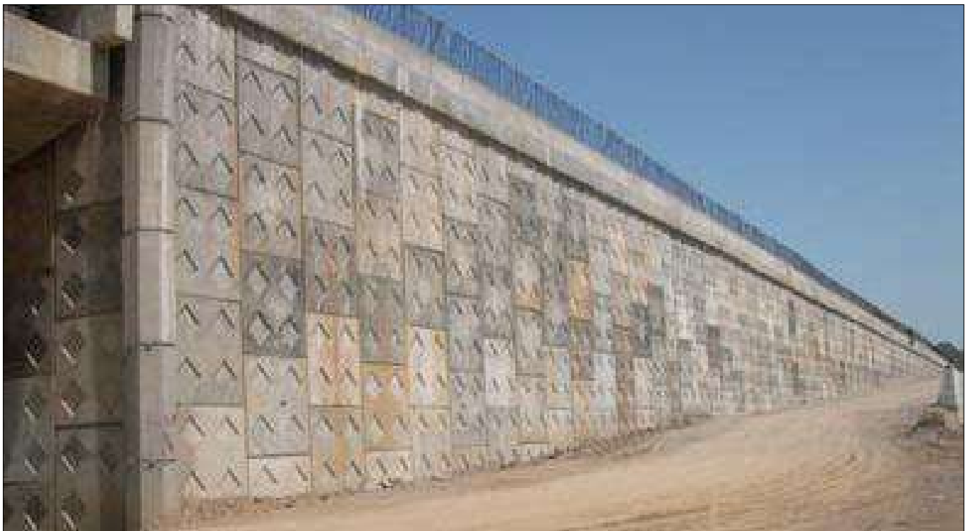
Photo 1 : Elevation view of RS Wall
