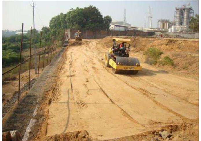
Compaction behind the wall
