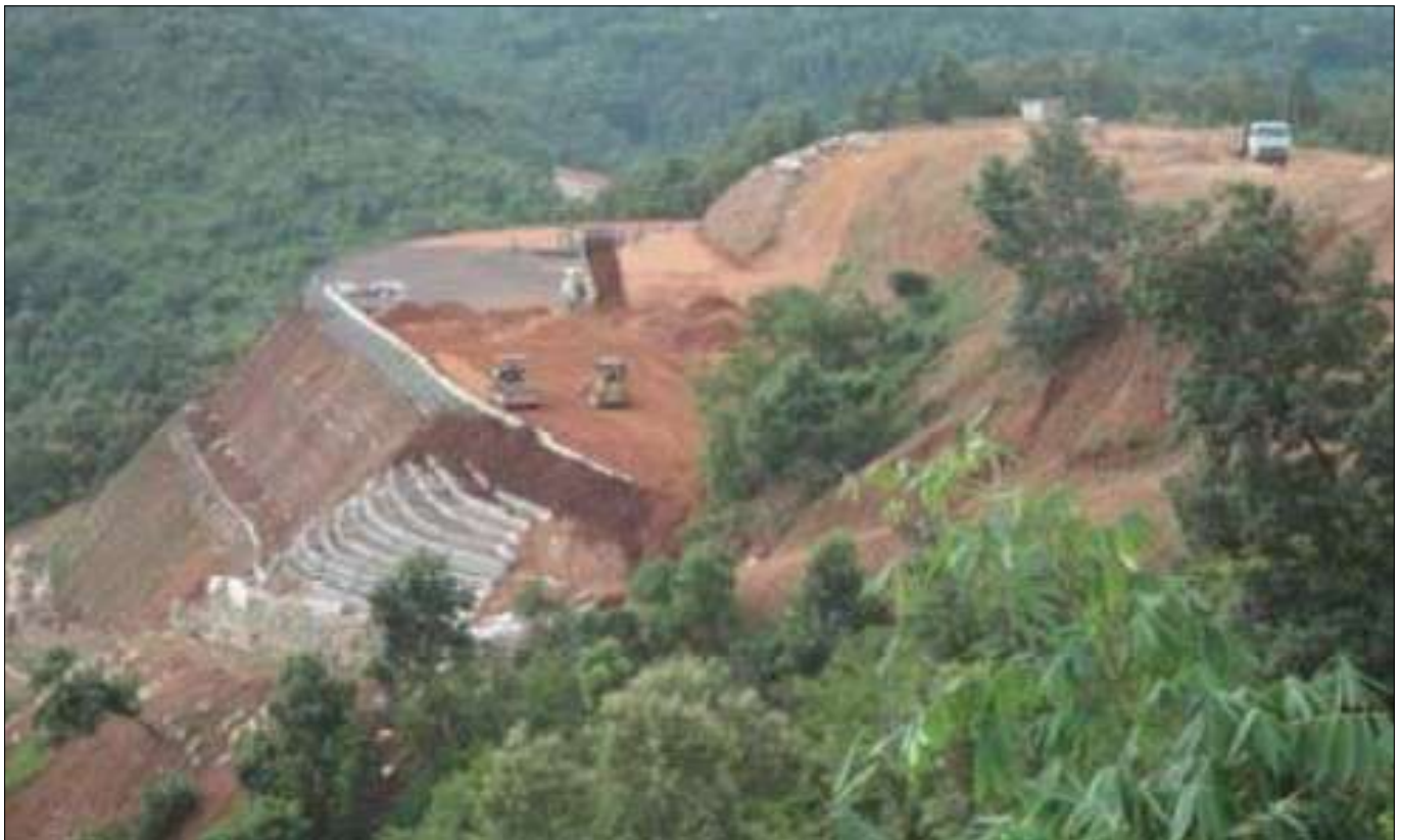
Reinforced Soil Slope – Top View
