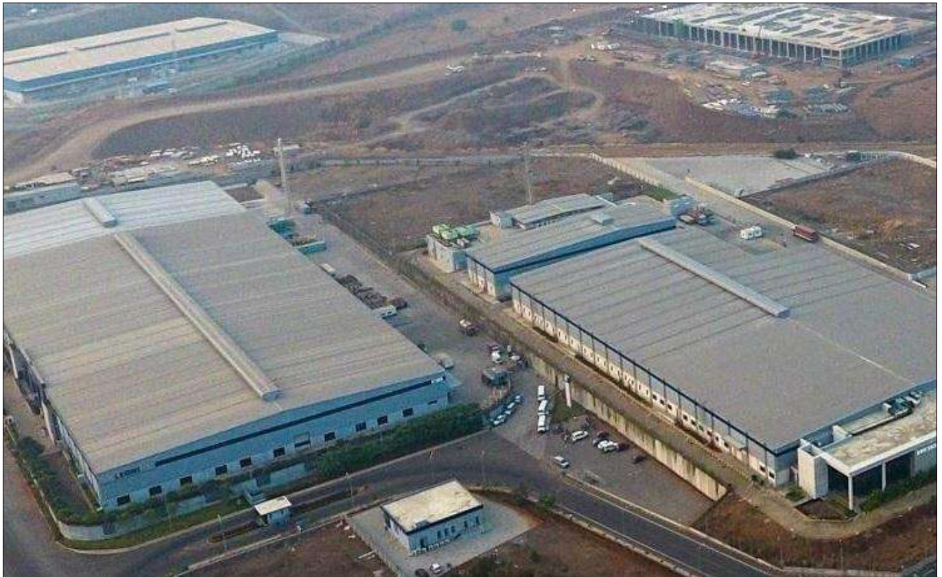
View of ESR industrial park
