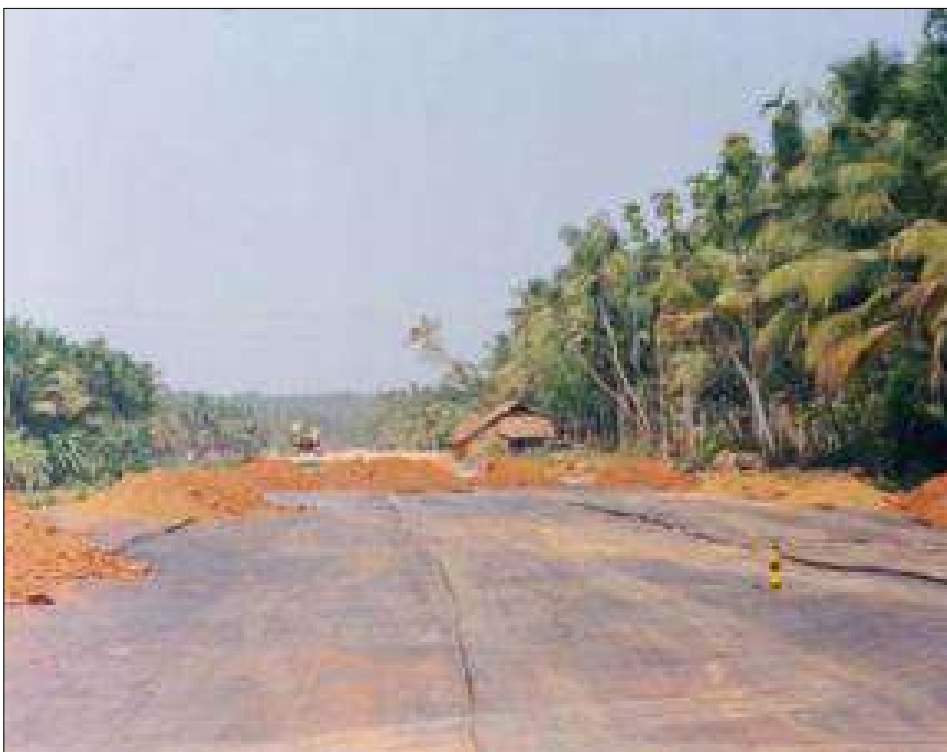
Installation of Techfab TPP 250 Woven Geotextile
