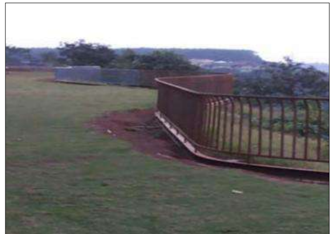
Techfab Metal Gabion Wall - Completed
