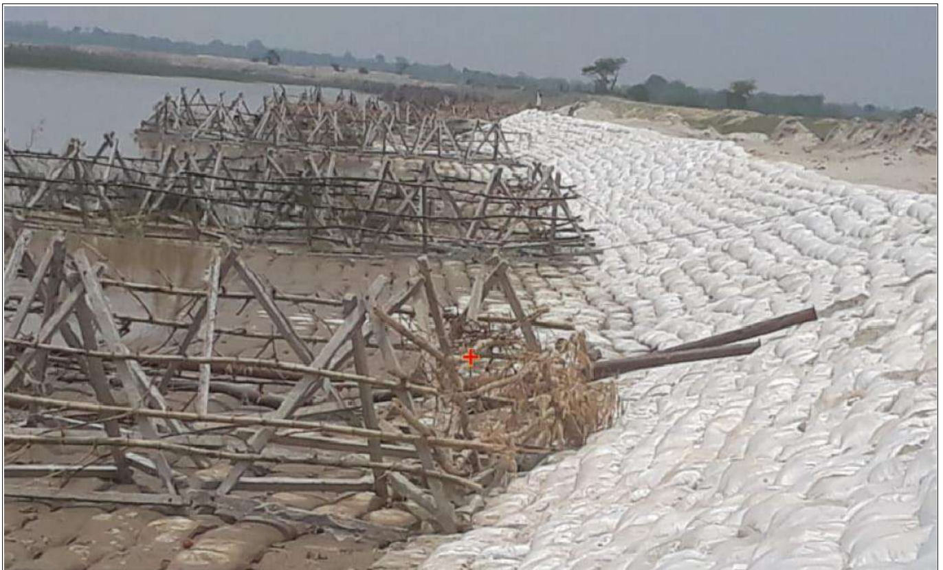
Photo 3: Porcupine concrete spurs
