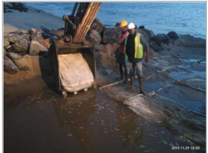
Laying of Geotextile bags in progress
