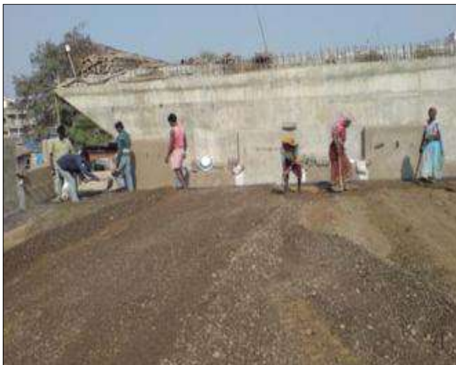
Erection of RS Wall
