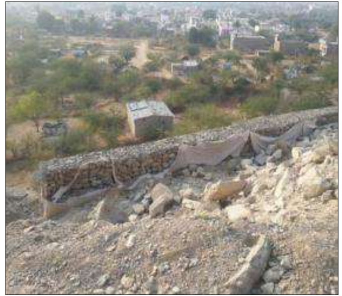
TechFab Metal Gabion – Top View
