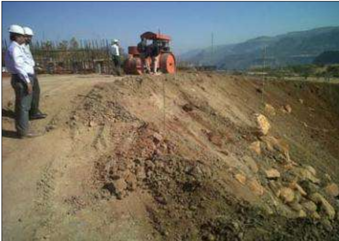
RSW with Weld Mesh - Under Construction
