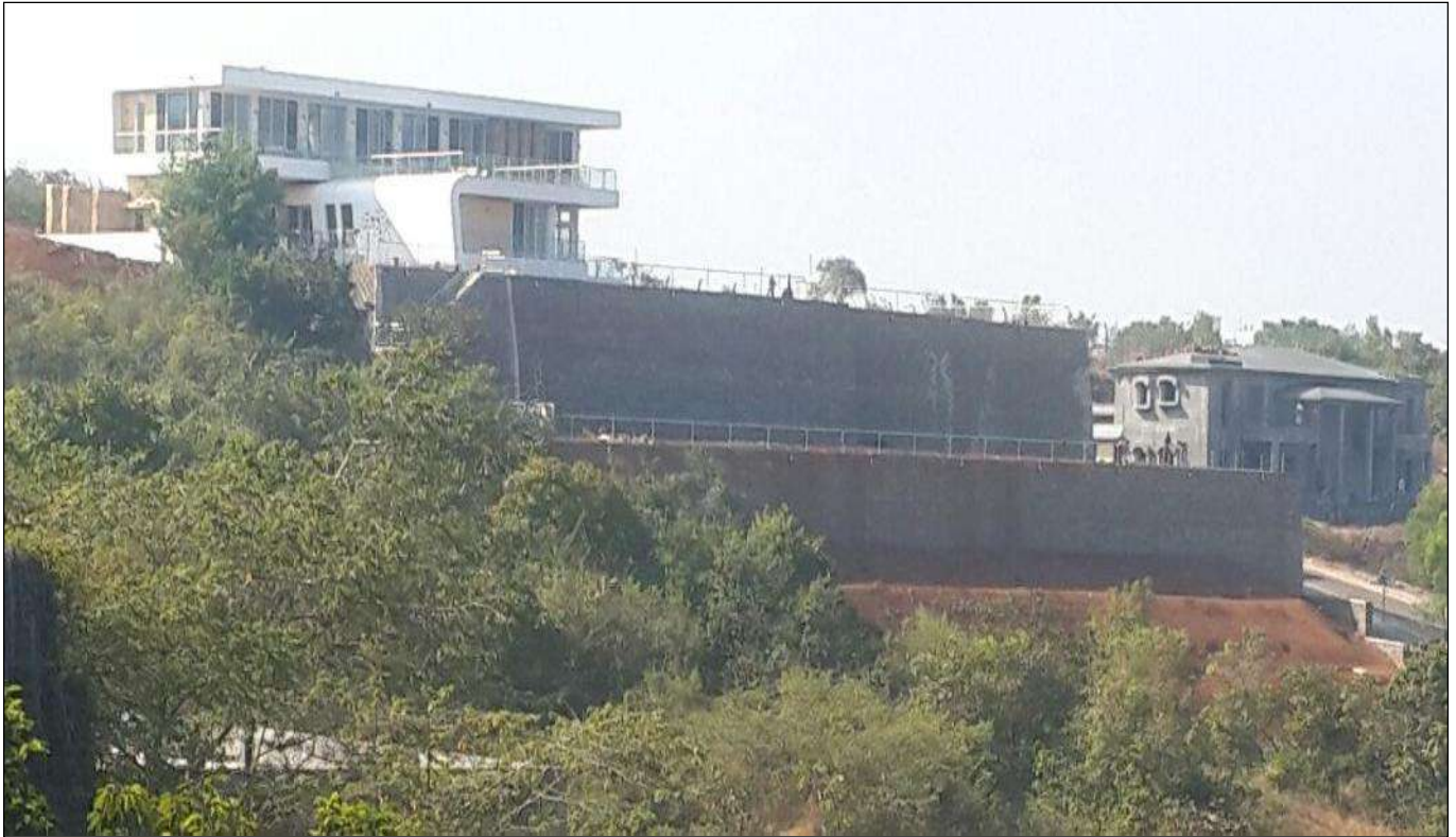
Fig 6 : Structure after Construction
