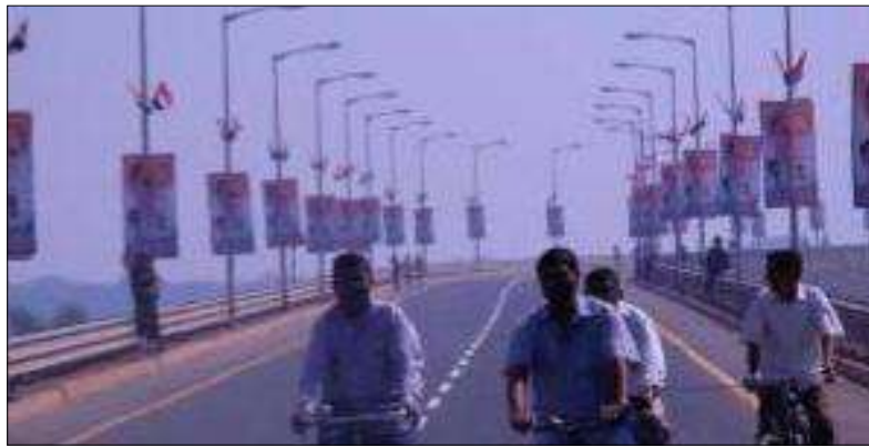
Rajiv Gandhi Setu Bridge completed & open for Traffic
