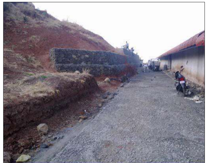
TechFab Metal Gabion - Installation
