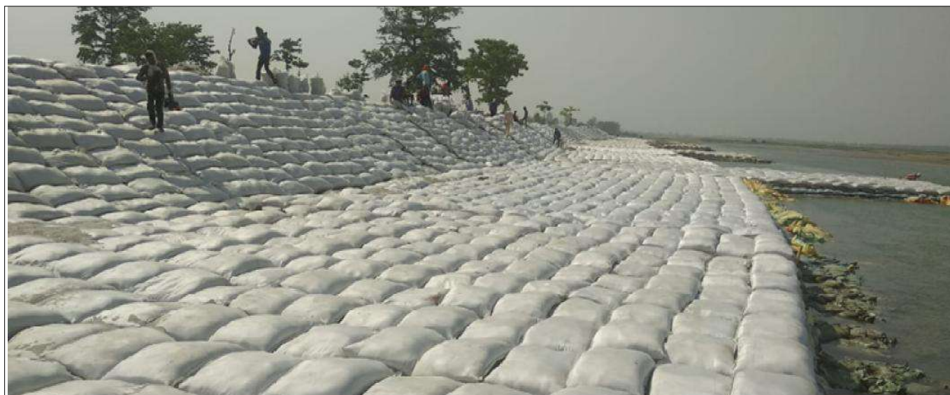
Photo 4: The Flood protection work / dikes using geotextile bags
