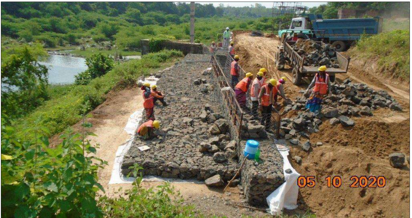
Work under Construction - Gabion Facia & Mattress Installation
