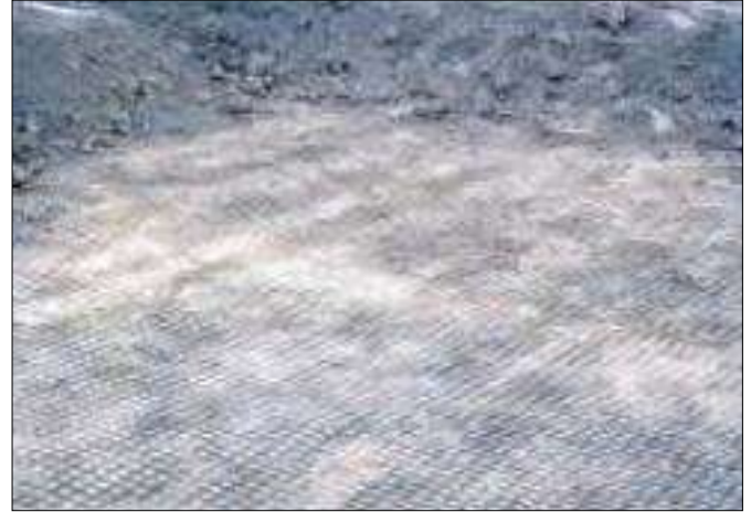
Laying down fill over TechGrid TGU-40 for Embankment
