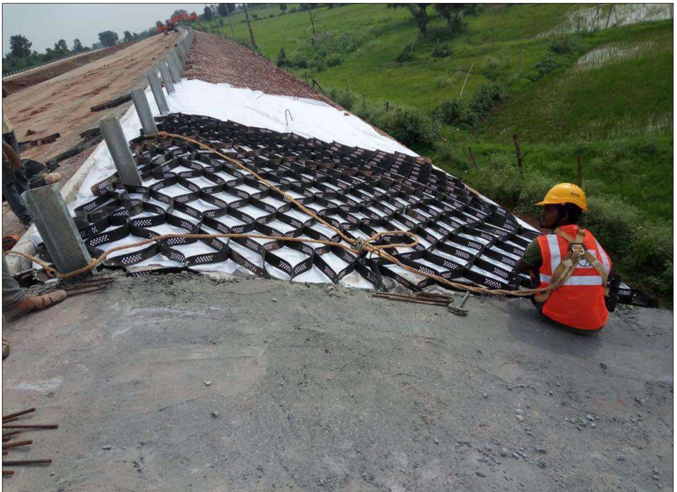
Progress of Concrete filling in Geocell
