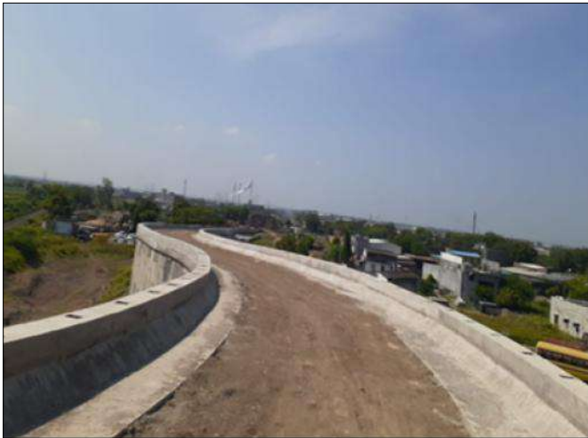
Coping beam installation completed
