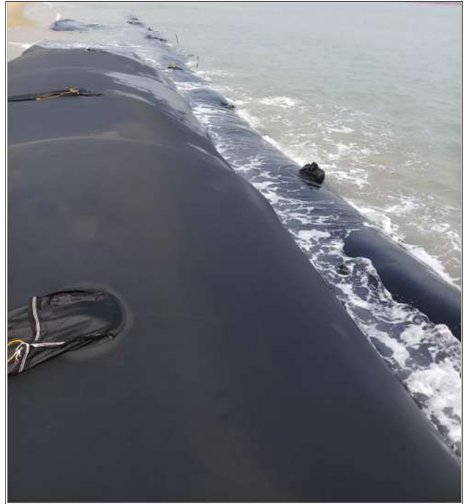
Filled first layer of Geotextile Tube
