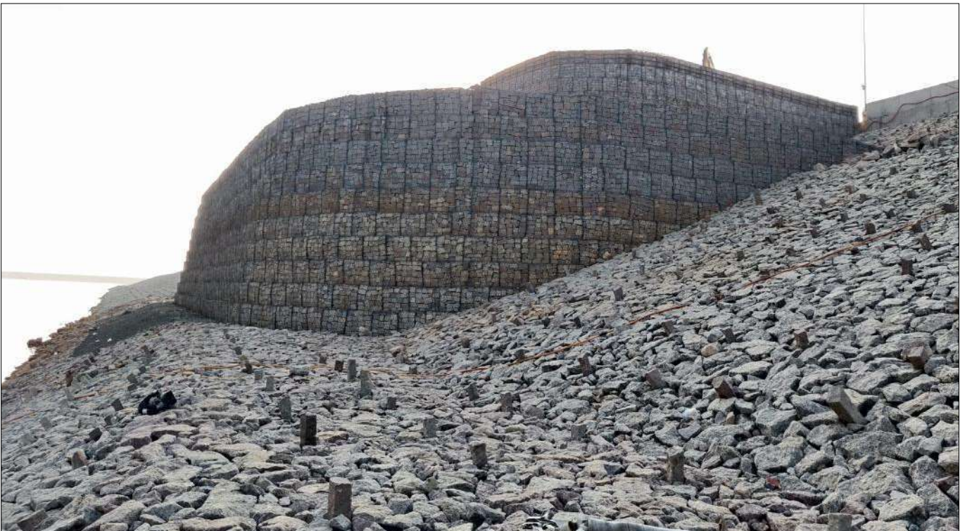
Photo 5 : Installation of Gabion fascia units on Top wall
