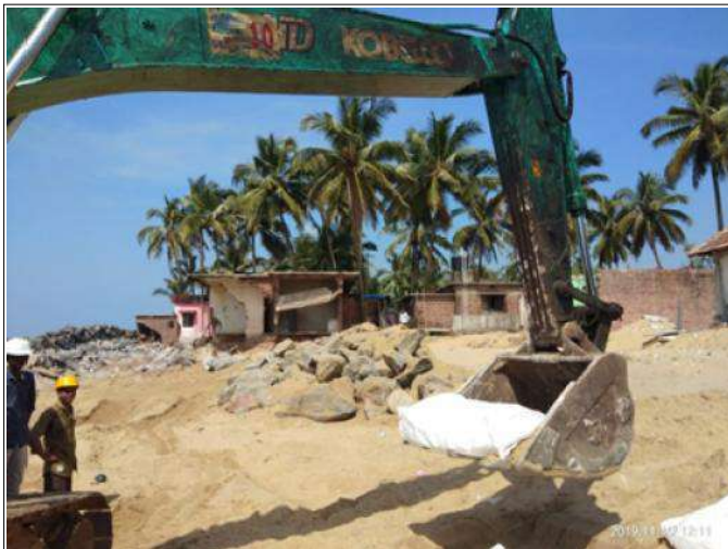
Dumping of Geotextile bags in progress
