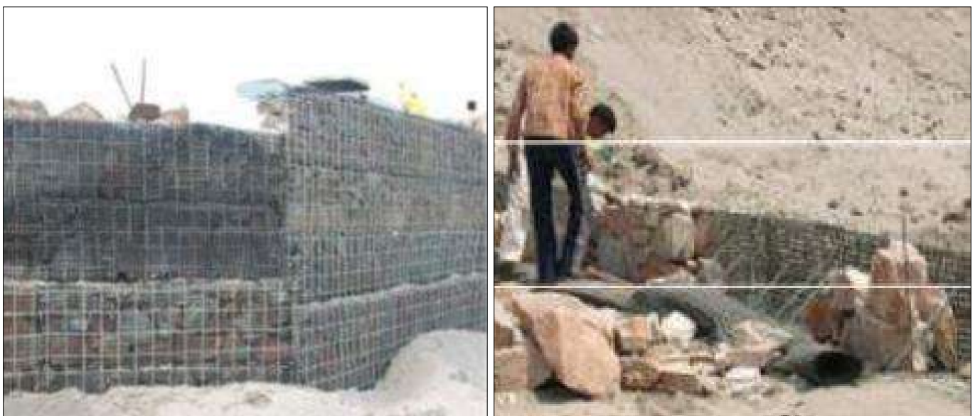
During Construction Photographs
