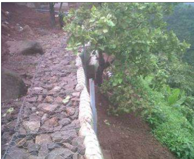
Techfab Metal Gabion Wall - Valley Portion
