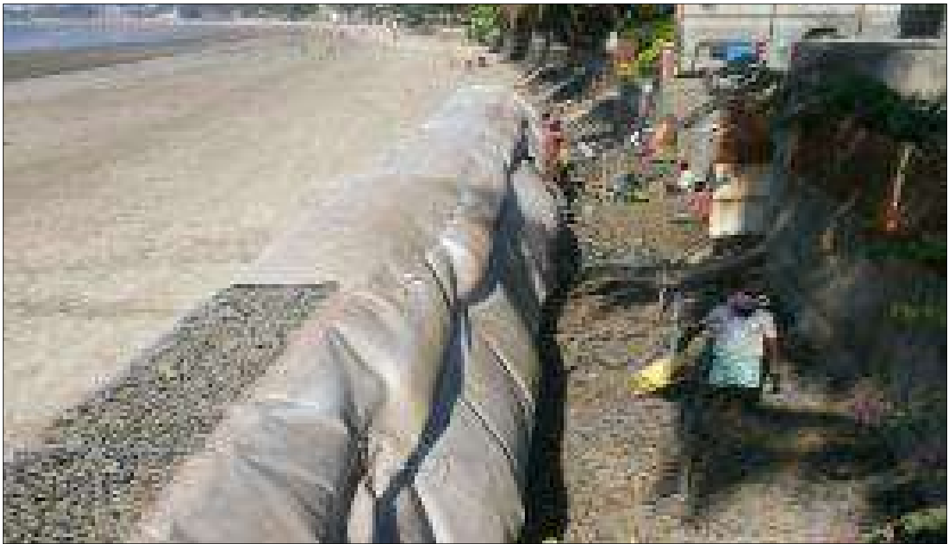
Photo 2 : TechFab Metal Gabion Installation
