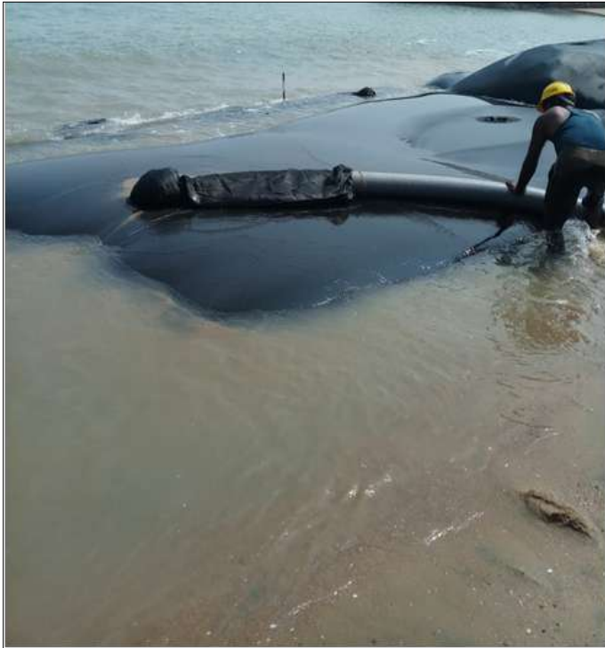
Geotextile Tube filling is in progress
