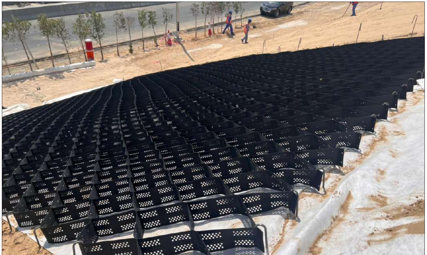
Photo 1 : Installation of Techcell Geocell over the slope
