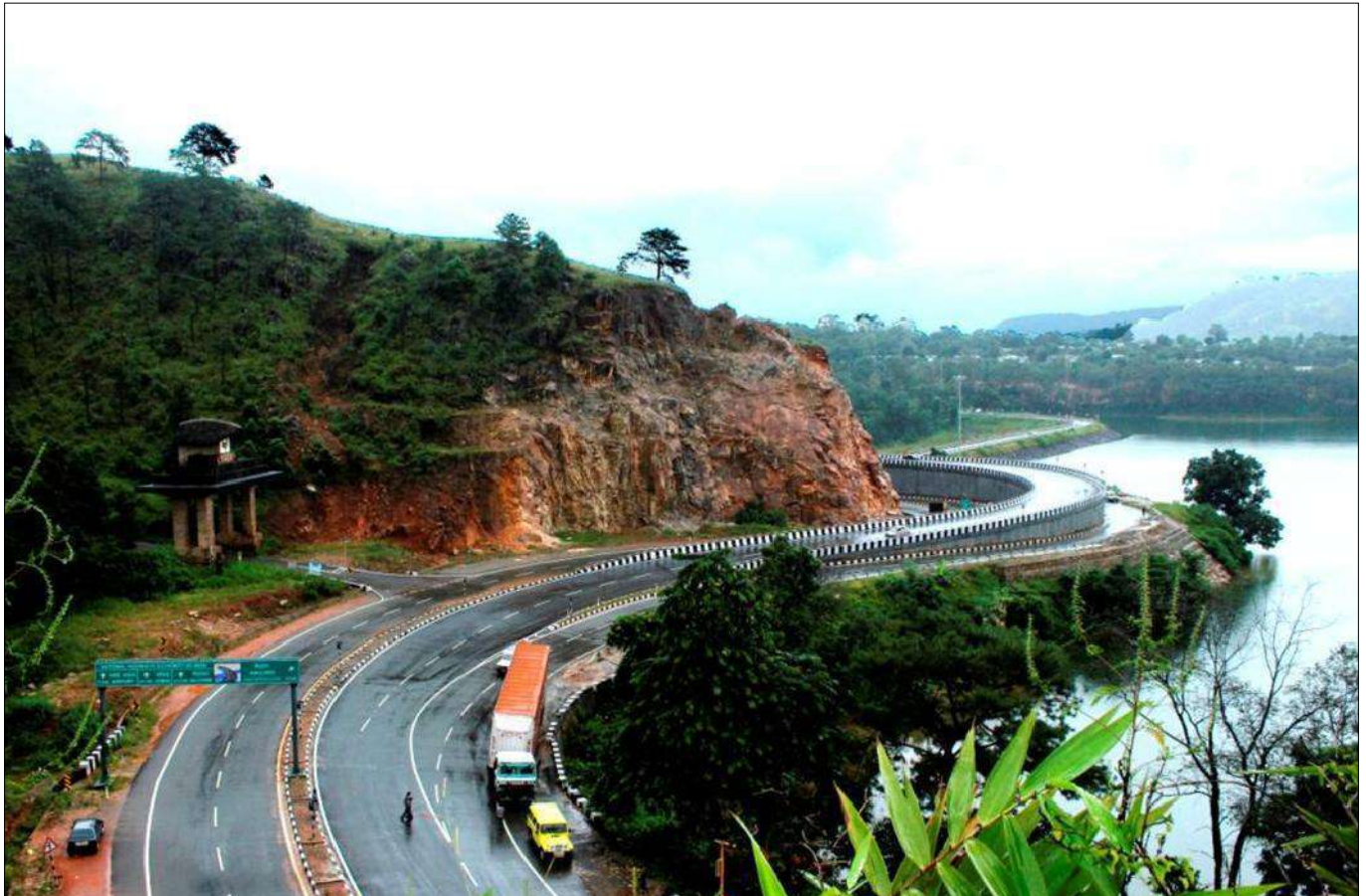
Before implementation of Rockfall Netting
