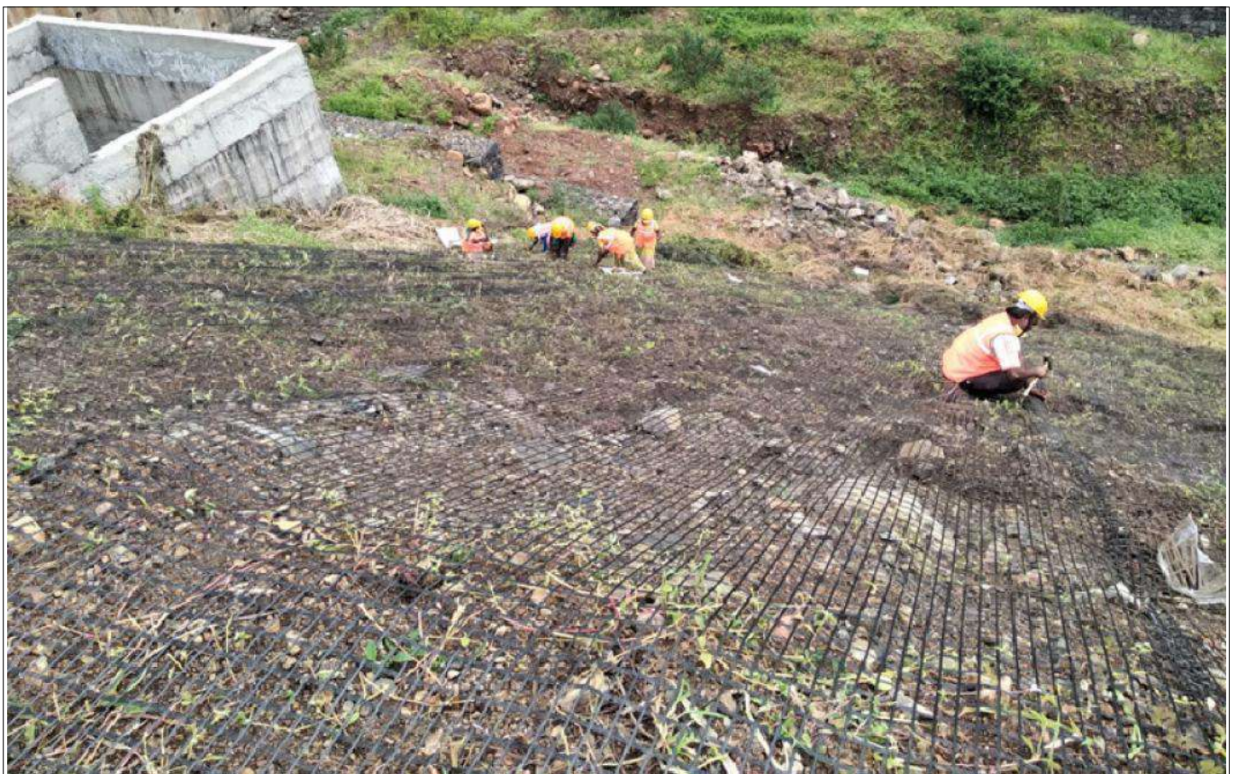
During Construction Photographs
