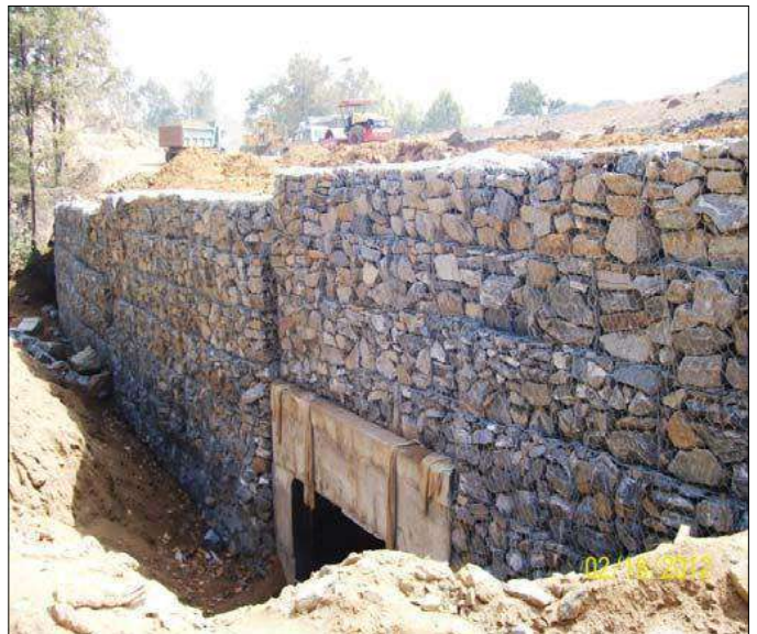
Photo 1 & 2 : TechFab Metal Gabion Installation in progress
