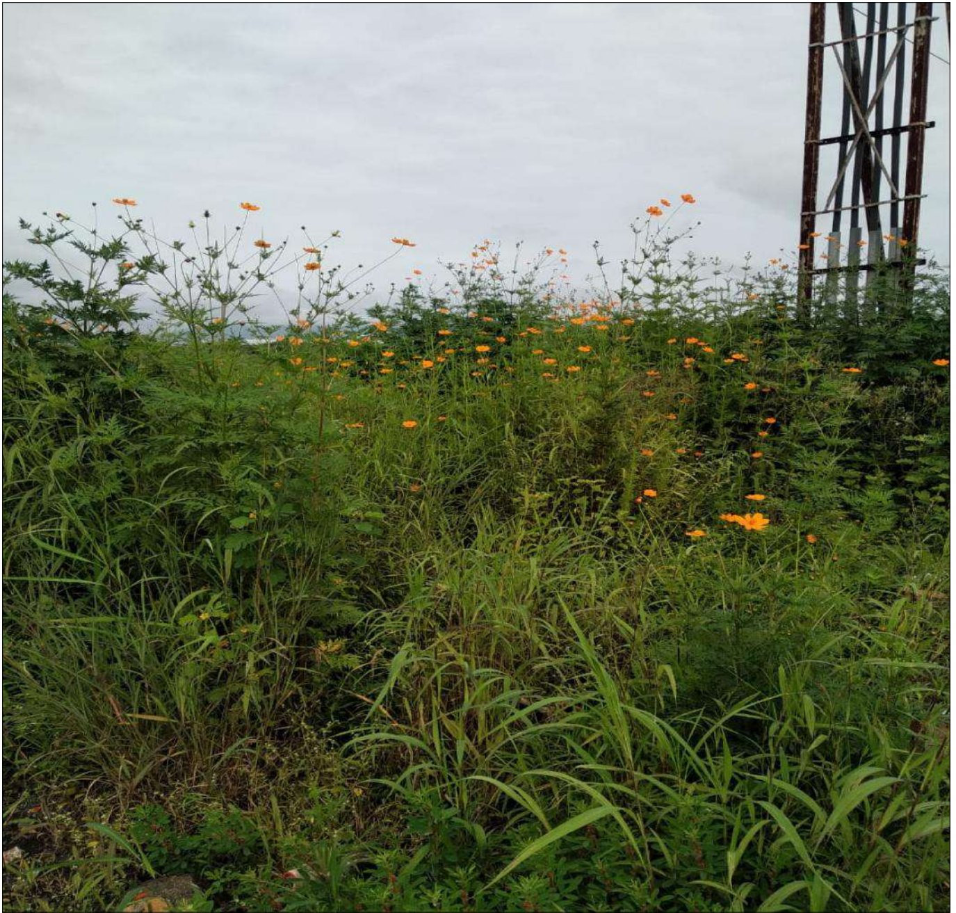
Slope after vegetation has grown
