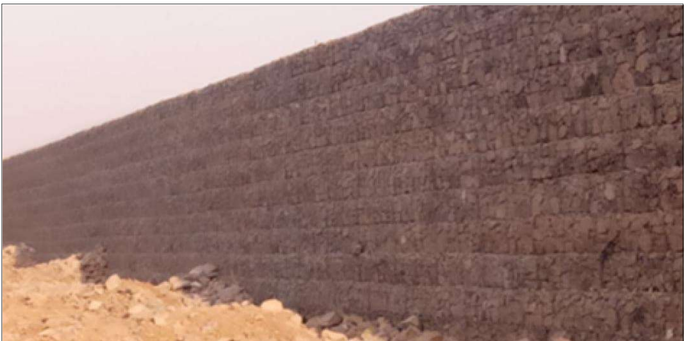
Figure 10 & 11 : Photographs of Completed Reinforced soil wall with Gabion Fascia
