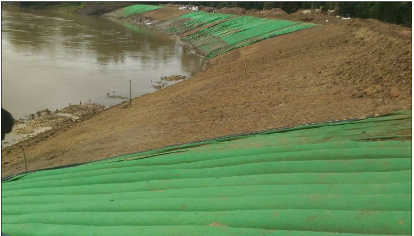
Photo 2 : Laying of Tech GeoMattress on Dressed Slope
