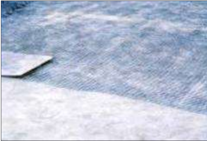
Laying of TechGrid TGU-40 as Basal Reinforcement
