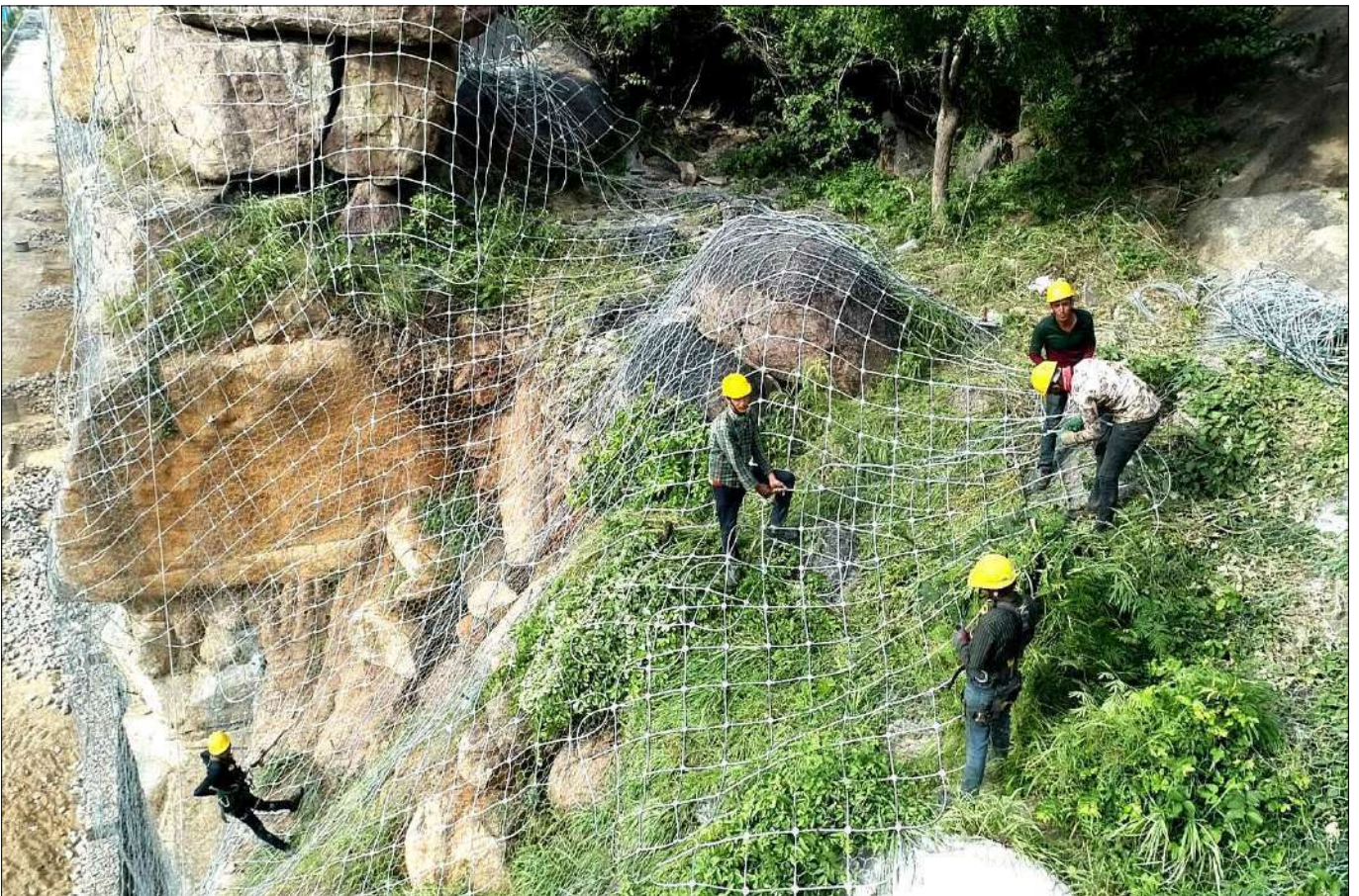
During Construction Photographs (Installation of TechRhombus)
