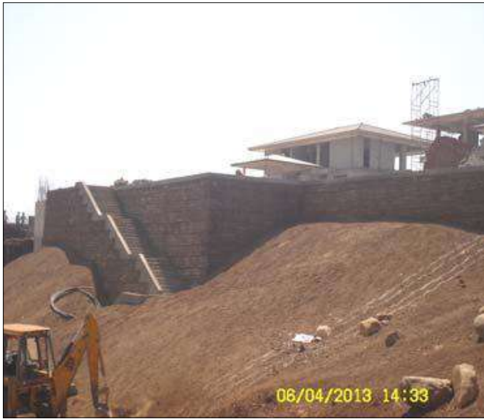
RSW with Weld Mesh - Entrance
