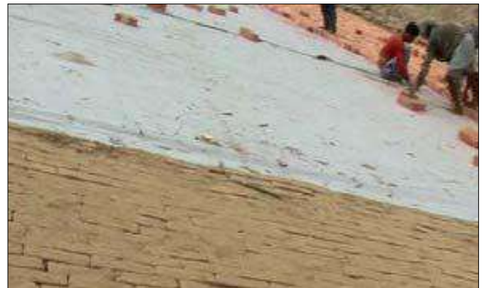
Unrolling of TechGeo Nonwoven Geotextile
