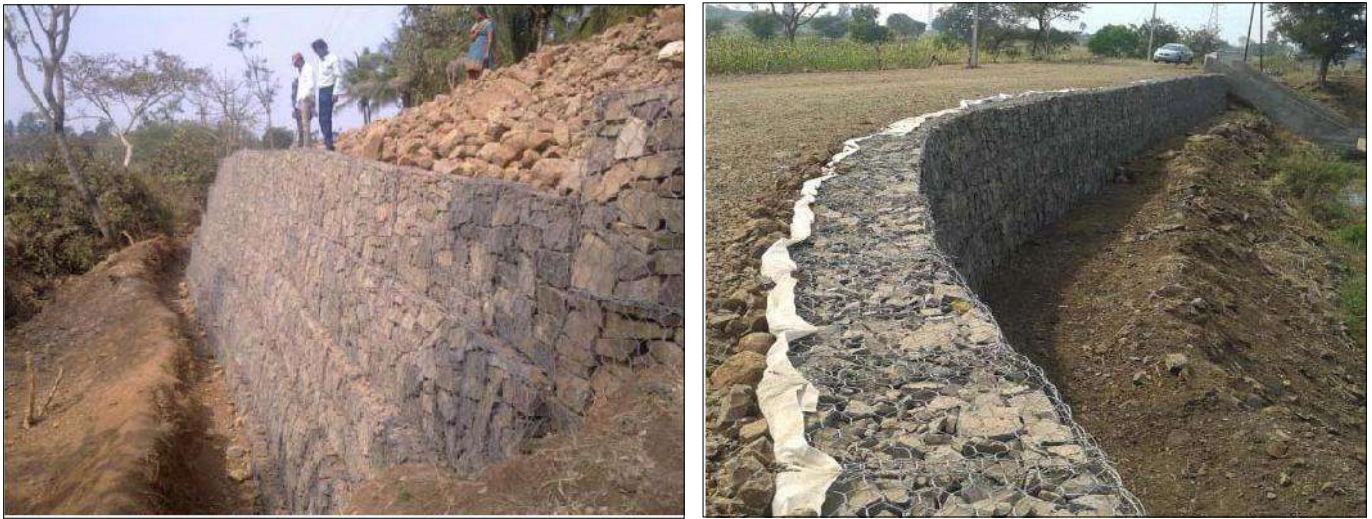
TechFab Metal Gabion Installation Photographs
