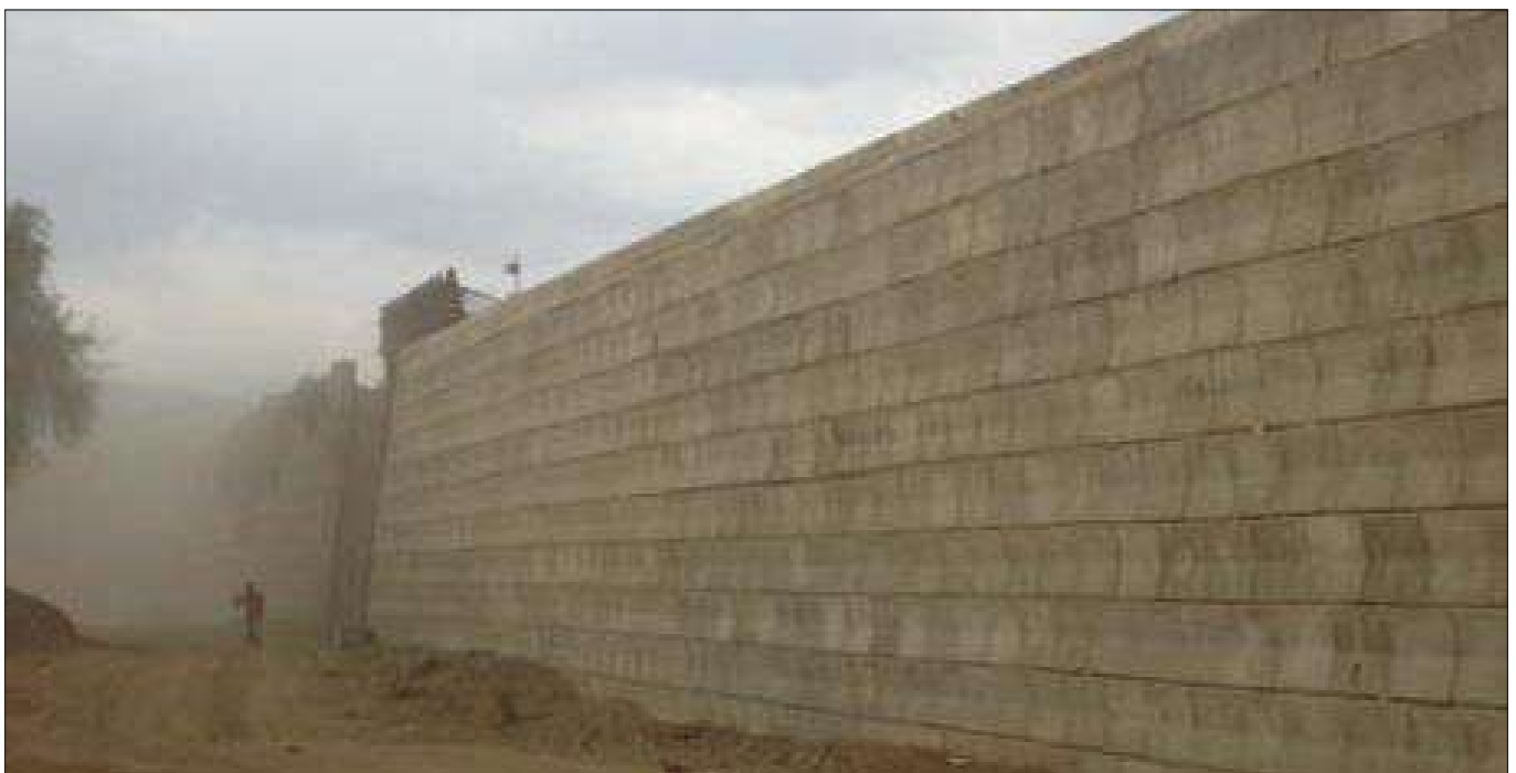
Photo 2 : Elevation view of RS wall
