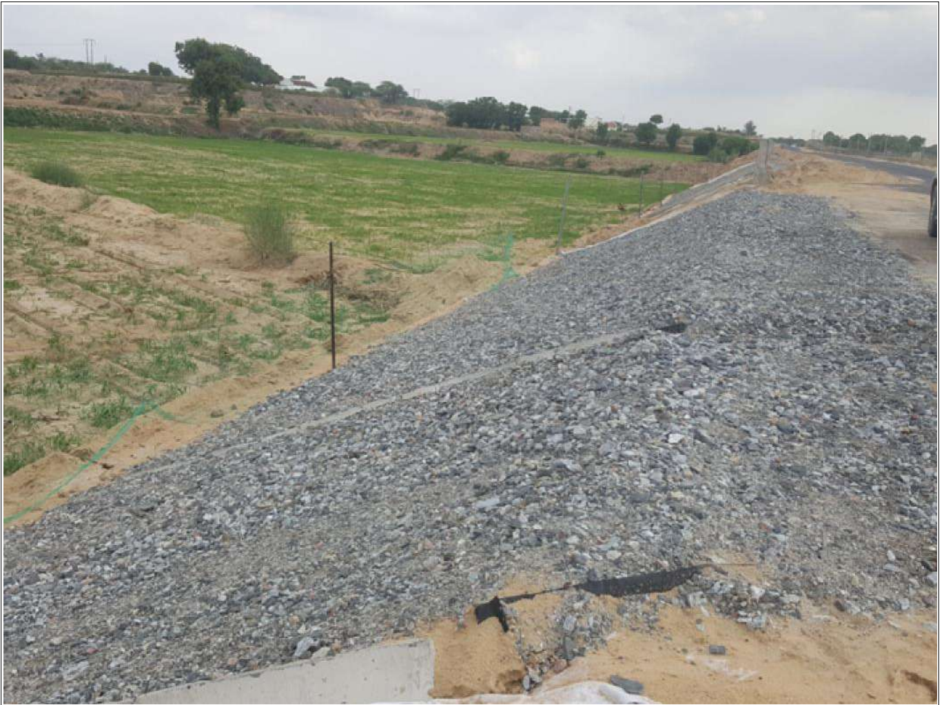
Slope is ready and filled with GSB
