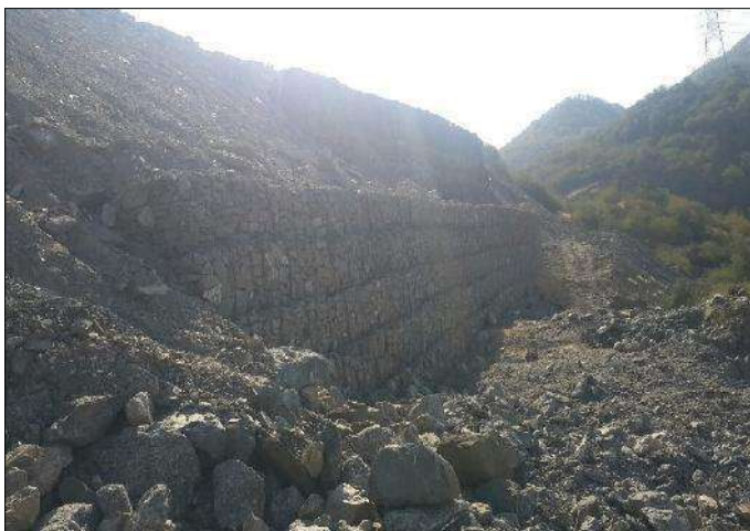
TechFab Metal Gabion - Initial Stage
