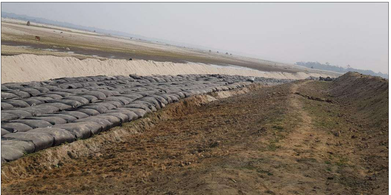
Photo 1 & 2 - Filling & Placement of TechFab Geotextile bags
