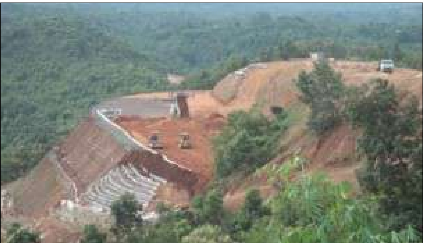
RSS with TechGrid GeoGrid – Under Construction
