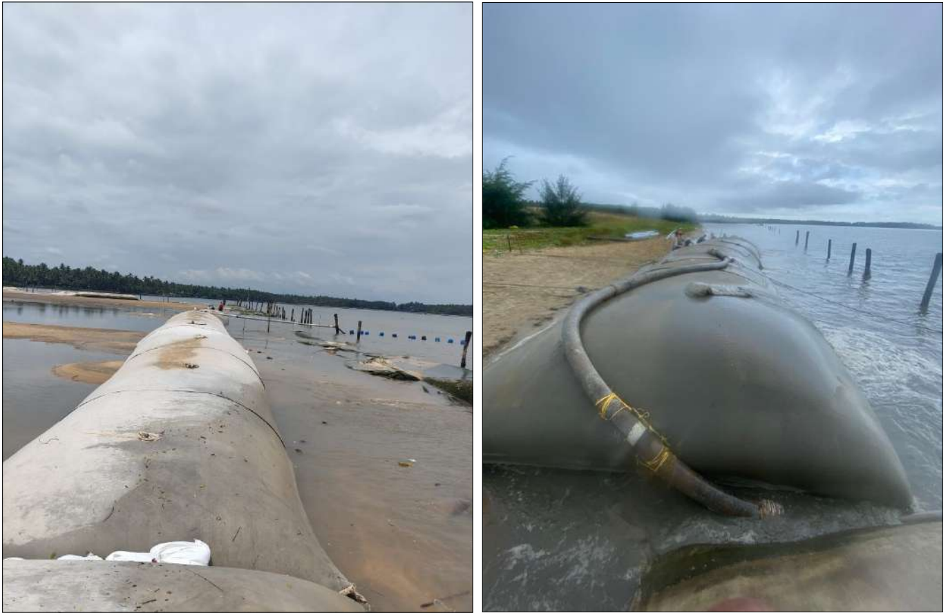
After Construction photographs
