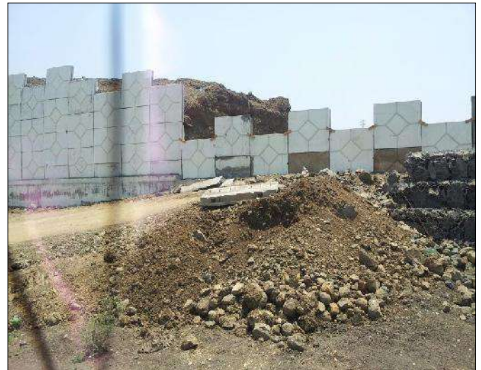
TechFab Reinforced soil wall - Installation
