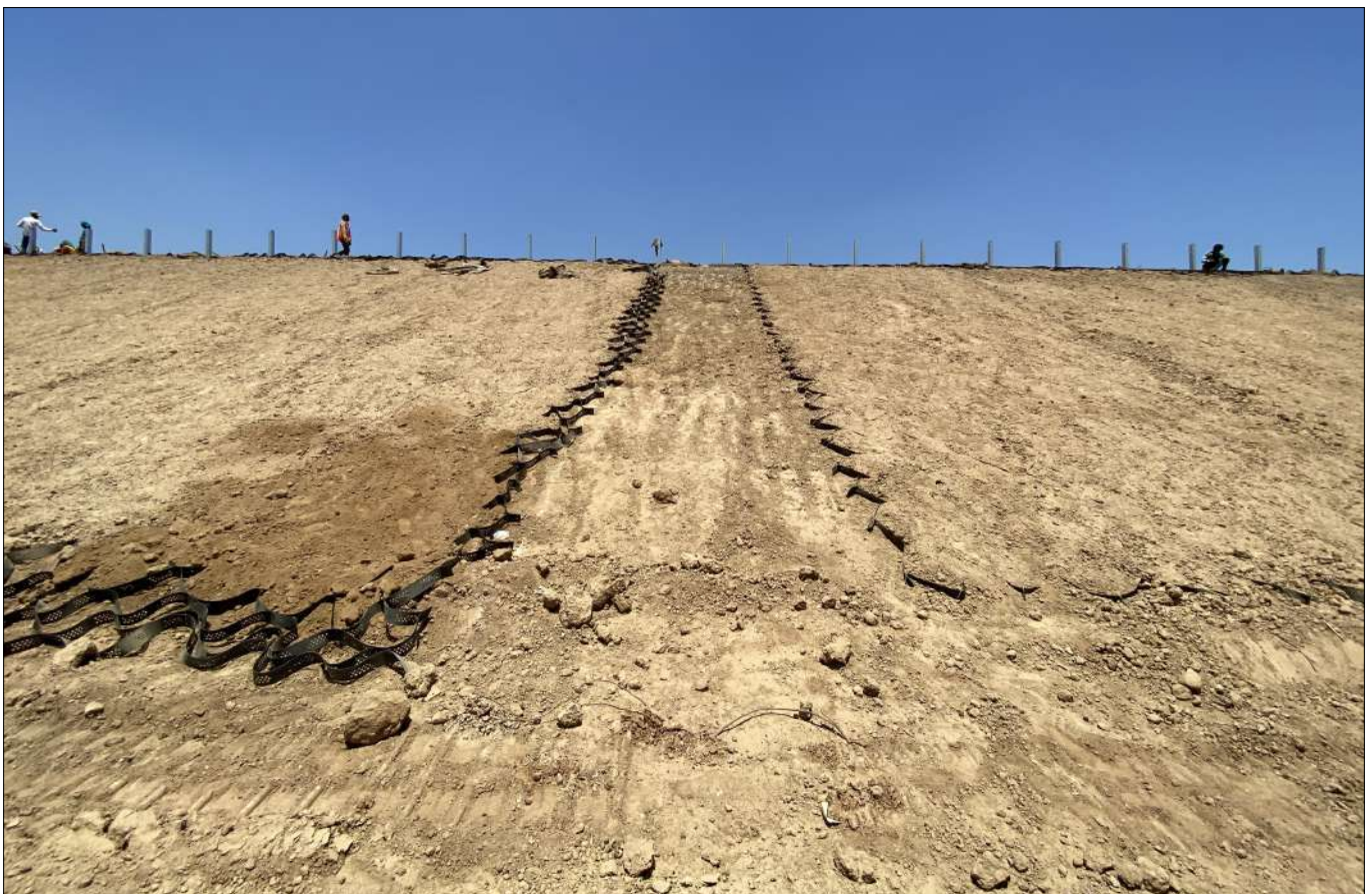
Photo 3 : Slope after filling of vegetative soil in Techcell Geocell
