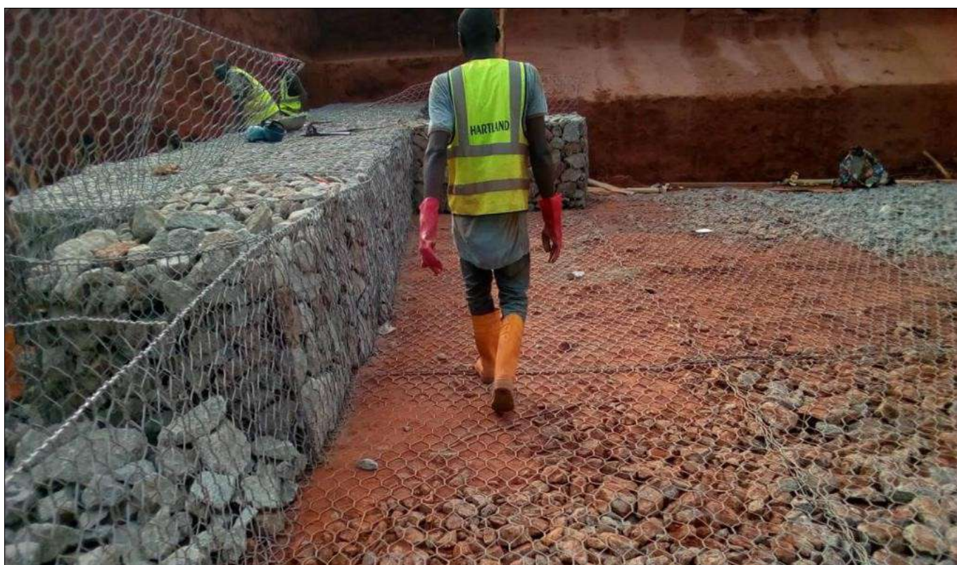
During Construction Photographs - Gabion filling with boulders
