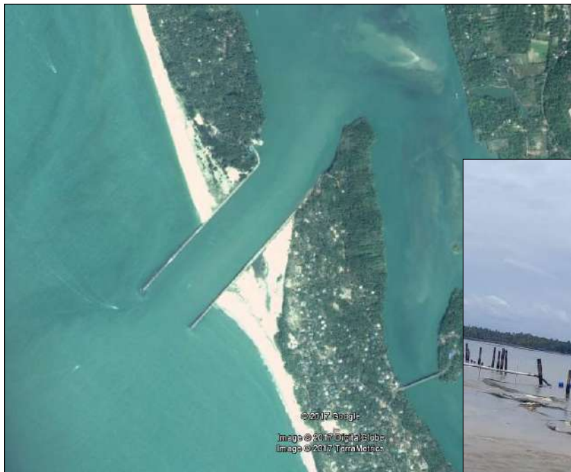
View of Artificial Island near Madakkara fishing harbour
