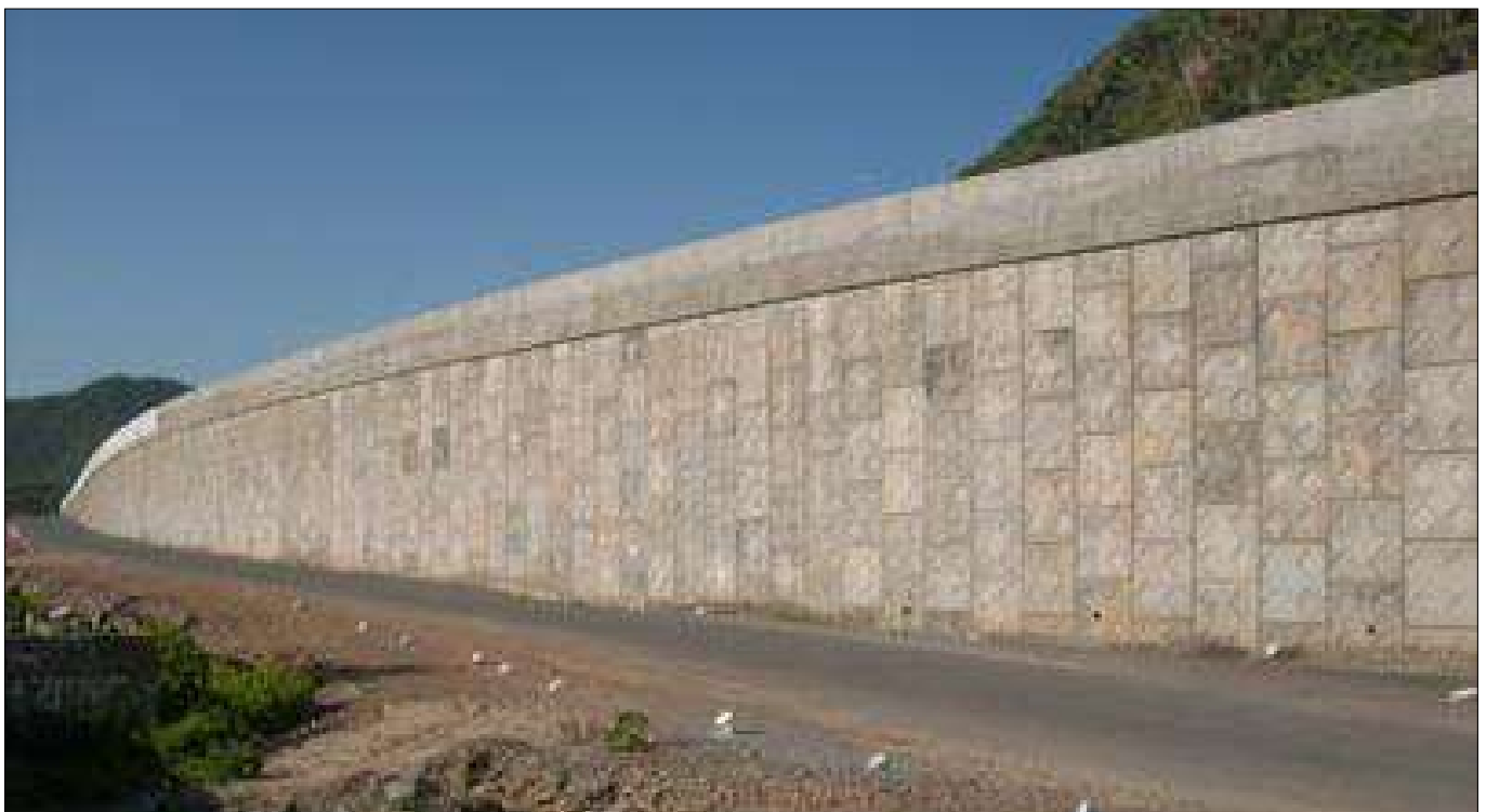
Photo 1 : Elevation view of RS Wall
