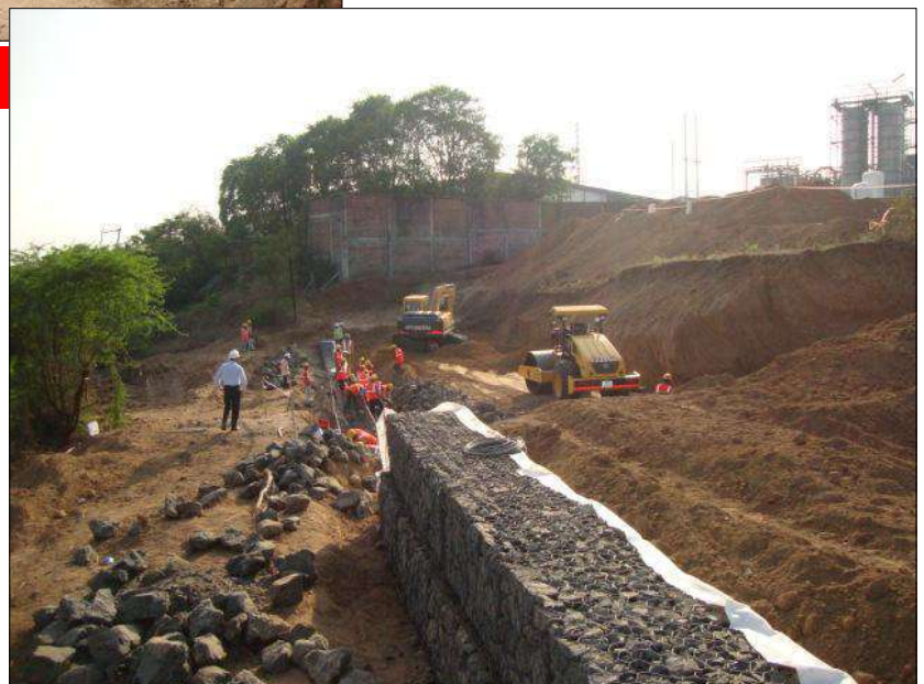
Installation of Gabion fascia units
