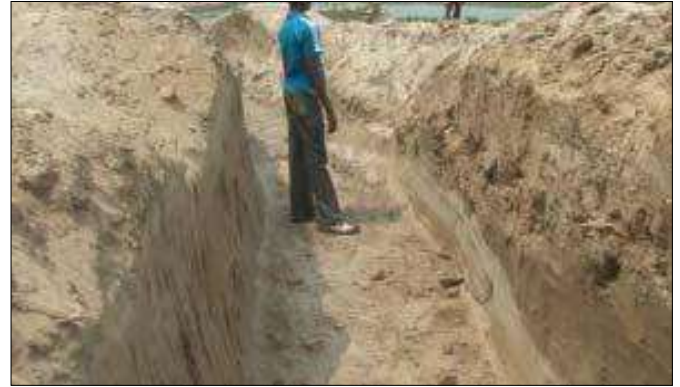
Excavation of Trench at the End
