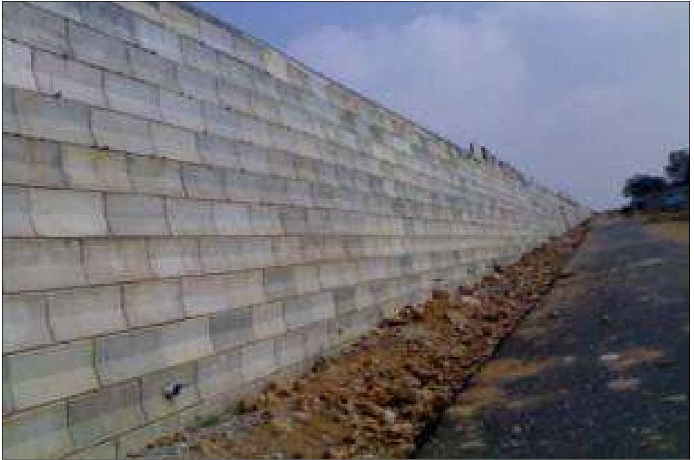
Elevation view of RS Wall
