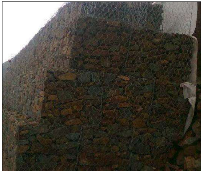
Photo 3: TechFab Metal Gabion Wall - Side View
