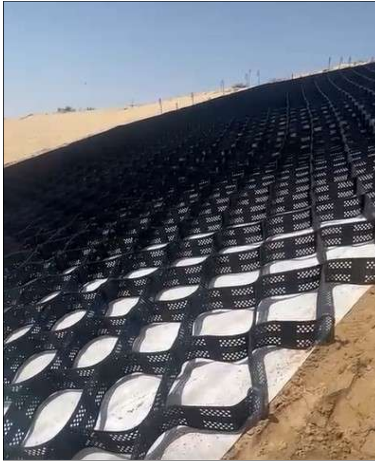
Photo 3 : During Construction Photograph
