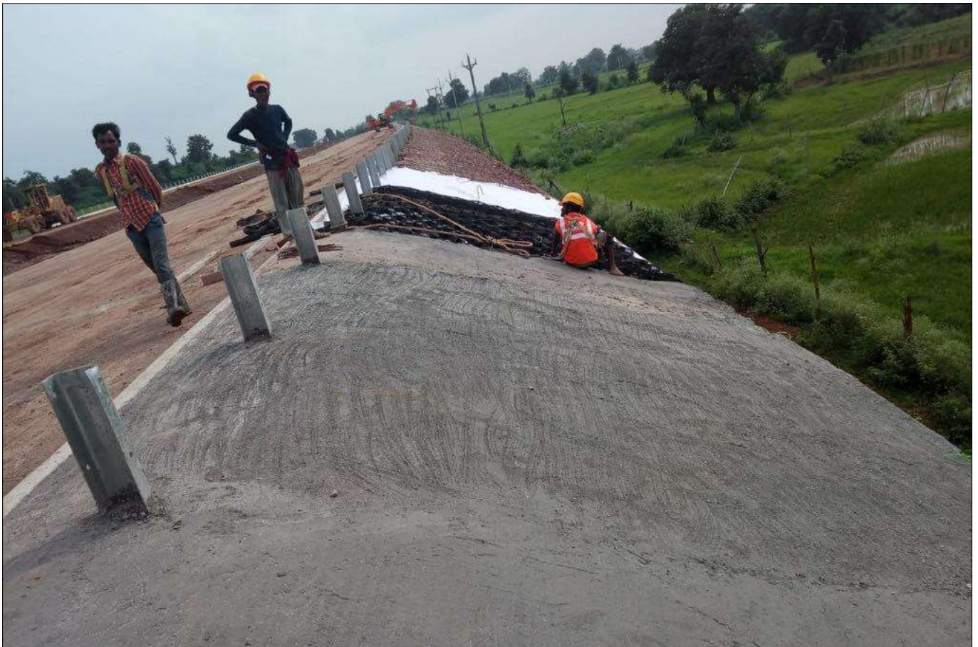
Progress of Concrete filling in Geocell
