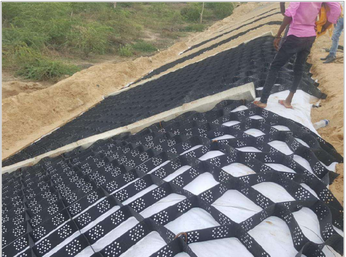
Installation of Nonwoven Geotextile & Geocell completed
