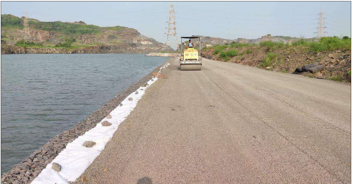
Figure 7 : Compaction behind the wall in progress
