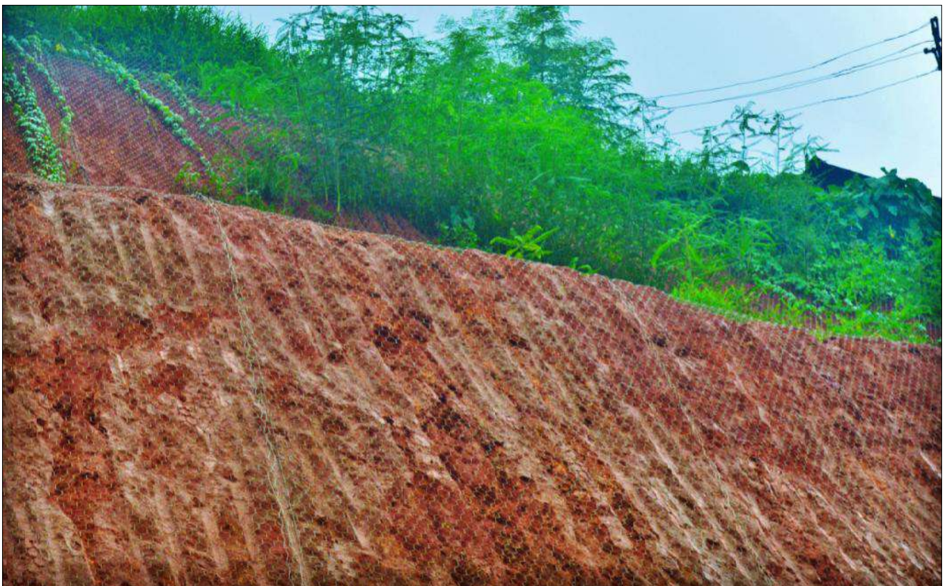
Slope after installation of Rockfall Netting
