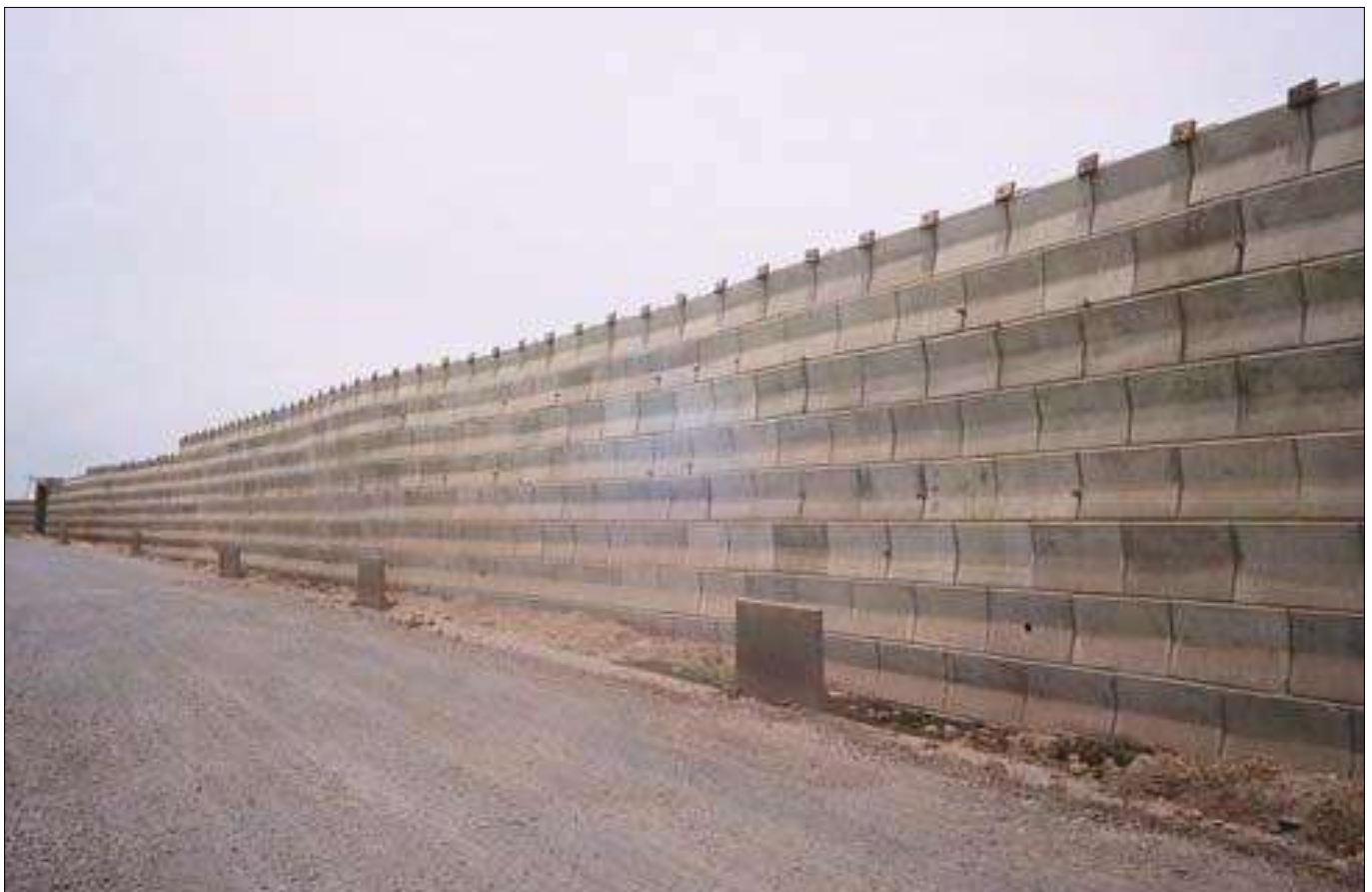
Elevation view of RS Wall
