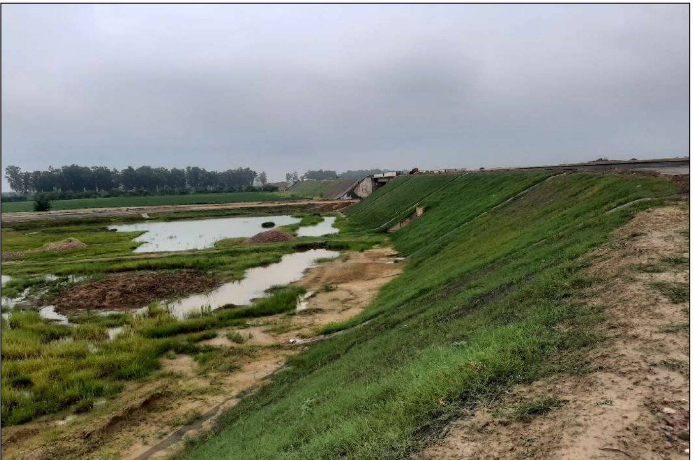
SCENIC VIEW OF PLANTATION GROWTH OVER SLOPE USING TECHGRID
