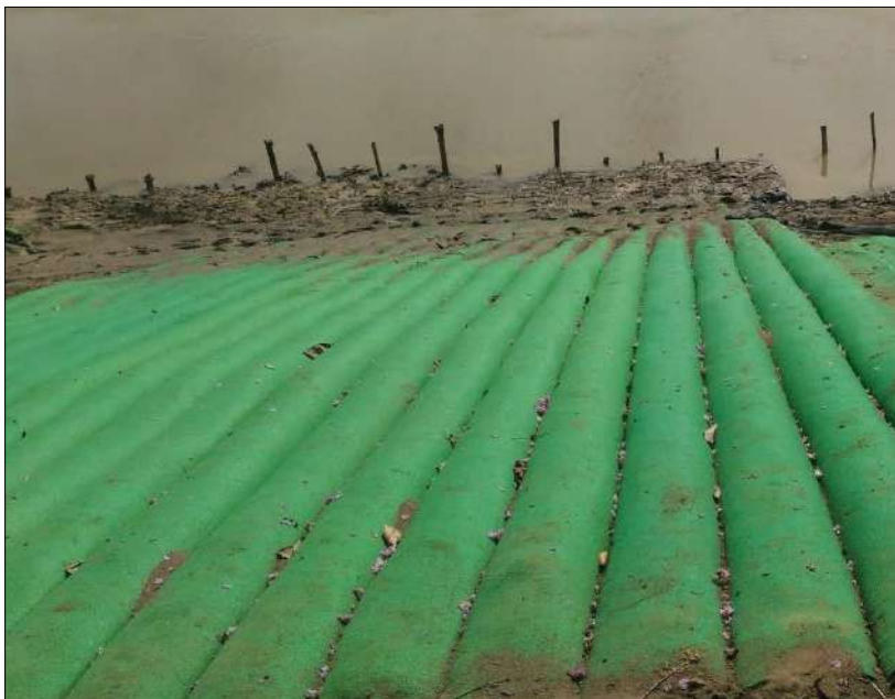
Photo 1 : Installation of Tech GeoMattress
