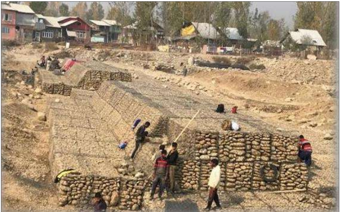
Photo 1: Gabion Installation in progress
