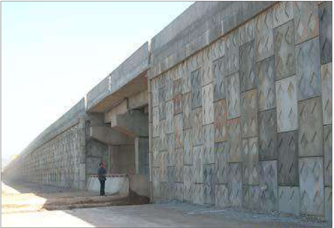
Elevation view of RS wall
