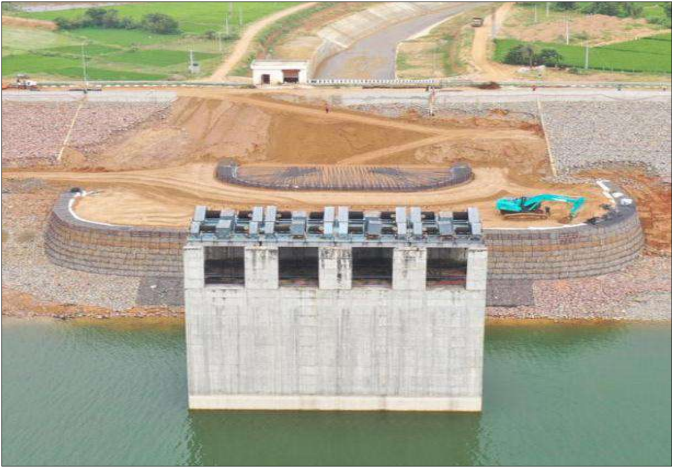
Photo 2 : During Construction - TechStrap Geostrips installation
