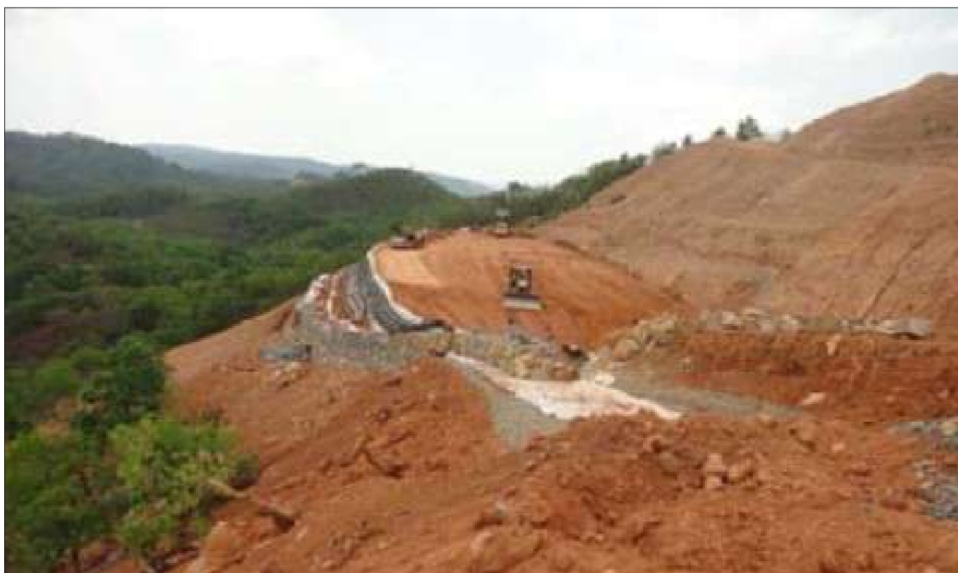
TechFab Metal Gabion Wall Layout – Initial Stage
