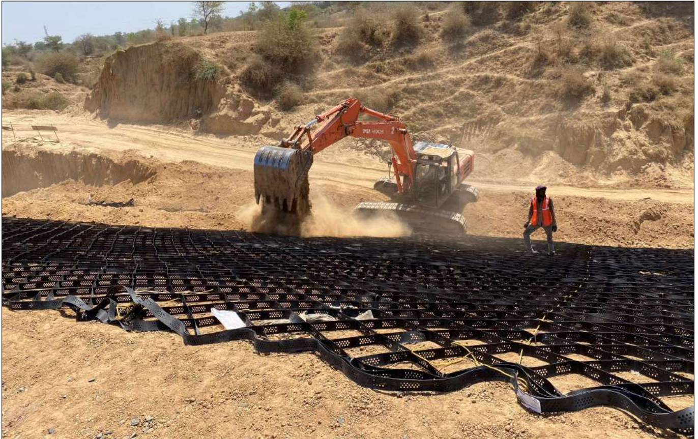
Photo 2 : Filling of vegetative soil in Techcell Geocell
