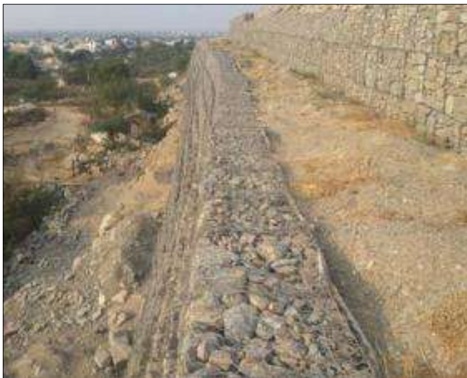
Two Tier Wall – Longitudinal View
