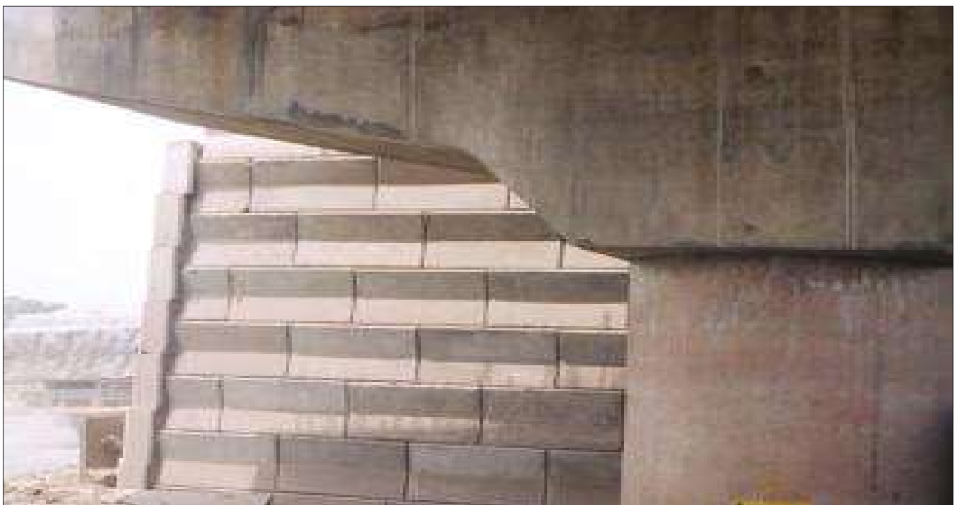
Abutment of RS Wall
