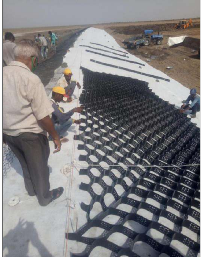
Techcell Geocell installation in progress
