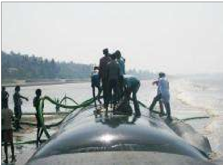
Installation of TechTube
