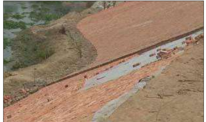
Two Layers of Brick Placed Along the Slope
