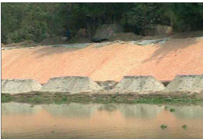
After Rehabilitation – Churni River Bank
