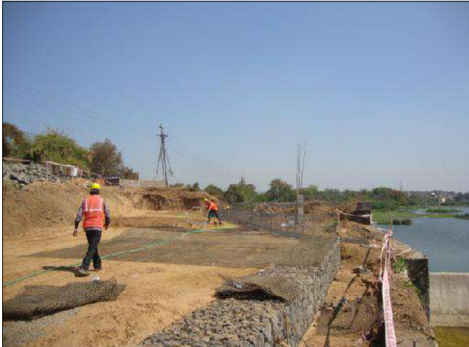
Installation of TechGrid Geogrid
