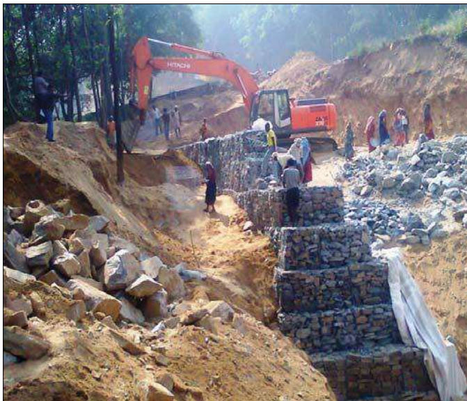
Photo 1 & 2 : TechFab Metal Gabion Installation in progress
