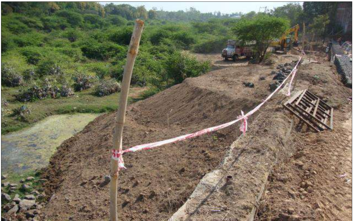
Orsang river bank - Before Construction
