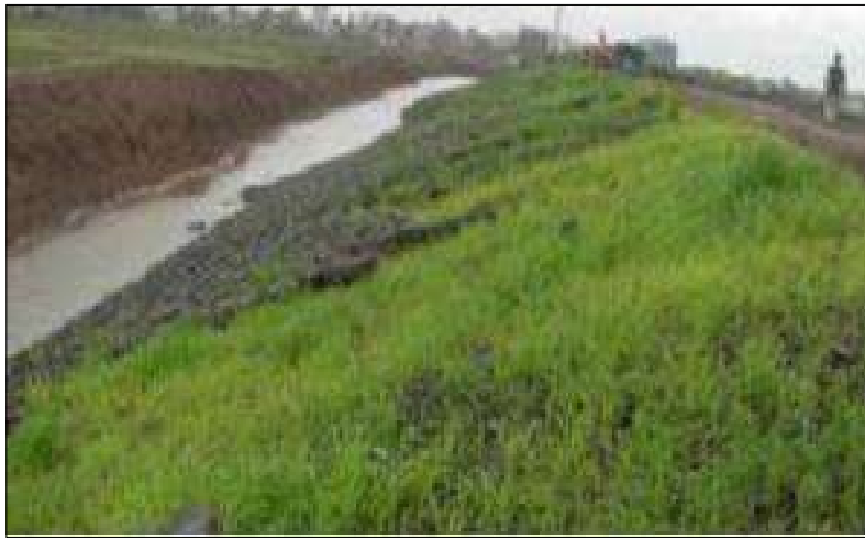
Embankment work in progress & partially completed
