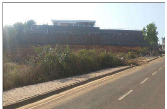
Fig 5 : After Construction - View from far
