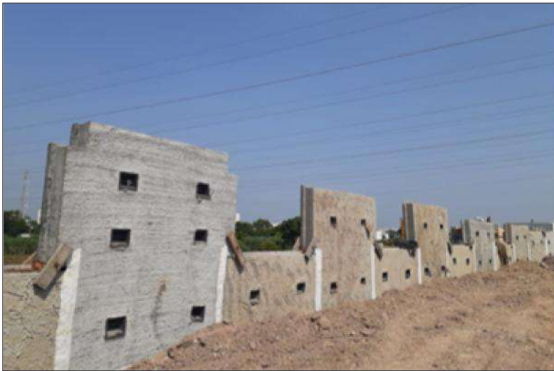
Erection of RCC Facia Panel in Progress
