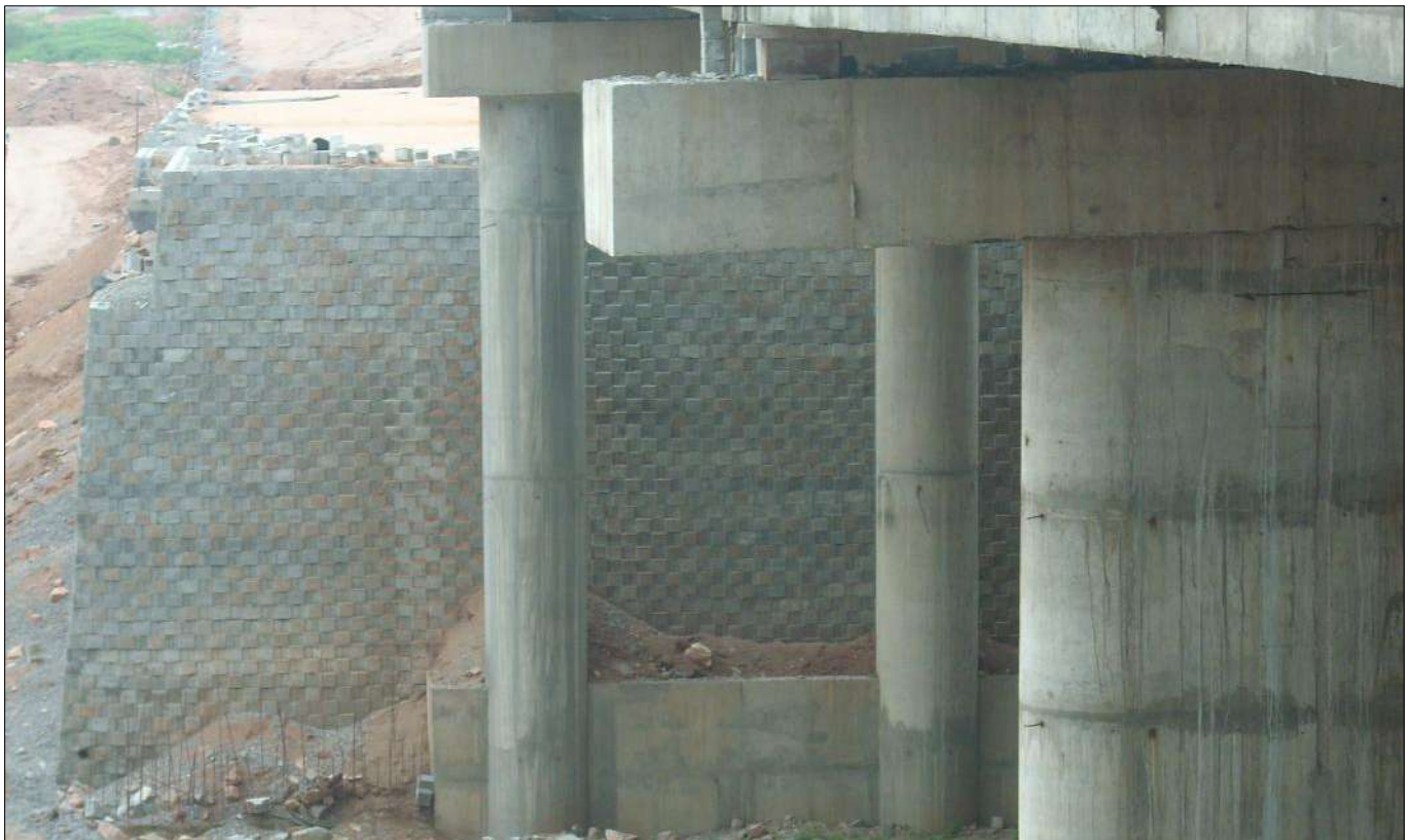
Photo 2 : Abutment RS wall
