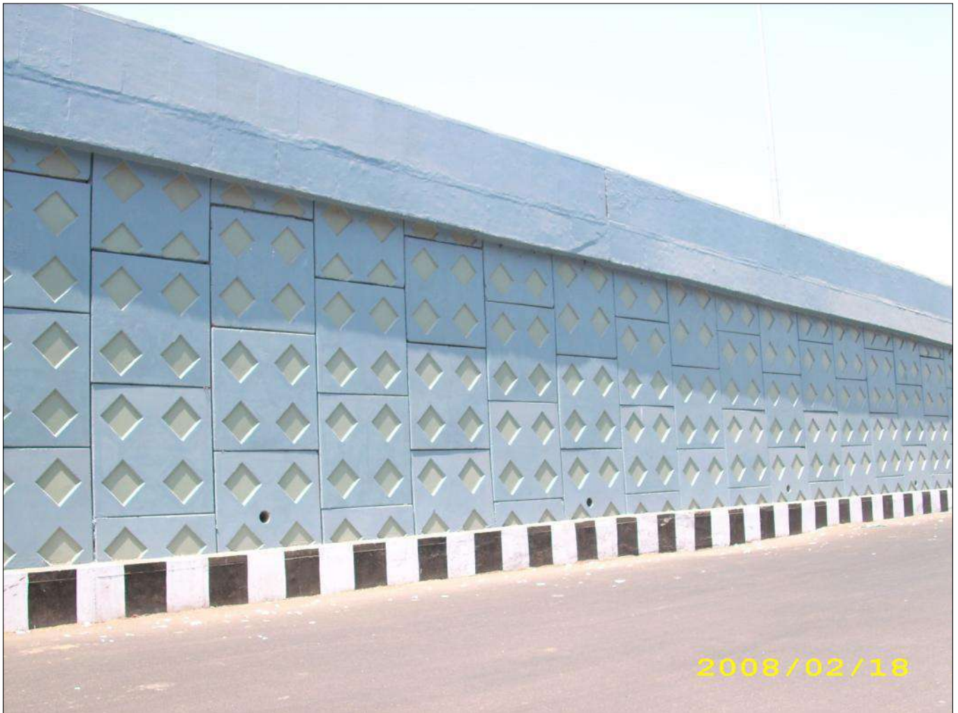
Elevation view of RS wall
