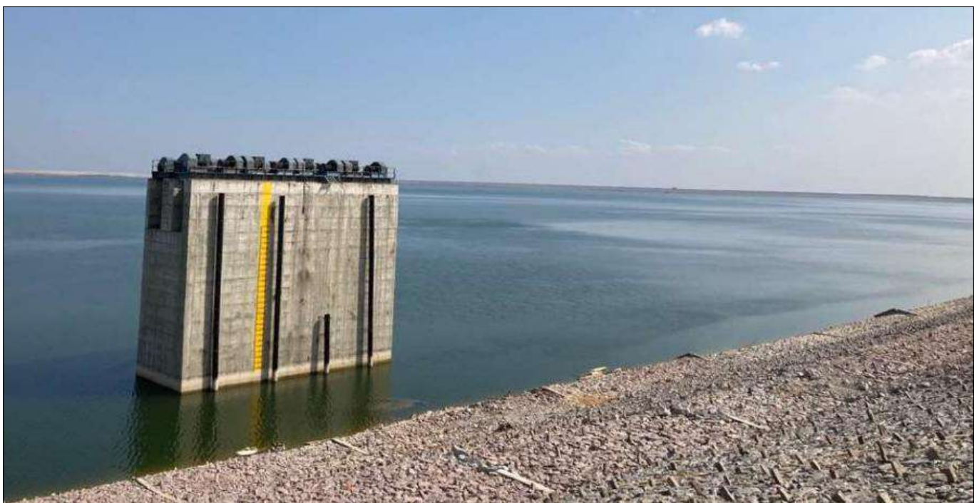
Photo 1 : Photograph of Reservoir before construction of Reinforced Soil Wall
