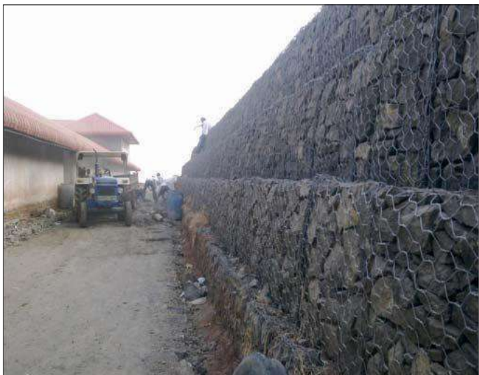
TechFab Metal Gabion - Installation
