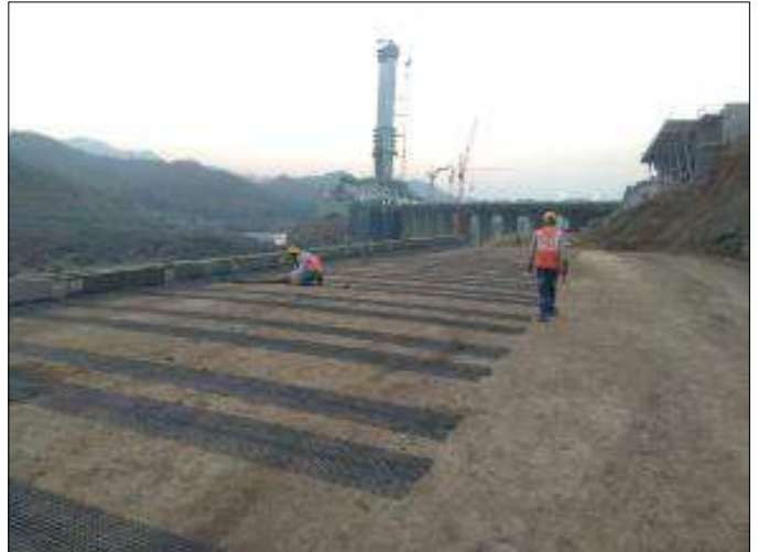
Geogrid Laying for RS Walls
