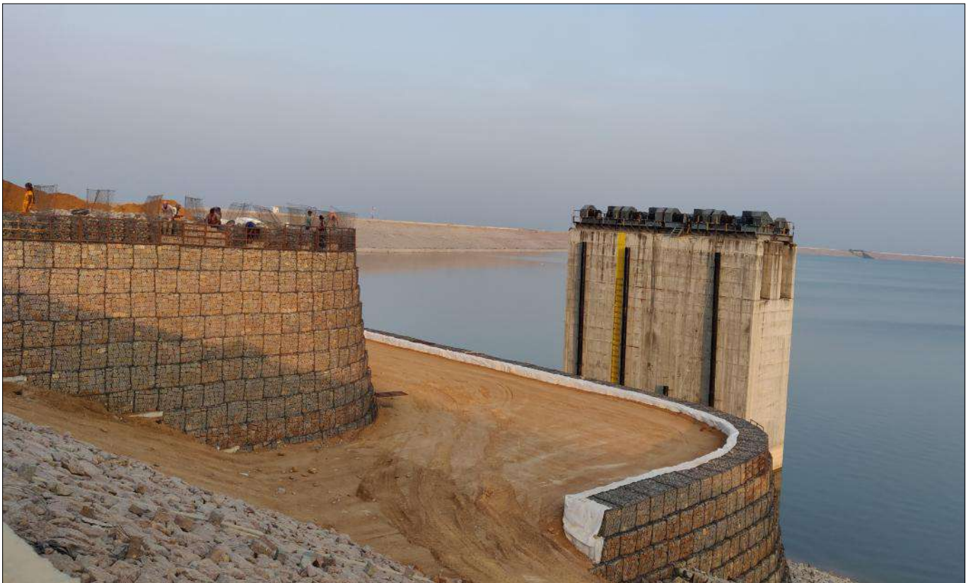
Photo 3 : Installation of Gabion fascia units on Top wall
