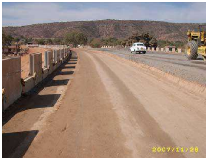
Photo 2 & 3: Erection of RS wall
