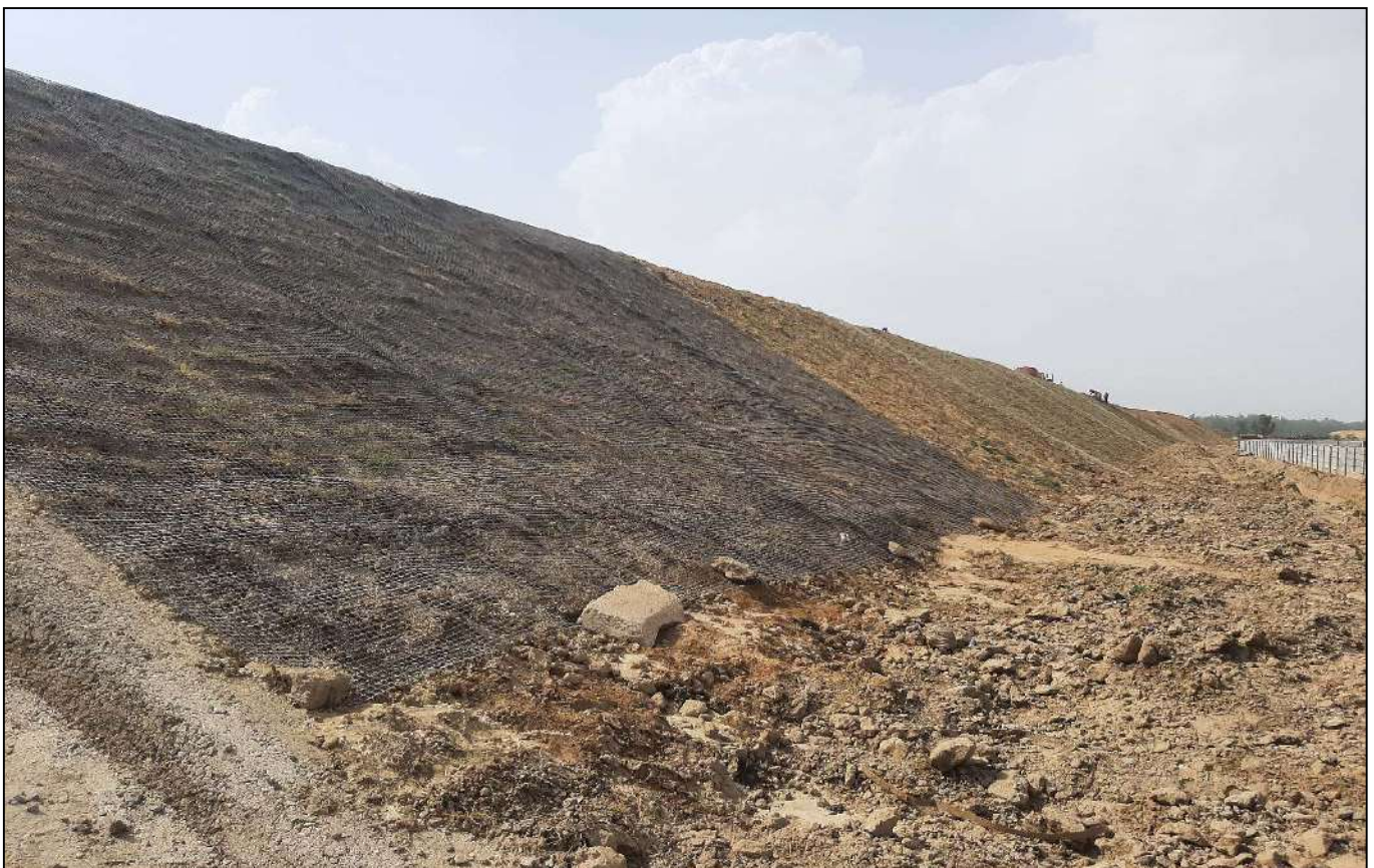
LAYING OF TECHGRID OVER THE SLOPE
