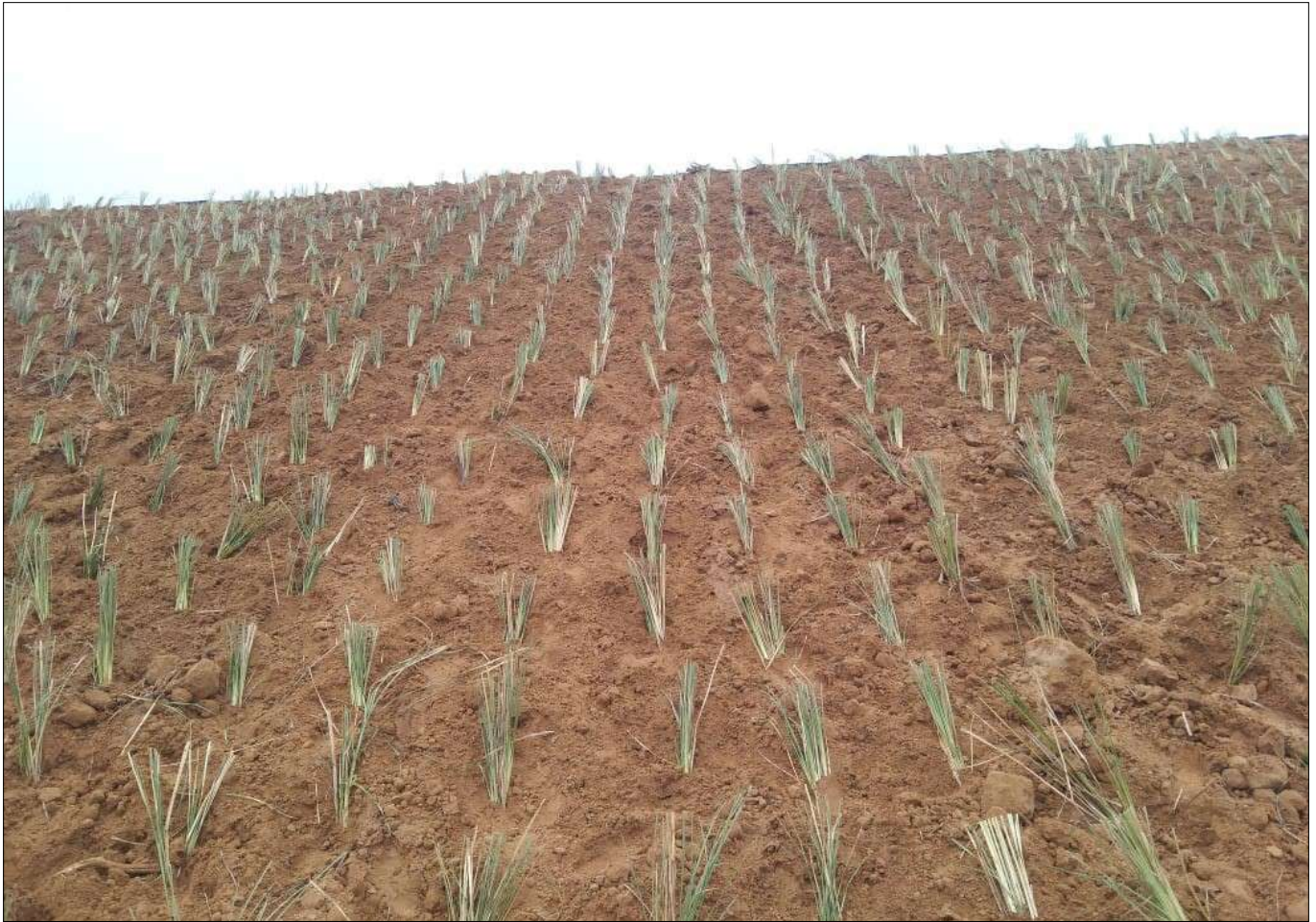
Photo 5 : Grass was planted on finished surface of road embankment
