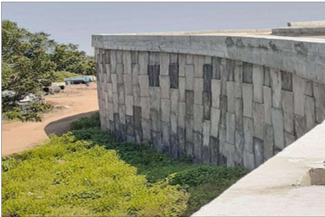
Completed Reinforced Soil Wall with Panel Facia and TechStrap Reinforcement
