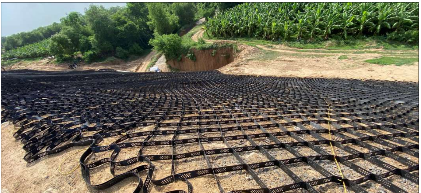
Photo 1 : Installation of Techcell Geocell over the embankment slope
