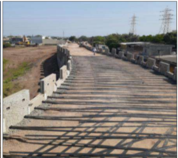
Installation of top layer TechStrap Polymeric Strip
