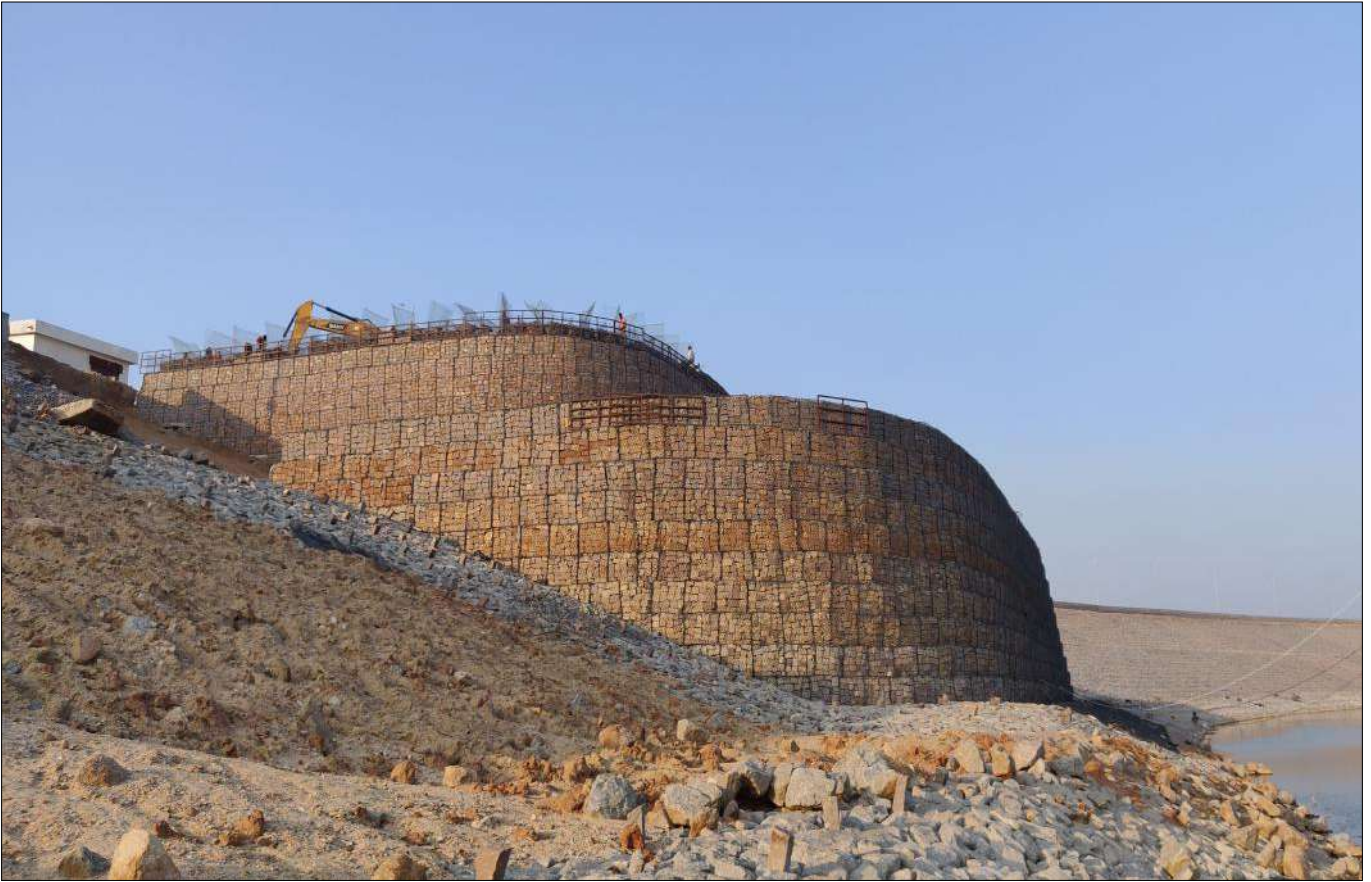
Photo 4 : During Construction - Top Wall
