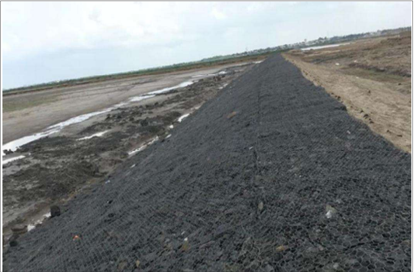
Sea side slope with Metal Gabion Mattress
