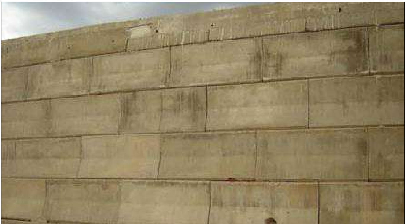
Photo 1 : Elevation view of RS wall
