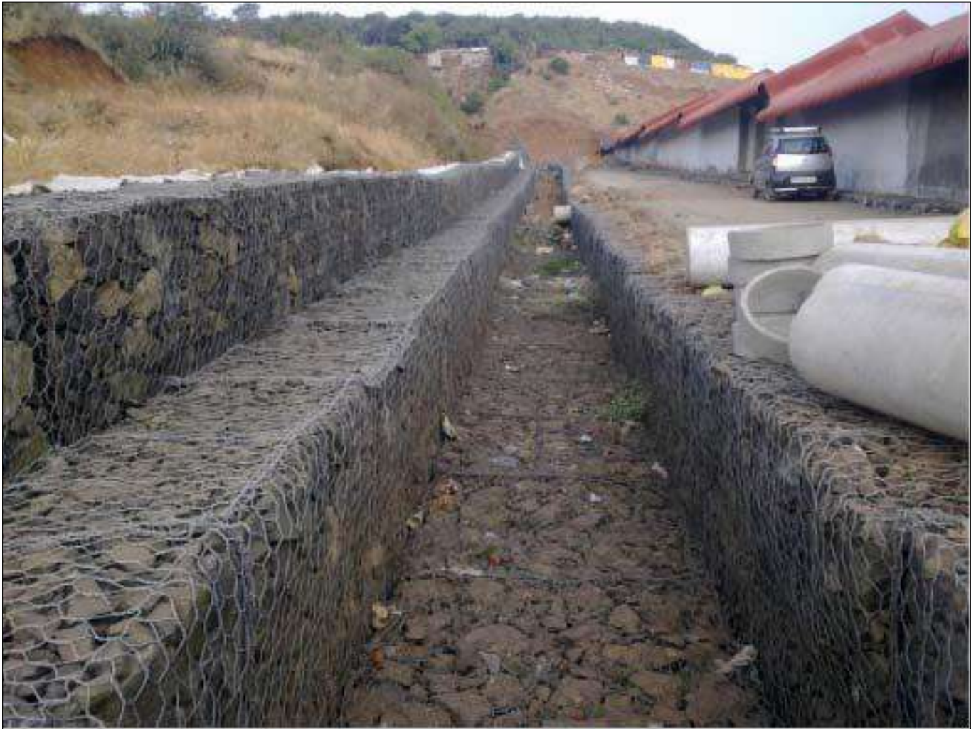
TechFab Metal Gabion - Longitudinal View
