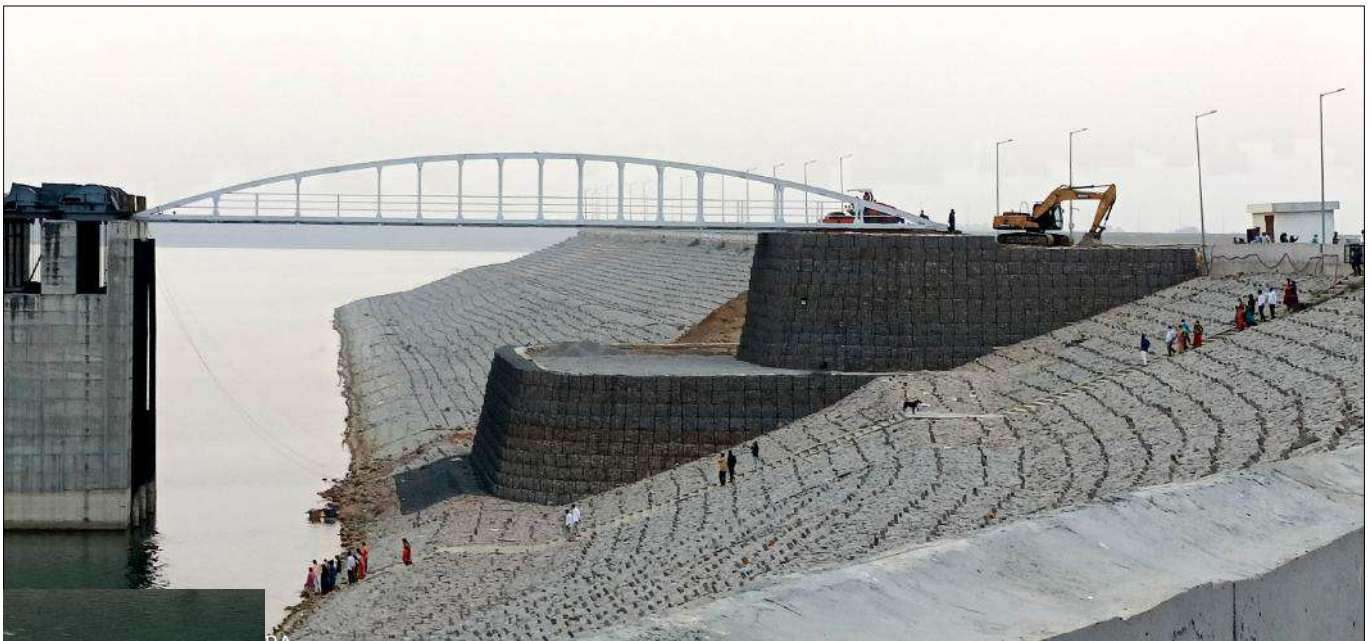
Photo 7 : Photograph of Completed Structure
