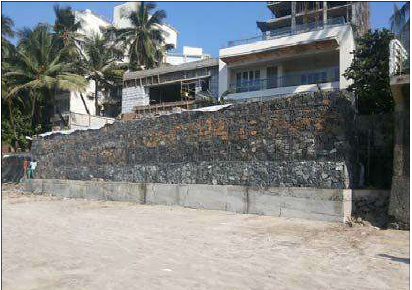
Photo 1 : TechFab Metal Gabion - Longitudinal view
