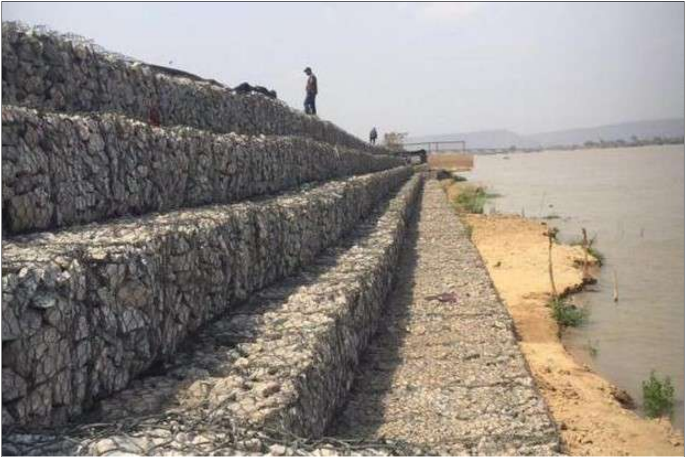
Completed Structure of Gabion Wall
