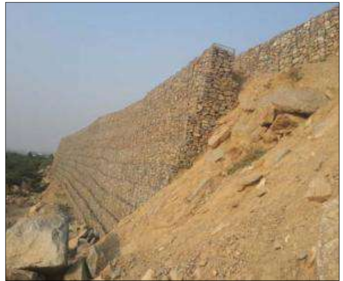
Construction Stage - II
