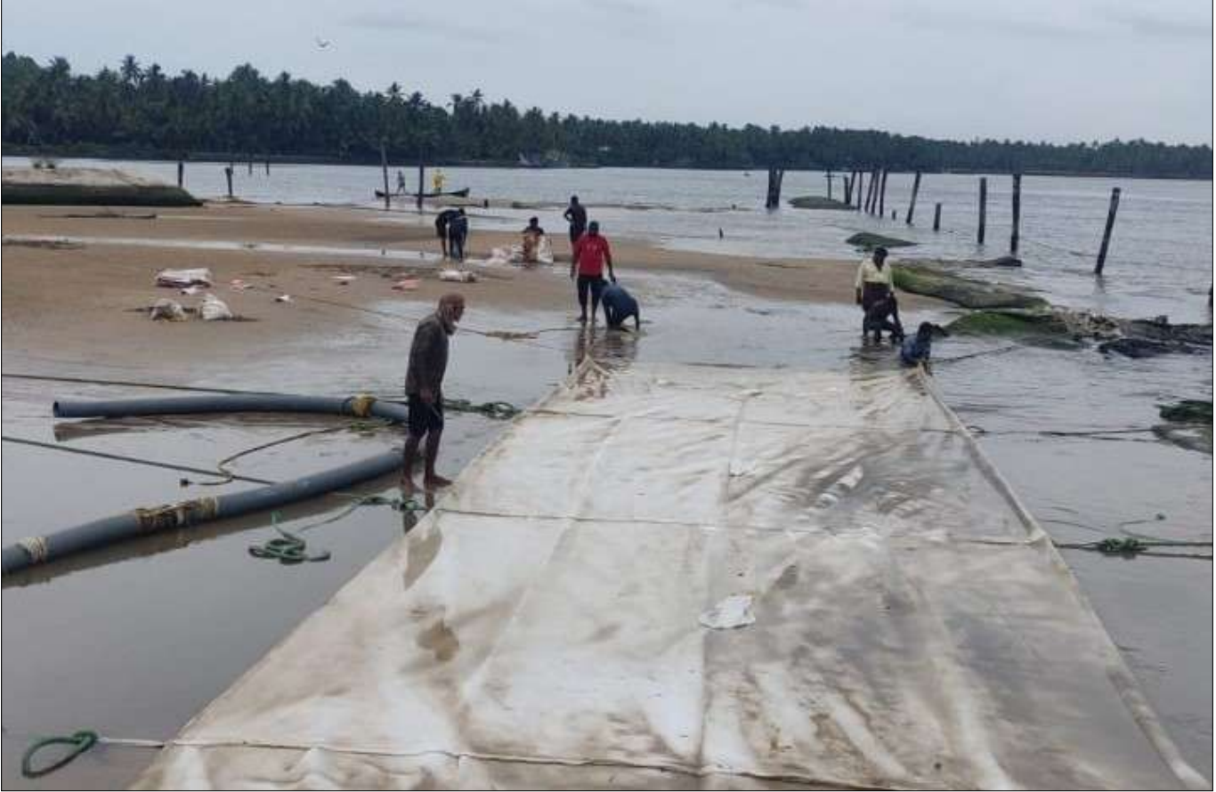
Laying of TechTube Geotextile Tubes in progress
