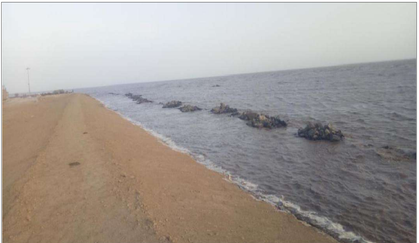
Prepared Embankment with low tide
