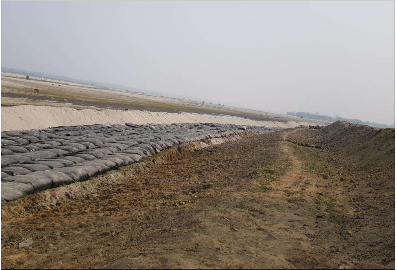
Photo 4 - Placement of Techfab Geotextile bags
