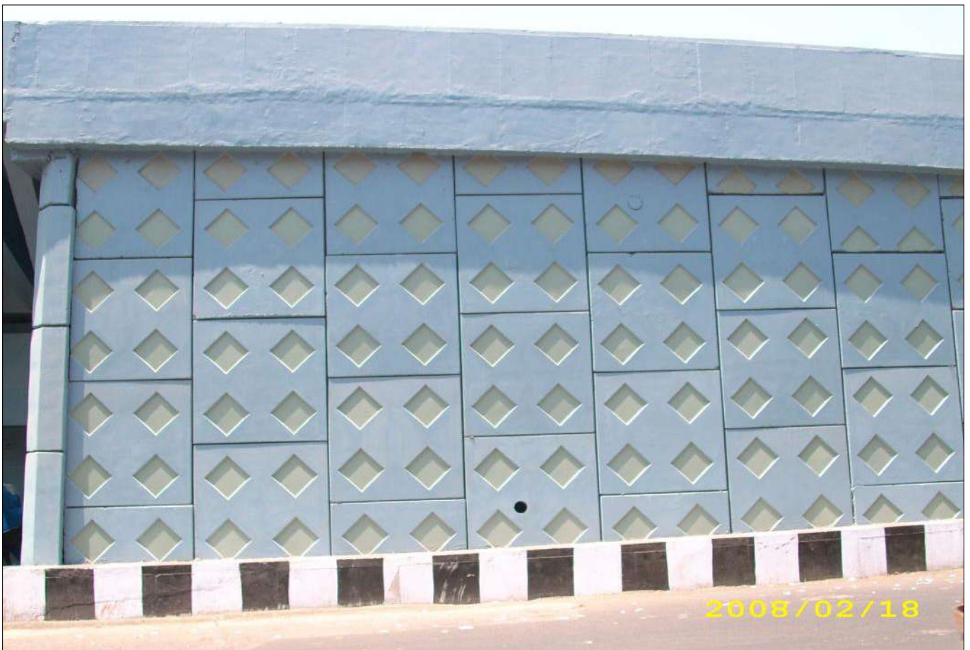
Elevation view of RS wall
