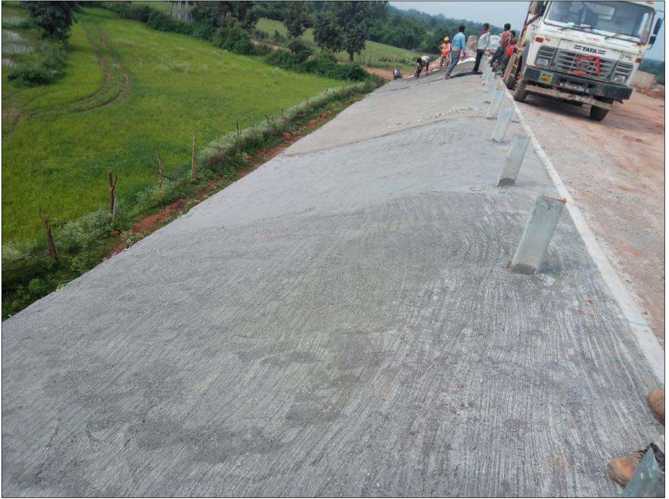
Finished surface of road embankment
