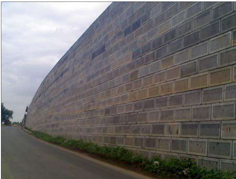
Photo 1 : Elevation view of Nagpur-Hyderabad Section
