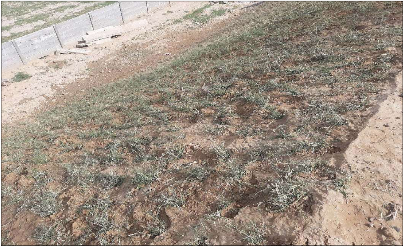
PLACEMENT OF GRASS OVER THE SLOPE
