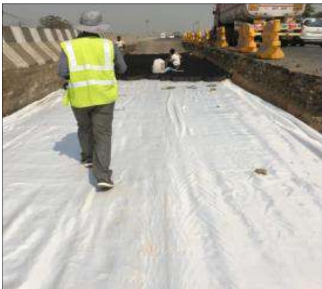
High Strength Woven PET Geotextile laid
