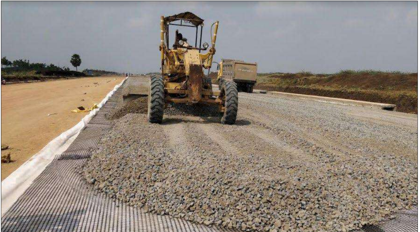
Spreading and compaction of GSB material on the geogrid + geotextile layer
