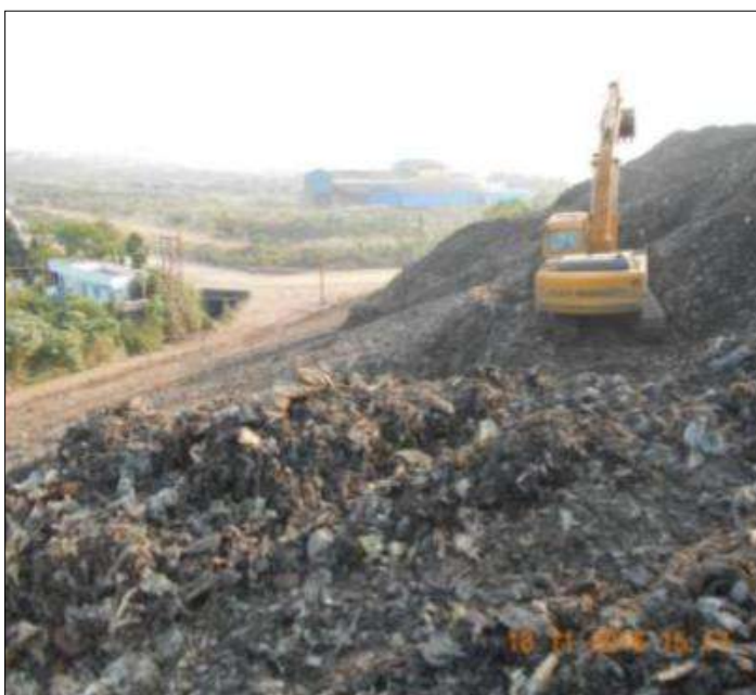
Excavation, Loading & Reshaping of waste
