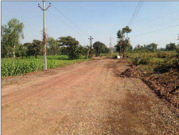
Earthwork after Scarifying Distressed
