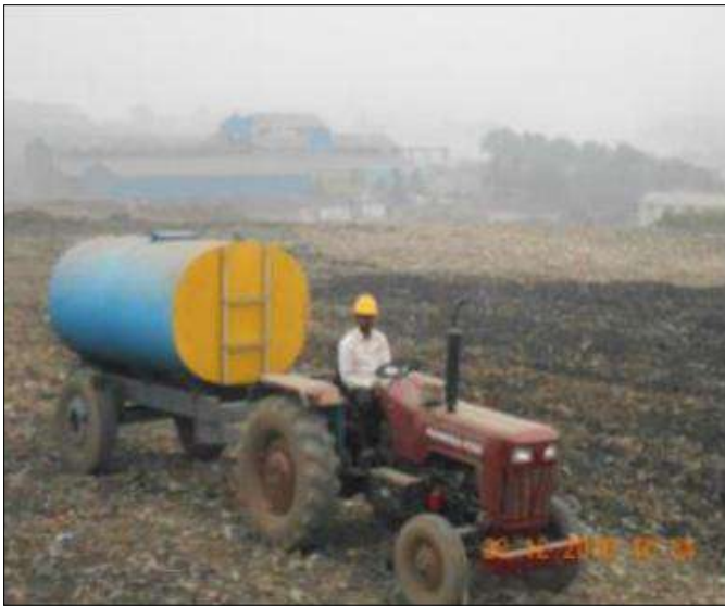
Maintaining moisture content by sprinkling water
