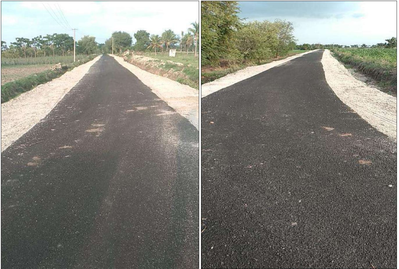
Road Pavement after completion
