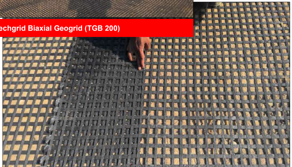
Photo 3 : Geogrid overlaps at the side edges
