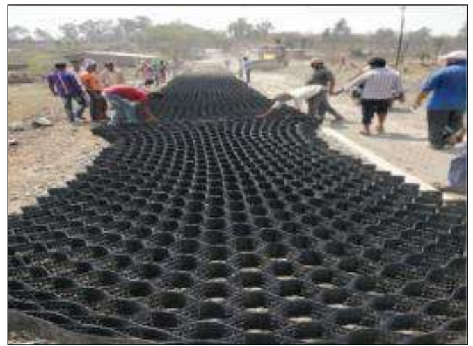
Laying of Techcell Geocell in Progress
