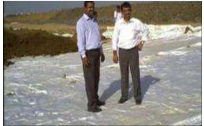
Laying of High Strength Geotextile TFI 3200
