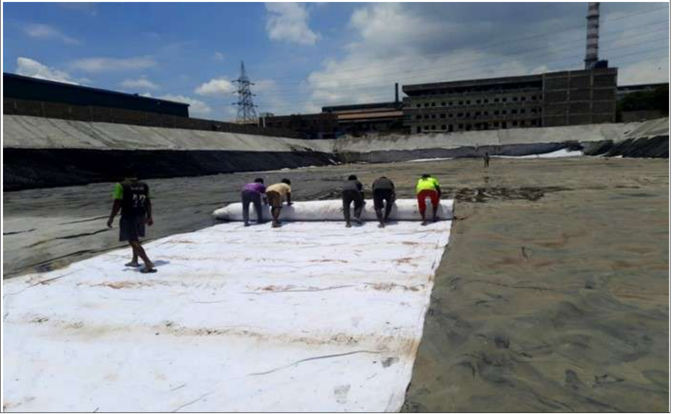
Photo 4 : Installation of second layer of geotextile on the top of geomembrane
