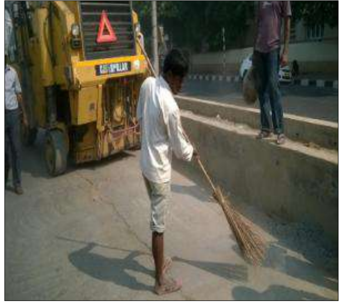
Surface Preparation Before Laying TechPave
