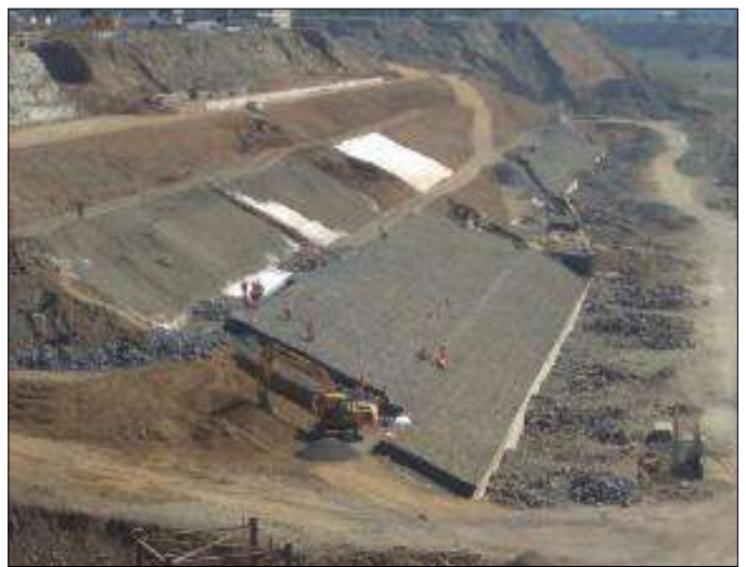
TechFab Metal Gabion Mattress laying in progress
