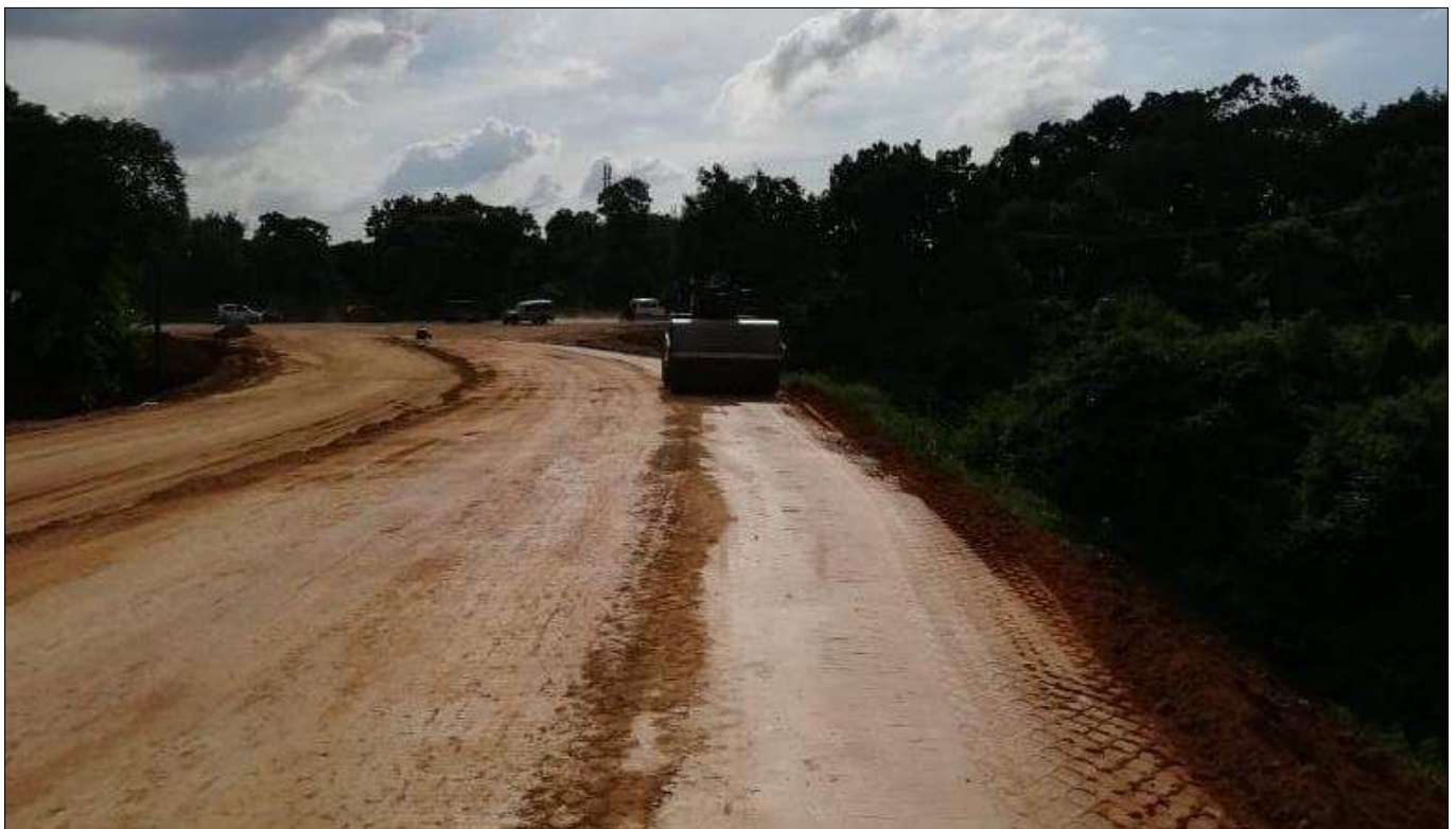
Fig 1 : Preparation of subgrade before laying granular layers.
