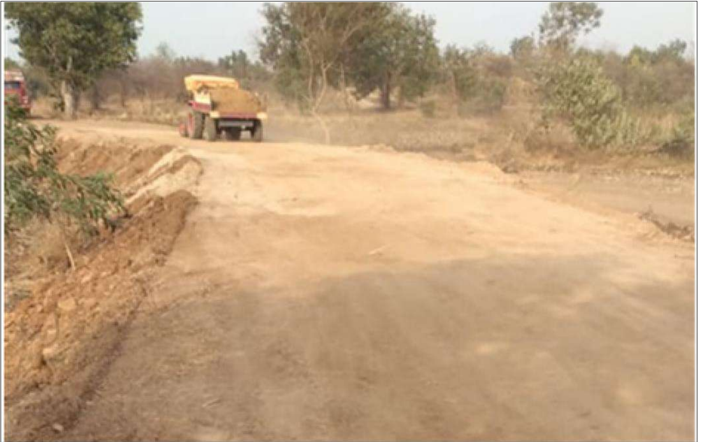
Road Pavement after completion of base layers
