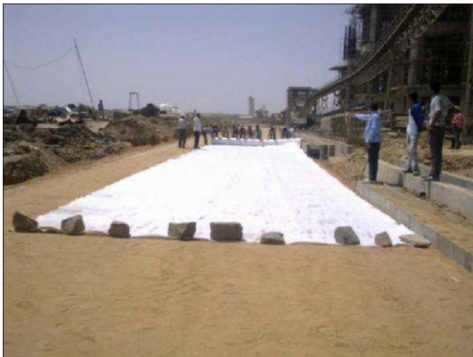
Fig 4 : Laying of TechGeo PR-20 (Non-Woven Geotextile)
