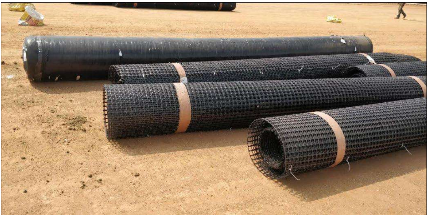
Rolls of Techgrid PP biaxial Geogrid and Techgeo Non-Woven Geotextile ready to be laid
