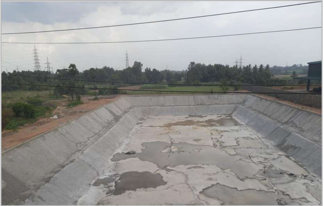
Photo 6 : Finished raw water reservoir lining
