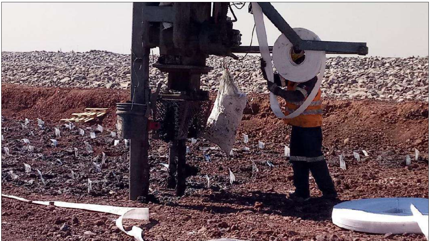
TechDrain PVD Installation in progress
