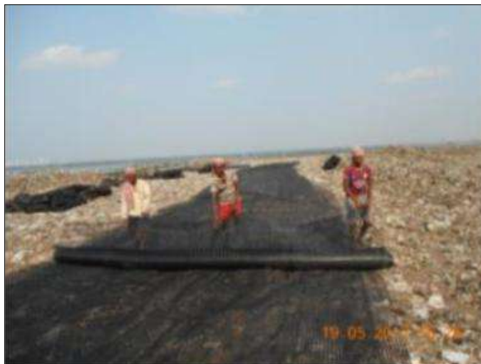
Laying of Geogrid
