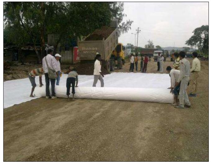
Laying of TFI PR-25
