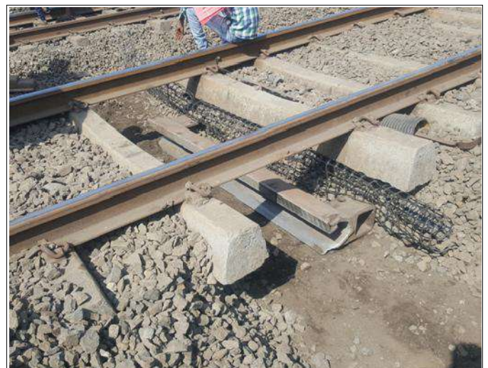
Placement of Sleeper Blade
