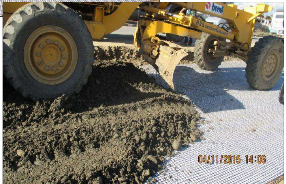
Laying of GSB on Geosynthetic Material
