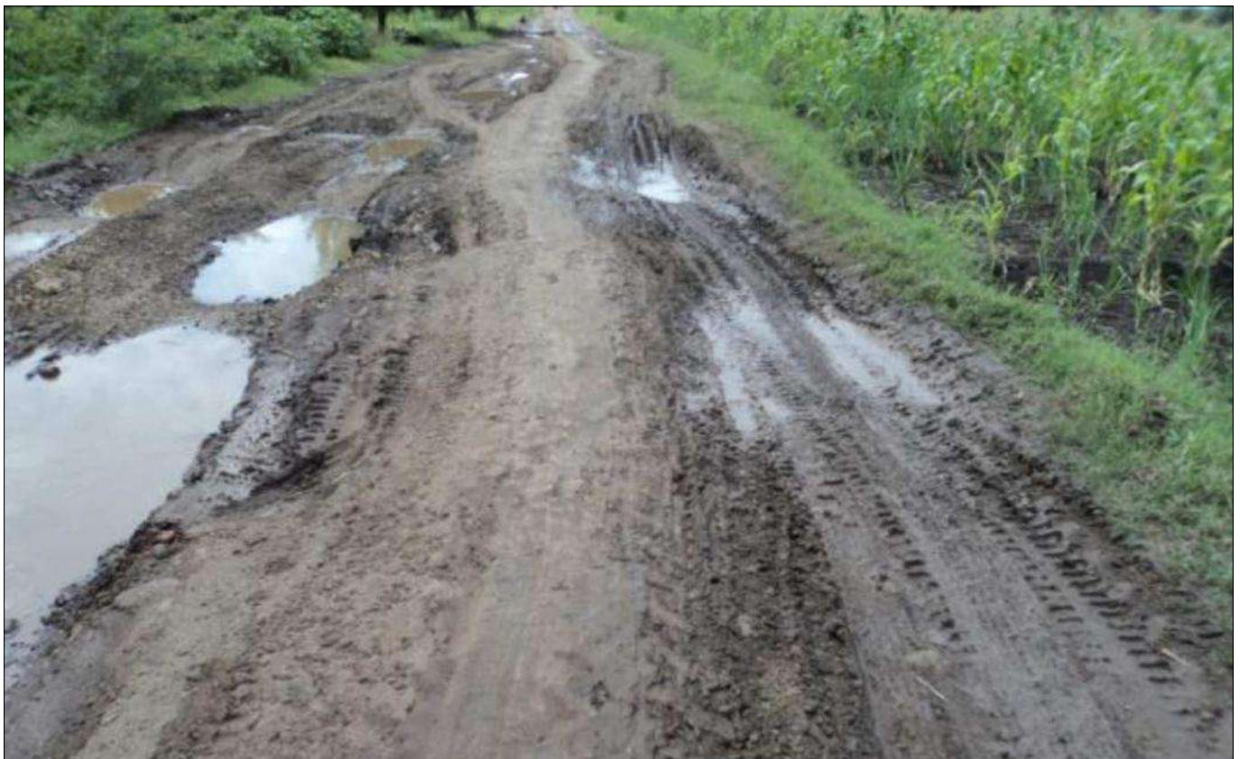
Original Site condition - In monsoon
