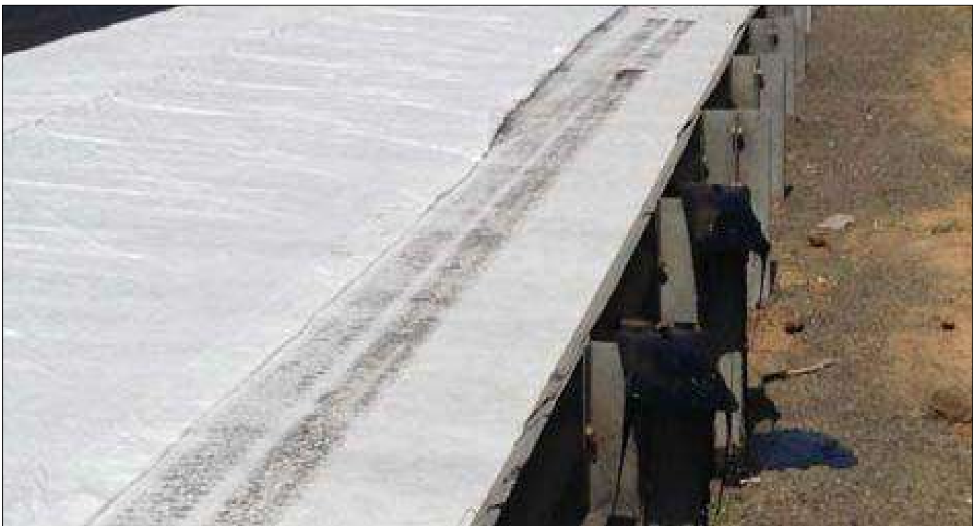
Installed TechFab Paving Fabric
