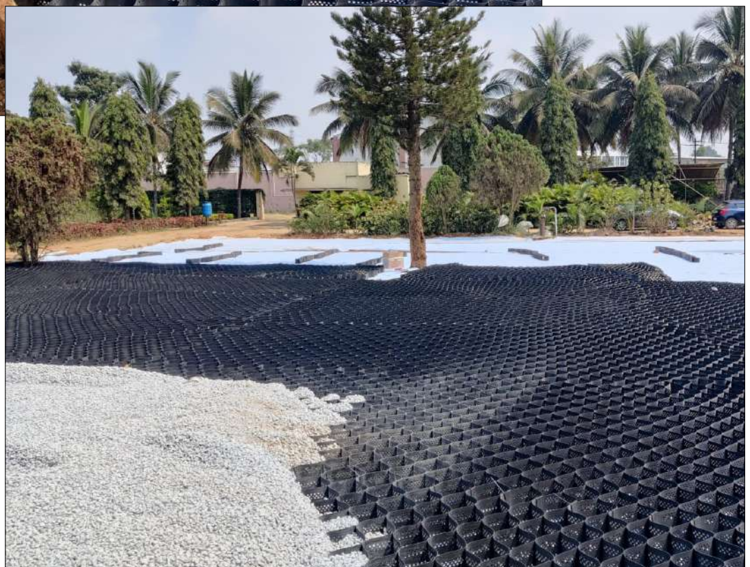
Photo 4 & 5 : Expansion of Techcell Geocell & Filling of Geocell with GSB
