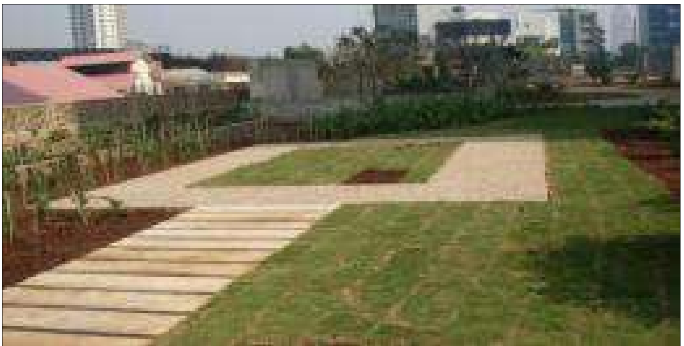
Fig 9 & 10 : completed Podium Garden / Landscape
