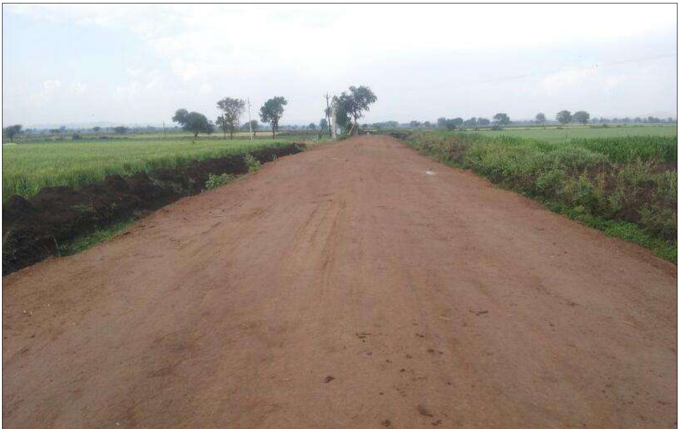
Photo 3 : Pavement Subgrade Surface is Prepared
