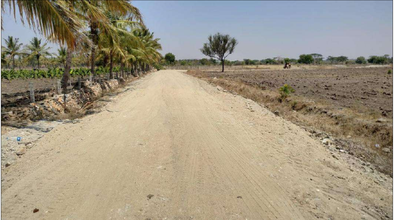
Compaction and preparation of subgrade for laying Techcell Geocell
