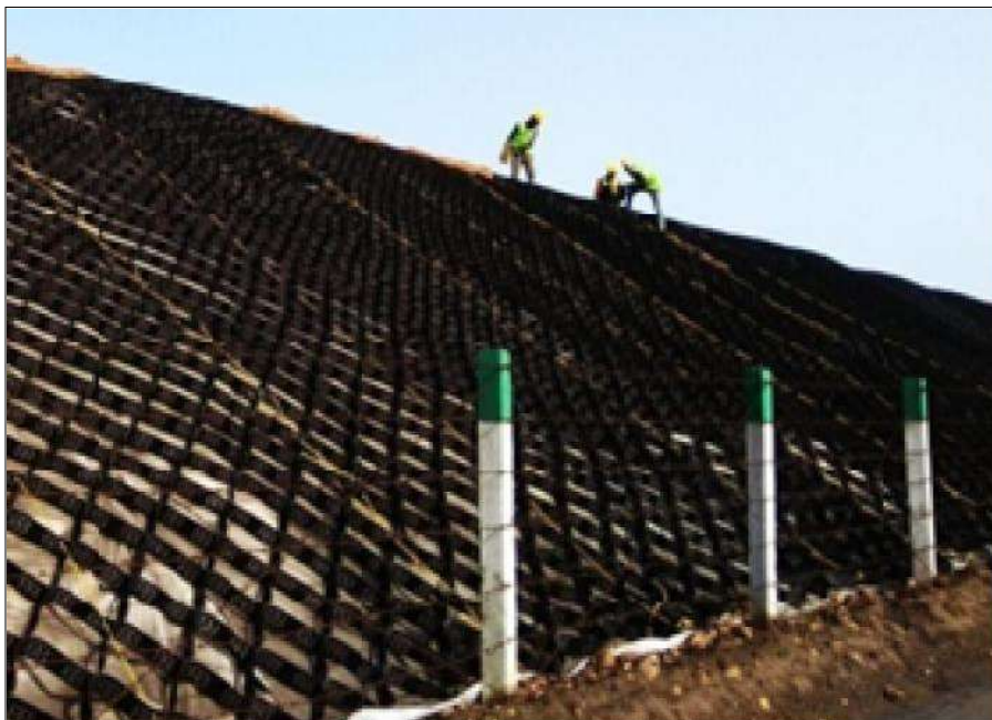
Laying of Techcell Geocell
