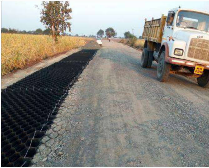
Laying of GSB in progress
