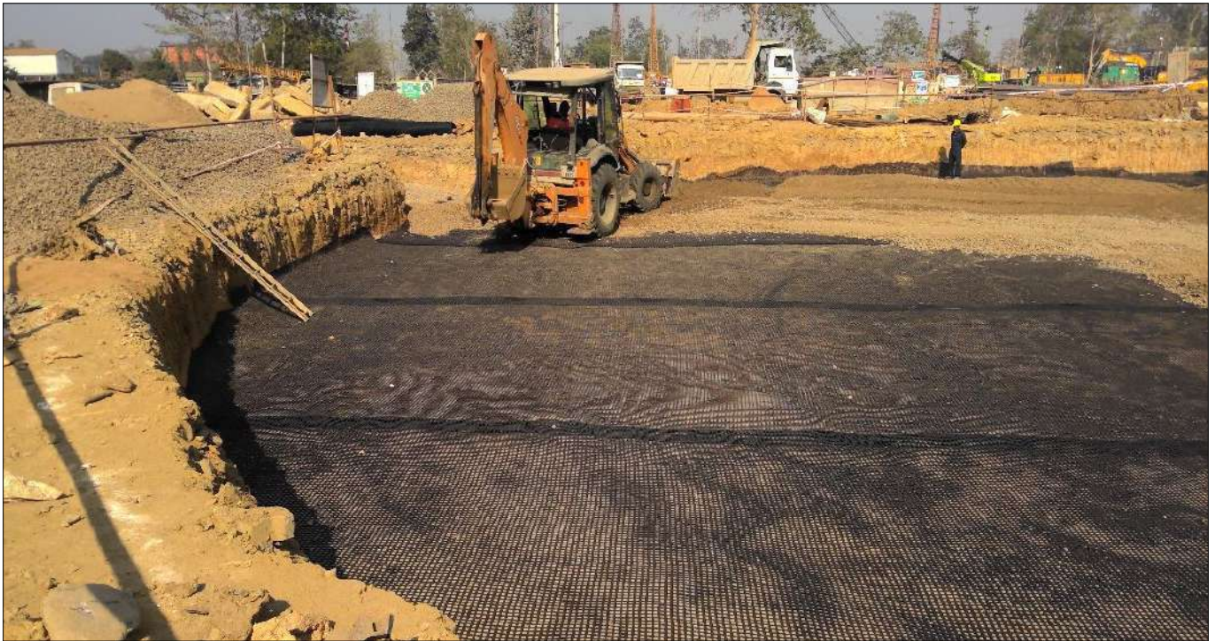
Photo 6 : Spreading of Fill Material
