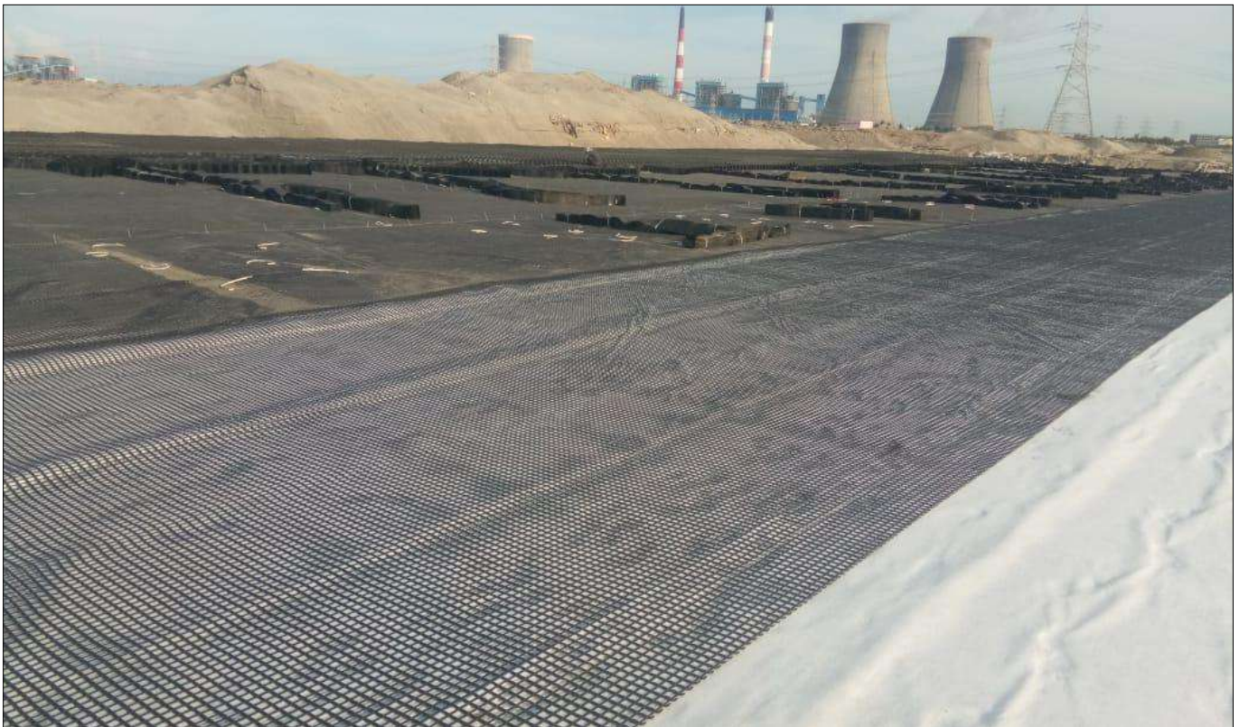
Photo 4 - Laying of TechGrid Biaxial Geogrid over geotextile
