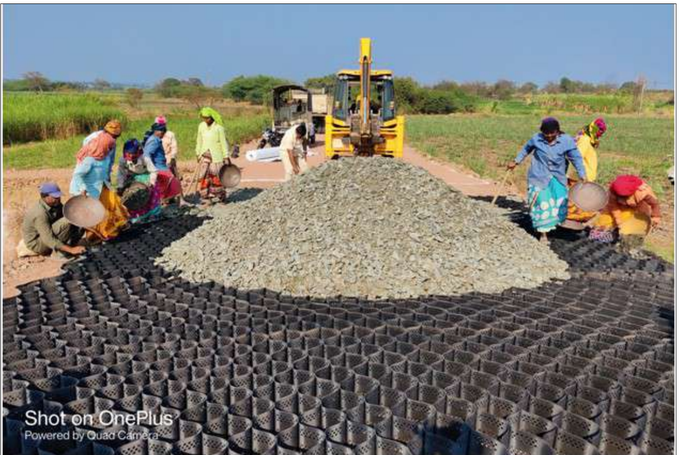
Techcell Geocell Stretched and Infill Material Dumped for Compaction
