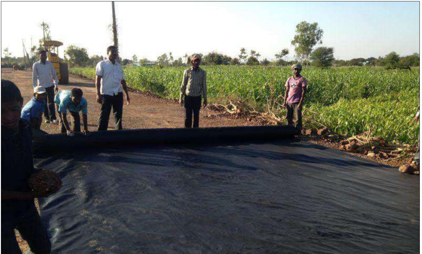
Laying of TFI-5300 Type-I
