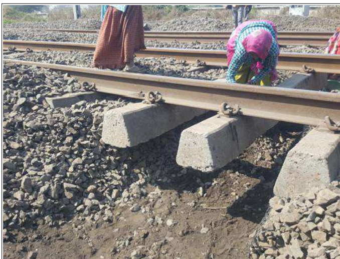
Manual Removal of Ballast in Progress
