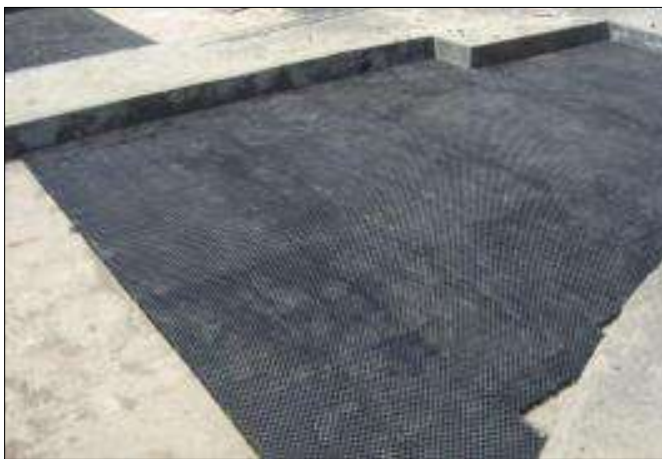
Fig 1 & 2 : Laying of Drain Board
