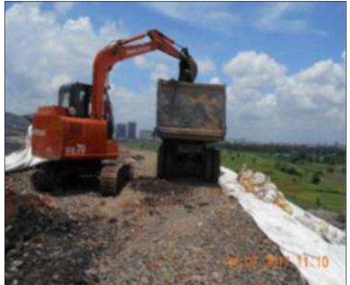
Laying of Geotextile
