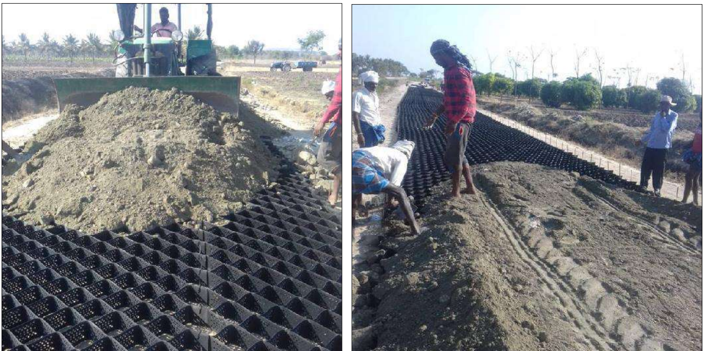
Filling and Compaction of granular material into the TechCell Geocell
