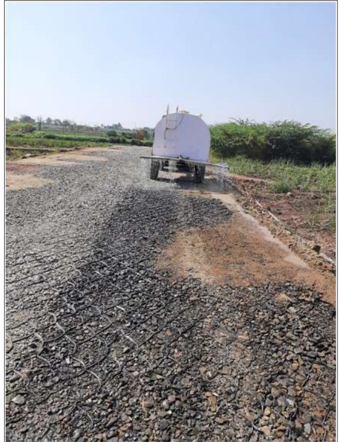
Compaction Process of Infill Material in the Geocell
