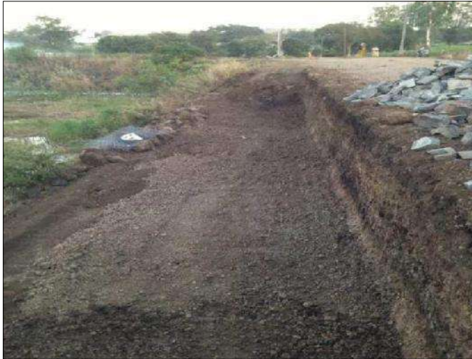
Excavation for Gabion Retaining Wall
