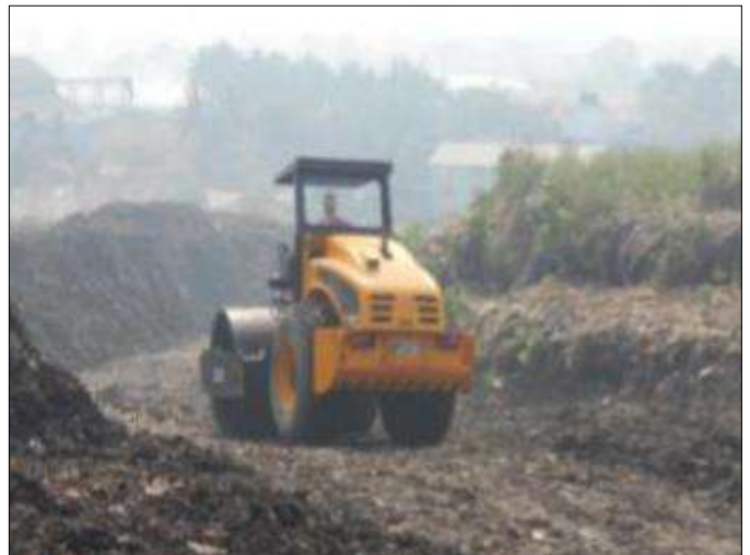
Compaction of waste by Vibratory Roller
