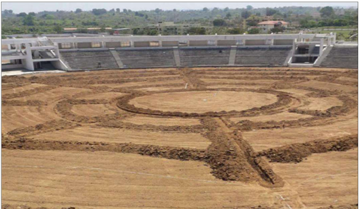
Excavation in progress for radial pipe drain
