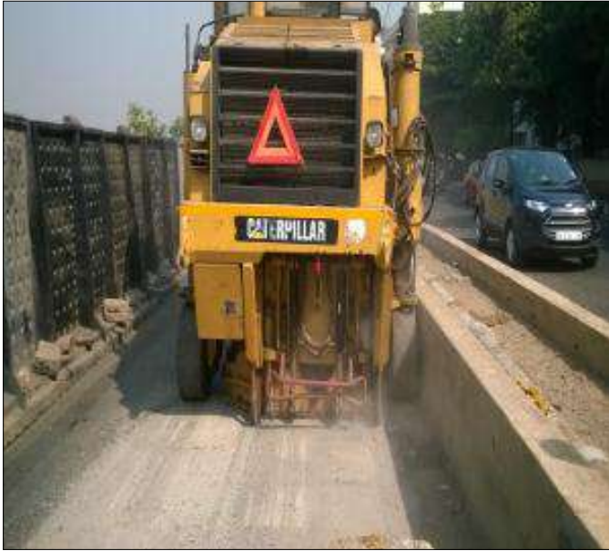
Milling Operation – Before Installation
