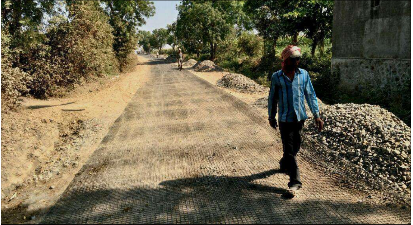
Photo 9 : Laying of TechGrid Geogrid TGB-40
