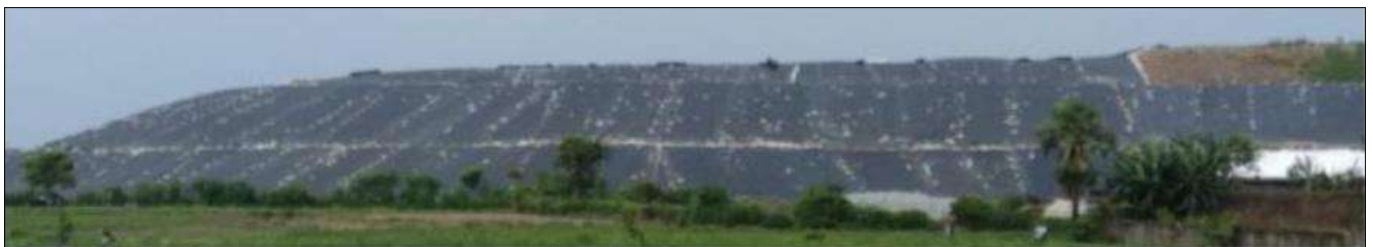
Laying of 1.5mm Both side Textured HDPE Liner
