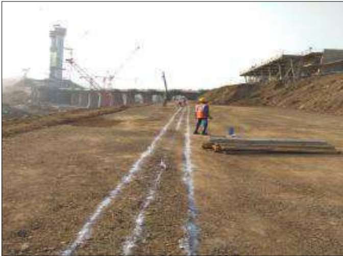
Marking in progress for RS Walls
