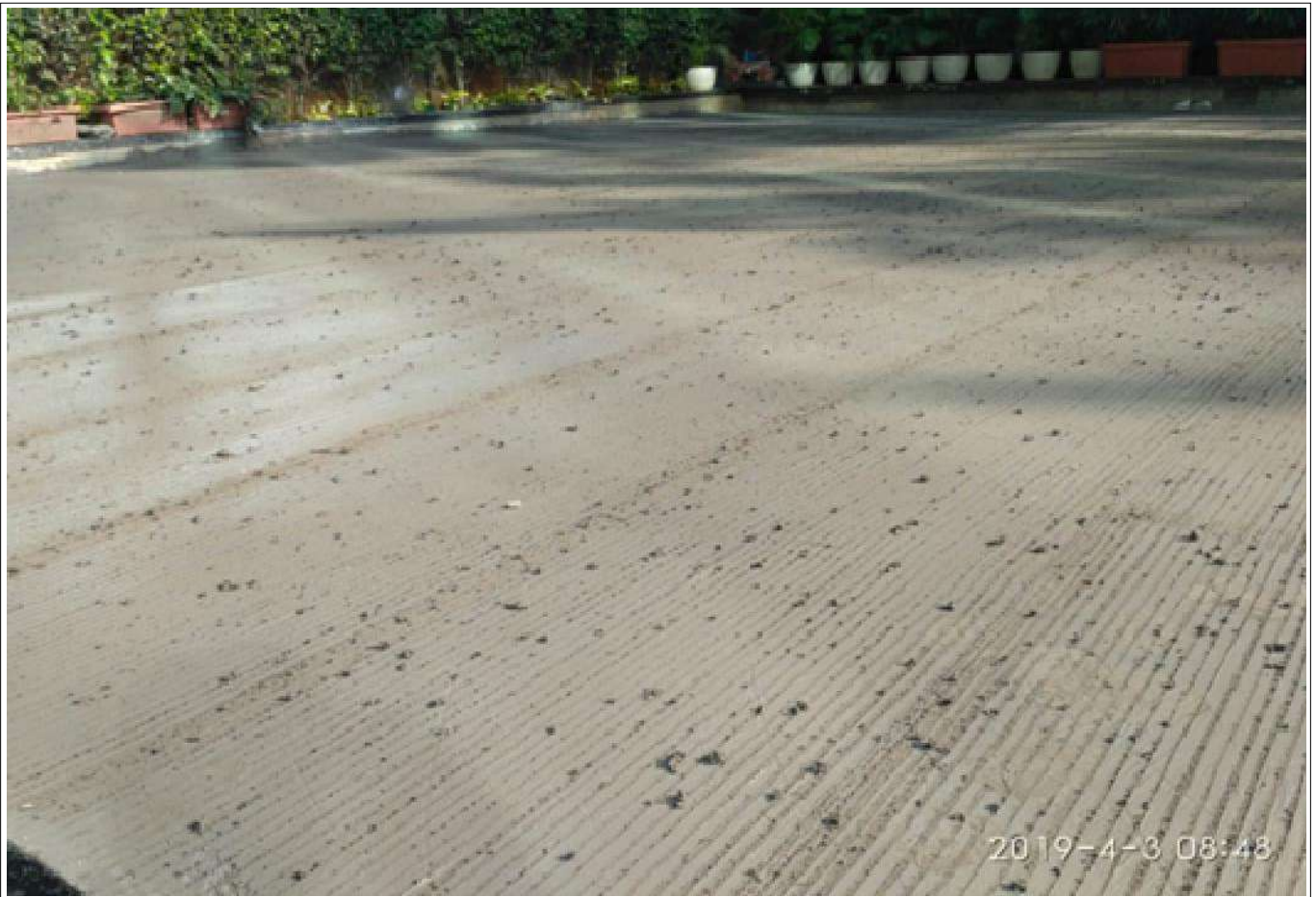
Finished parking area in less than week time
