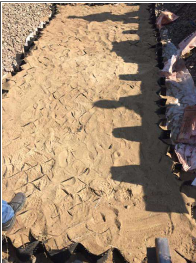
Filling of Techcell Geocell in Progress
