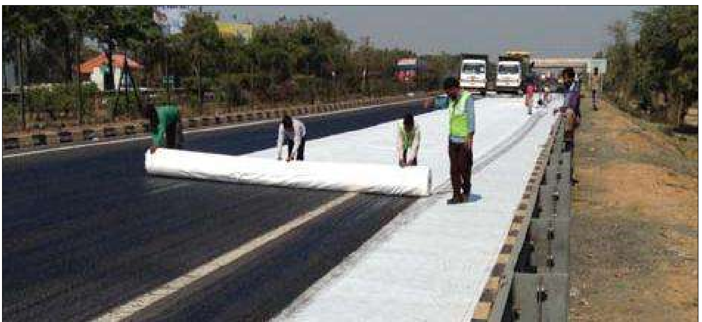
TechFab Paving Fabric - Installation
