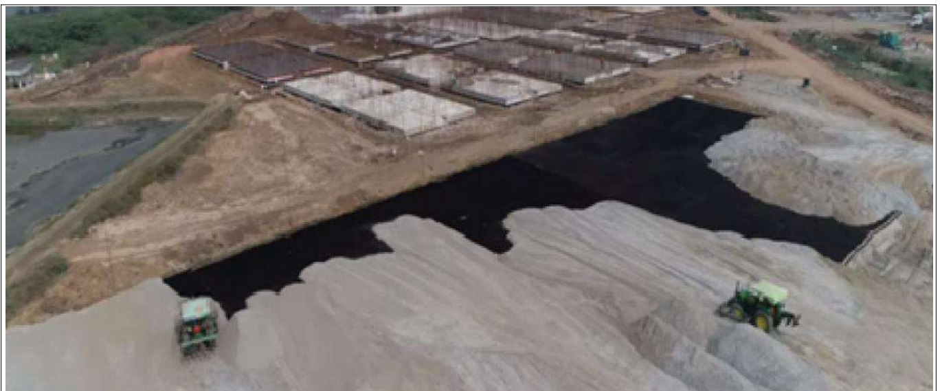
Aerial View: Techcell laid and Infilling in progress
