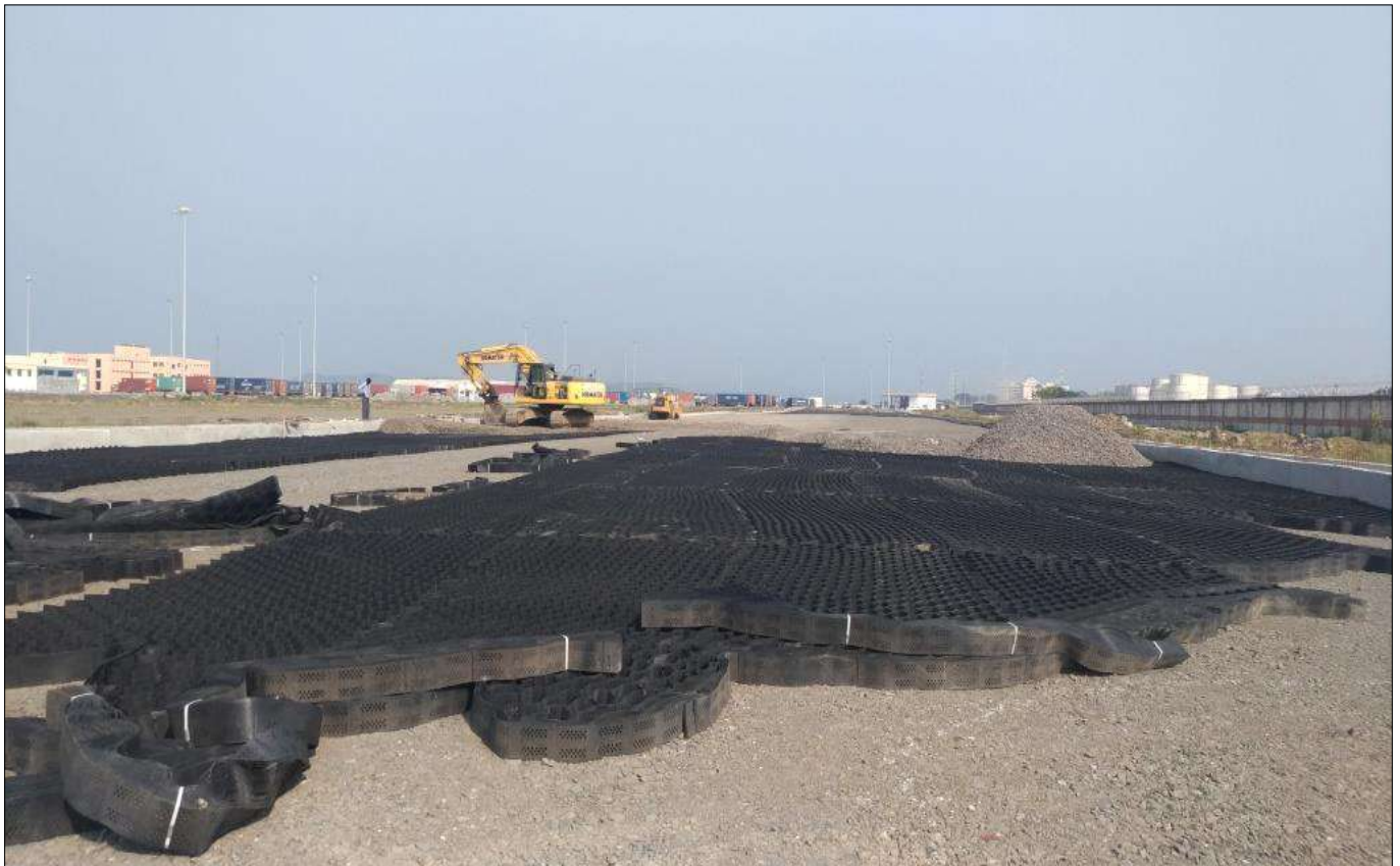
Laying of Techcell Geocell in progress
