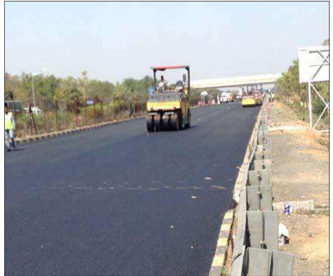
Compaction after placement of Overlay
