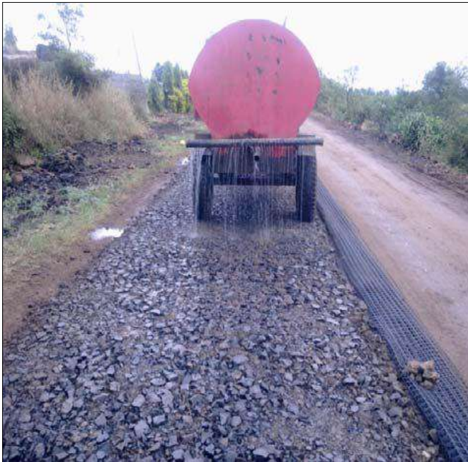
Watering on Compacted layer
