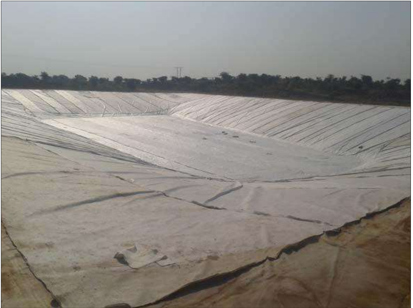
TechGeo Laying Completed at Landfill Site
