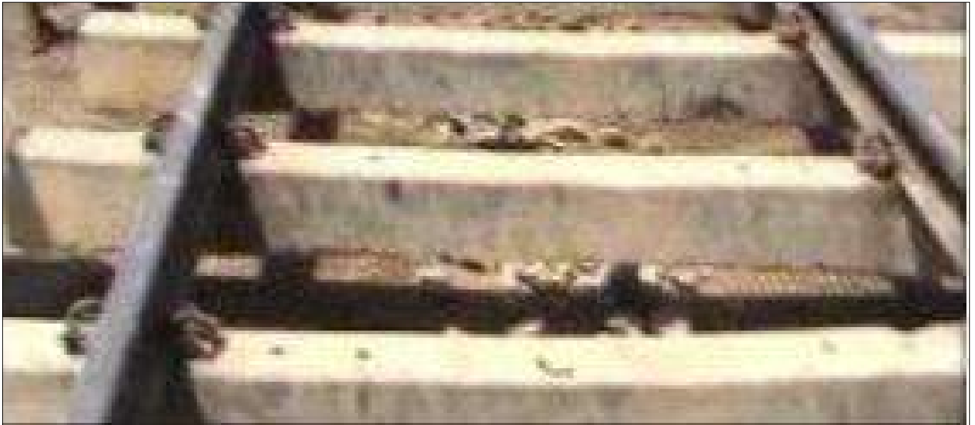
Photo 9 : Placing ballast over the geogrid
