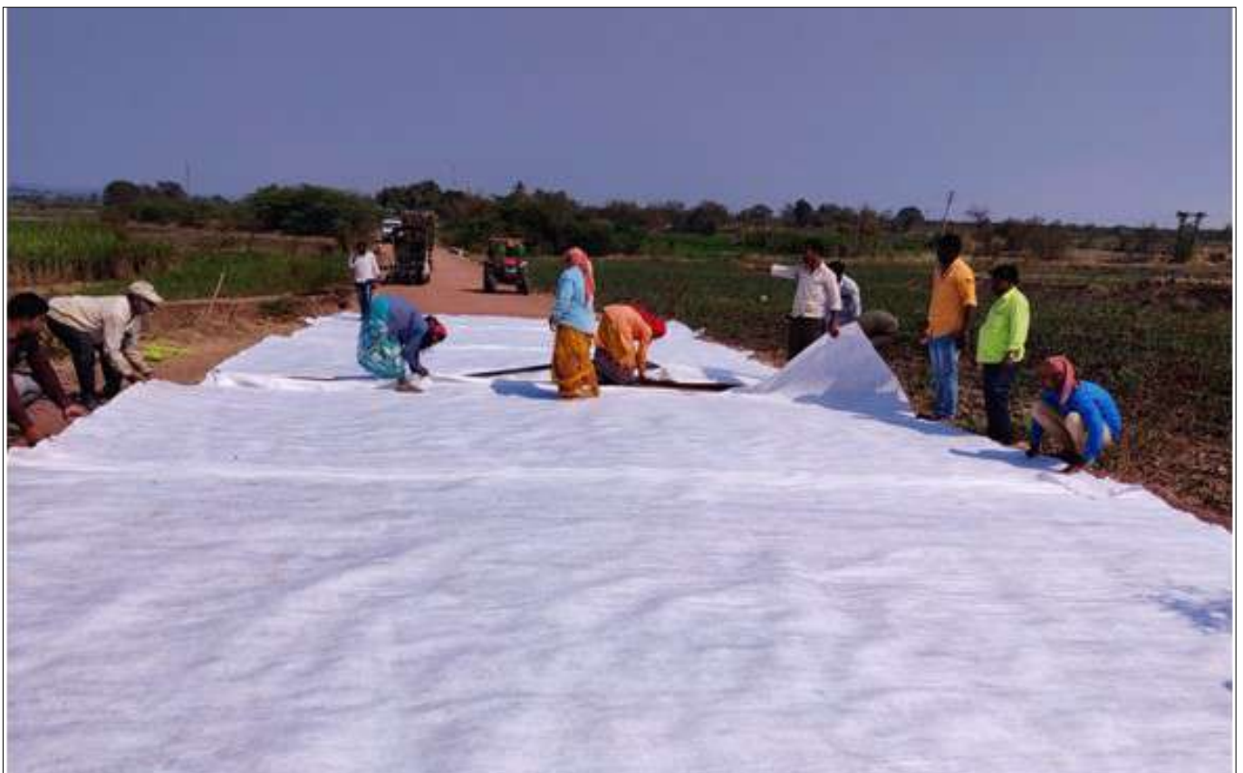
Laying of TechDrain Drainage Composite (With Necessary Overlaps) in progress
