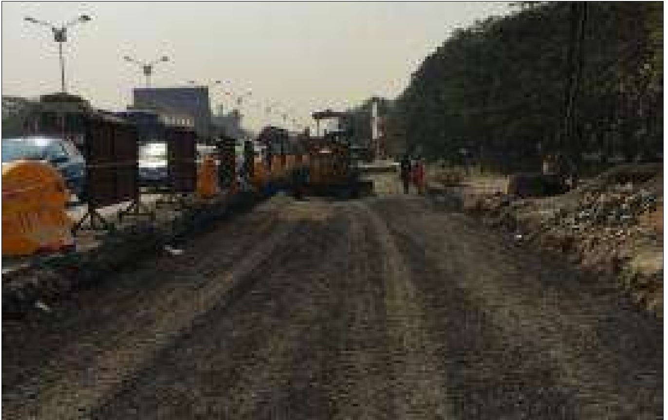
Compaction of Infill material in progress
