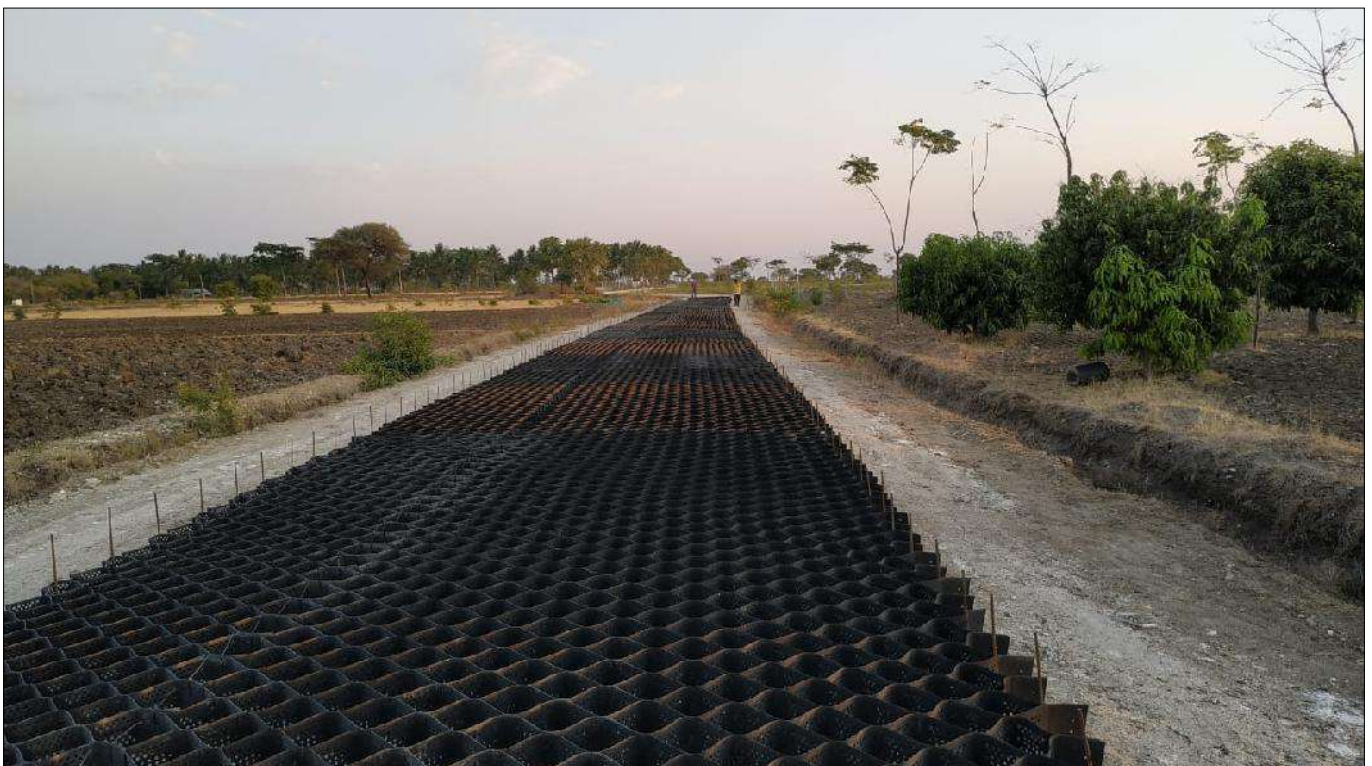
Spreading of TechCell Geocell above the subgrade
