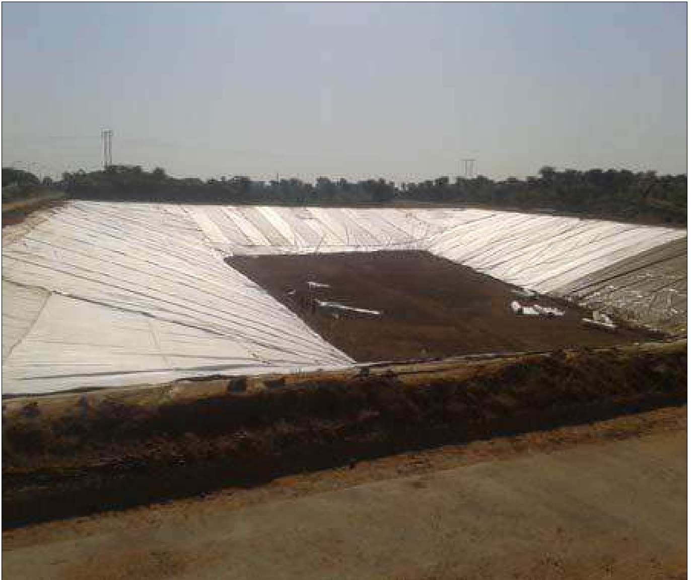
Top View – Himmatnagar Landfill Site
