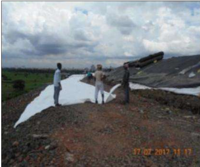
Laying of Geotextile
