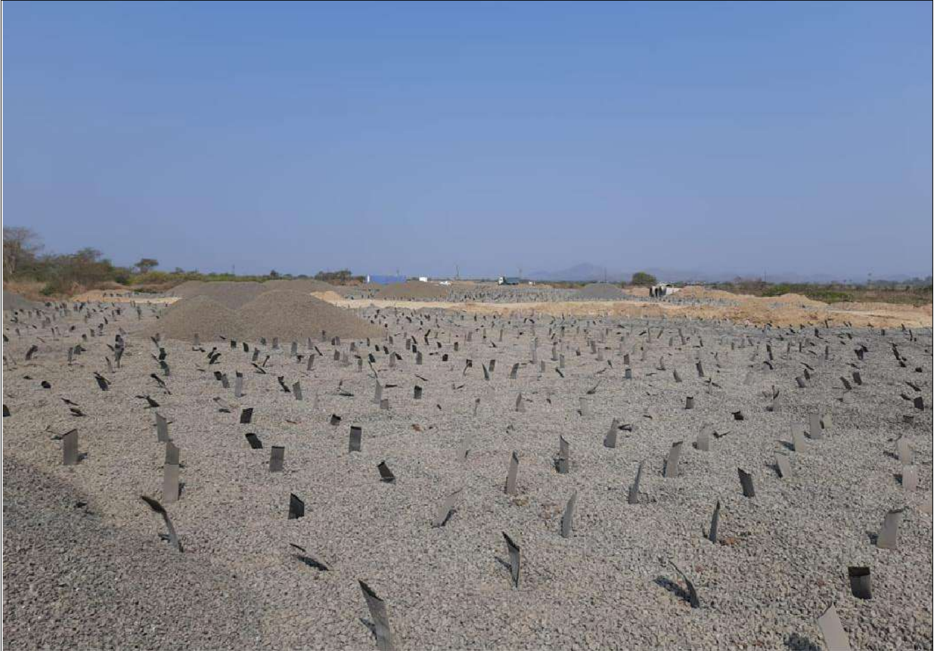
TechDrain PVD installed with preloading in progress
