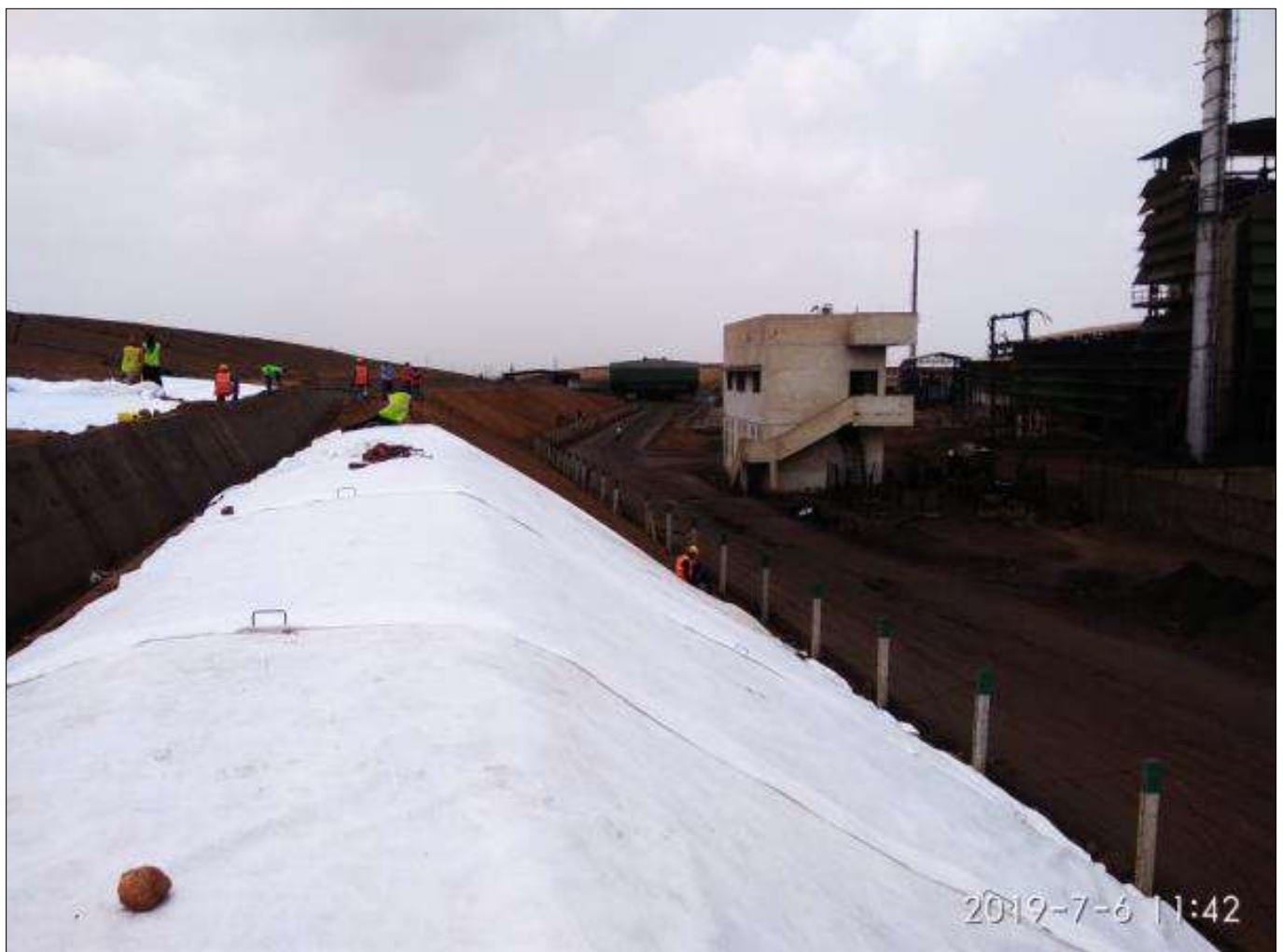
Laying of TechGeo Nonwoven geotextile
