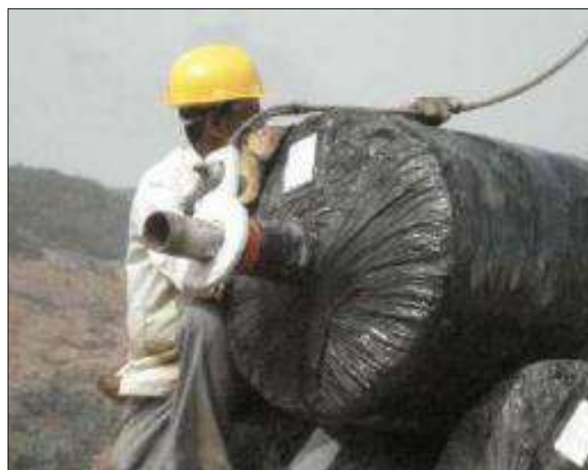
Figure 3 : Handling of Geosynthetic Rolls
