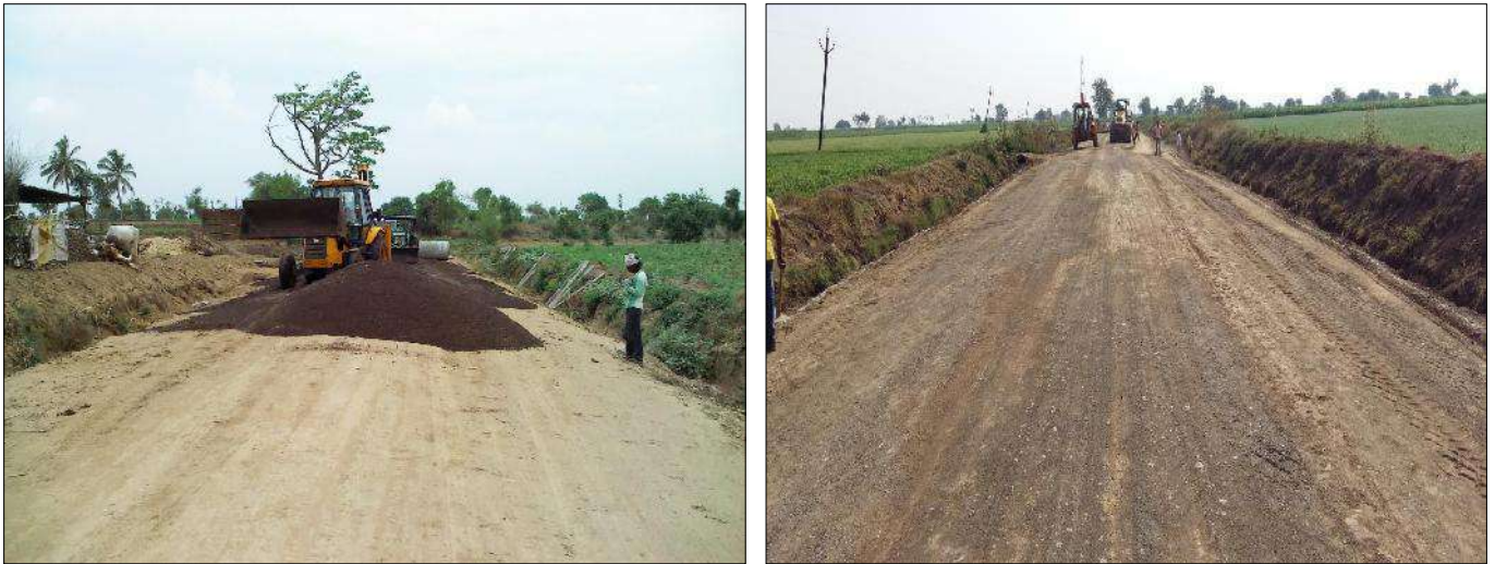
Photo 4 & 5 : Sand Layer laid on prepared surface
