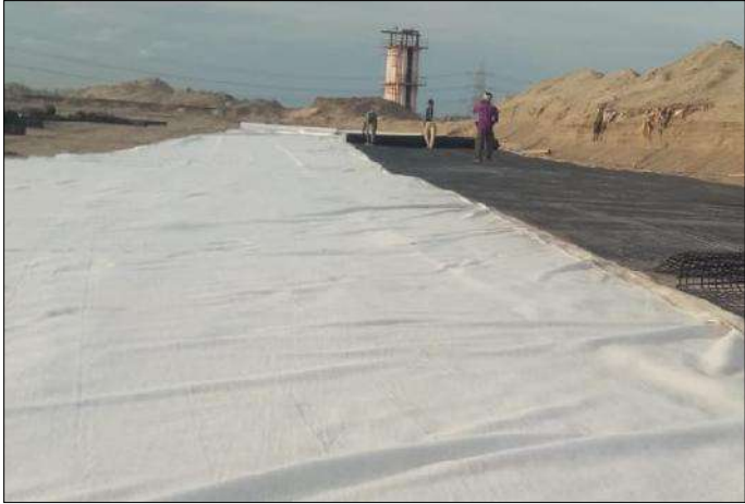
Photo 2 & 3 - Laying of Geotextile is in progress
