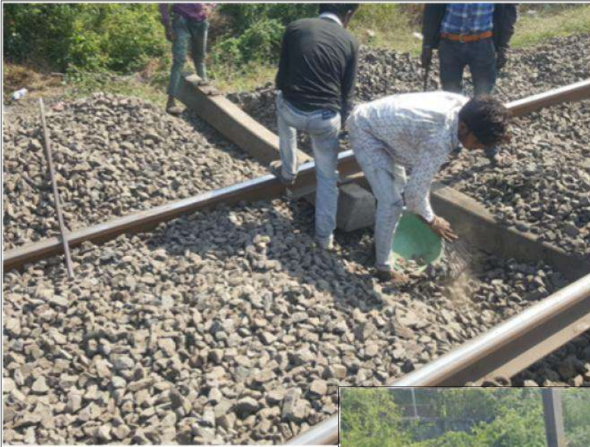
Placement of sleeper back to position
