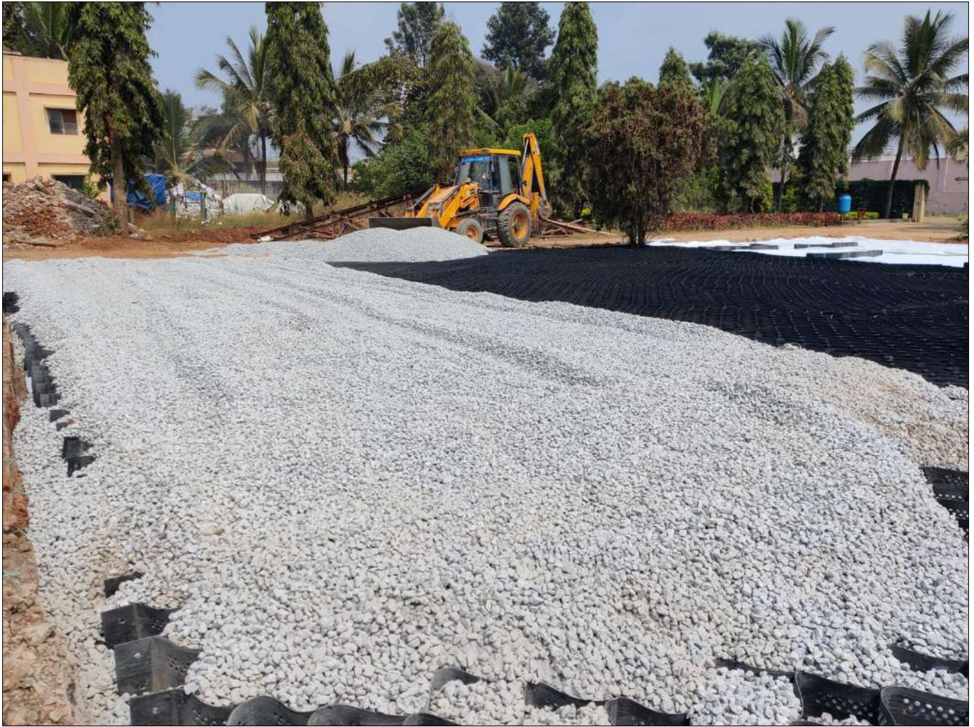
Photo 6 : Filling of Techcell Geocell with GSB
