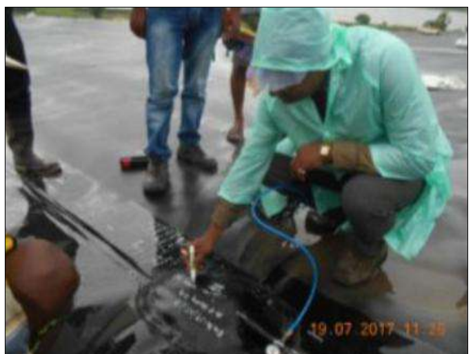
Laying of 1.5mm Both side Textured HDPE Liner
