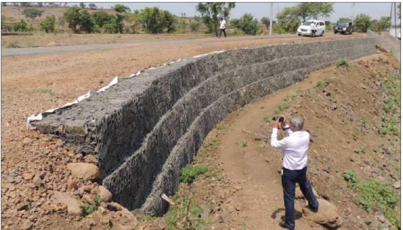
Gabion Retaining Wall
