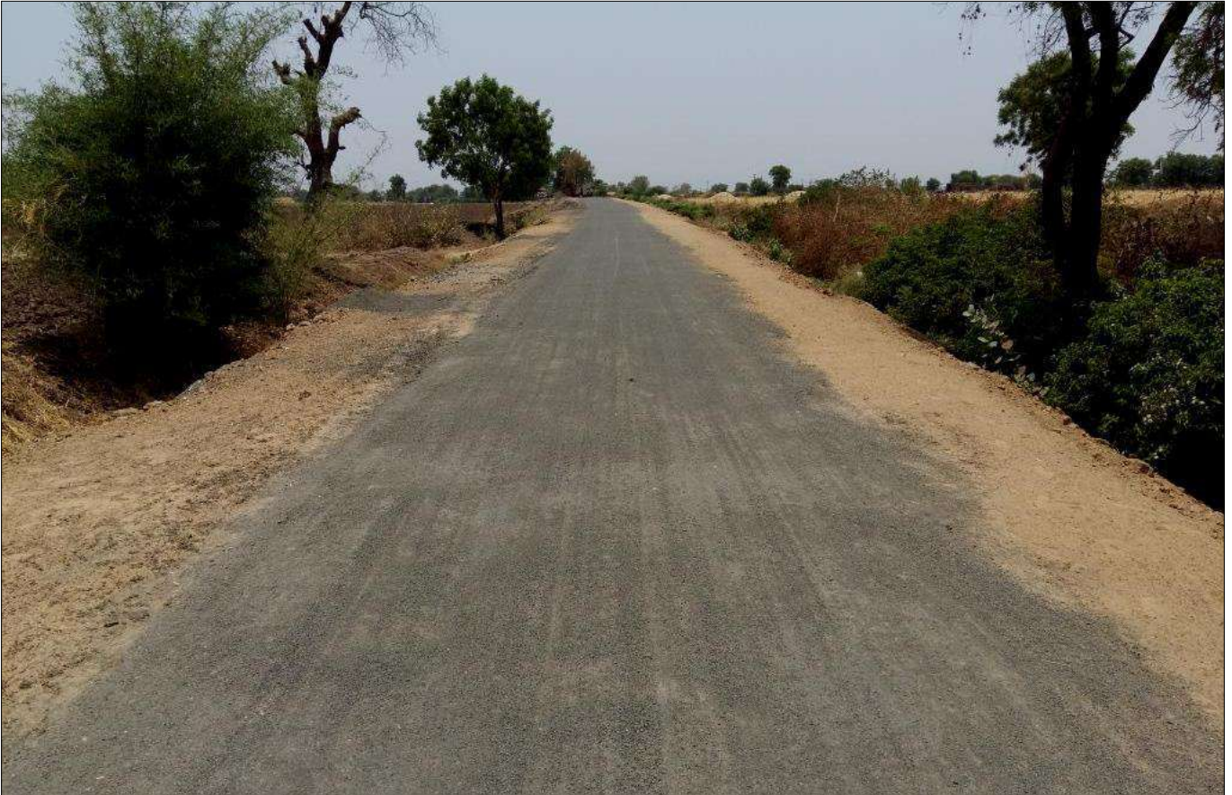
Photo 11 : Carpet in progress
