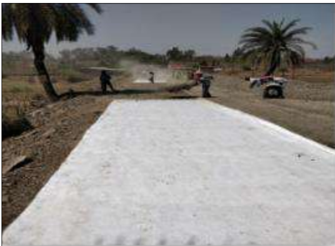
After laying geotextile, laying of 25mm bottom cushion of WMM
