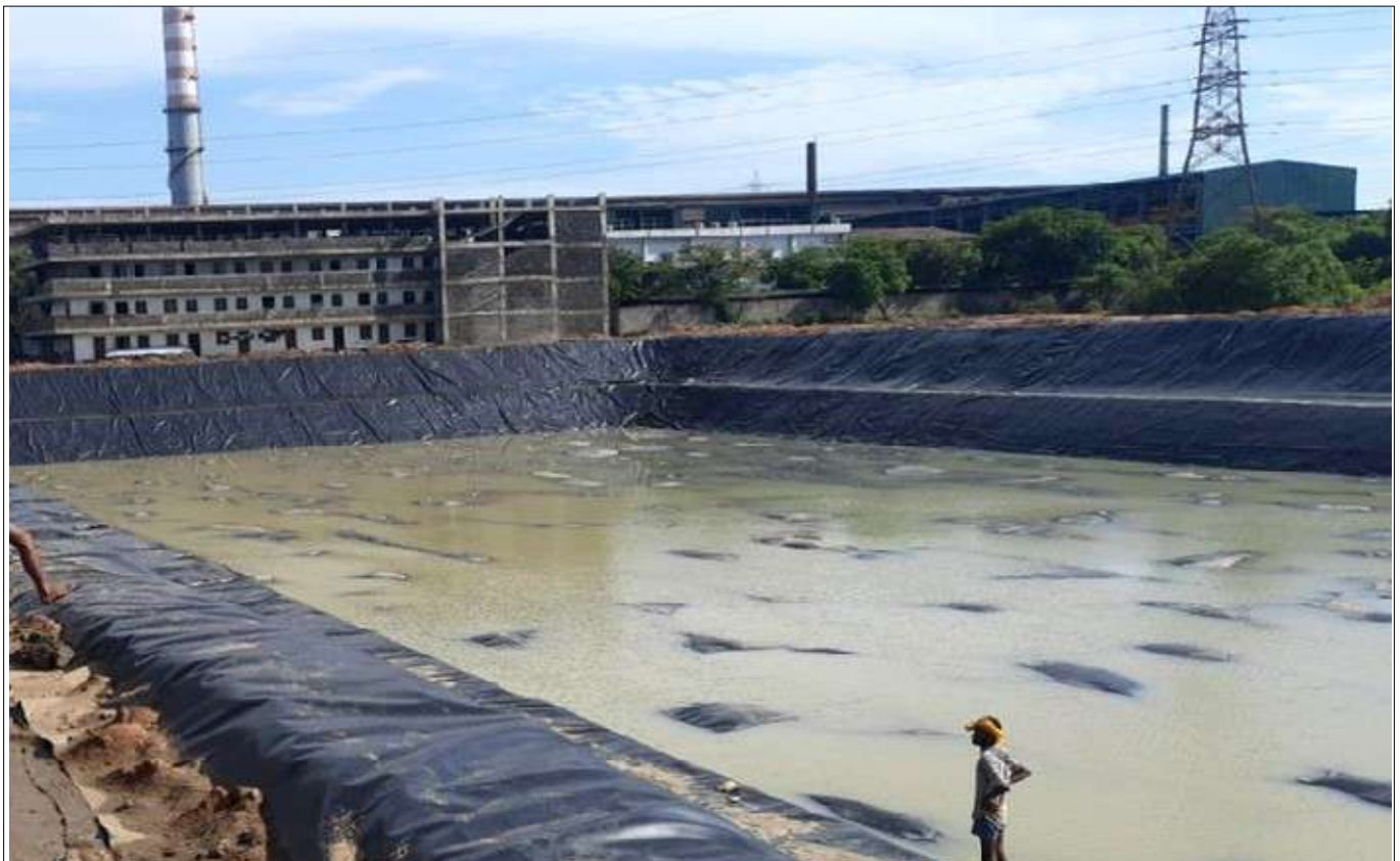
Photo 3 : Installed geomembrane layer on the surface of reservoir
