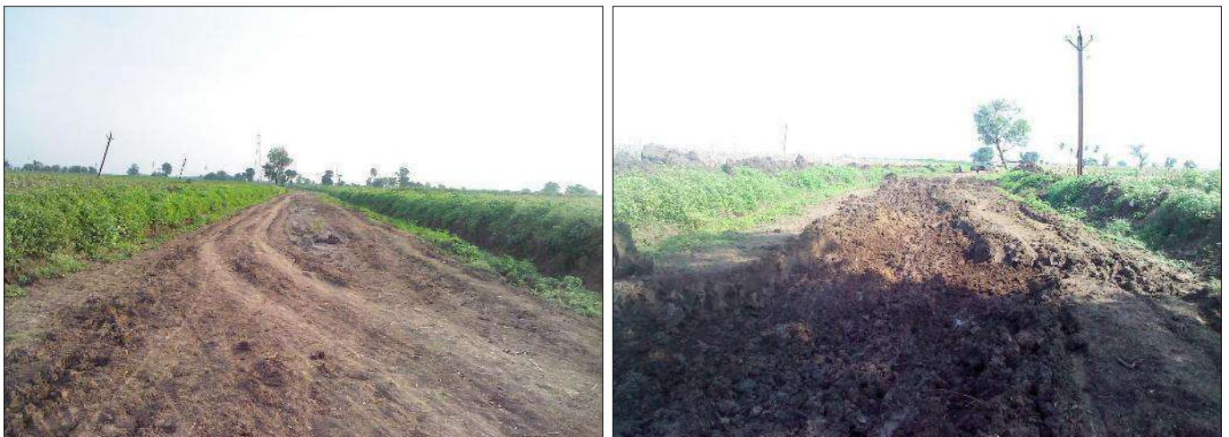
Photo 1 & 2 : Site Condition - Before Construction
