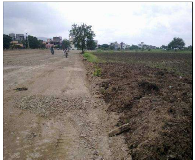
Subgrade Preparation (Stage-II)
