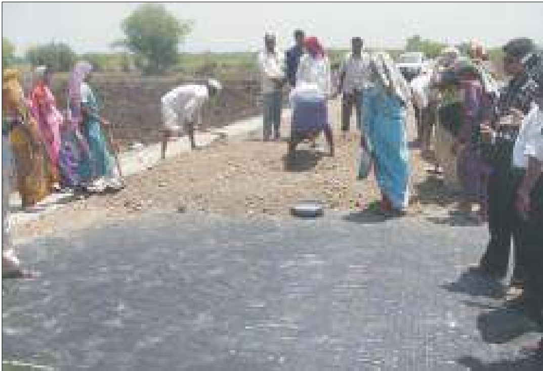
Levelling of soft murrum layer on top of the Geotextile
