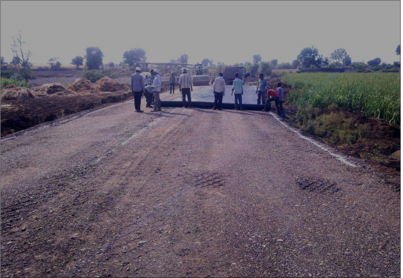
Photo 7 : Laying of woven Geotextile TFI - 5300 Type-1
