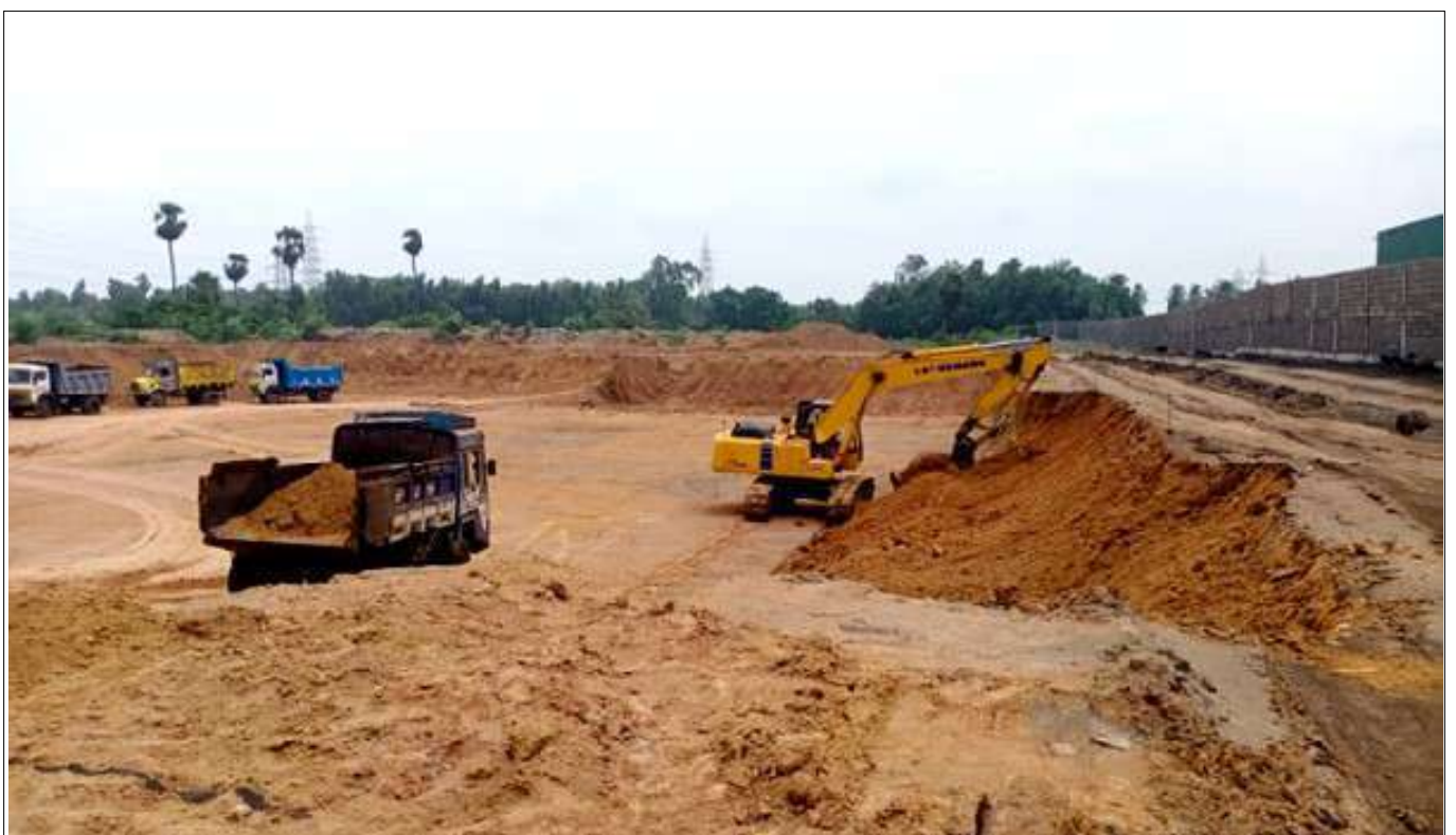
Photo 1 : Excavation to create the reservoir
