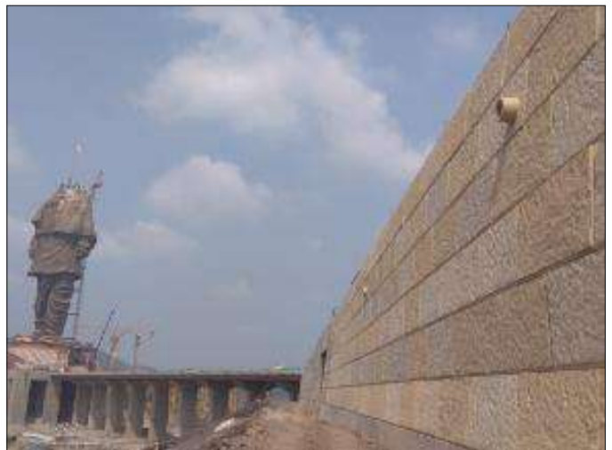
Finished view of RS Wall Panels
