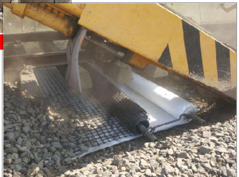
Laying of Techgrid PP and Techgeo non woven is in progress
