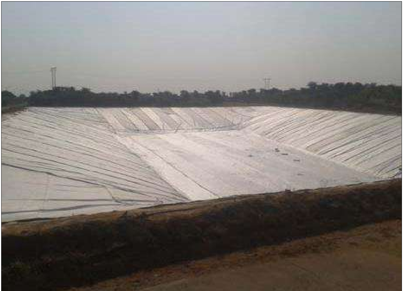
Top View – Himmatnagar Landfill Site
