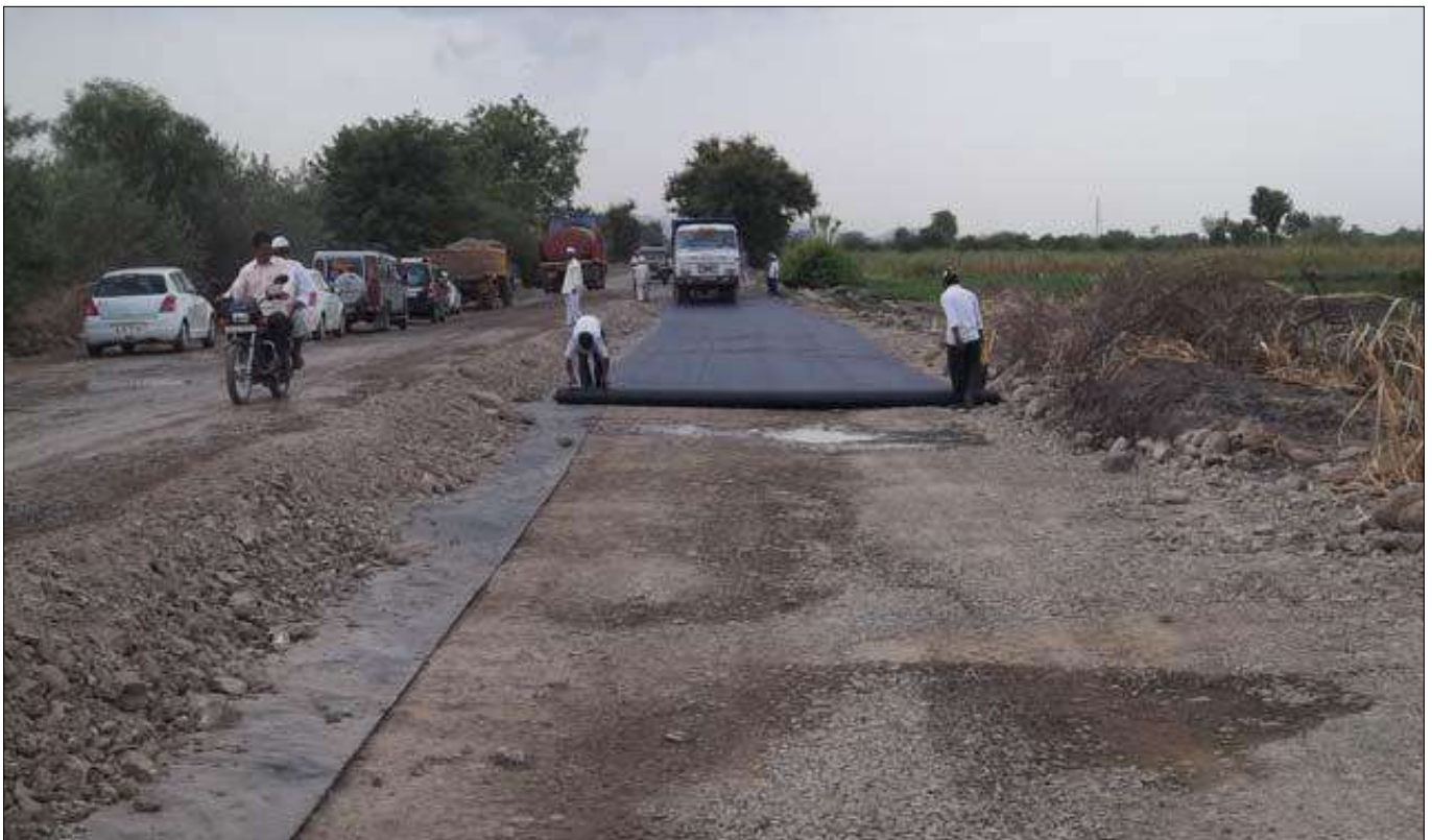
Unrolling TFI-5300 in 5m Widths
