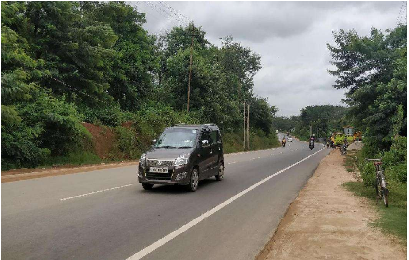
Fig 9 : Finished road stretch open to traffic since June 2018
