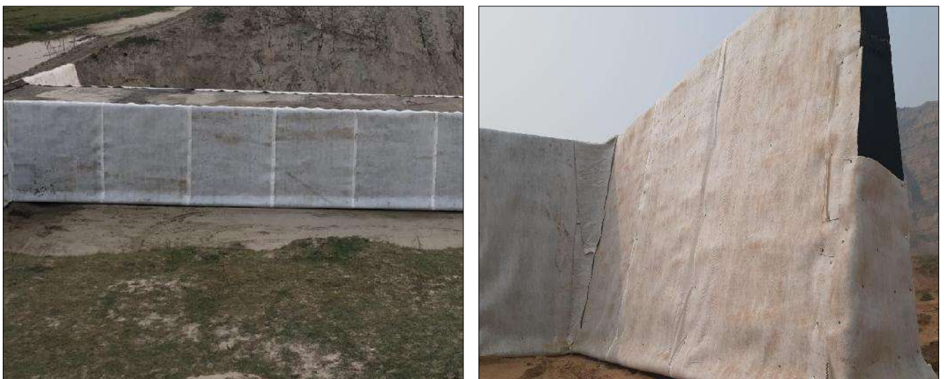
After Installation of TFI Drainage Geocomposite - TechDrains
