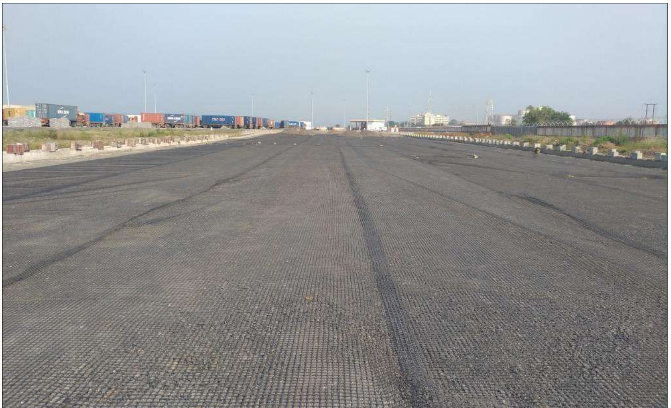
A layer of Techgrid PP Biaxial Geogrid was laid
