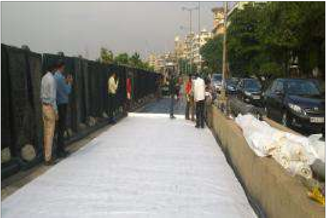
Installation of TechPave
