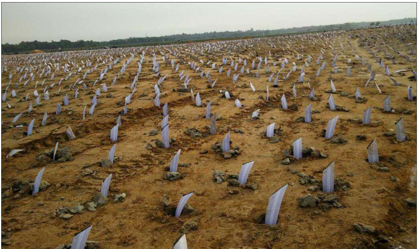
Installation of PVD
