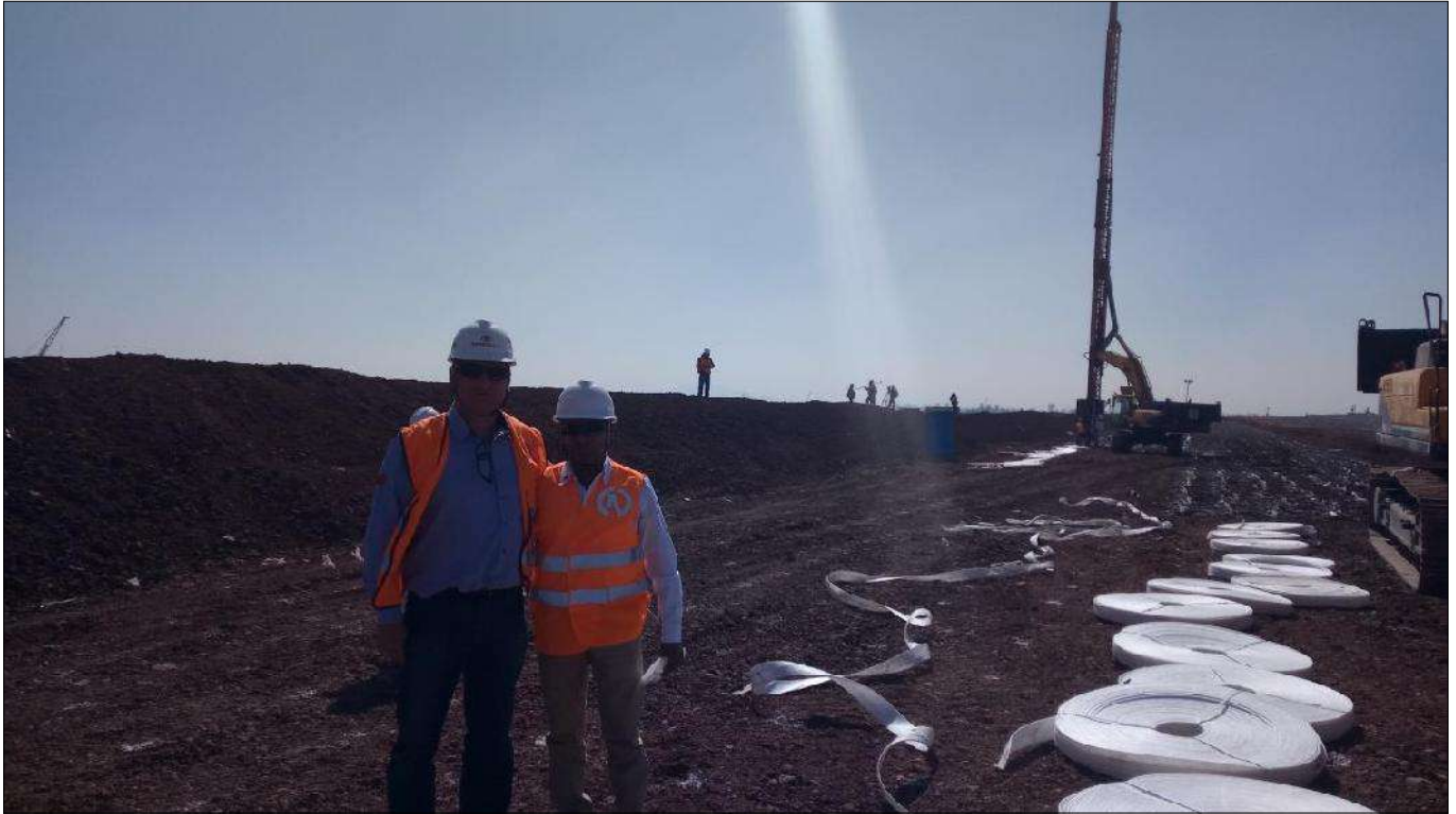
TechDrain PVD Installation in progress
