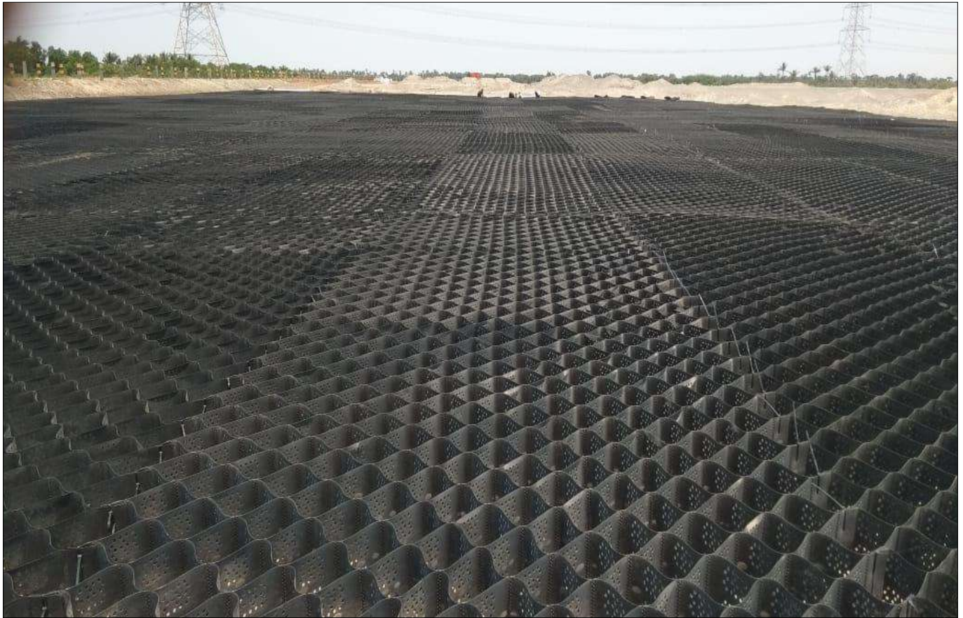
Photo 7 - Spreading of Techcell Geocell is in progress
