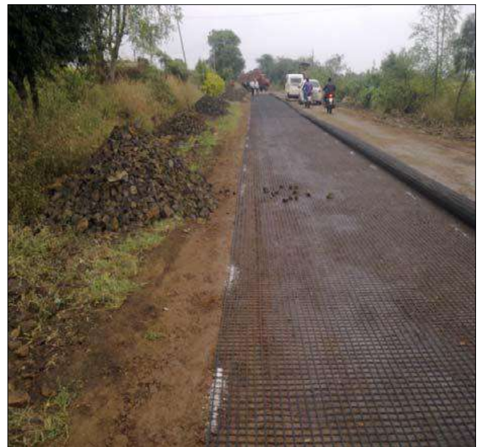
Laying of TGB-40
