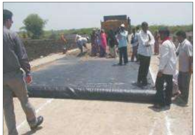
Geotextile being unrolled
