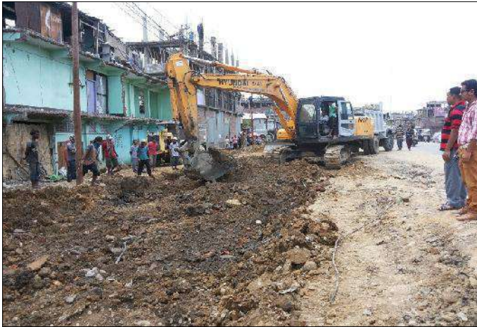
Preparation of sub-base for Road Expansion
