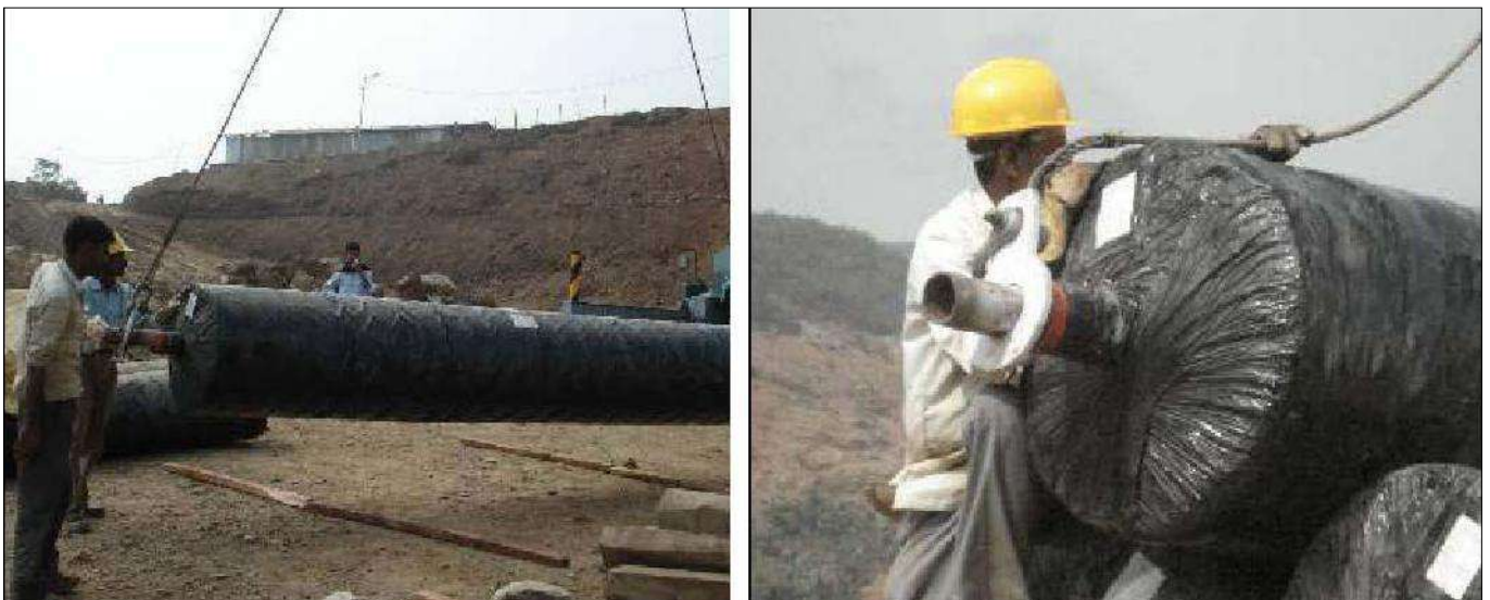
Handling of Geosynthetic Rolls
