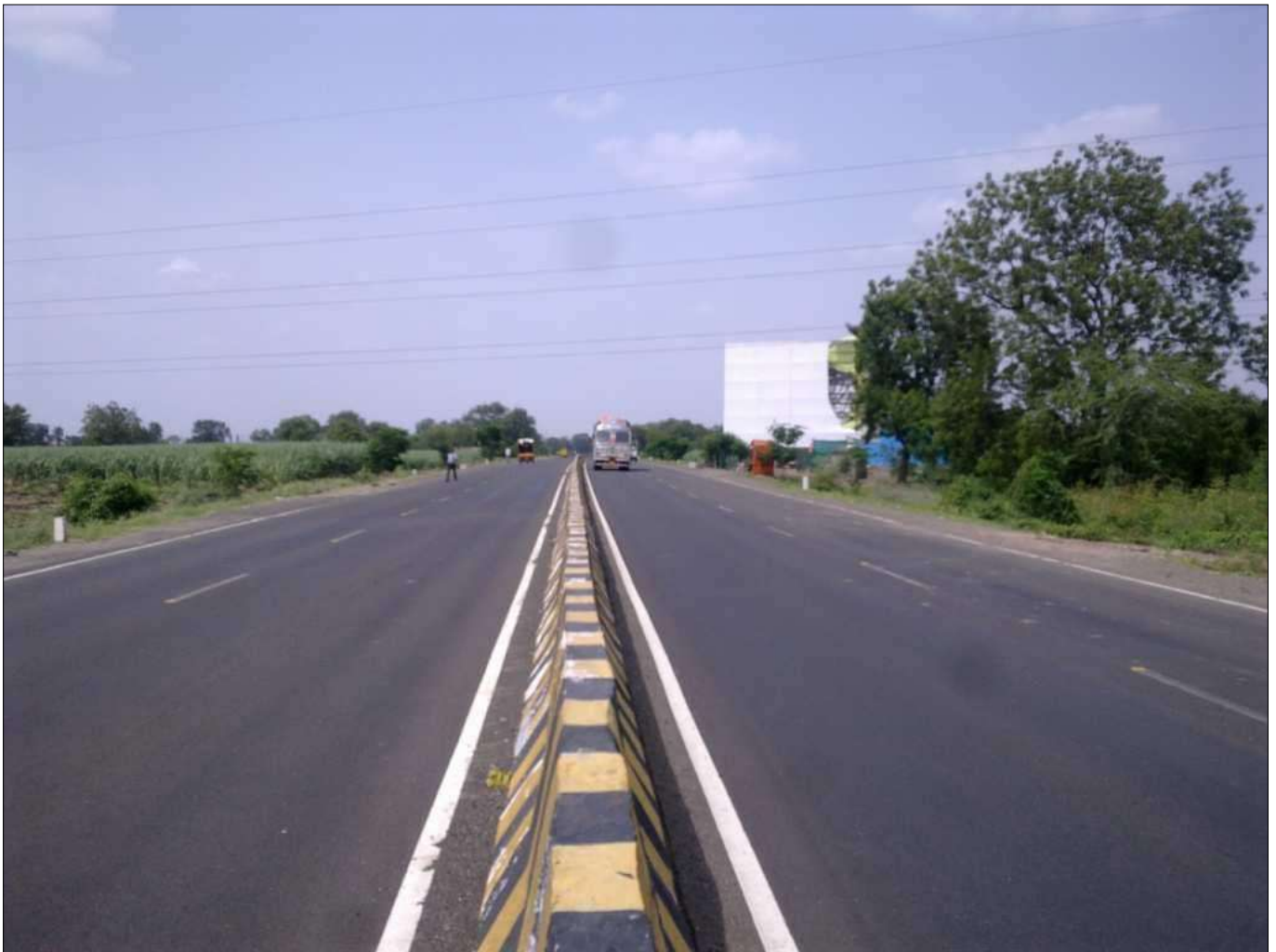
After Completion of Project
