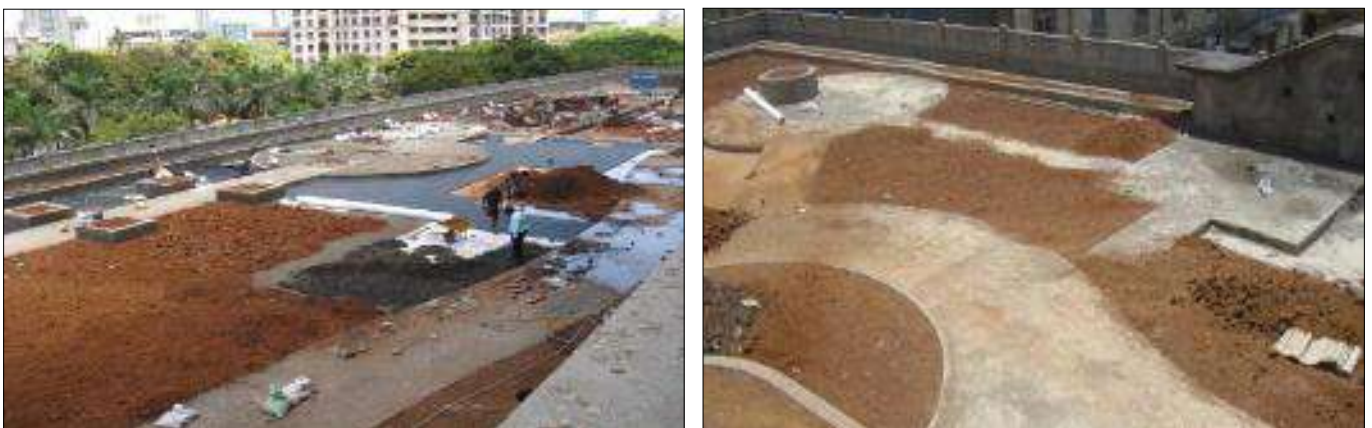
Fig 7 & 8 : Laying of Soil Planting Mixture
