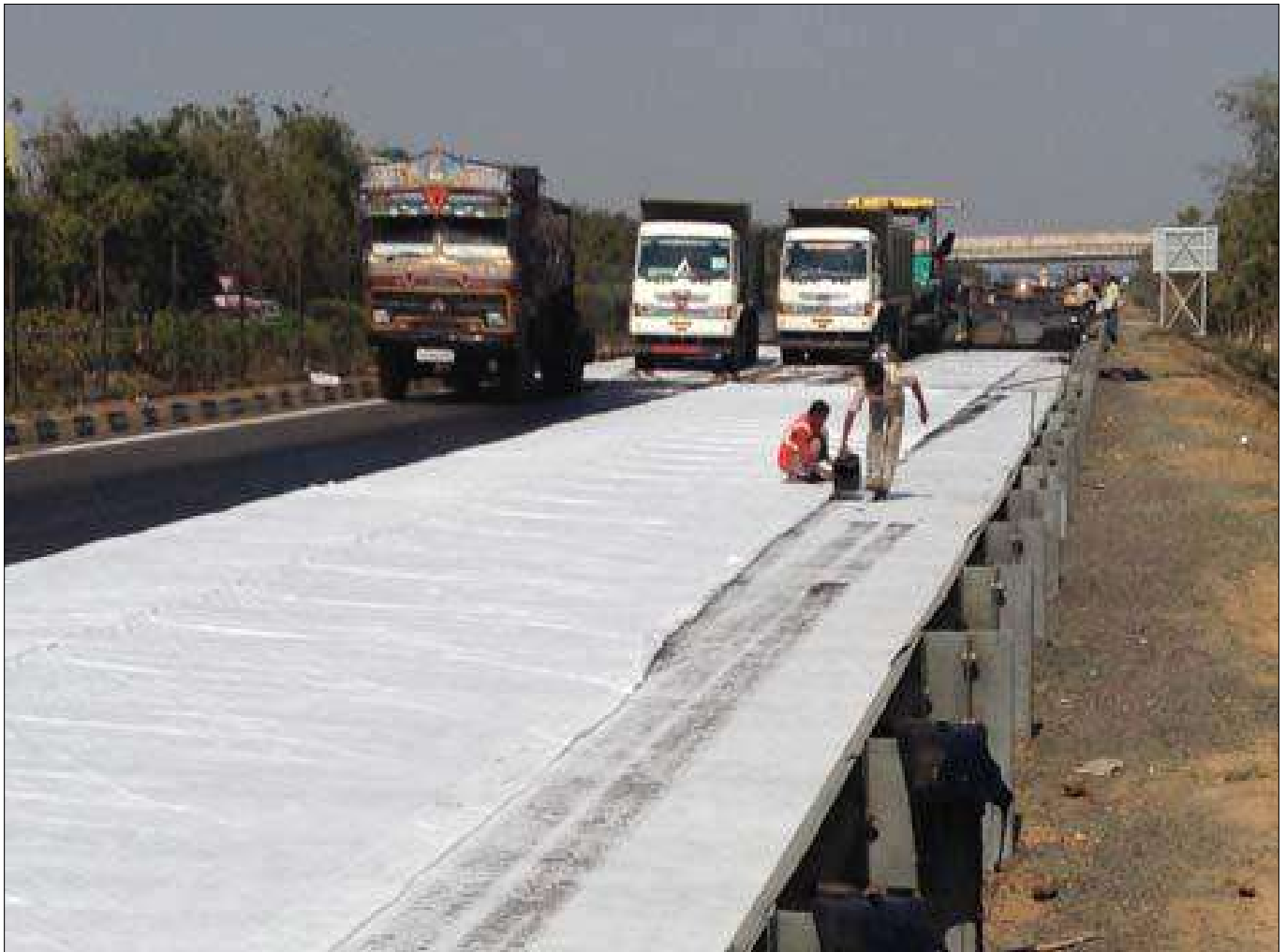
TechFab Paving Fabric - Installation
