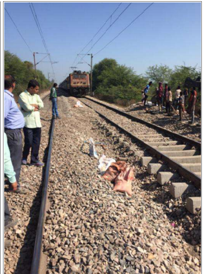
After laying of track in completed stretch
