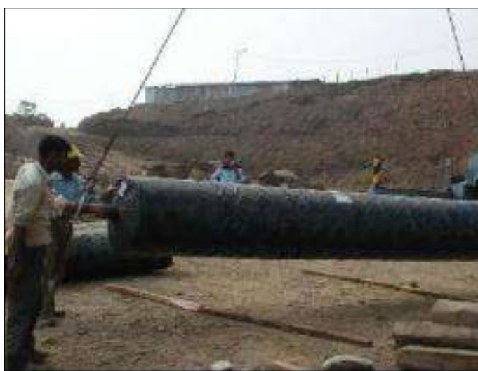
Figure 3 : Handling of Geosynthetic Rolls
