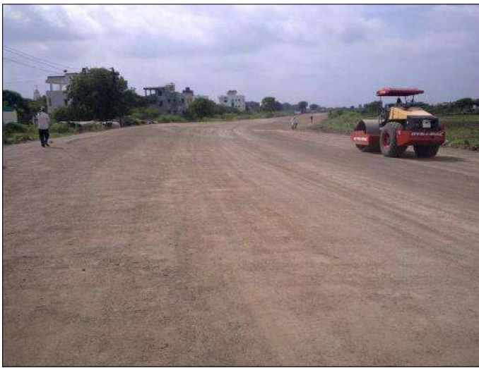
Subgrade Stabilization
