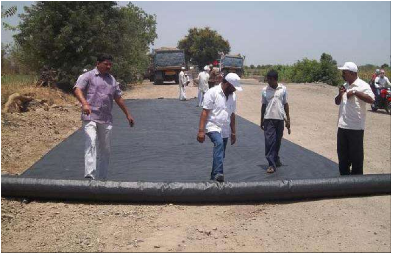
Laying of TFI-5300 at Subgrade
