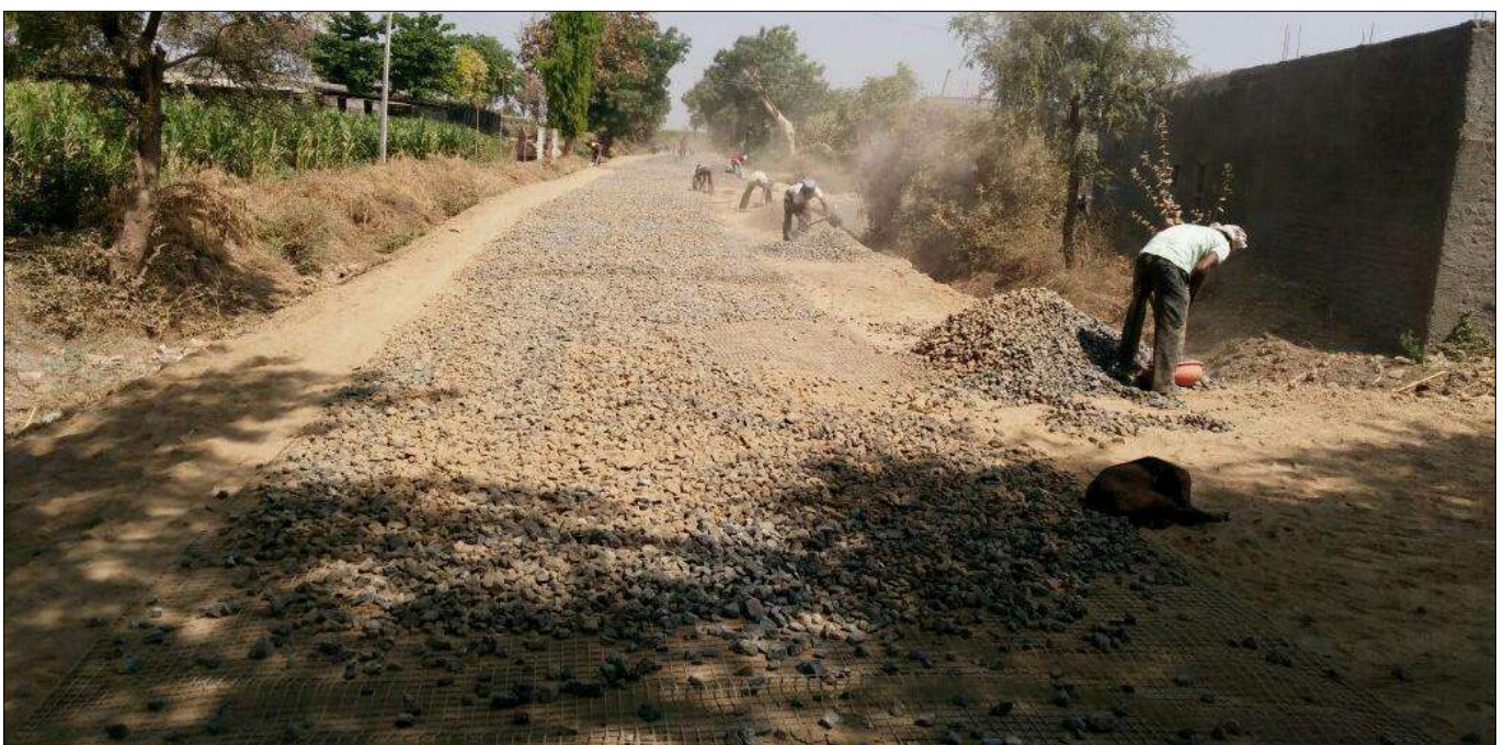
Photo 10 : Placing of MPM over TechGrid Geogrid TGB-40
