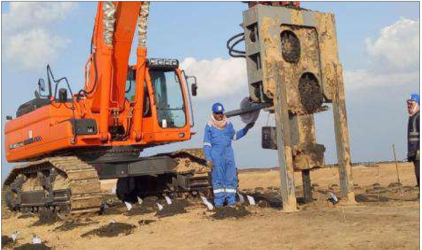
TechDrain PVD installation is in progress
