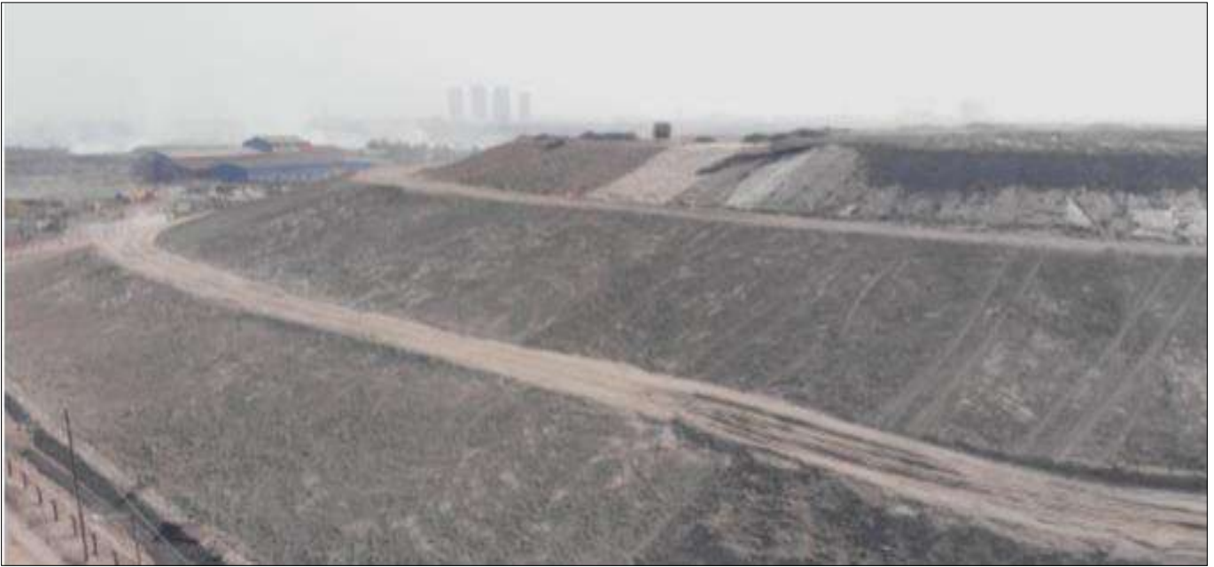
Laying of 500mm thick Non-contaminated Soil
