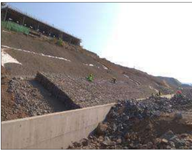
TechFab Metal Gabion Mattress laying in progress
