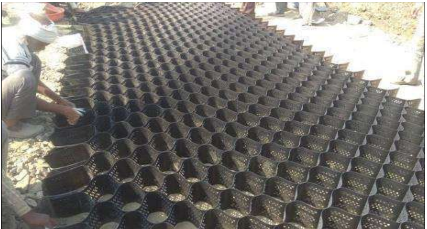
Techcell laying in progress
