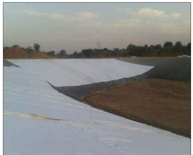
TechGeo laid over the Side Slopes of Landfill
