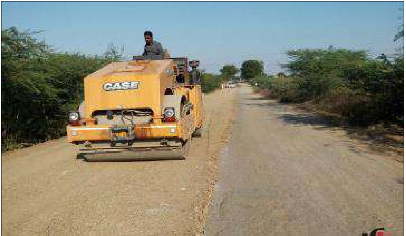
Sub-Grade compaction in progress
