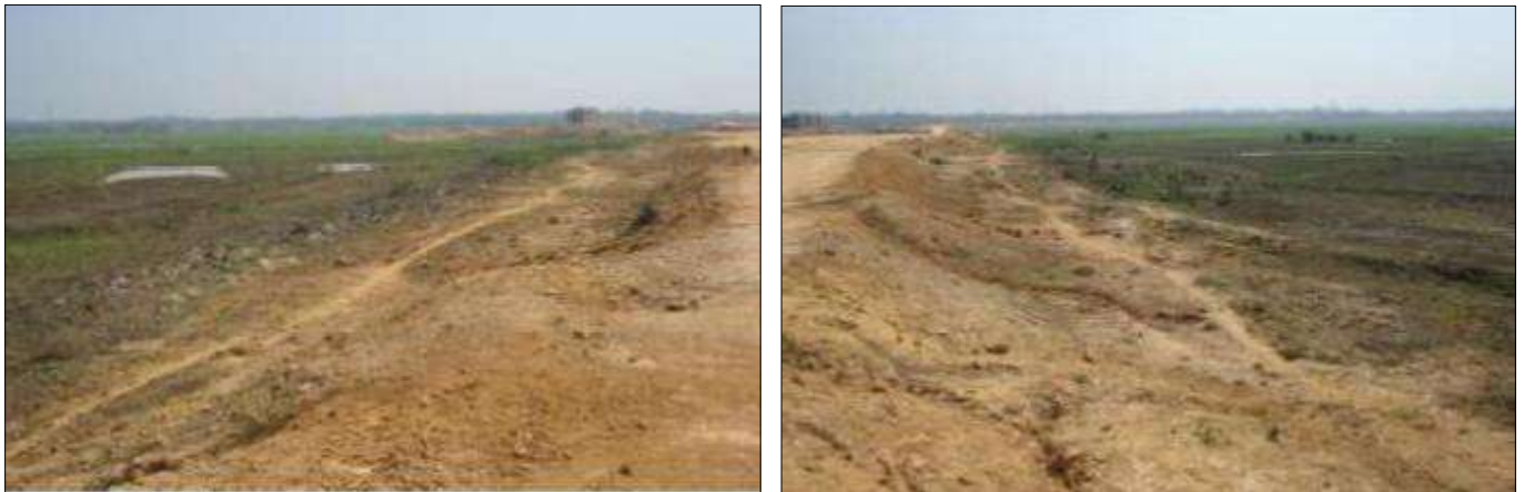
Figure 1 : Left and Right side of the Embankment
