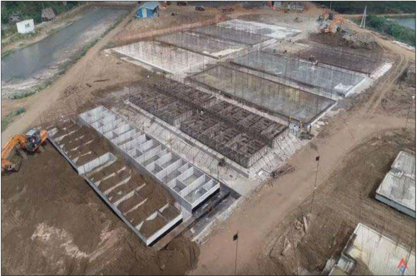
Aerial View: Raft Foundation completed
