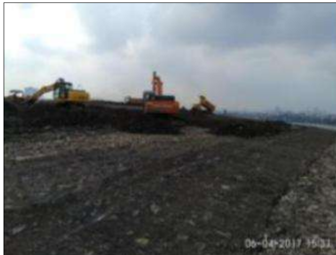
Laying of Geogrid
