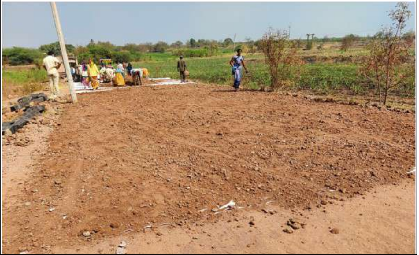
Murrum Cushion Layer Laid on Drainage Composite (To Prevent Puncture)
