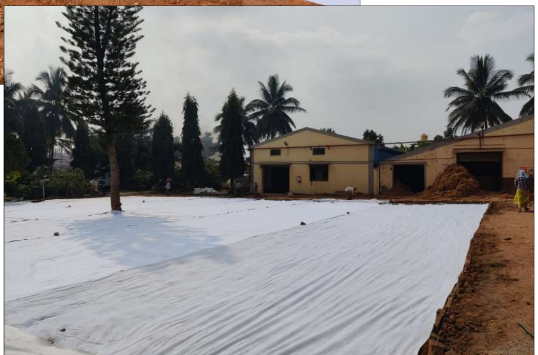
Photo 2 & 3 : Installation of TechGeo Nonwoven Geotextile
