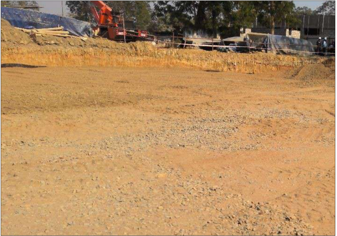
Photo 7 : Surface after completion of filling over the geogrid
