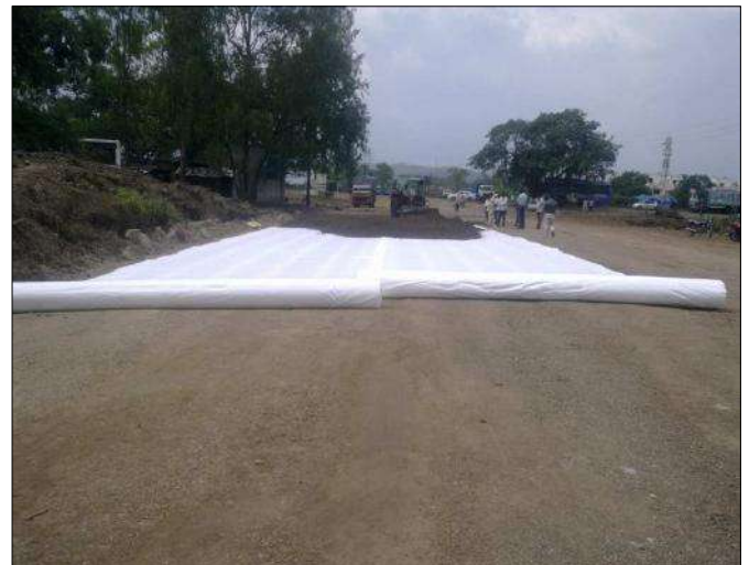
Placing of WMM Layer over PR-25
