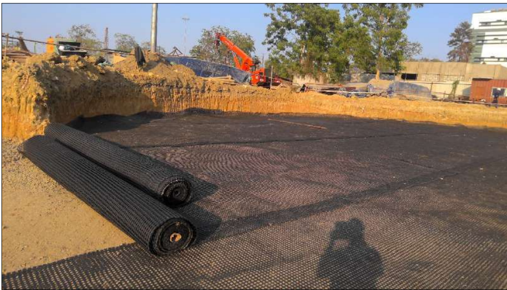
Photo 2 : Laying of Techgrid Biaxial Geogrid (TGB 200)
