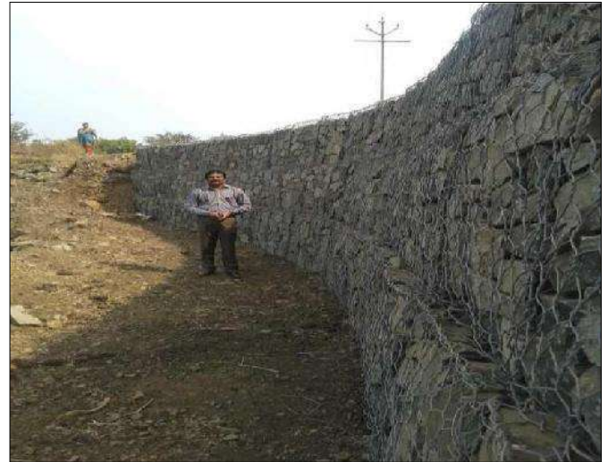
Construction of Gabion Wall
