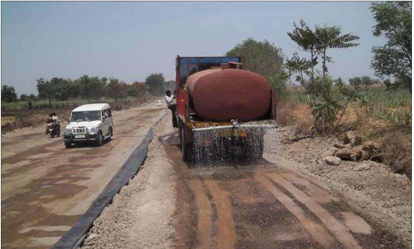
Sprinkling of Water & Compaction of Pavement
