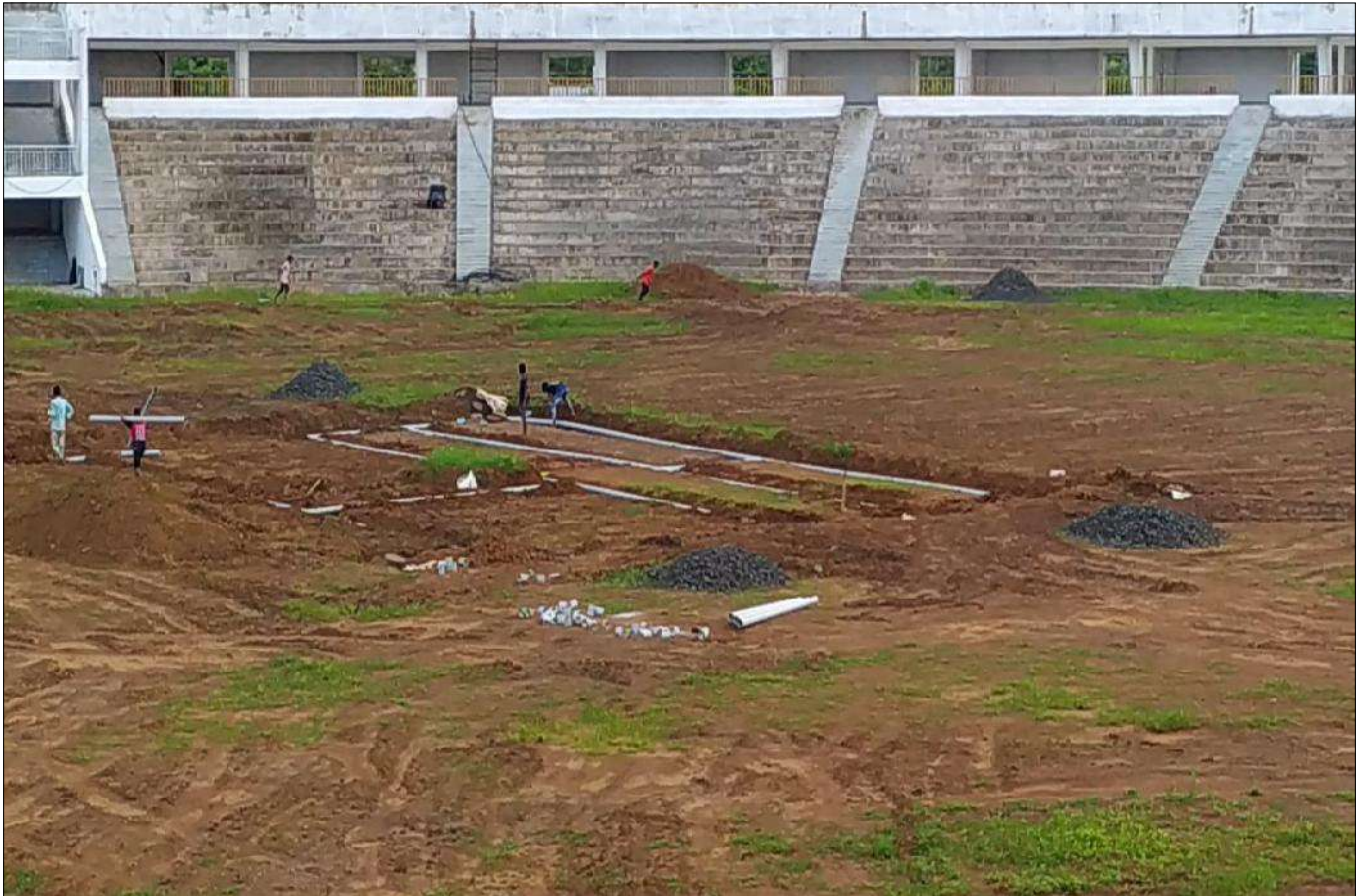
Drainage composite installation and Pipe drain laid
