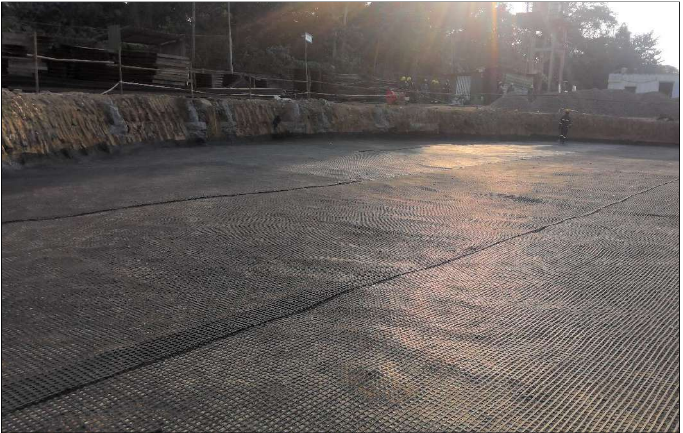
Photo 4 : After laying of geogrid layer
