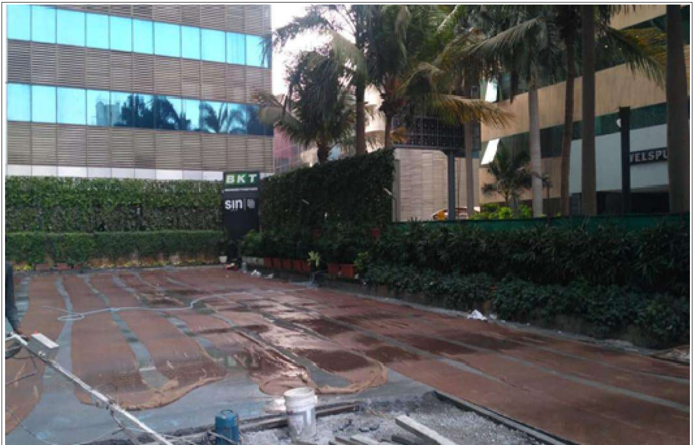
Concrete flooring above Techcell Geocell
