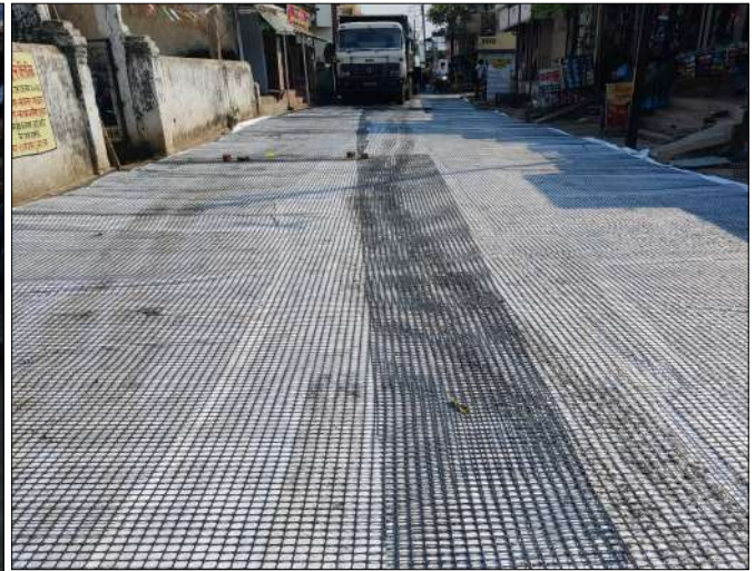
Photo 2 : Laying of PP Biaxial Geogrid over TechPave
