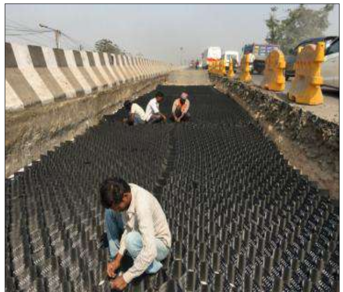
Techcell geocell tying in progress
