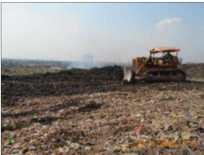
Levelling of waste by Dozer
