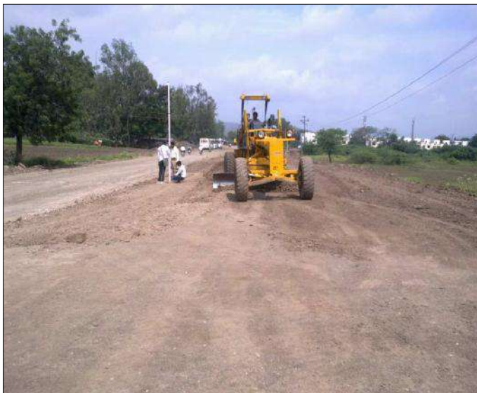
Subgrade Preparation (Stage-I)
