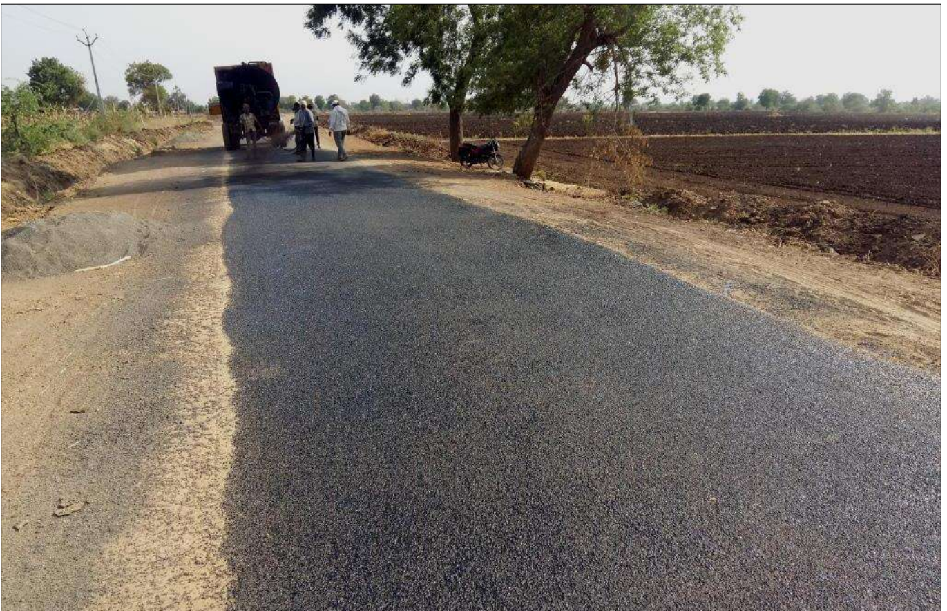
Photo 12 : Laying of Seal coat
