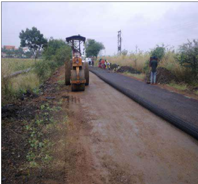
Compaction of Subgrade
