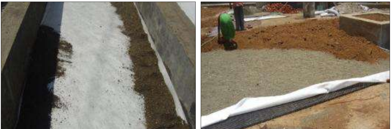
Fig 5 & 6 : Laying of Coarse Sweet Sand
