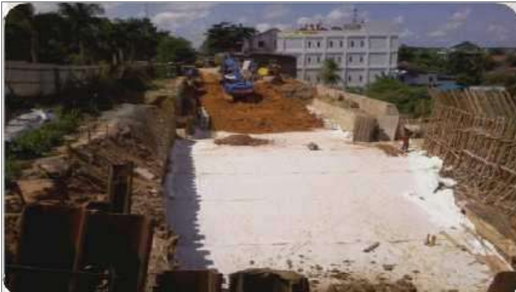
Installation of TGC Geotextile
