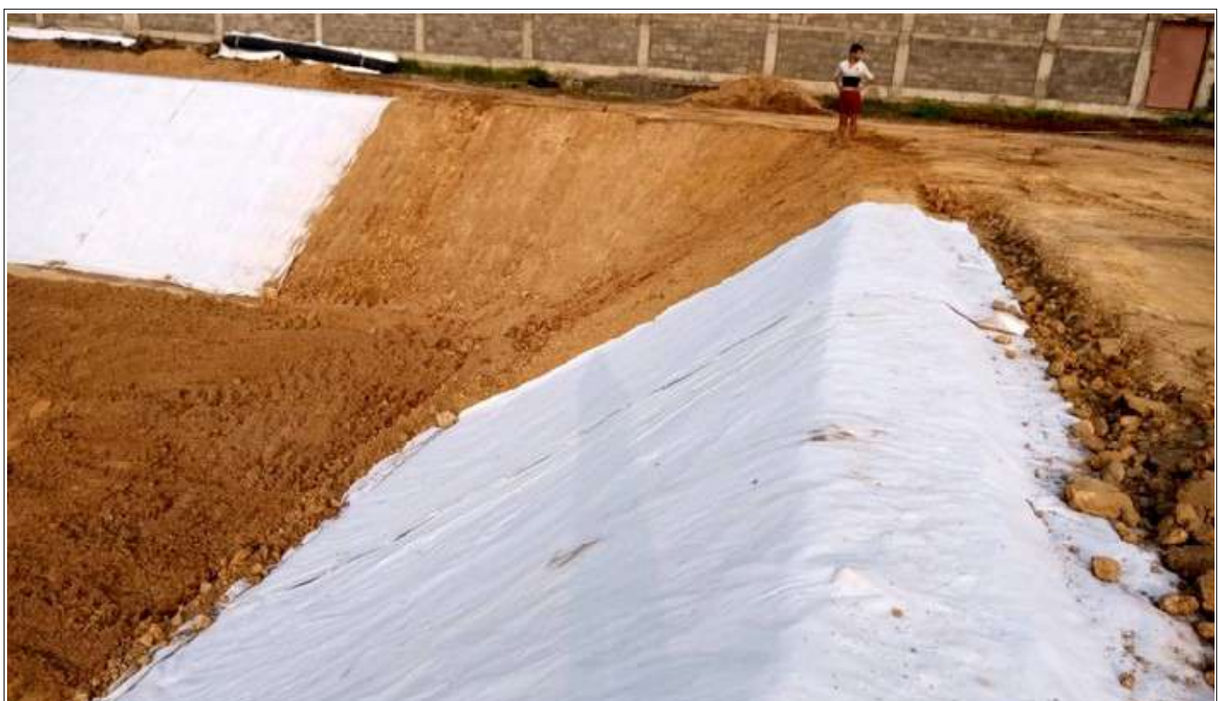
Photo 2 : First later of geotextile laid over the prepared surface
