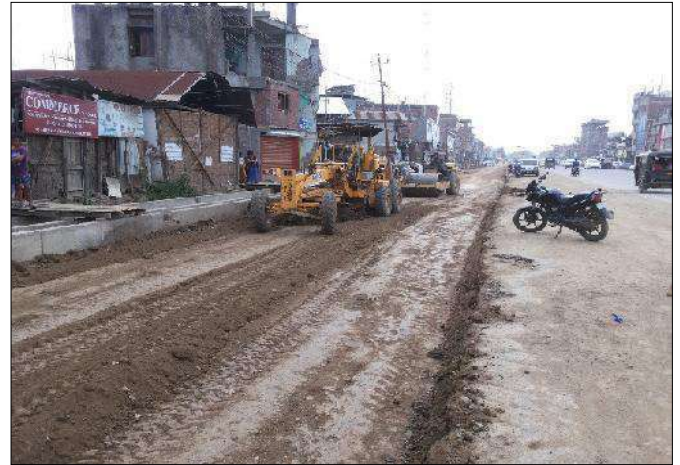
Preparation of subgrade for Road Expansion
