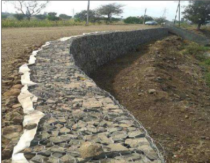
Gabion Retaining Wall
