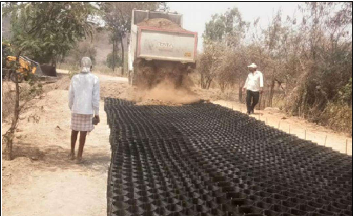
Filling and Compaction of granular material into the TechCell Geocell
