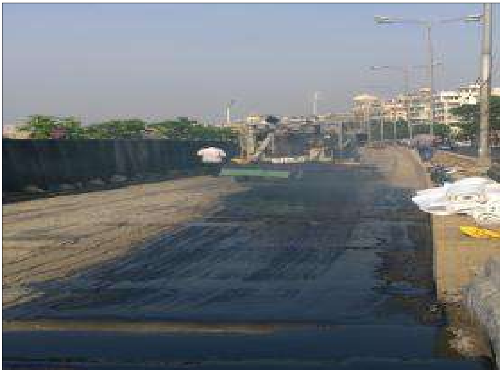
Spraying of Bitumen – Before TechPave
