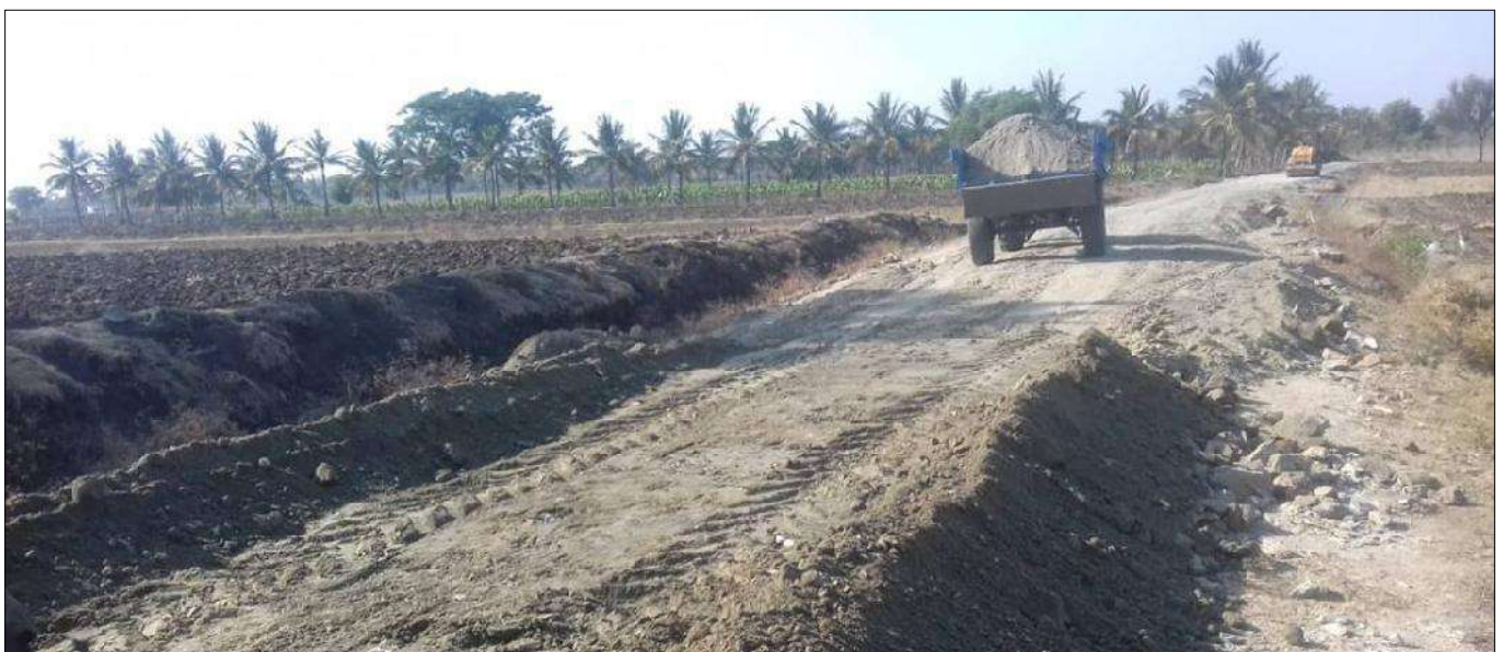
After filling and Compaction of granular material into the TechCell Geocell
