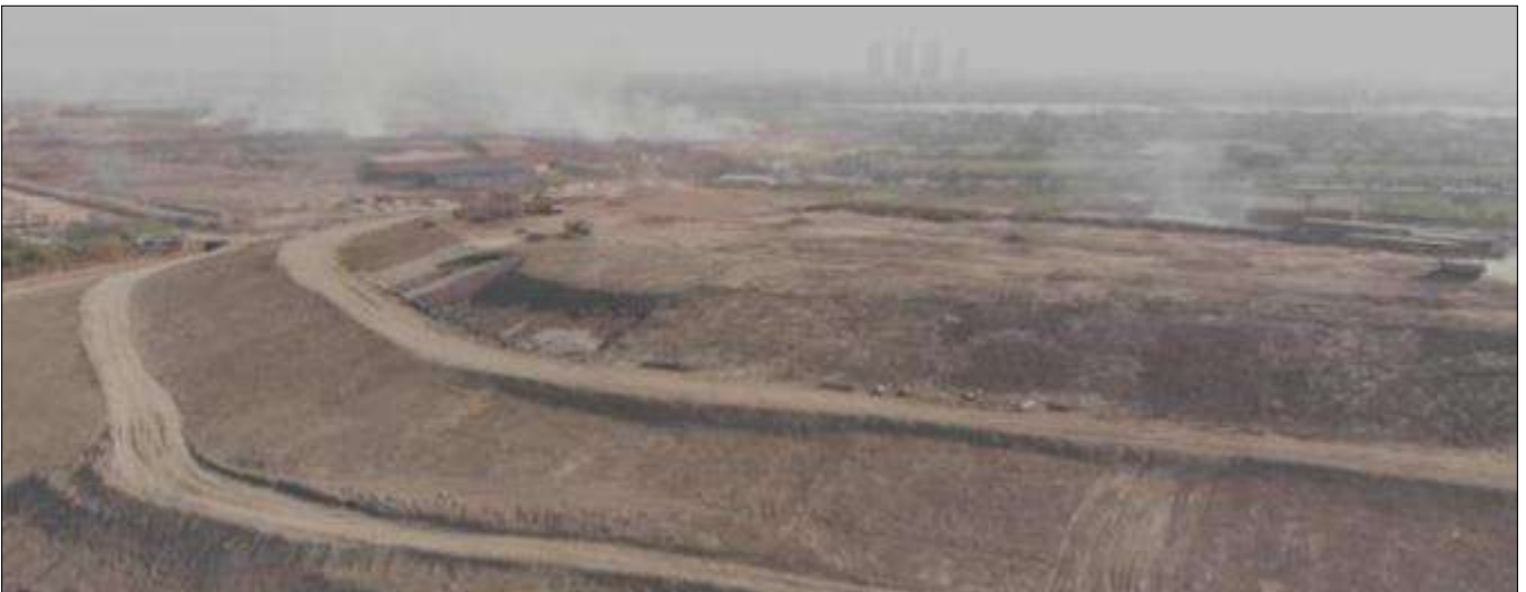
Laying of 450mm thick Vegetative Soil
