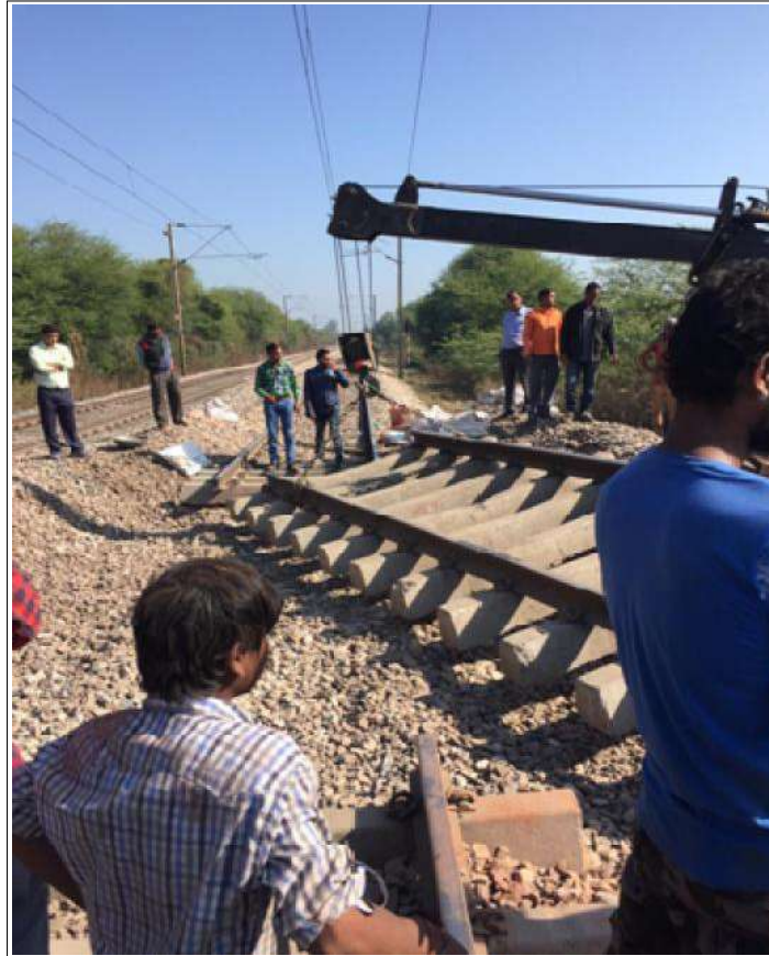
Removing another track panel
