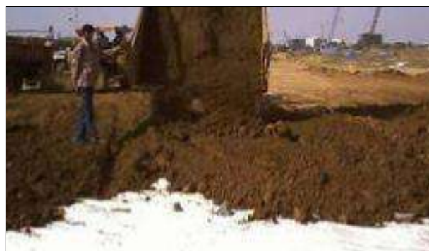
Murum Layer Being placed over Geotextile
