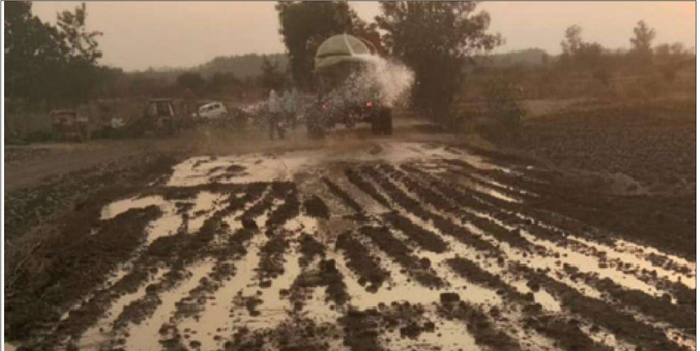
Compaction and preparation of subgrade for laying Techcell Geocell
