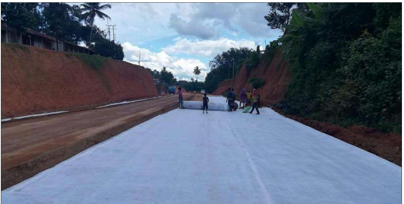
Fig 5 : Unrolling of TechDrain Drainage Composite on the Compacted GSB Layer
