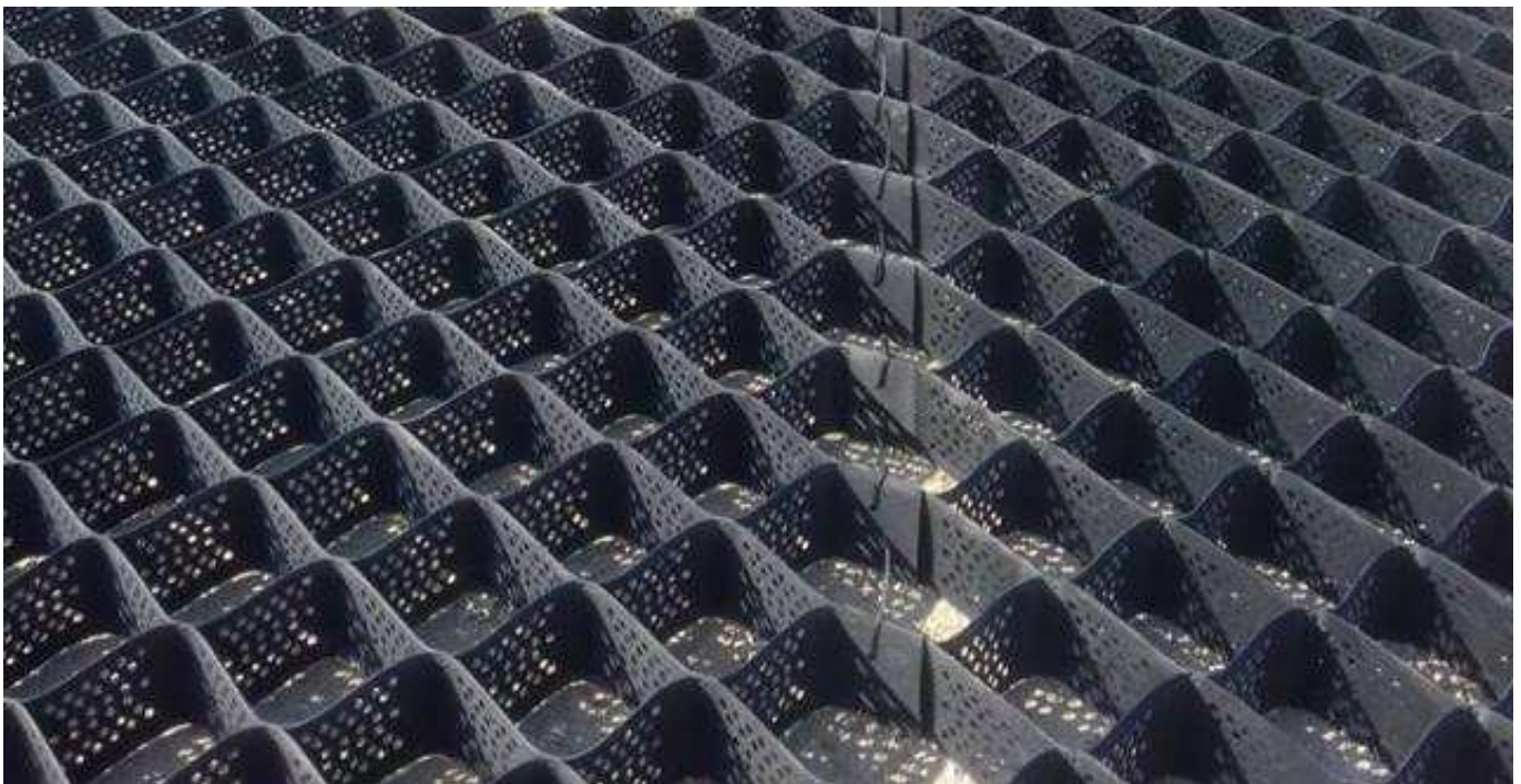
Joining of two Geocells with Cable Ties
