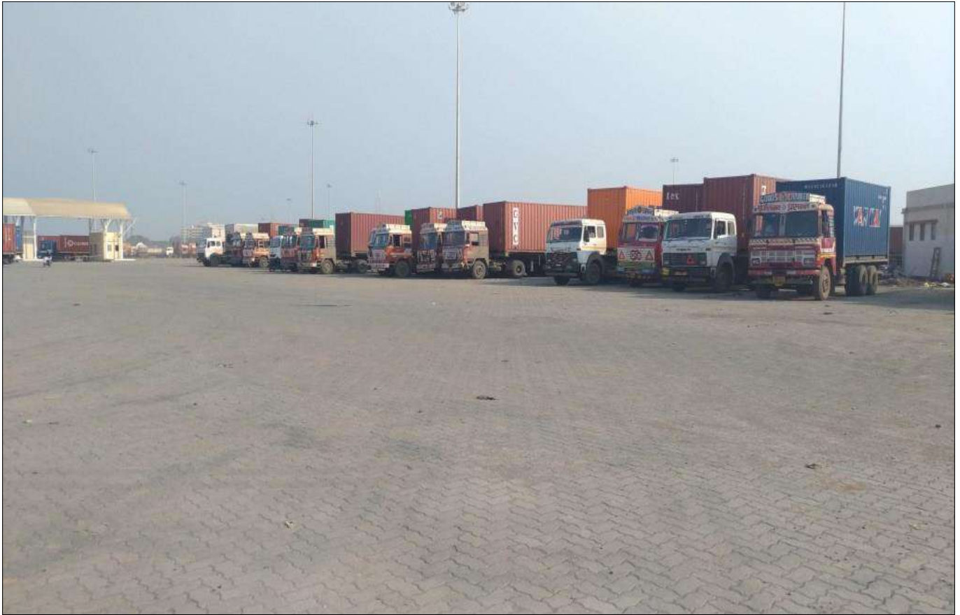
After Completion of Parking Lot
