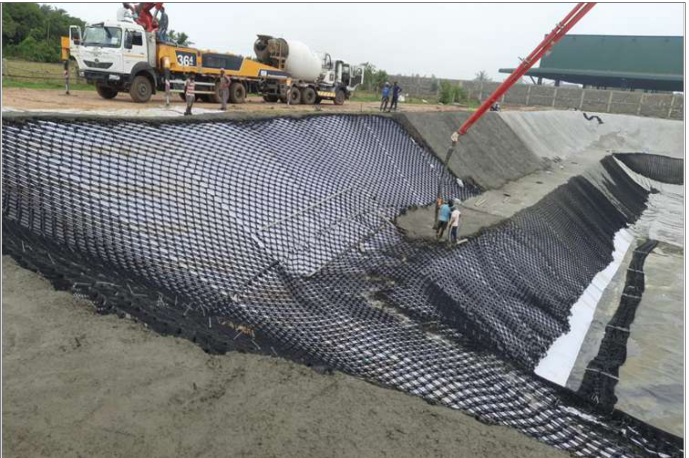
Photo 5 : Filling of concrete on the installed geocell layer
