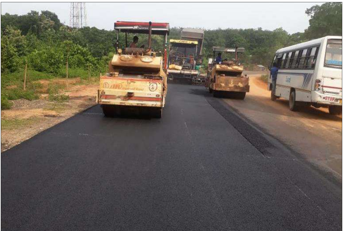
Fig 7 : Laying of Bituminous layers
