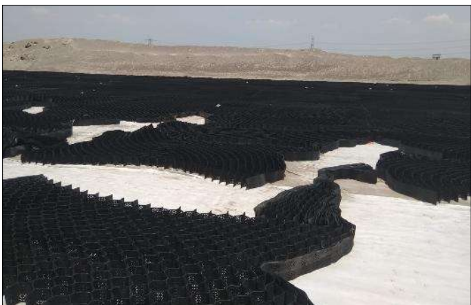
Photo 5 - Laying of Techcell Geocell
