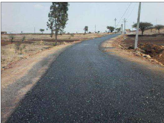
Laying of Seal-Coat
