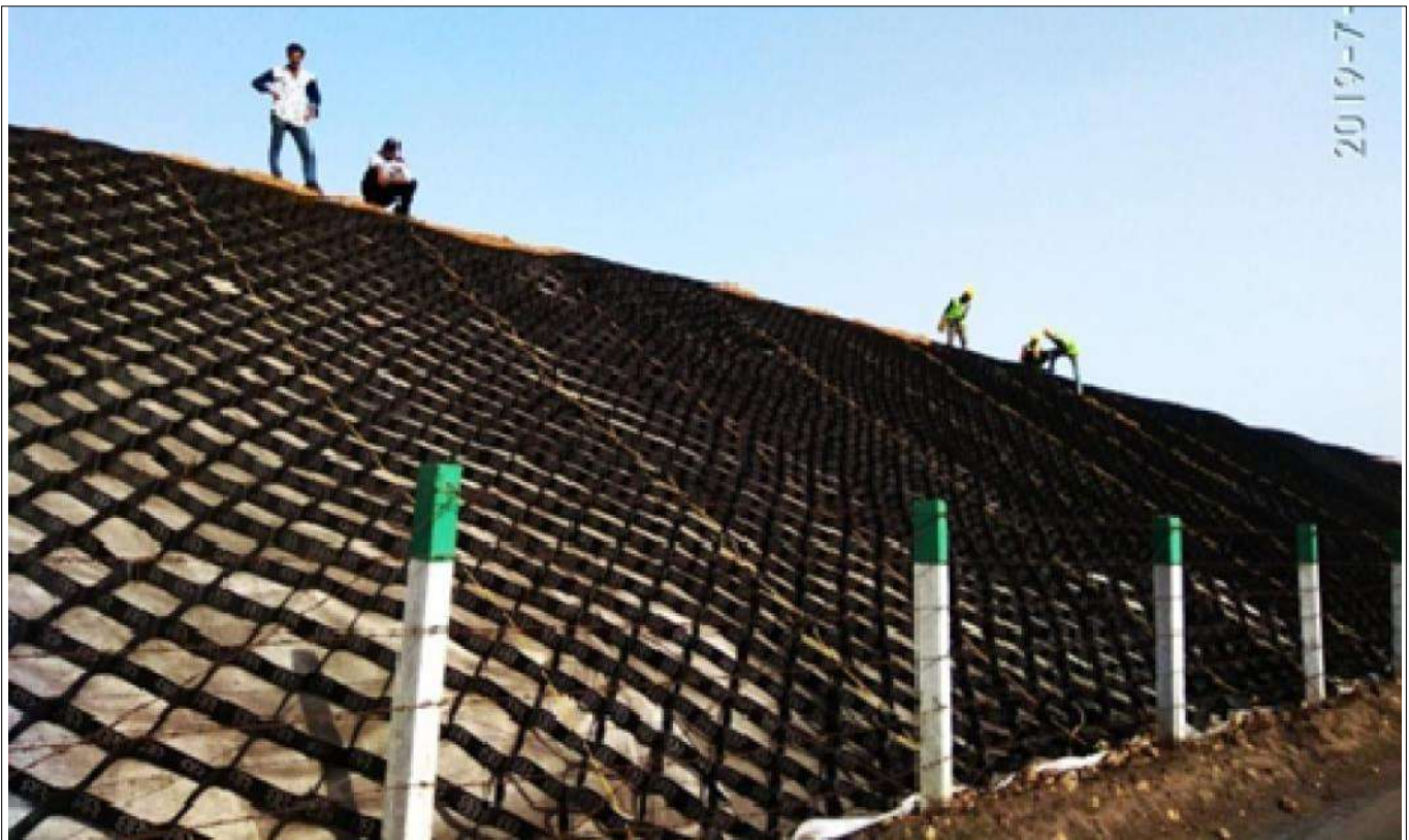
Laying of Techcell Geocell
