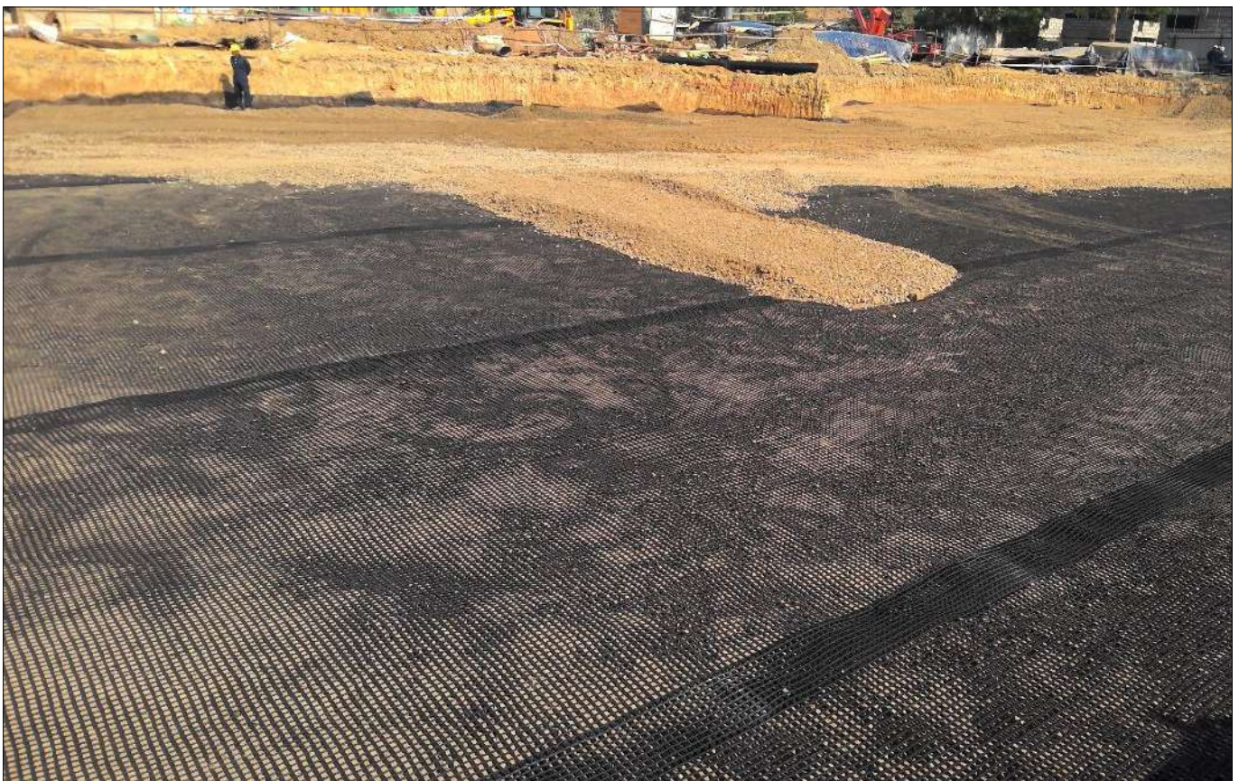
Photo 5 : Spreading of Fill material over geogrid
