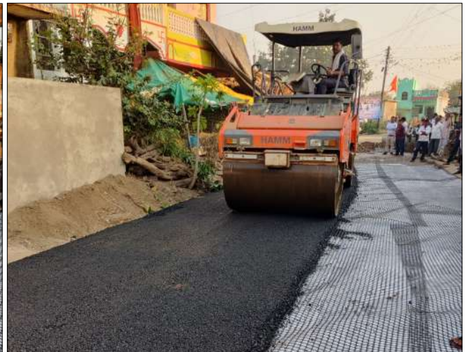
Photo 4 : Compaction
