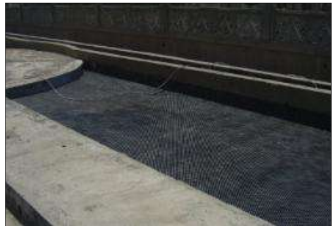
Fig 1 & 2 : Laying of Drain Board
