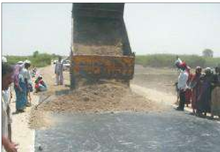
Soft Murrum layer being placed over Geotextile
