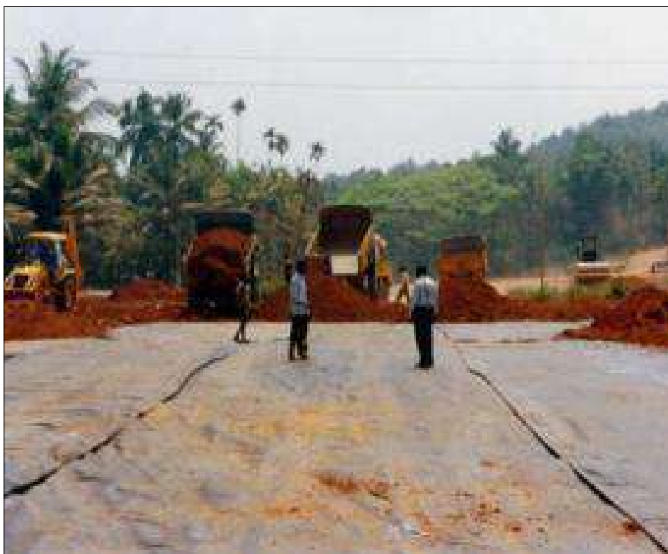
Installation of Techfab TPP 250 Woven Geotextile
