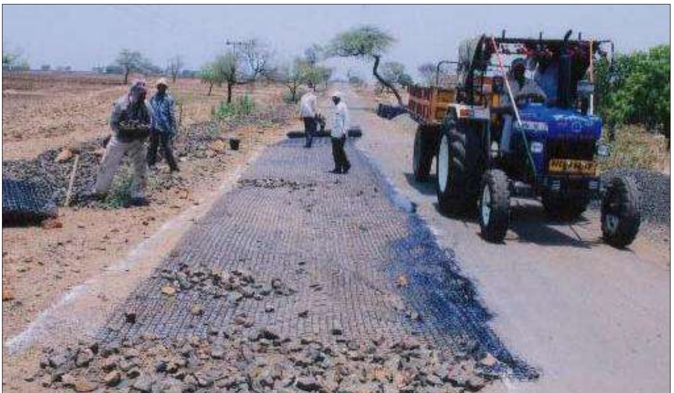
Laying of TechGrid TGB 40
