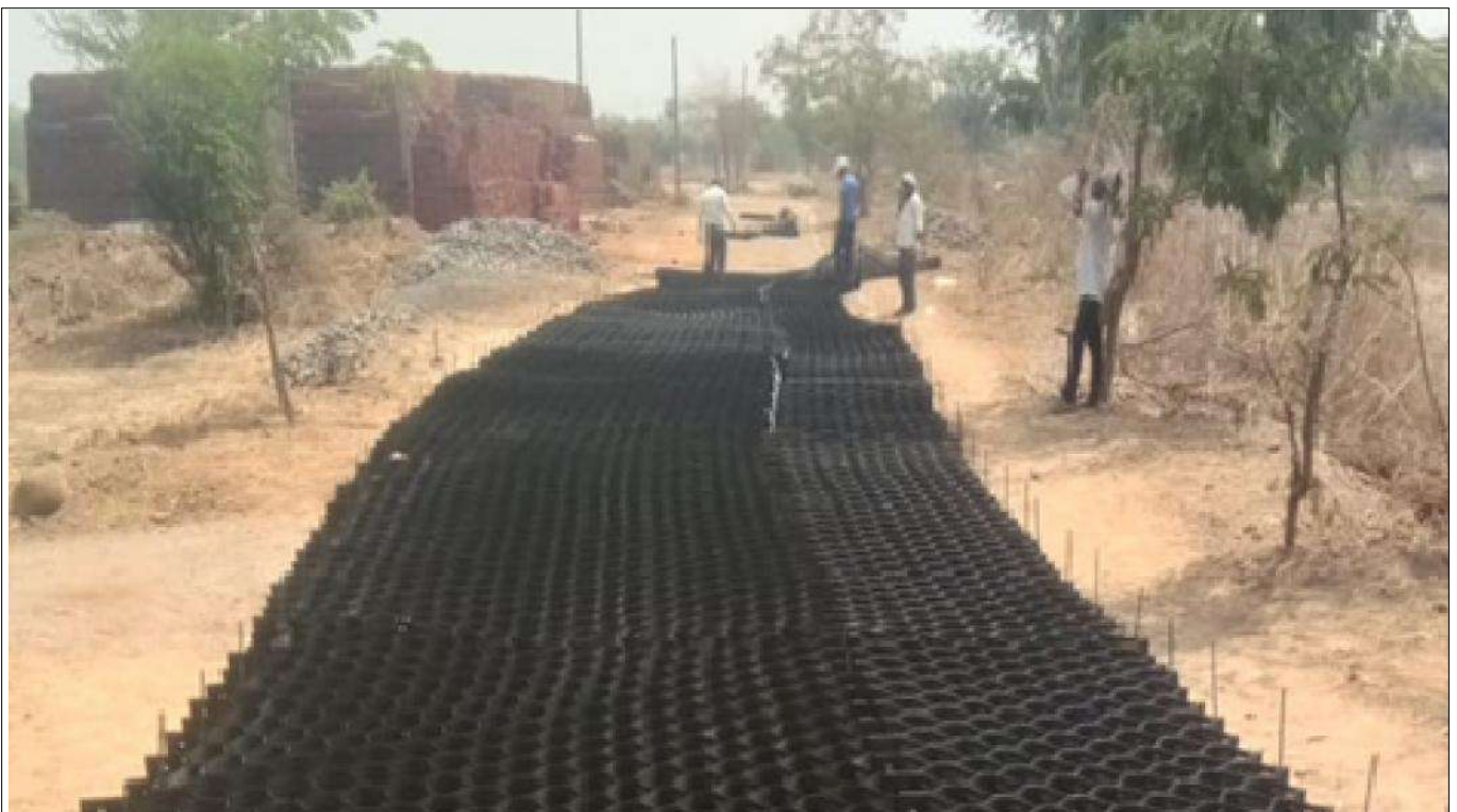
Spreading of TechCell Geocell above the subgrade
