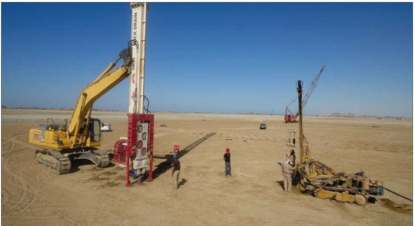
Photo 1 : TechDrain PVD installation starting at site
