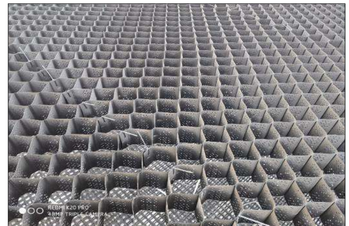
Photo 6 - Laying of Techcell Geocell over TechGrid Geogrid
