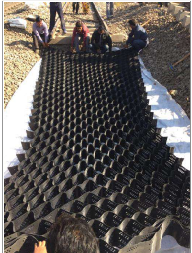
Laying of Techcell Geocell in Progress
