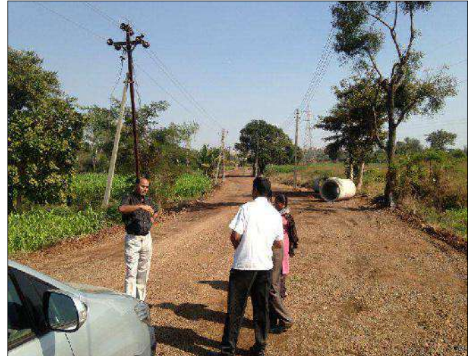
Checking of Subgrade – Exe. Engineer
