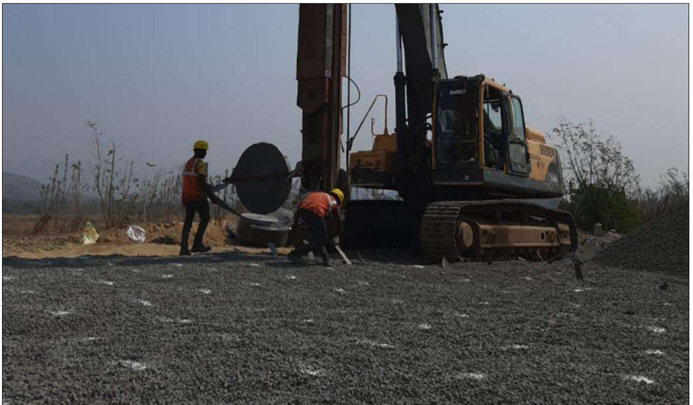
Techdrain PVD Installation in progress Overview
