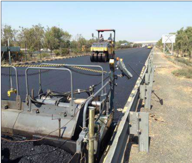
Overlay Placement above TechPave
