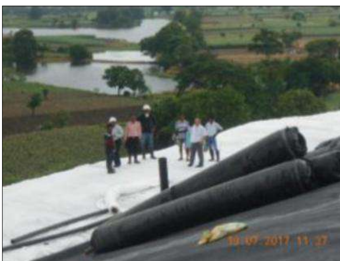
Laying of 1.5mm Both side Textured HDPE Liner
