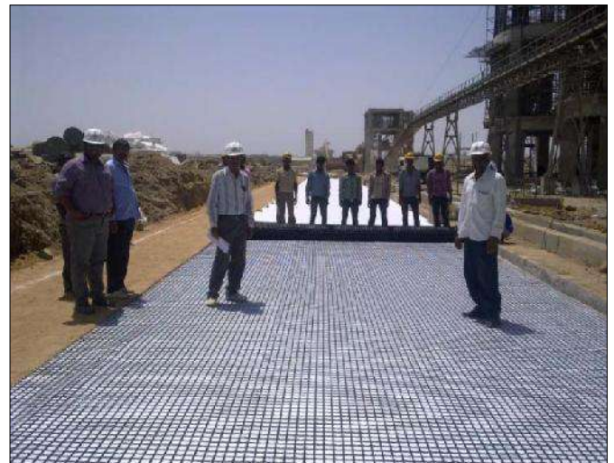
Fig 5 : Laying of TFB-40 over TechGeo PR-20
