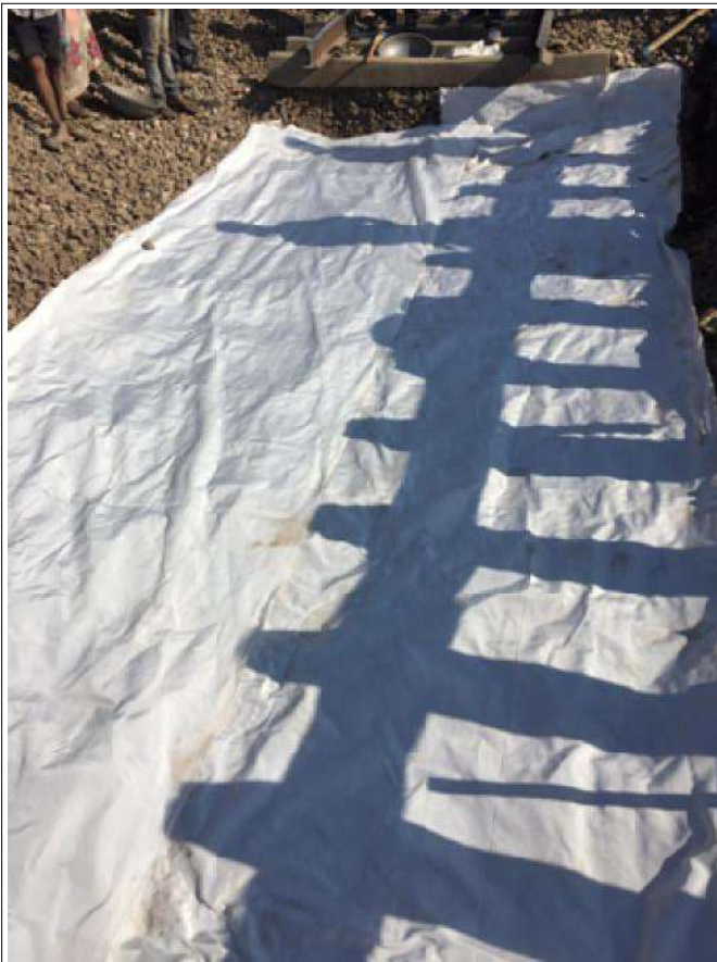
Laying of Woven Geotextile
