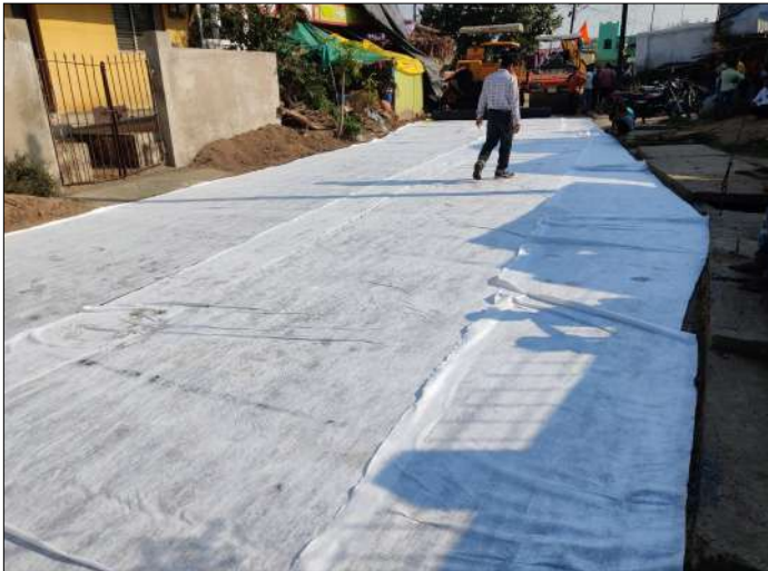
Photo 1 : Laying of TechPave C040
