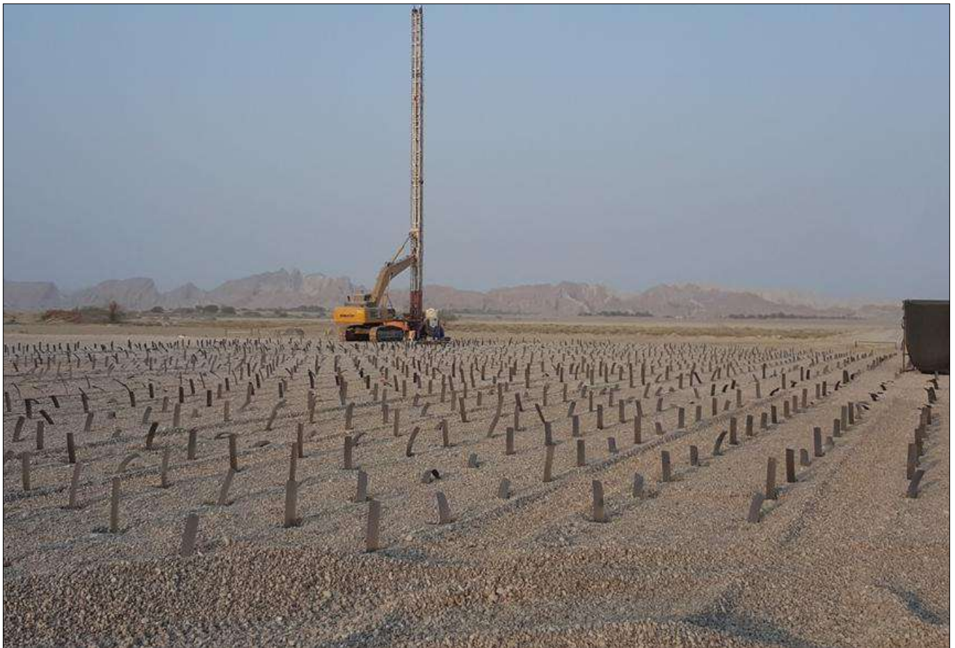
Photo 4 - TechDrain PVD installation is in progress
