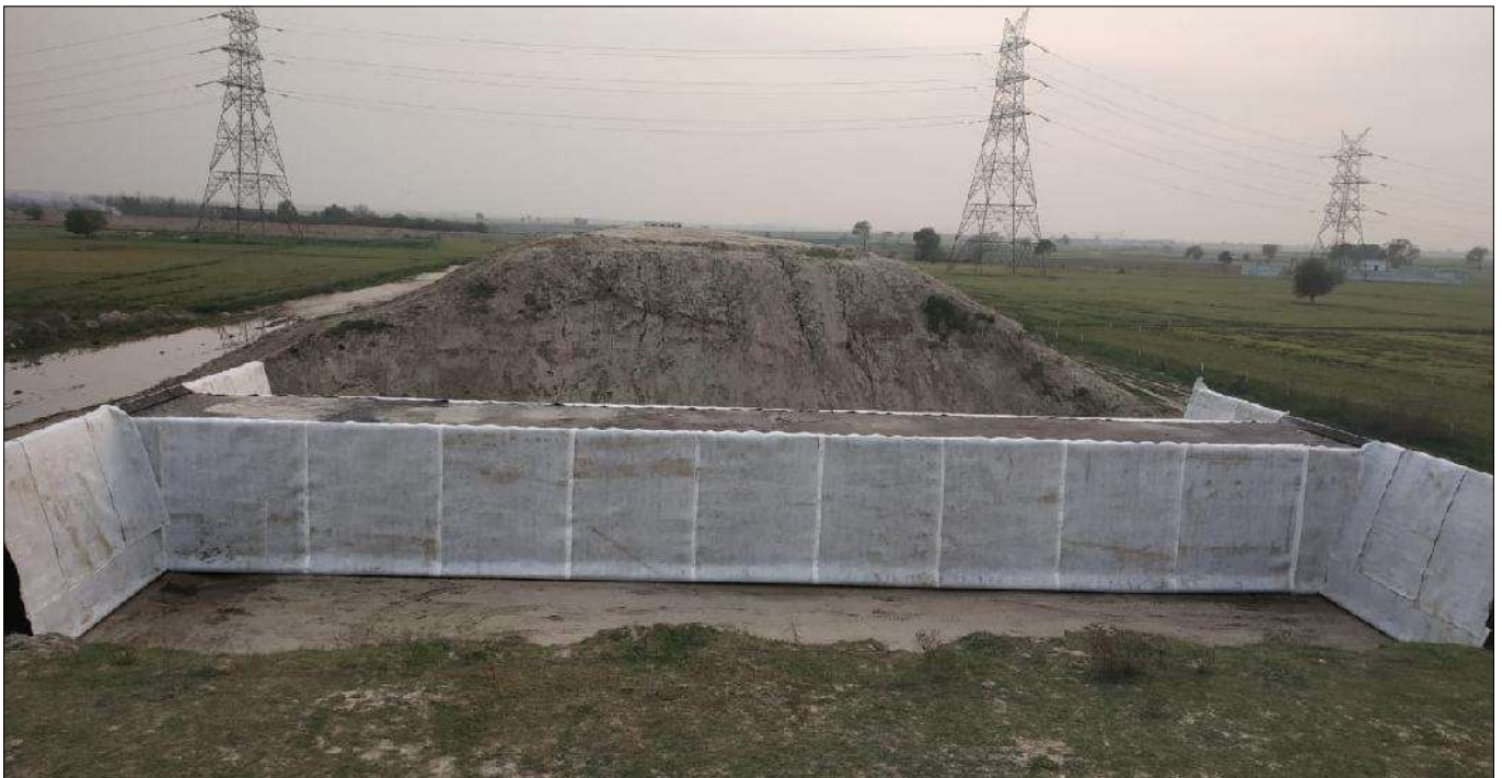
After Installation of TFI Drainage Geocomposite - TechDrains
