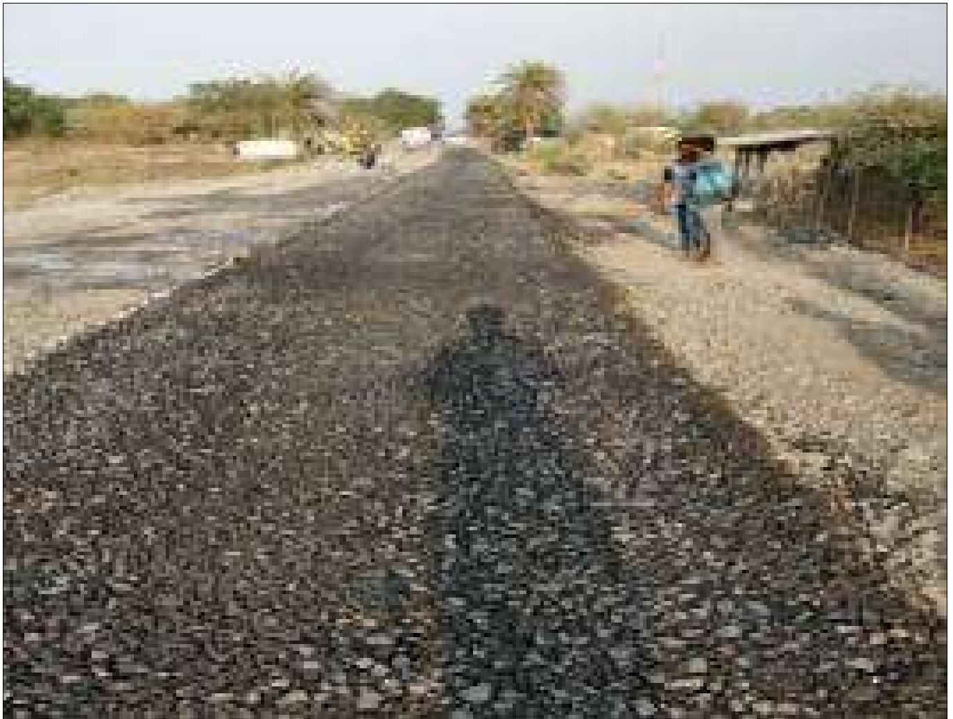
WMM compaction in progress
