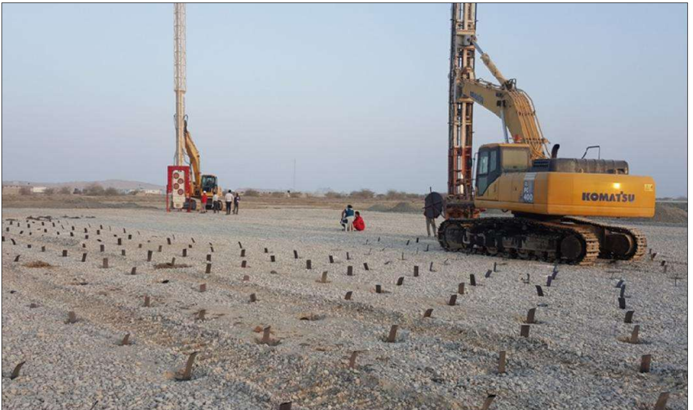
Photo 2&3 - TechDrain PVD installation is in progress
