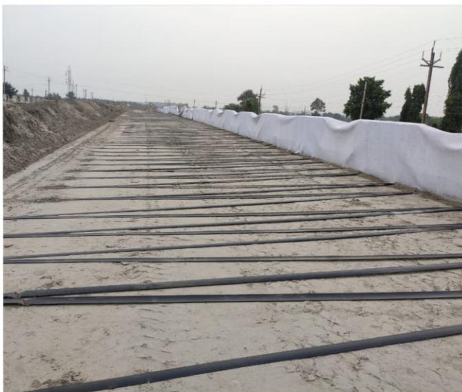
Reinforced Soil Wall during construction (TechStrap)
