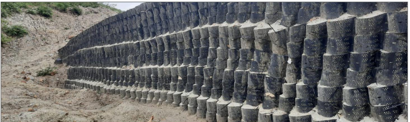
Reinforced Soil Walls with TechCell Geocell Facing
