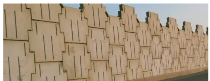
Reinforced Soil Wall during construction (TechStrap)
