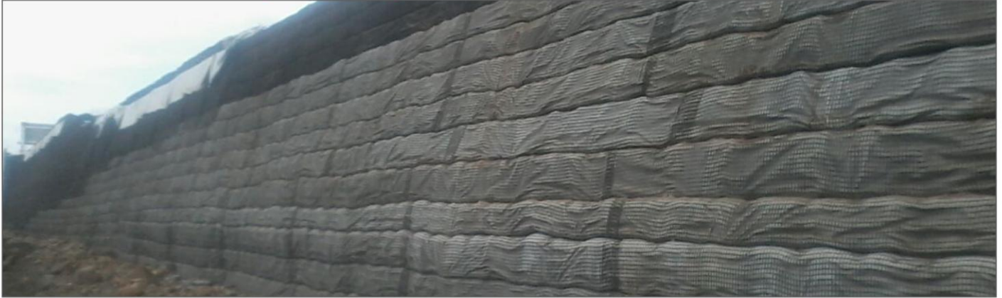
Reinforced Soil Walls with Wrap Around Facing
