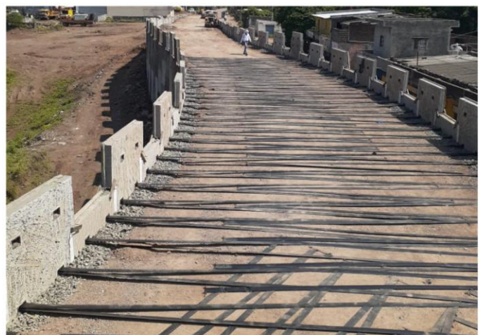
Reinforced Soil Wall during construction (TechStrap)
