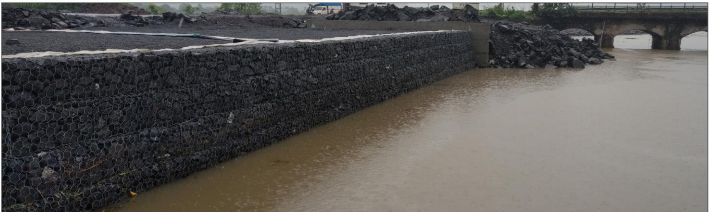
Reinforced Soil Walls with Gabion Facing
