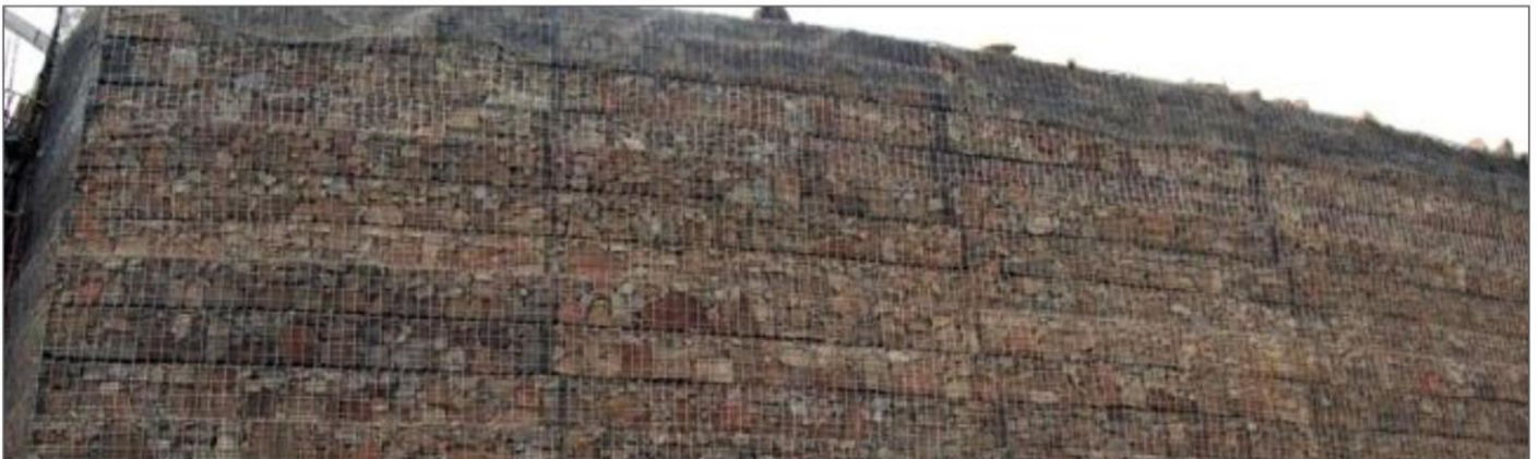
Reinforced Soil Walls with Welded Wire Mesh Facing
