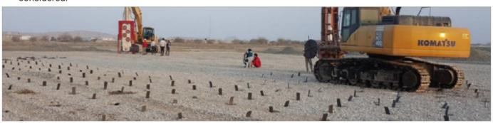
Ground improvement using PVDs is a very good example of the observational method of design in geotechnical engineering. At most sites, the soil strata may show appreciable variability and there are significant difficulties in accurate determination of compressibility characteristics of soil. Hence, the magnitude and rate of settlements predicted in the design phase are only approximate estimates.
