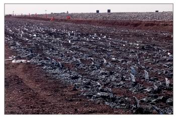
Acceleration of consolidation using PVDs is one of the most cost-effective methods of ground improvement for relatively weak and compressible silts and clays. PVDs do not reduce the settlements, but only accelerates the settlement. The idea is to minimize the post construction settlement. As the soil consolidates, the shear strength also increases.
