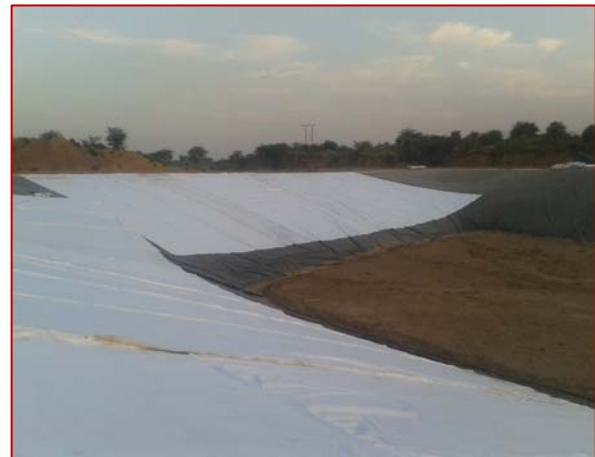
TechGeo laid over the Side Slopes of Landfill
