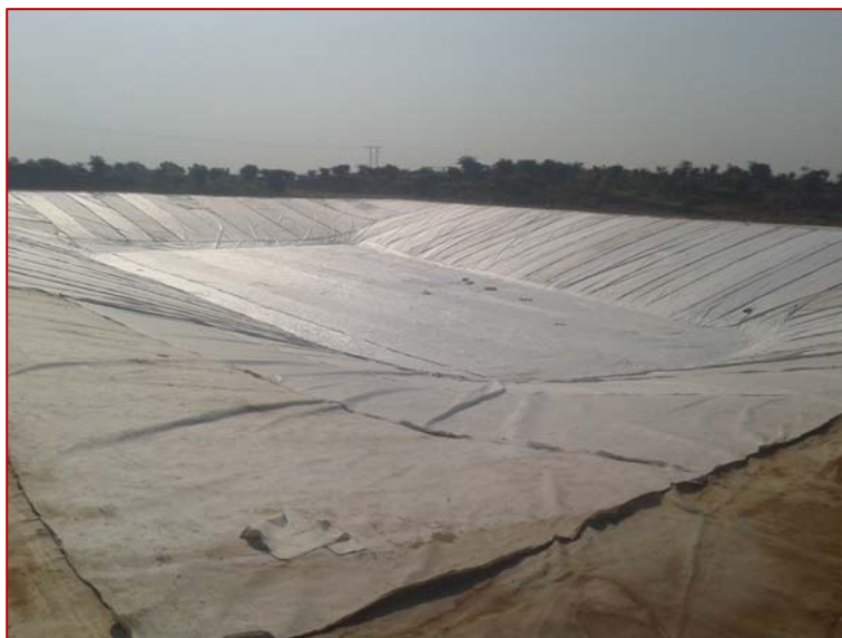
TechGeo Laying Completed at Landfill Site
