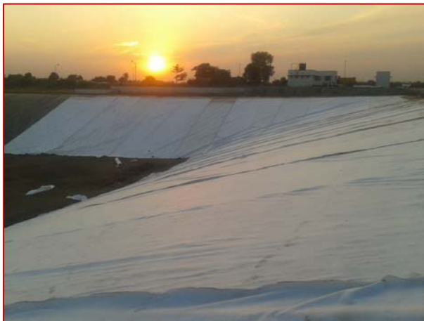
TechGeo laid over the Side Slopes of Landfill
