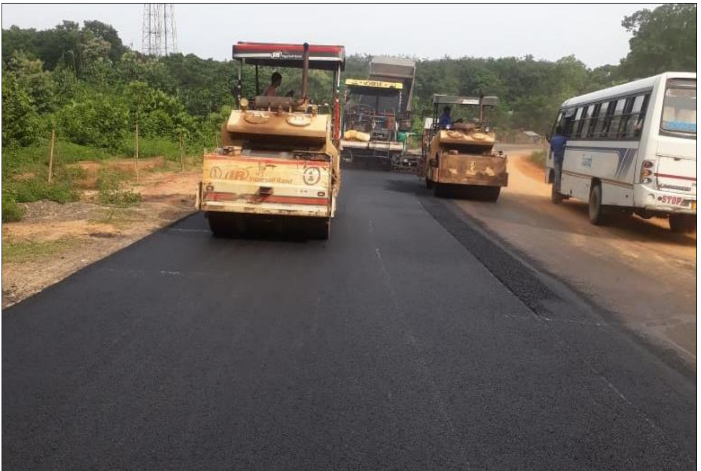
Fig 7 : Laying of Bituminous layers
