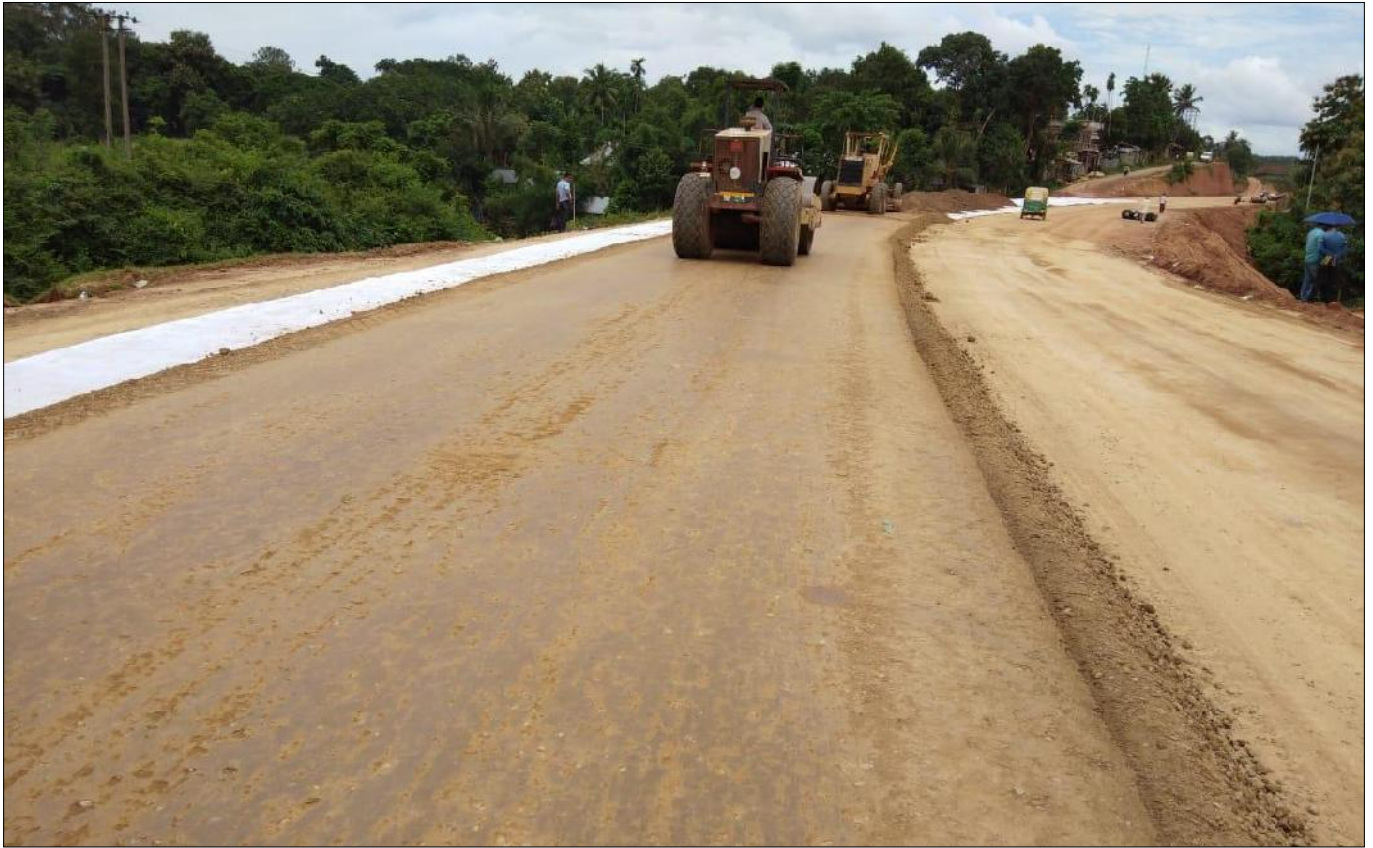
Fig 6 : Spreading and Compaction of base course on the Drainage Composite
