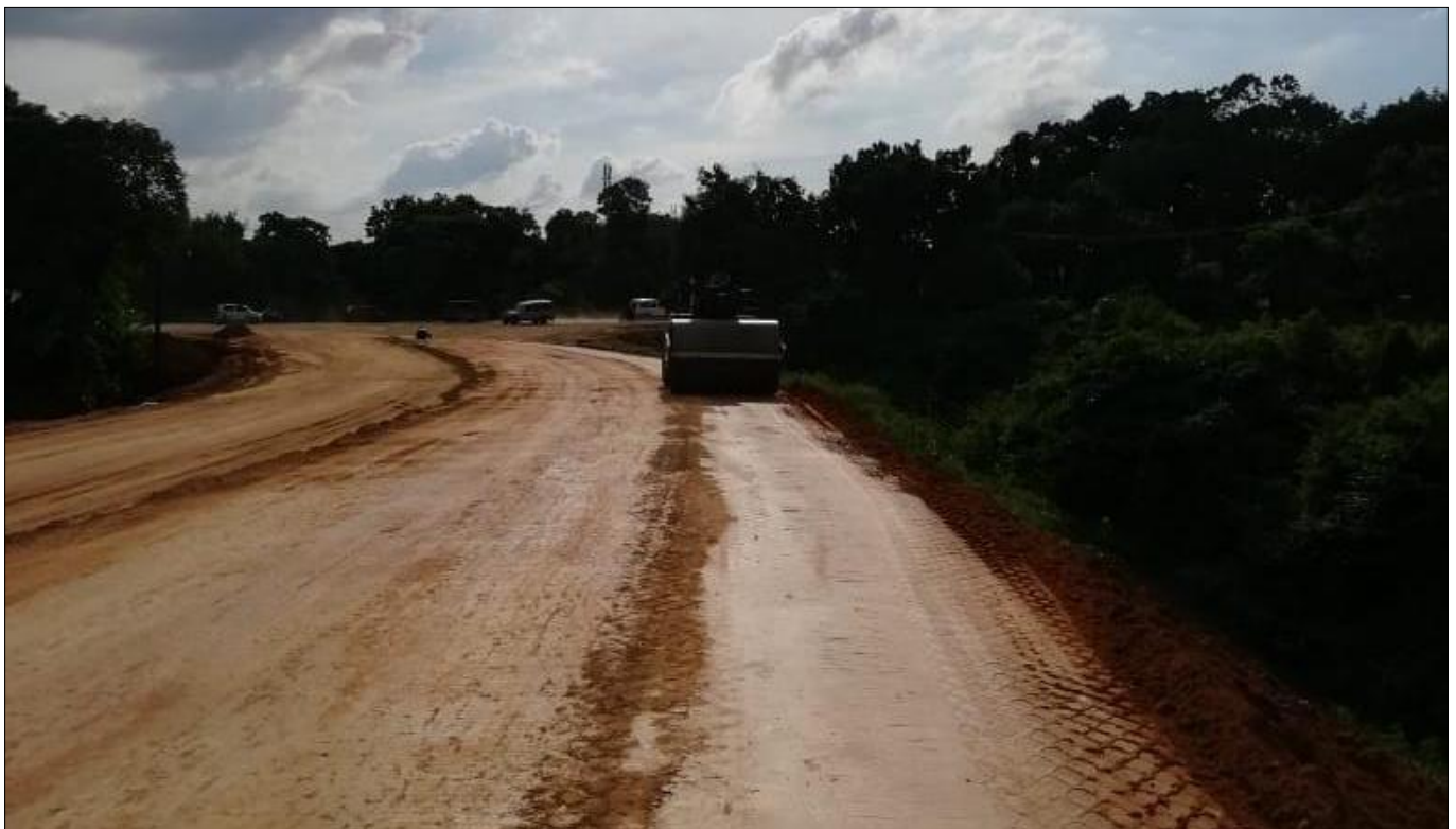
Fig 1 : Preparation of subgrade before laying granular layers.
