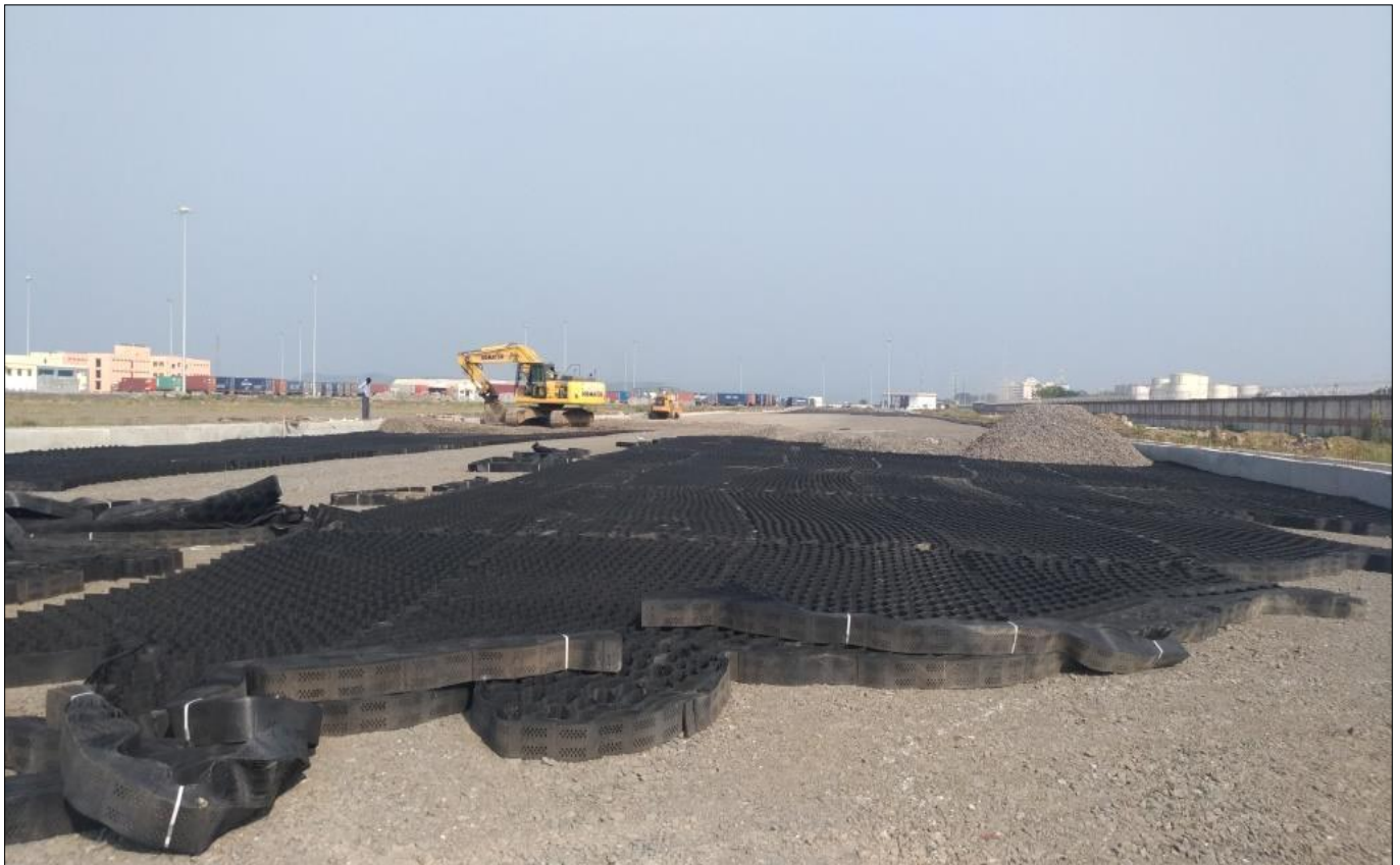
Laying of Techcell Geocell in progress
