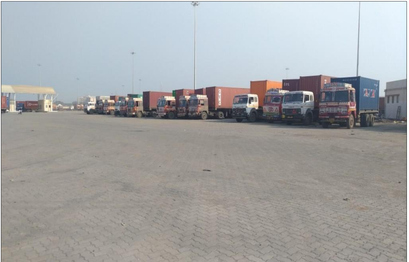
After Completion of Parking Lot
