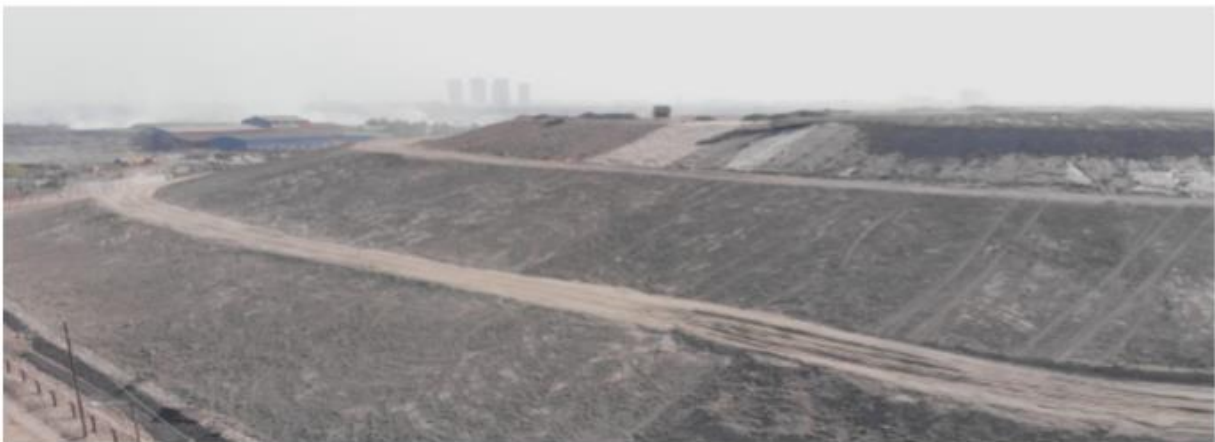
(Laying of 500mm thk. Non-contaminated Soil)
