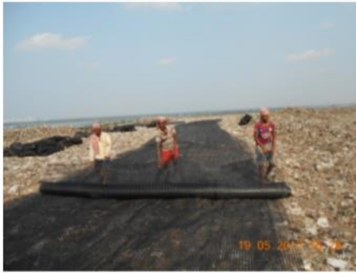
(Laying of Geo-grid)
