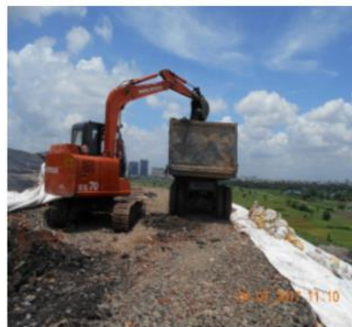
(Laying of Geo-Textile)
