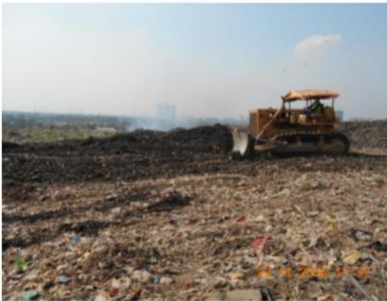
(Leveling of waste by Dozer)
