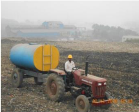
(Maintaining moisture content by sprinkling water)
