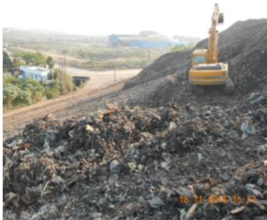
(Excavation, Loading & Reshaping of waste)
