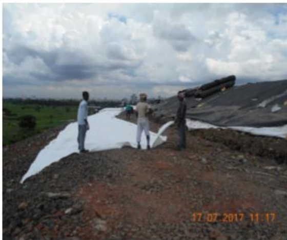
(Laying of Geo-Textile)
