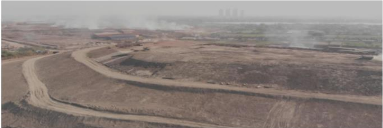
(Laying of 450mm thk. Vegetative Soil)
