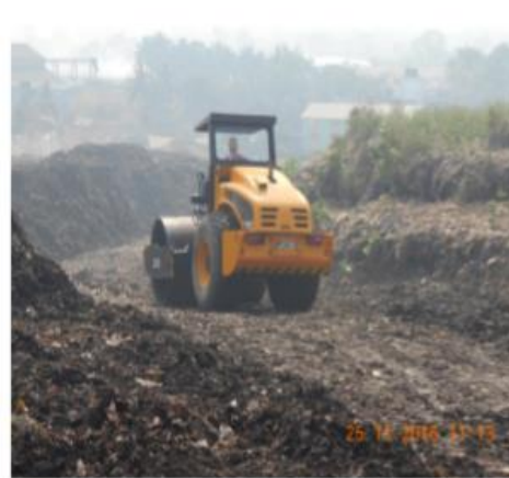
(Compaction of Waste by Vibratory Roller)
