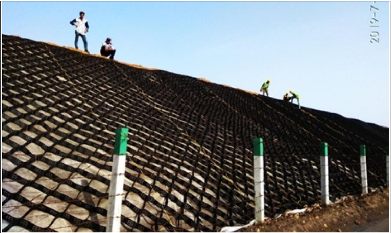
Laying of Techcell Geocell
