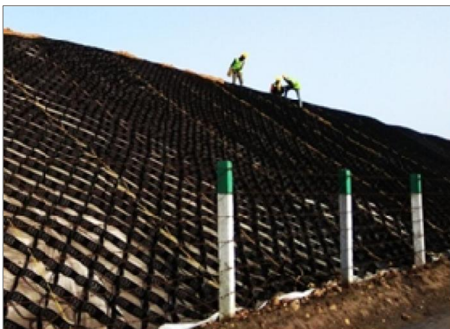
Laying of Techcell Geocell
