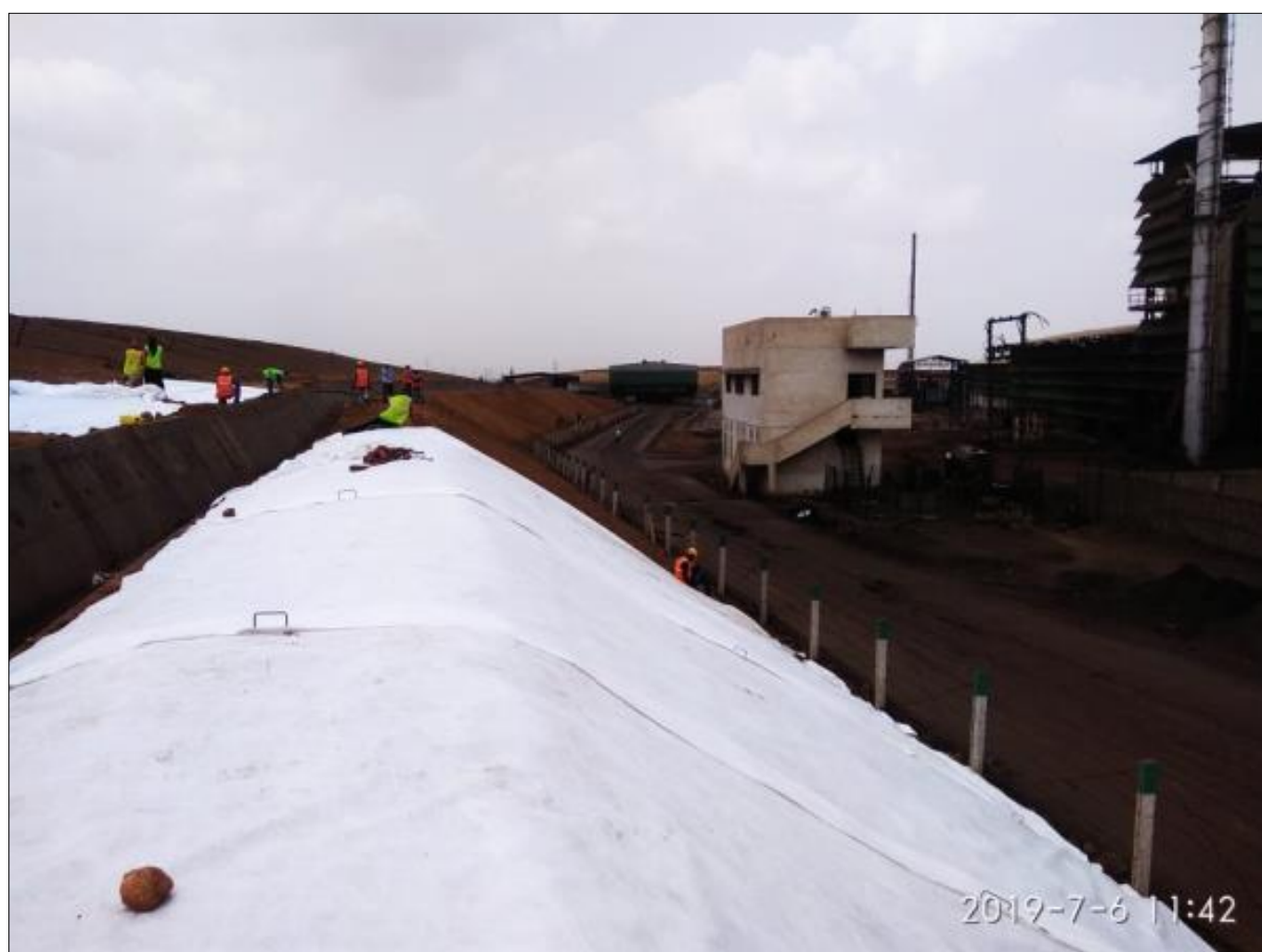
Laying of TechGeo Nonwoven geotextile
