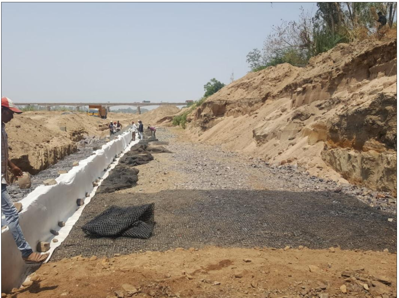
During Construction Photograph
