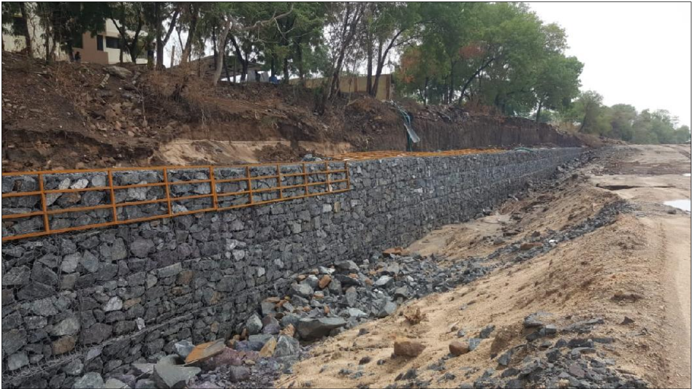
During Construction Photograph
