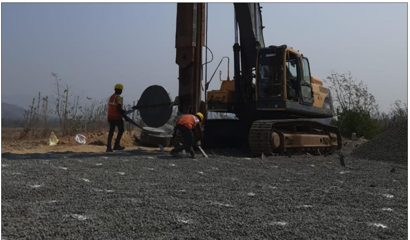
Techdrain PVD Installation in progress Overview
