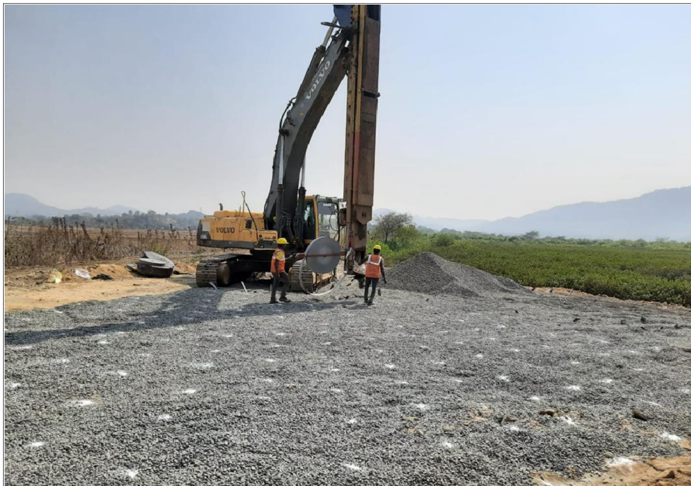
Marking done as per design for Techdrain PVD Installation
