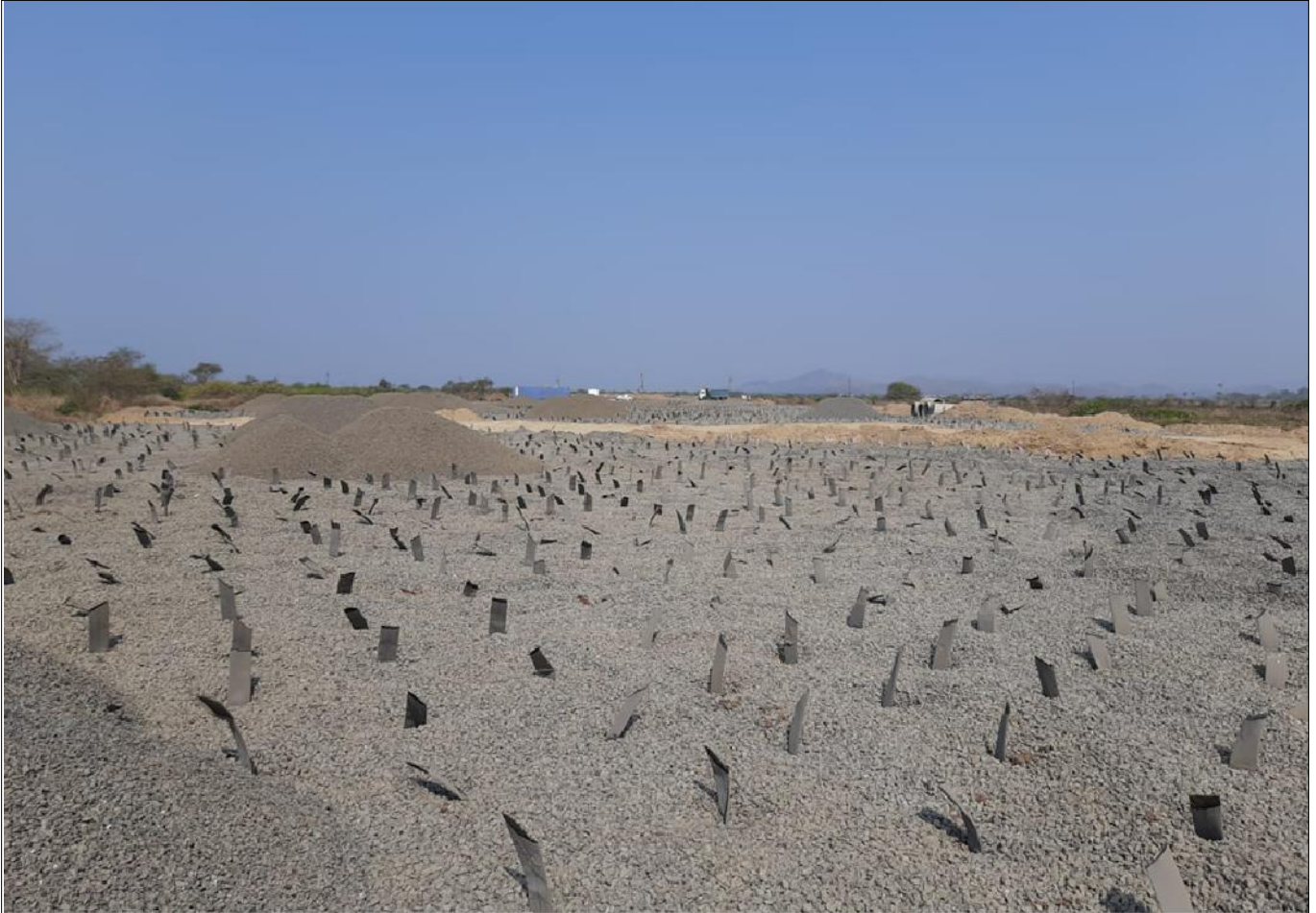
TechDrain PVD installed with preloading in progress
