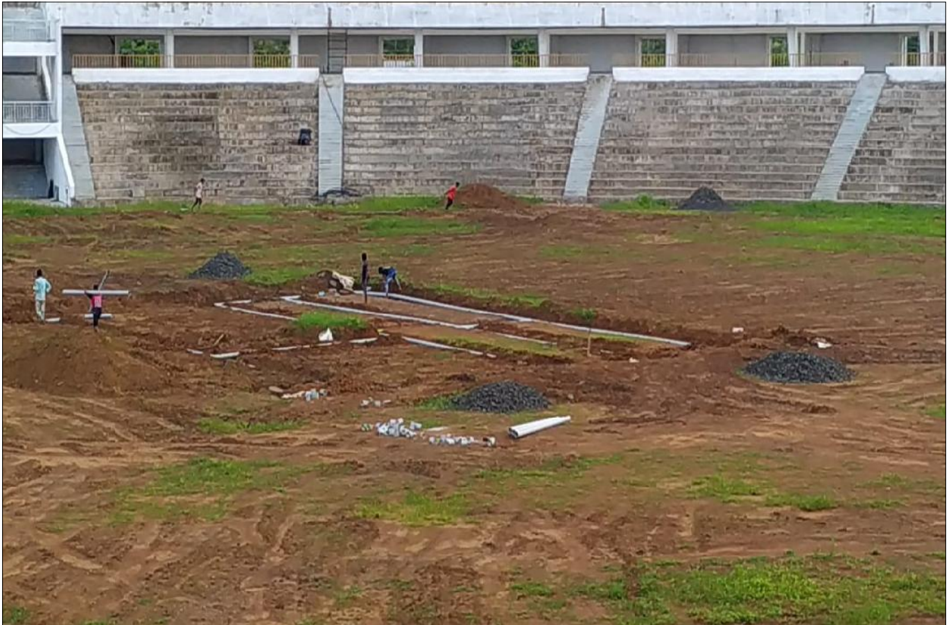
Drainage composite installation and Pipe drain laid
