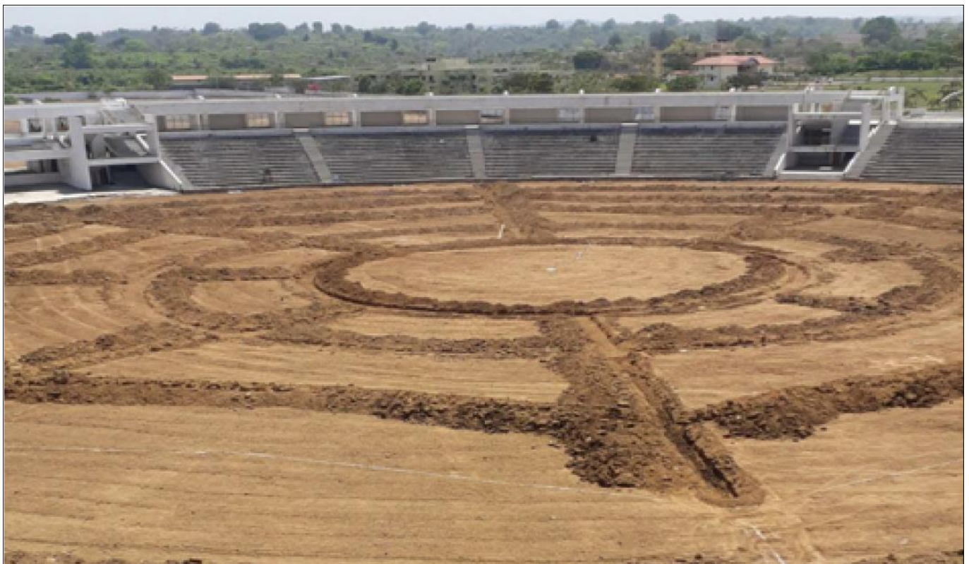
Excavation in progress for radial pipe drain
