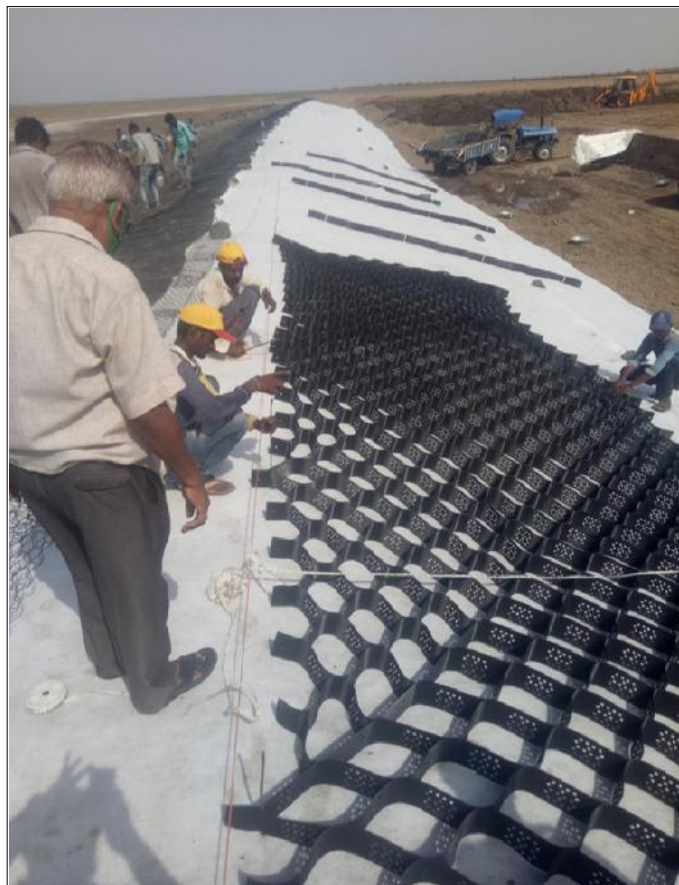
Techcell Geocell installation in progress
