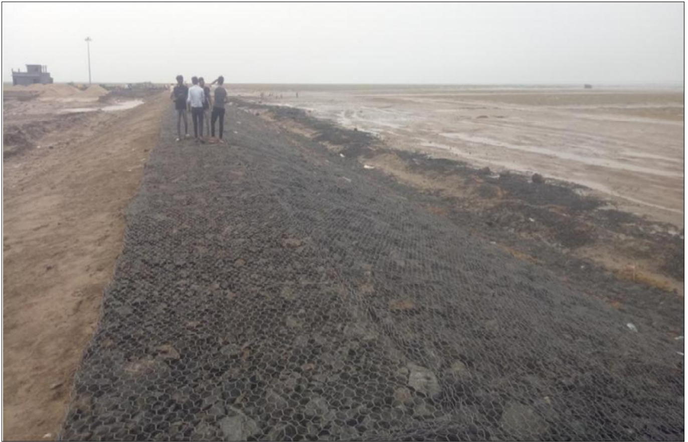
On the sea side slope - Gabion Mattress laying in progress
