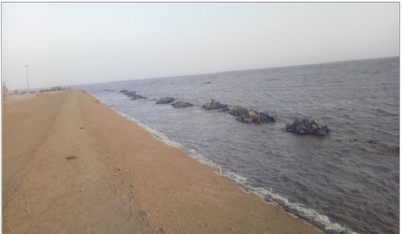
Prepared Embankment with low tide
