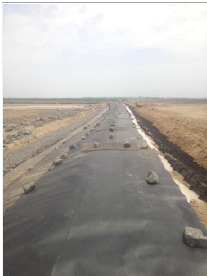
Geomembrane & Nonwoven geotextile layer is laid and Gabion Mattress installation in progress
