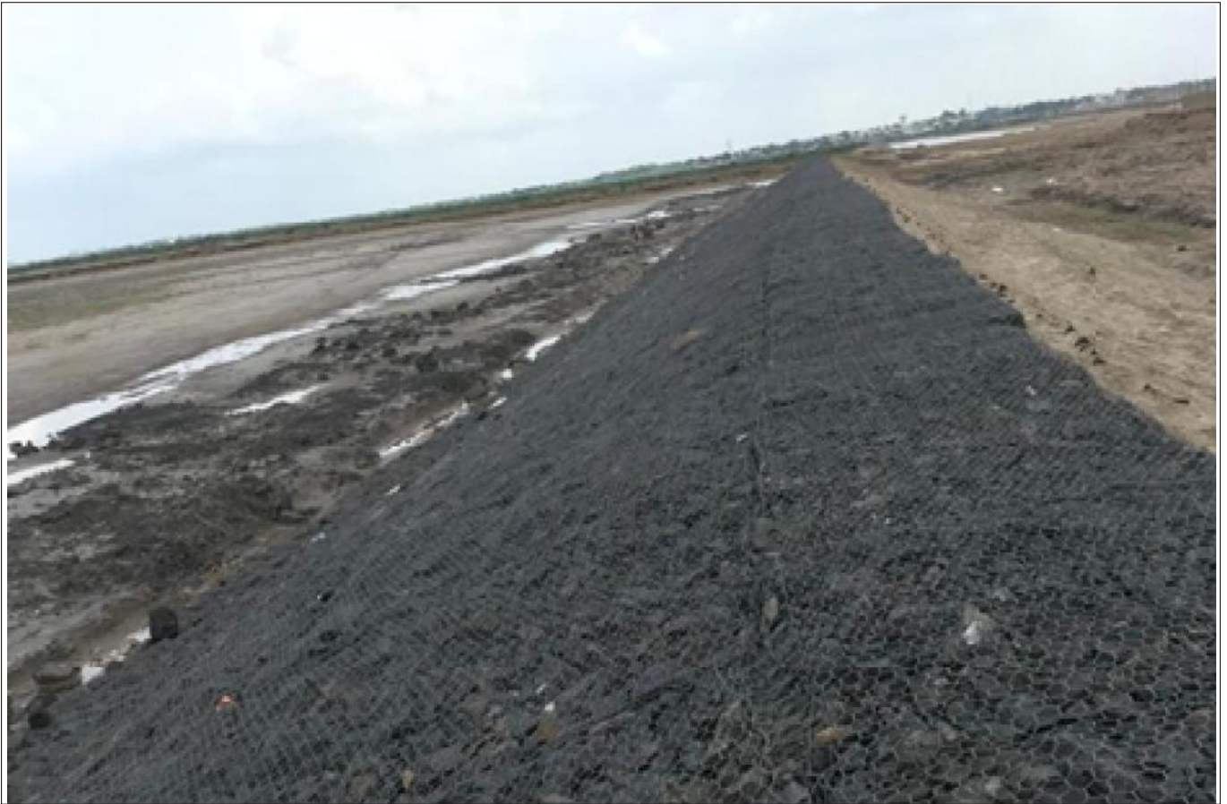
Sea side slope with Metal Gabion Mattress
